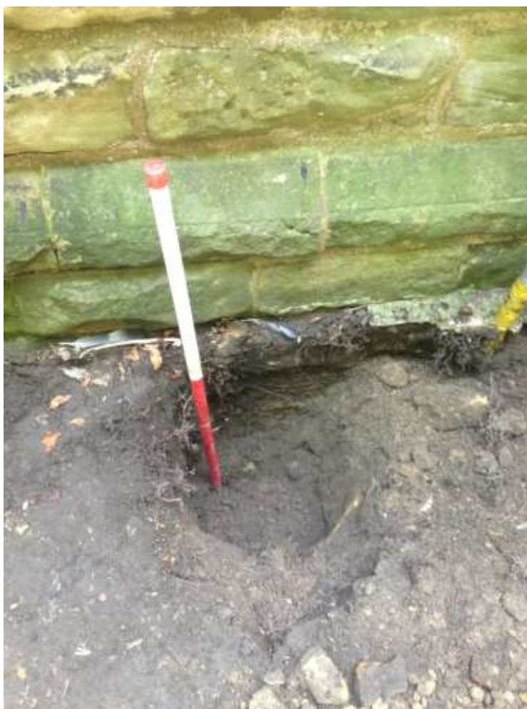
Figure 3. Test pit 1 against the north wall of St Thomas Church
