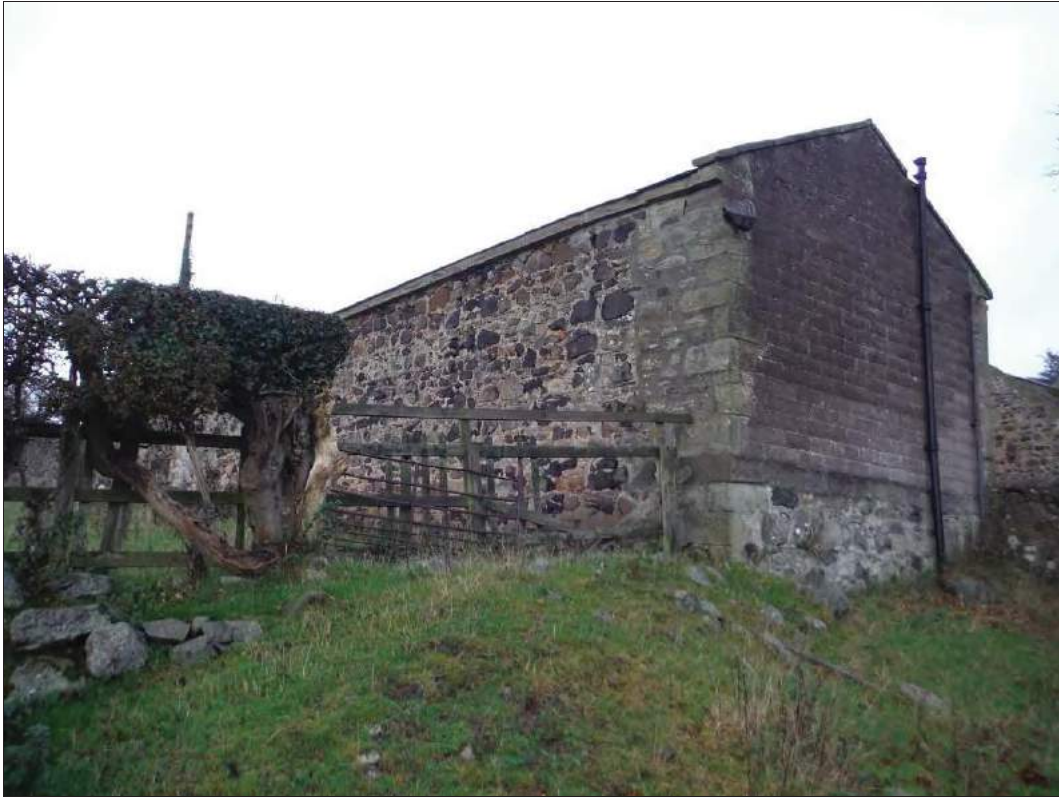
Figure 35: East elevation of the cart shed showing rebuilt blockwork walling.
