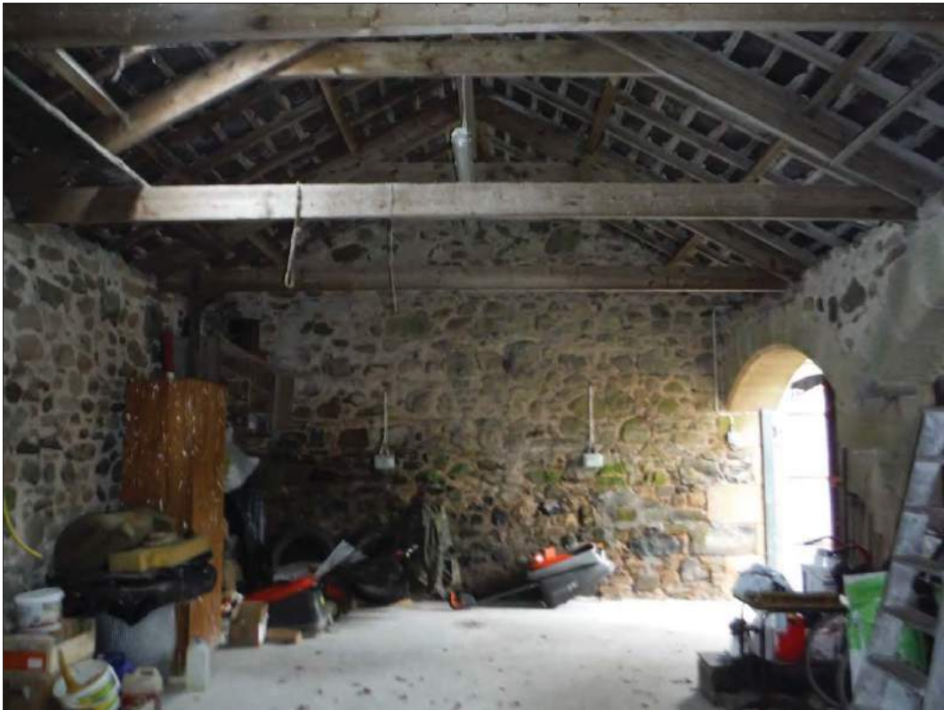
Figure 37: Interior of the cart shed, looking west.
