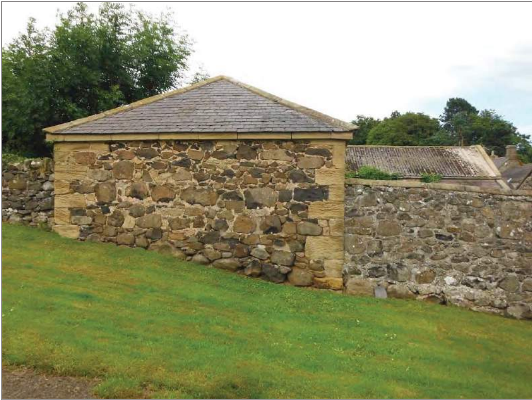
Figure 27: South elevation of the shelter shed with adjoining yard walls.
