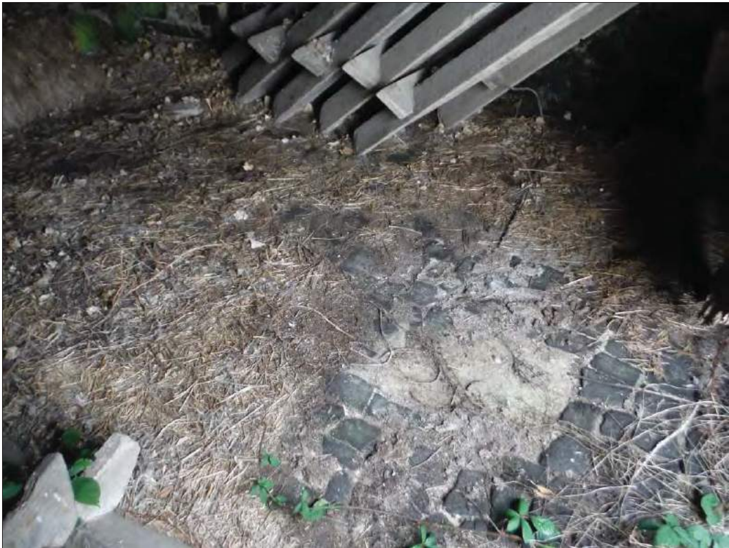
Figure 31: Surviving cobbled floor within the northern arches of the shelter shed.
