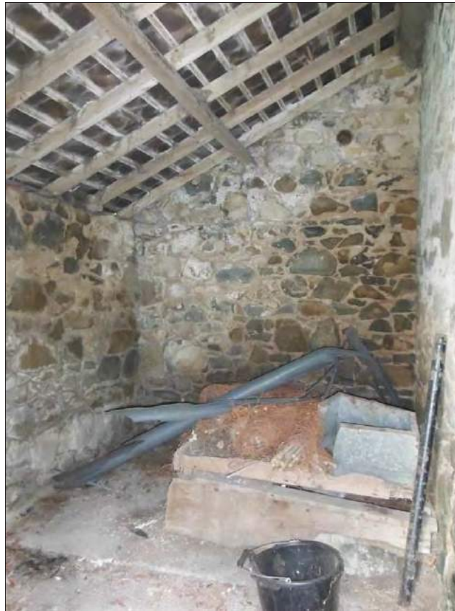
Figure 25: Interior of the possible turnip store, looking west.
