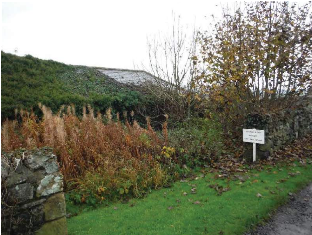
Figure 15: View of the overgrown western side of the farm buildings and attached yards to the south-west of Greensfield Farmhouse, looking south-east.
