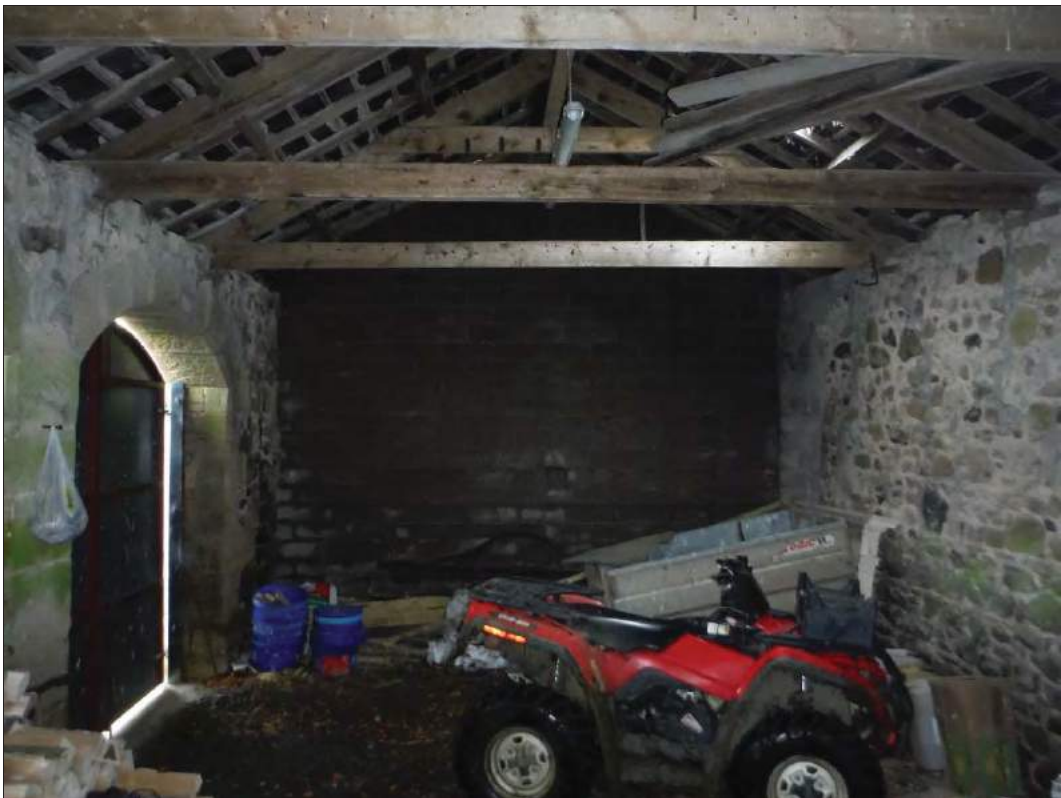
Figure 38: Interior of the cart shed, looking east.
