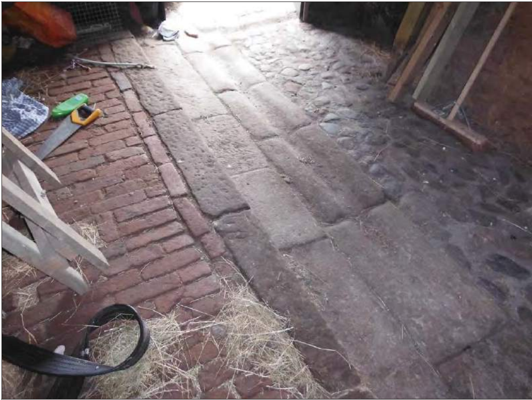
Figure 23: Original, or early, floor at the east end of the cow house showing a brick floor to the stalls, a stone drain and a cobbled feeding passage.
