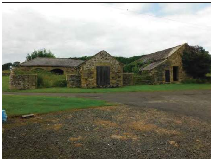
View of the eastern frontage of the Shelter Sheds and foldyards.
