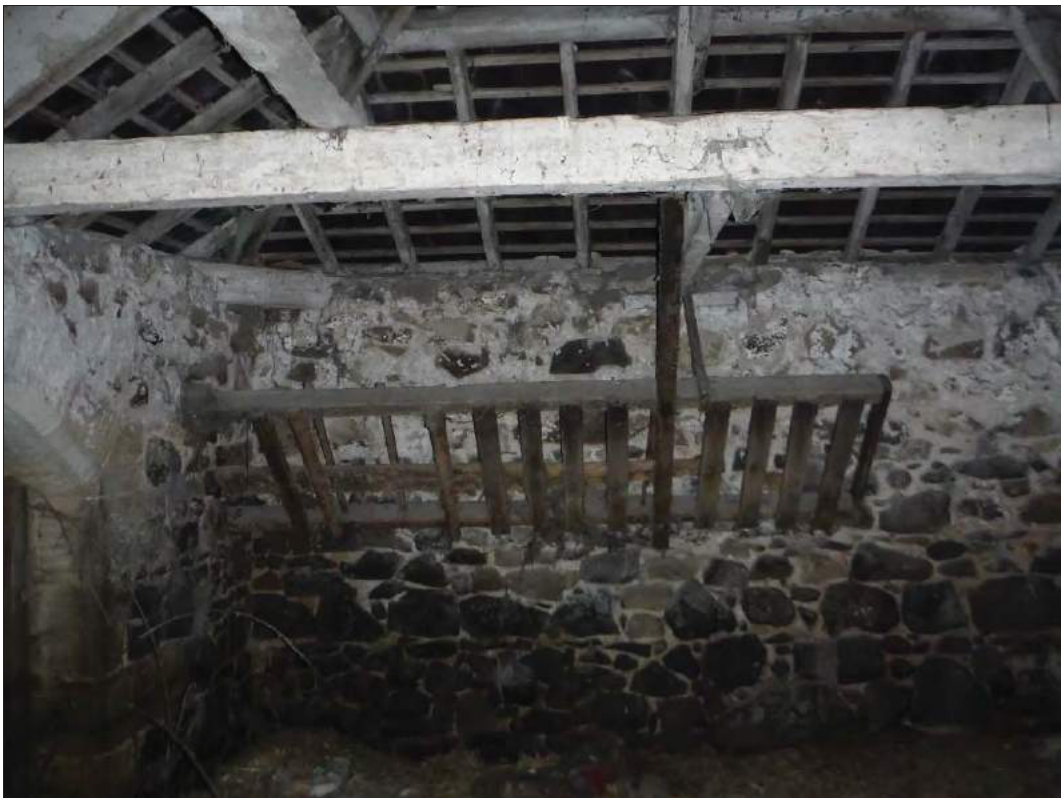
Figure 30: Inserted timber hayrack on the southern wall of the shelter shed.
