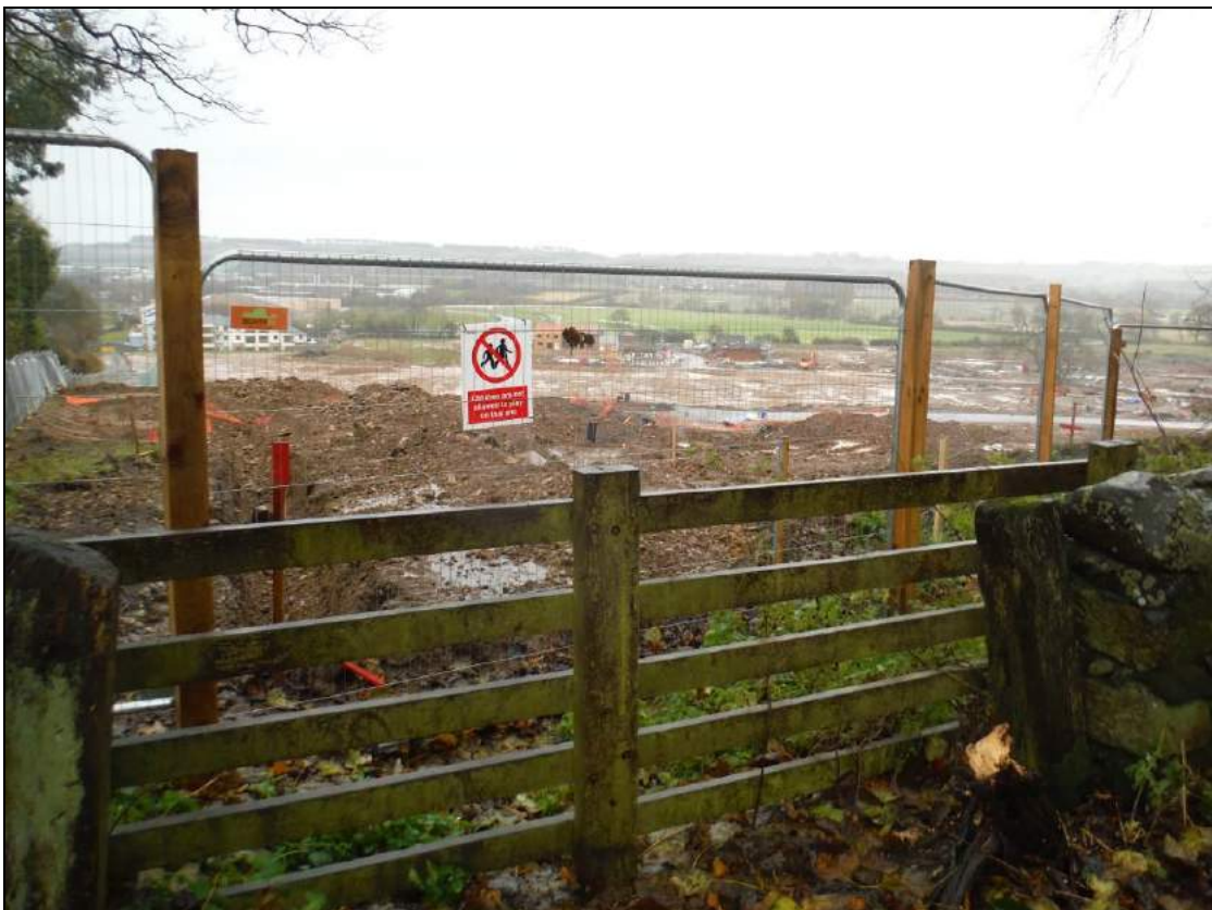
Figure 4. Looking towards the construction site to the east of the PDA.
