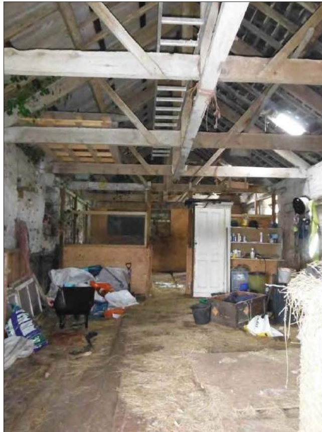
Figure 21: Interior view of the cowhouse, looking west.
