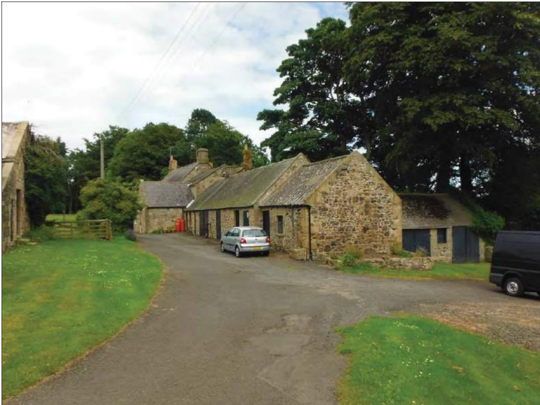
Figure 39: View of the Listed farmhouse and attached stables at Greensfield Farm with the Listed cowhouse to the left of the photograph, looking north.
