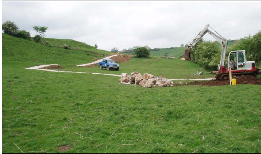
Fig. 3 Completed footpath/cycleway to the south of the stream (facing west)
