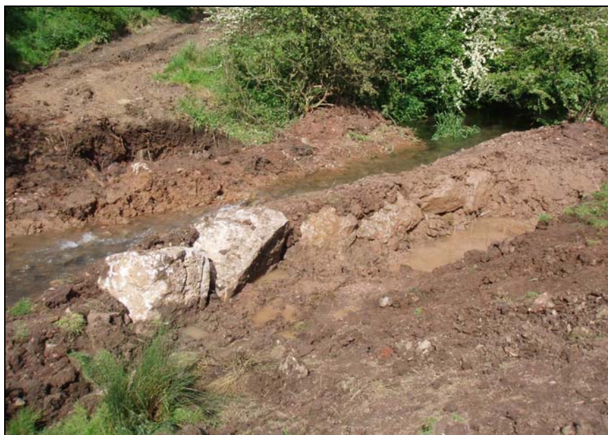
Fig: 8. Post excavation photograph of the trenches (facing north-east)
