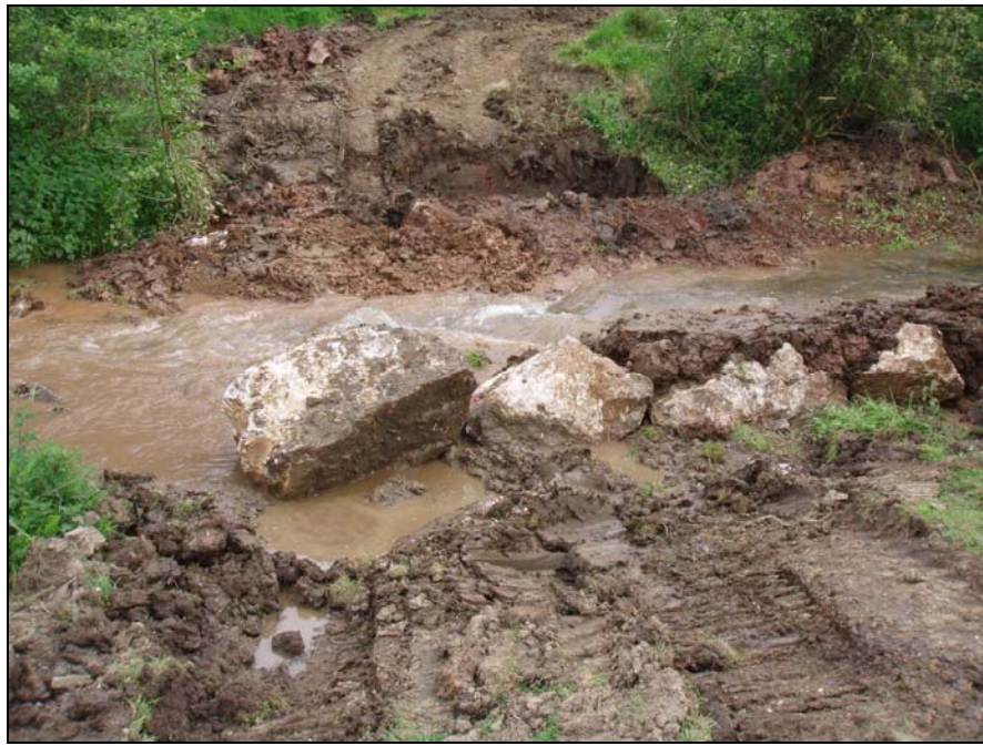
Fig. 4 Construction of stream diverting walls (facing NE)
