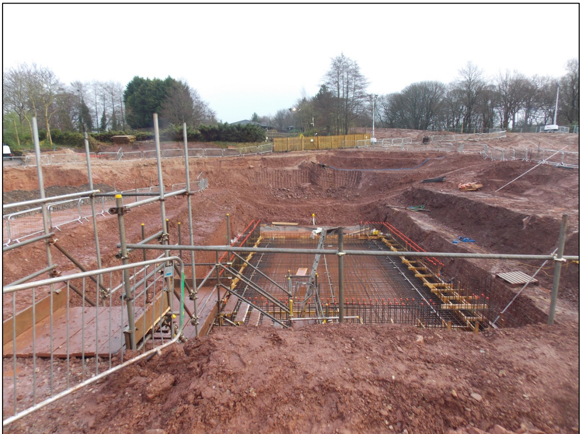
Figure 5. The foundations for the new attraction.
