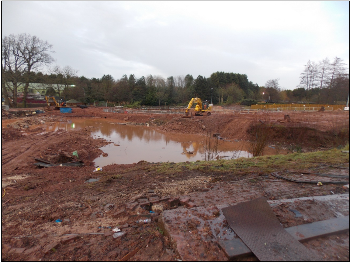
Figure 4. The development area seen from the south.
