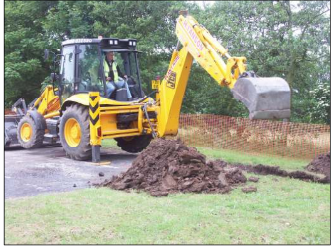
Excavation of Trench Five
