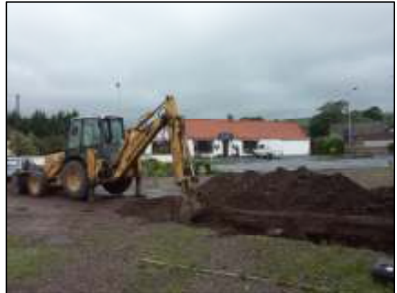
Opening of Trench One
