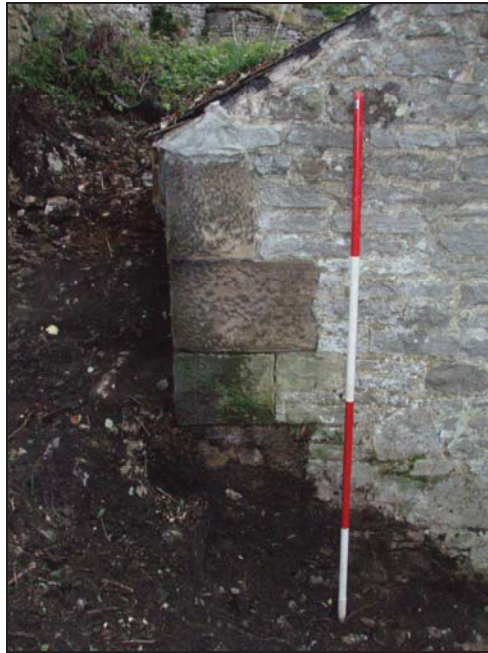
Figure 4. Limestone blocks and sandstone cornerstones (facing north-east) (scale = 2m).
