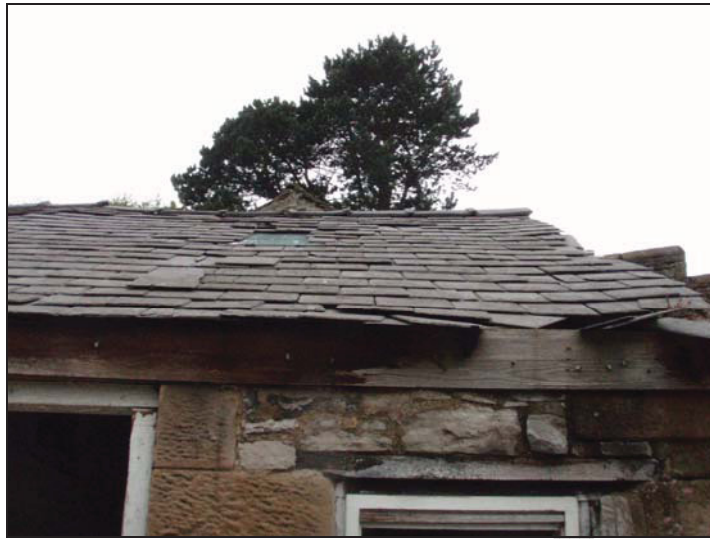
Figure 6. Roof slates on the south-east side of the building (facing north-west).
