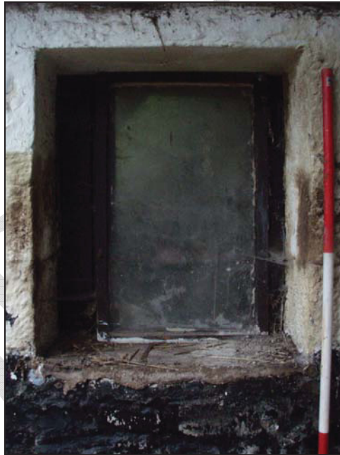
Figure 19. Window in north-west wall of southern room (facing north-west) (scale = 2m).
