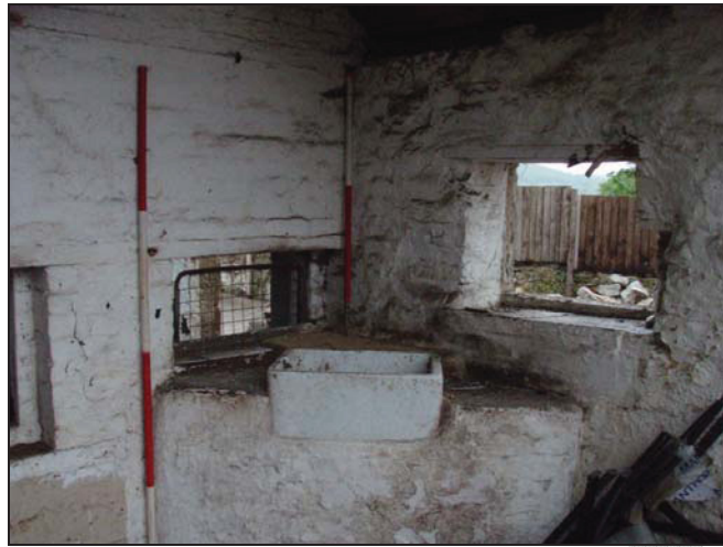
Figure 22. Sink addition to the southern room (facing east) (scale = 1m).
