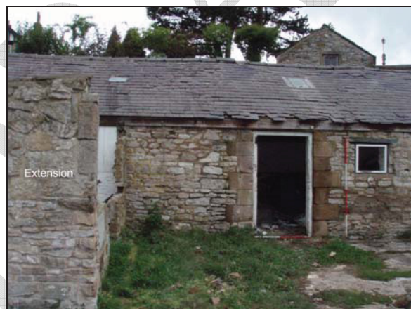
Fig. 15. Later extension onto south-east wall of building (facing north-west) (scale = 2m).
