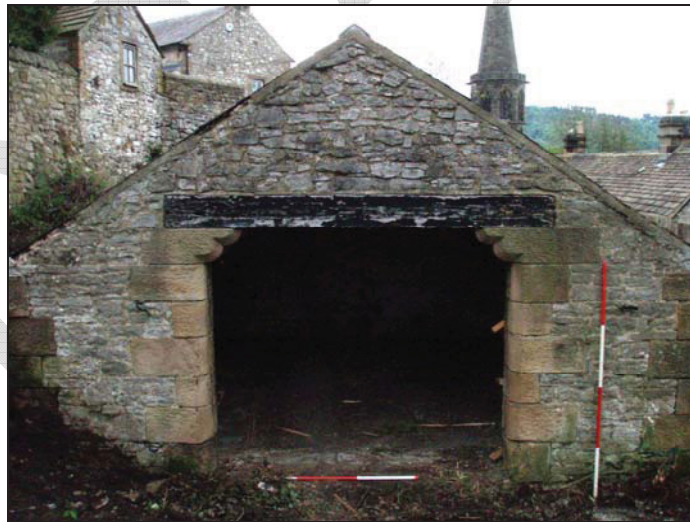
Figure 7. South-west exterior wall of the building (facing north-west) (scale = 2m).
