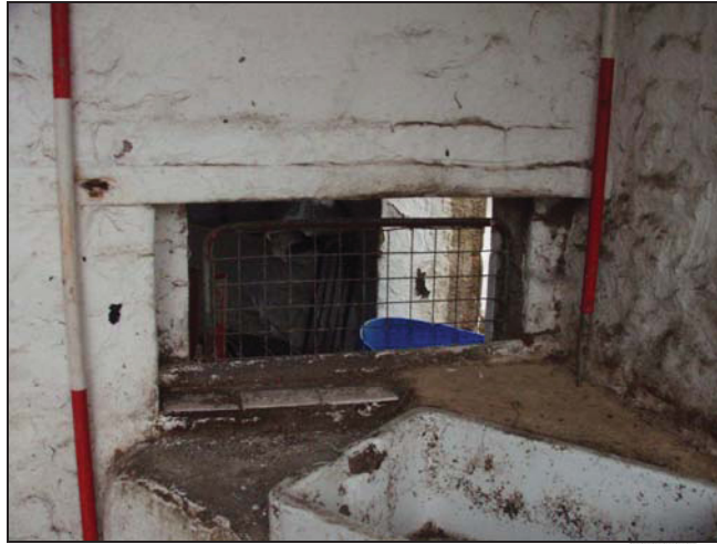
Figure 26. Window in north-east wall of southern room (facing east) (scale = 1m).
