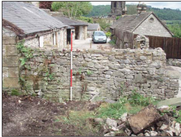
Fig. 16. South-east wall of extension (facing north) (scale = 2m).
