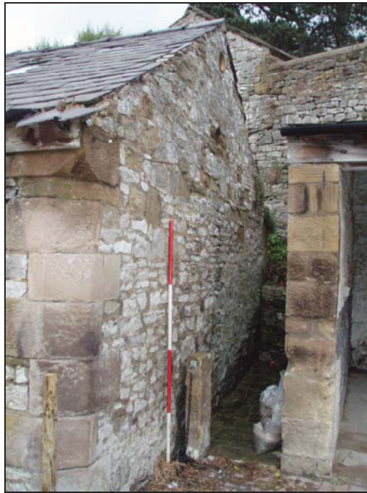
Figure 8. North-east wall of building (facing north-west) (scale = 2m).
