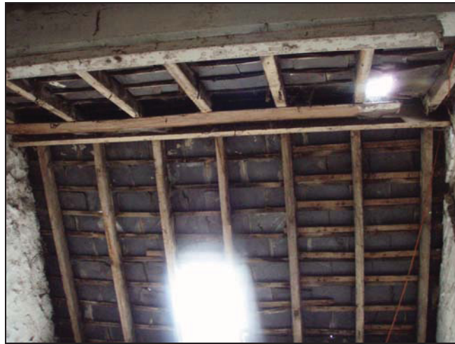
Figure 32. North-west roof of the central room (facing north-west).
