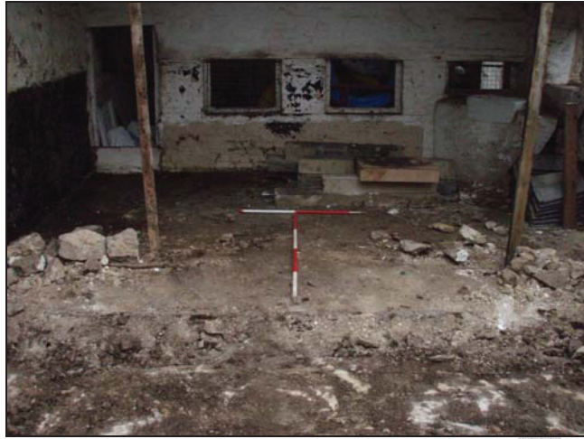
Figure 18. Concrete floor of the southern room (facing north-east) (scale = 2m).
