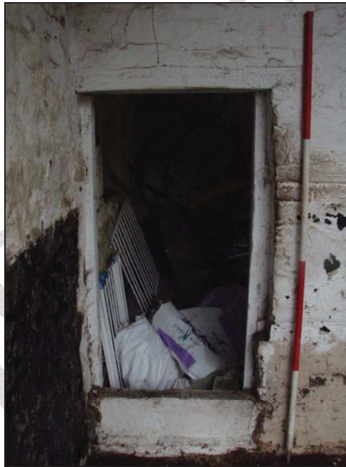
Figure 27. Door in north-east wall of southern room (facing north-east) (scale = 2m).
