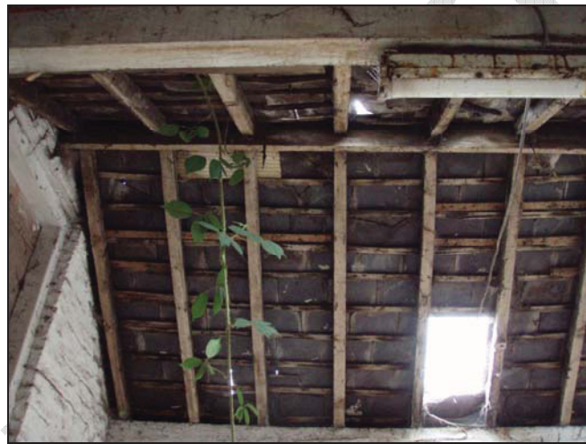
Figure 33. South-east roof of the central room (facing south-east).
