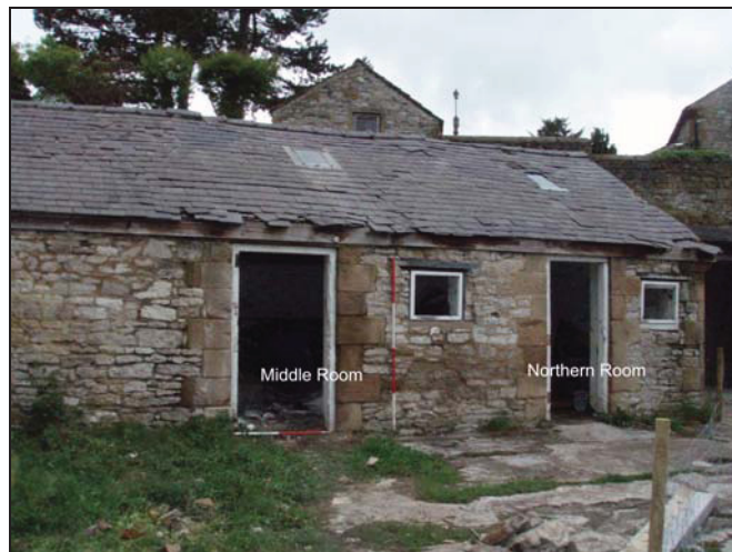
Figure 10. The south-east wall of the building (facing north) (scale = 2m).
