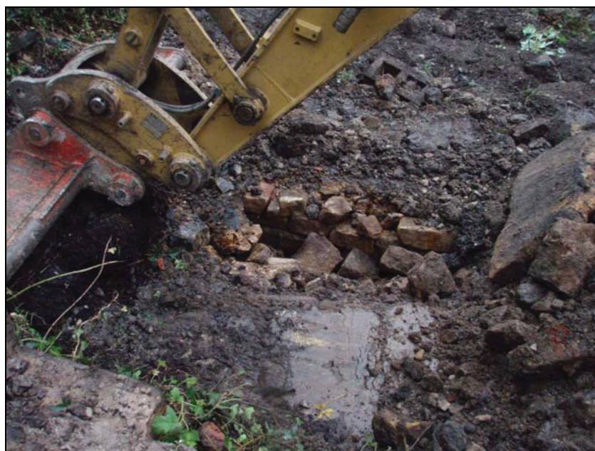
Fig. 7. Excavation of the area of contamination and the sandstone culvert (facing east)
