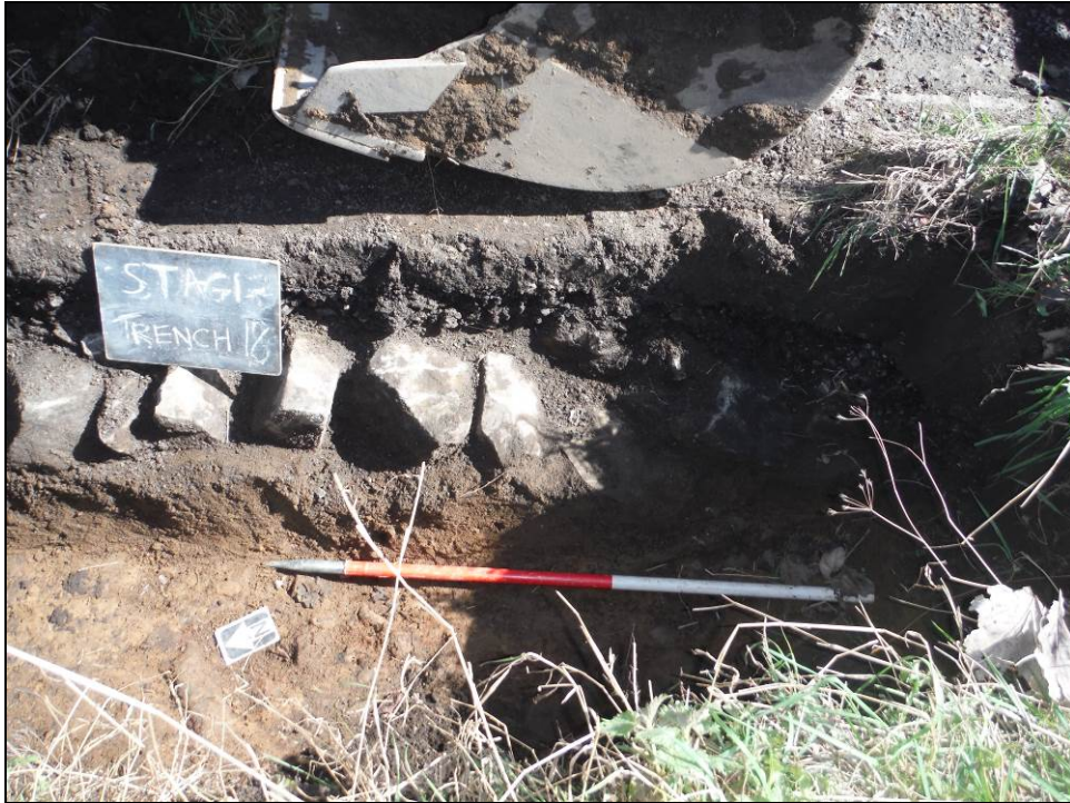
Figure 30. View facing south-east of Trench 18 with substantial modern road penning visible immediately below the modern road surface base layers (Scale = 1 x 1m).
