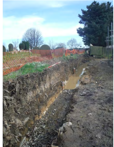
South facing section of construction trench, looking northeast.
