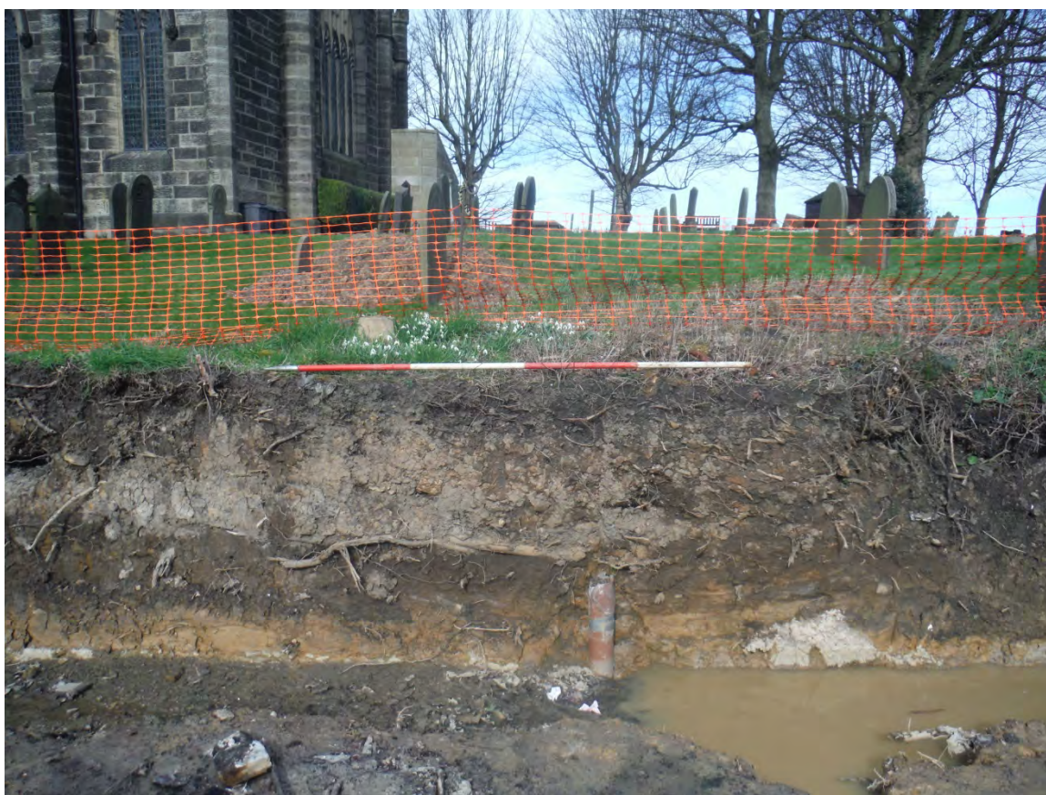
Figure 2. South facing section of construction trench.
