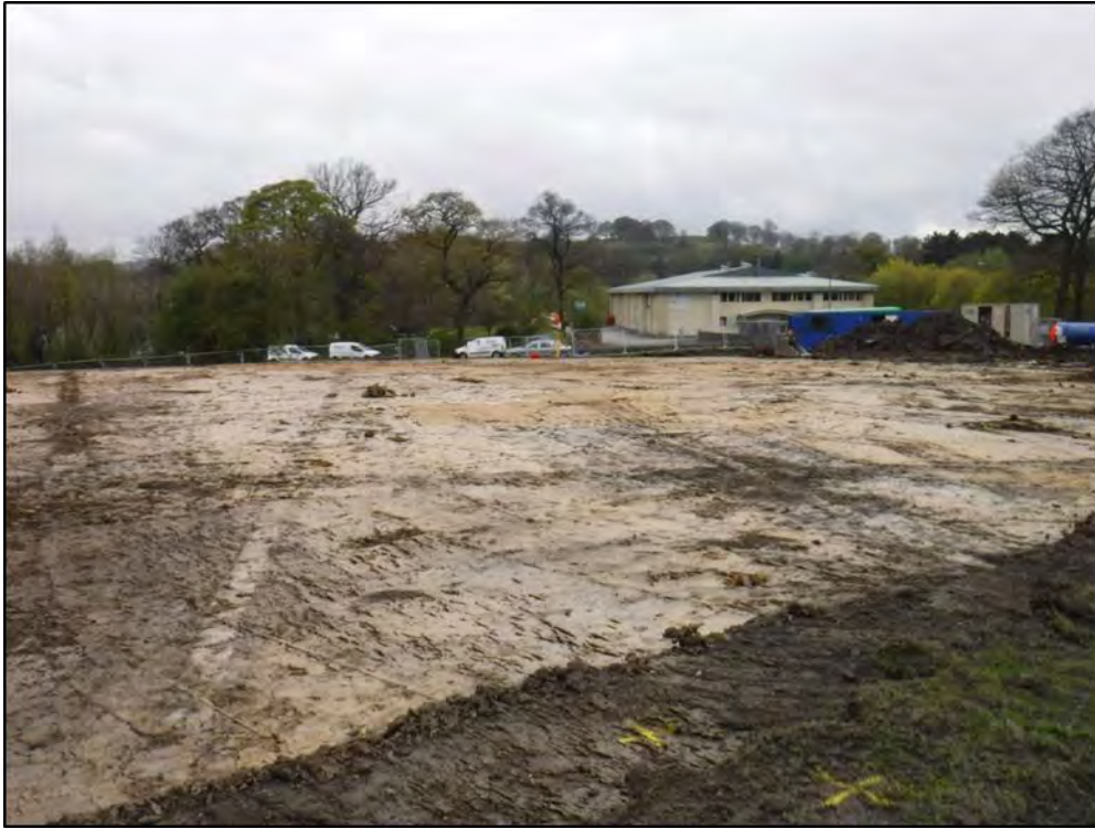
Figure 3. General shot of site post-strip looking southwest
