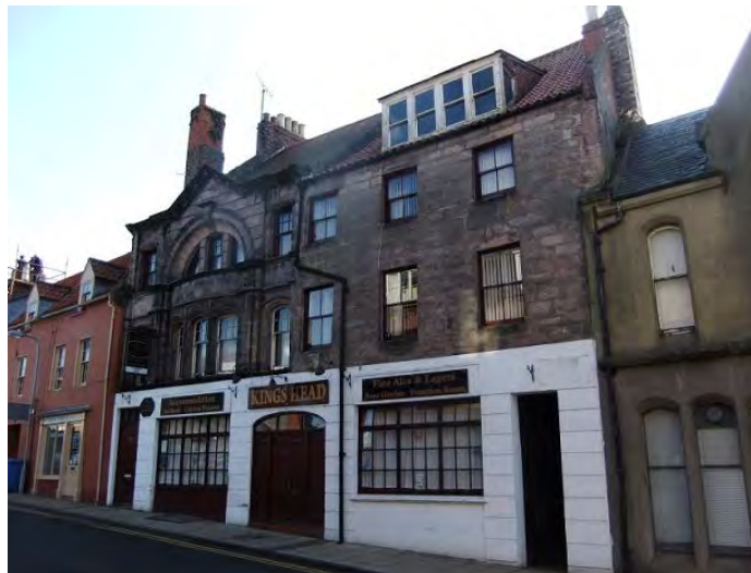
View facing south-west towards the Kings Head Public House, Church Street, Berwick-upon-Tweed
