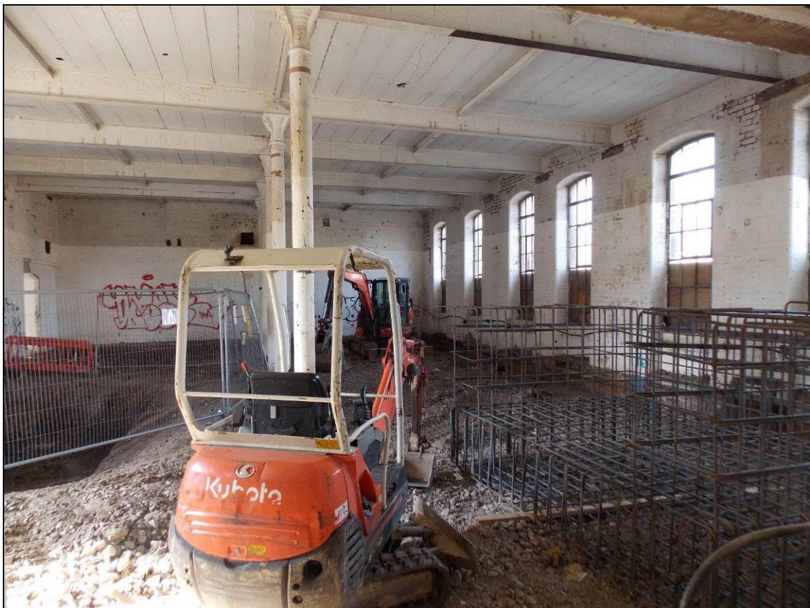
Figure 50: View of the interior of G6, with a central line of cast-iron columns.
