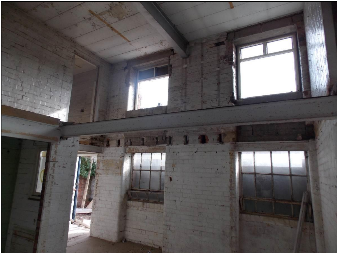
Figure 48: View of the south-east wall of G4, with slots indicating the former ceiling joists.
