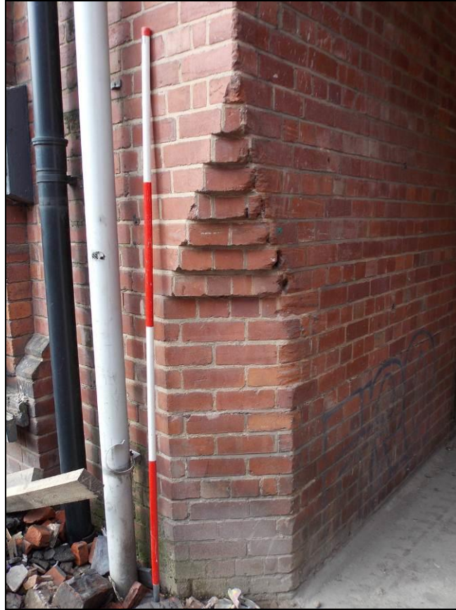
Figure 17: Chamfered edge to allow for the turning of trucks/ lorries, 2m scale.
