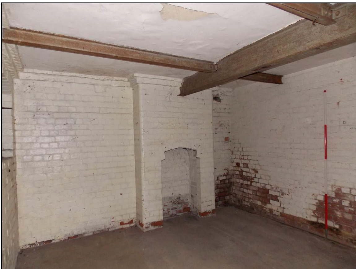
Figure 33: View of C6 with evidence of the former fireplace, 2m scale.
