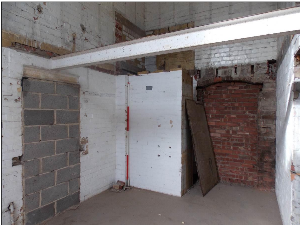
Figure 46: View of room G5, the position of the former ceiling joists are apparent, 2m scale.
