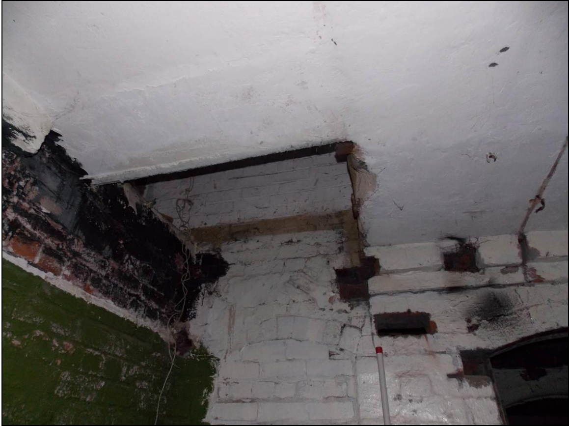
Figure 28: View of the hole in the ceiling which connects C5 to G5.
