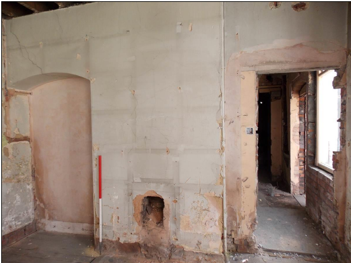
Figure 69: South-east wall with redundant fireplace in G1 in the North-East Range of building B, 1m scale.
