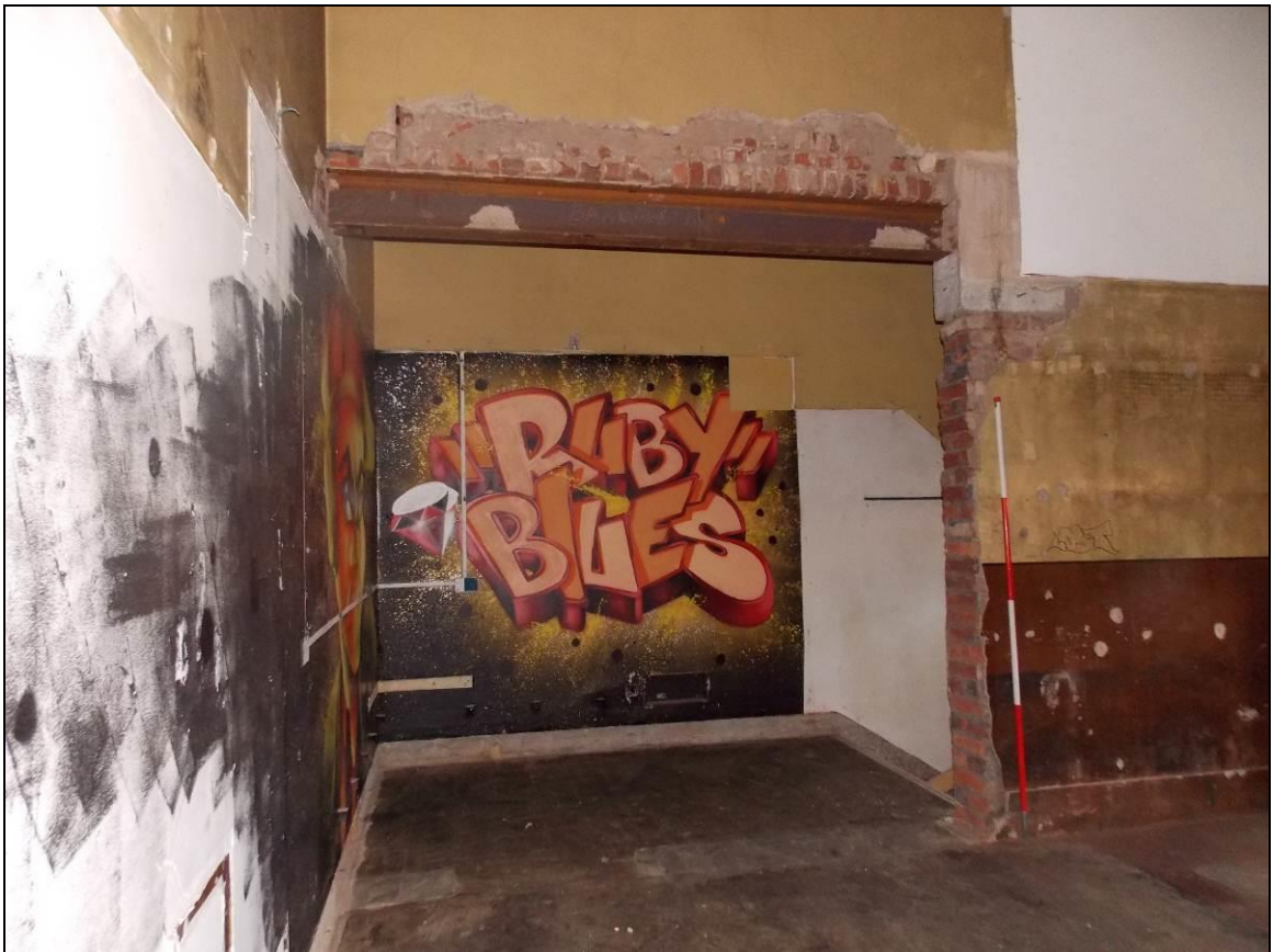
Figure 42: View of an opening containing an RSJ beam, 2m scale.
