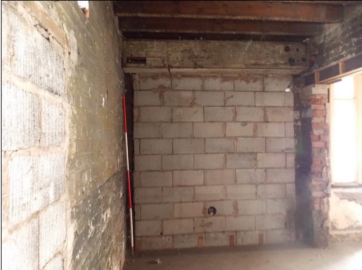
Figure 74: View of a concrete breeze-blocked opening along the south-west wall, 2m scale.
