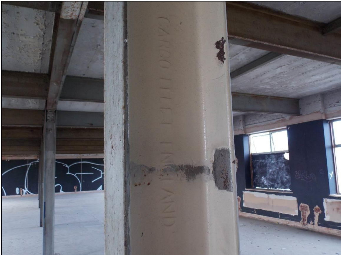
Figure 54: 'Cargo Fleet England' is moulded into the steel structure along the second floor.
