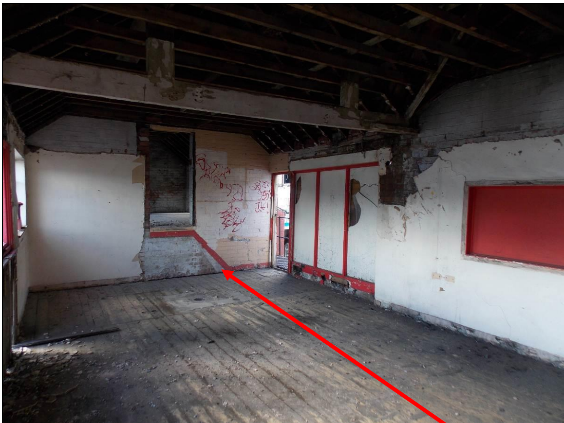
Figure 92: View of the upper floor in the South-East Range and the outline of the former staircase.
