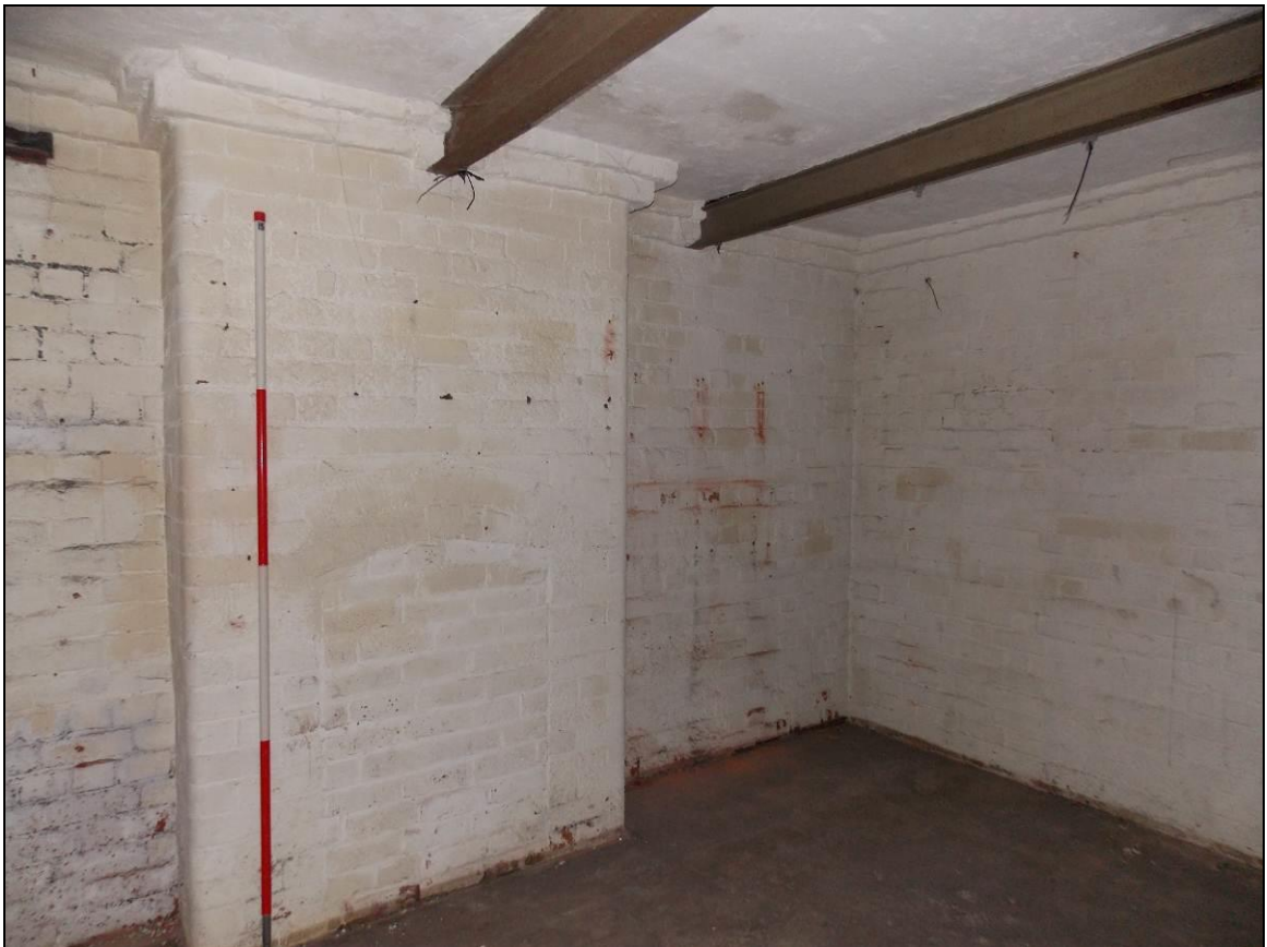
Figure 31: View of the blocked fireplace along the north-east wall in C5, 2m scale.
