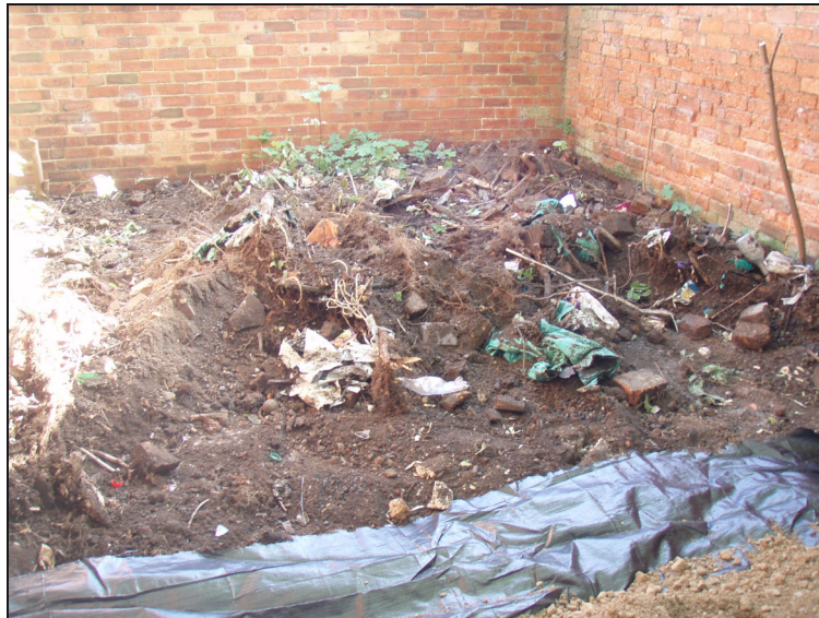
Fig. 6 View of the area surrounding the Pump House before clearance
