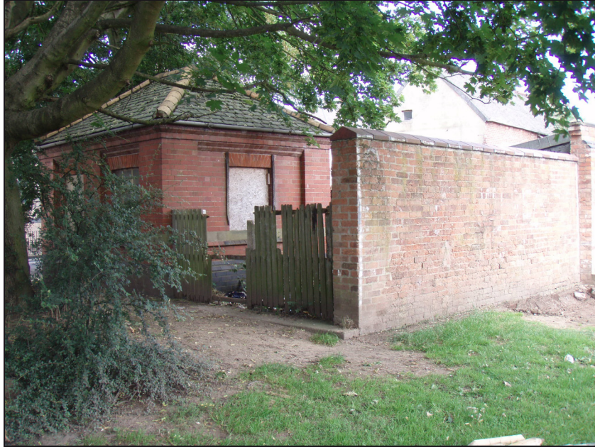
Fig. 2 View to the rear of the Pump House .
