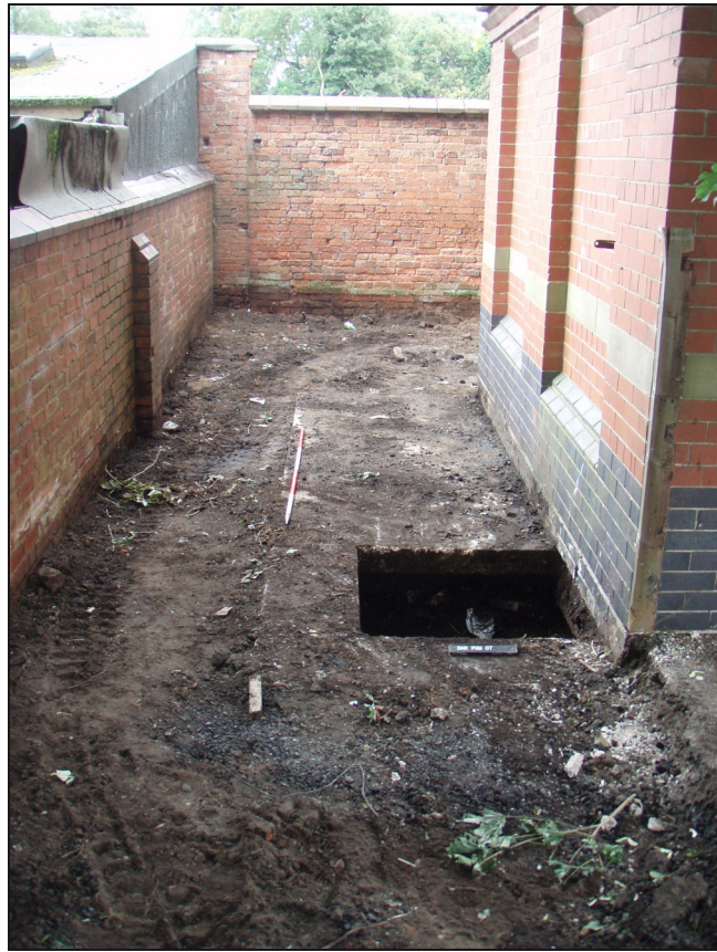
Fig. 8. View of the cellar entrance, looking east. Scale: 2m
