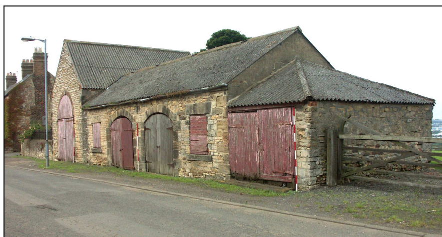
Figure 26: L-Plan barn, general view looking north-west
