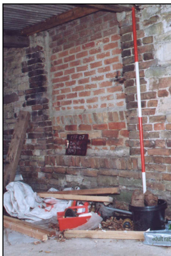
Figure 32: Blocked window, north-south range extension
