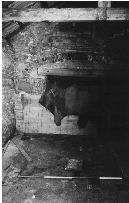
Figure 36: possible boiler base, Room 2
