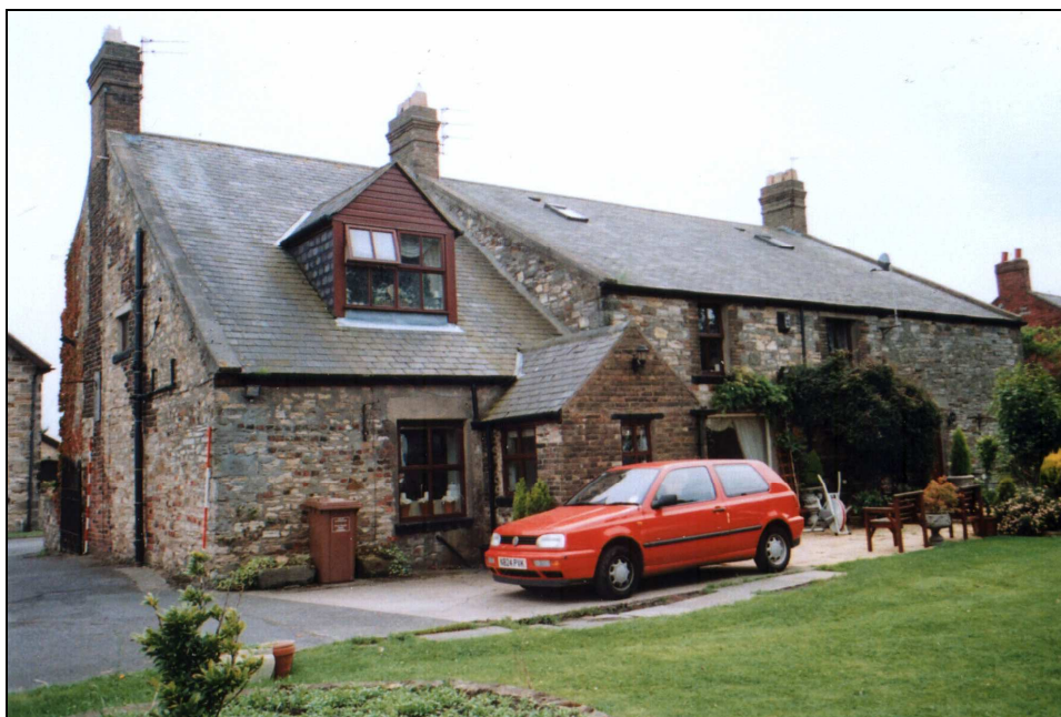
Figure 24: Farmhouse north (rear) elevation.
