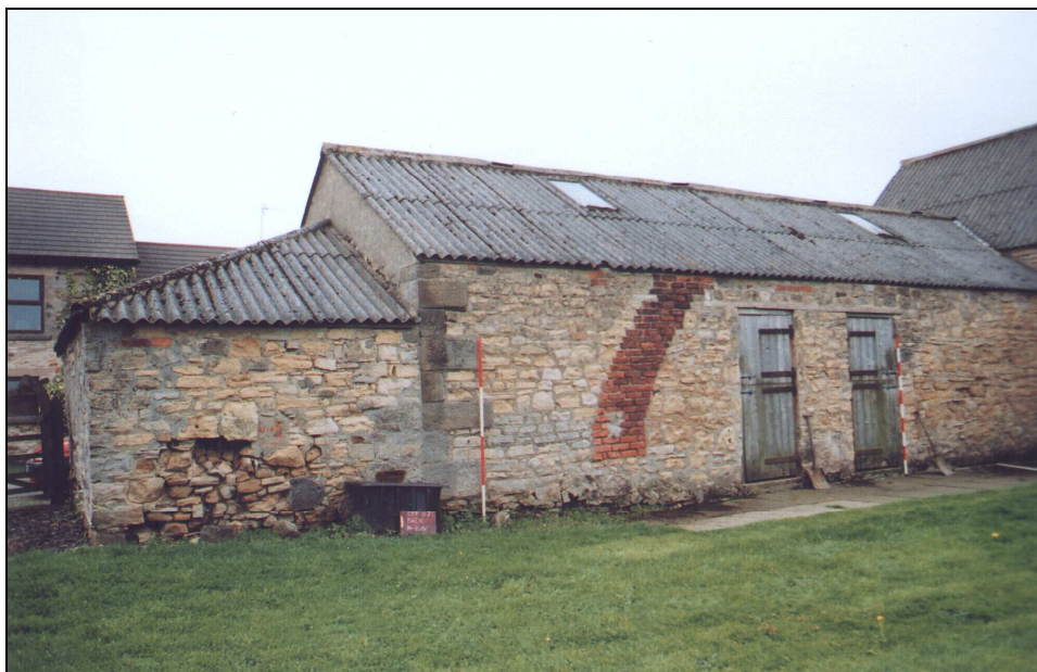
Figure 30: L-Plan Barn east-west range, north elevation
