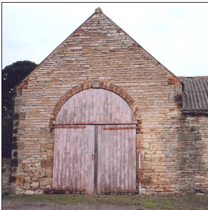
Figure 29: L-Plan barn north-south range gable end
