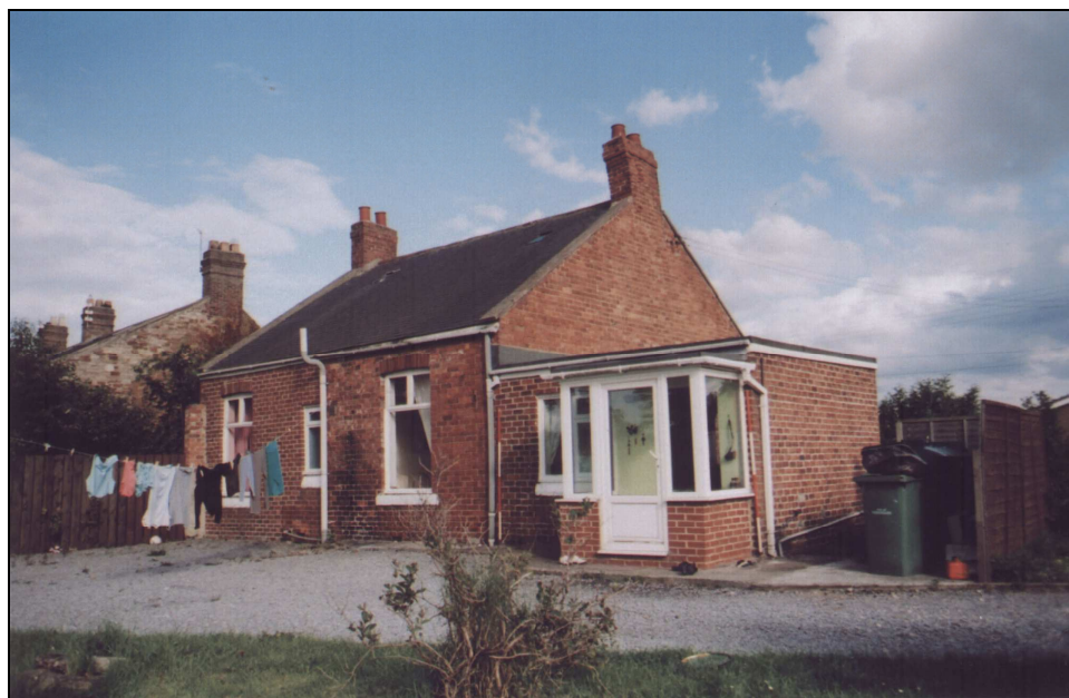
Figure 22: Ivy House north (rear) elevation. Scales = 2m
