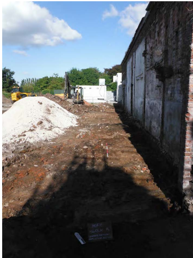
Figure 13. Exterior strip exposing natural clay (1002) beneath footings of former structures along north-west side of Block B. Scale: 2m.
