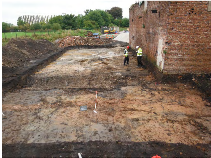
General view of the site behind Block C, looking northeast
