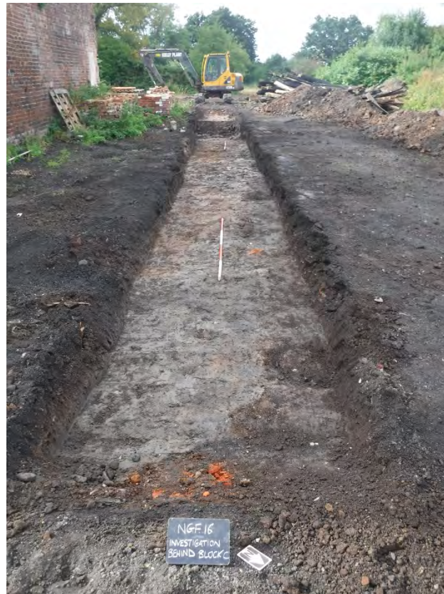
Figure 24. Initial investigation trench behind Block C. Note the concrete stanchion bases along the right hand side of the base of the trench which reflect the outer extent of a former lean-to structure, looking south-west. Scale: 2x2m.
