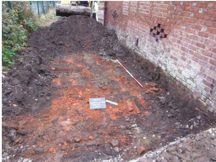
Figure 18. Rubble levelling/hardstanding deposit (1032) by south-east gable end of Block B. Scale: 2m.
