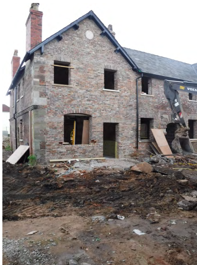
Figure 3. Block A outbuilding prior to removal of footings, looking south-east.
