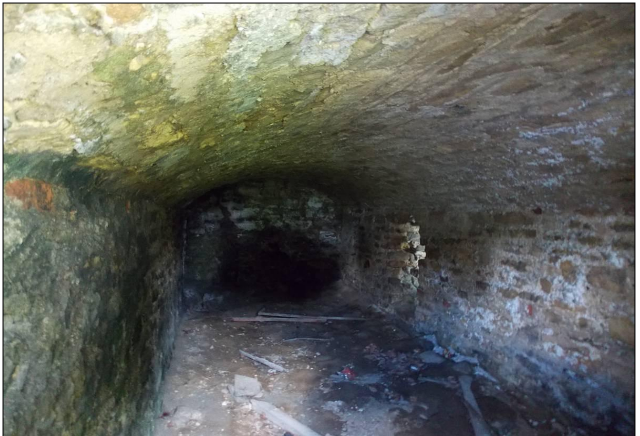
Figure 23: Vaulted basement, looking west in 2012.
