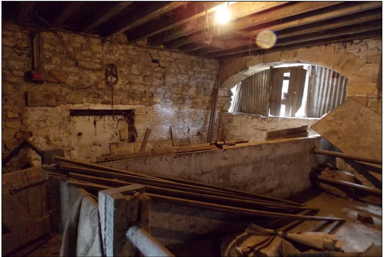
Figure 36: Ground floor with arched doorway and ceiling hatch, looking west in 2012.
