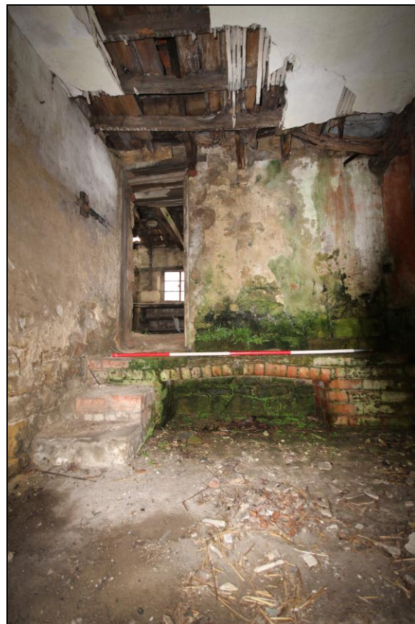
Figure 19: View of the interior of building D, 2m scale.
