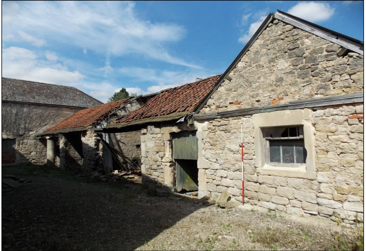
Figure 48: South elevation of Building K, looking north-west in 2012, 2m scale 2m.
