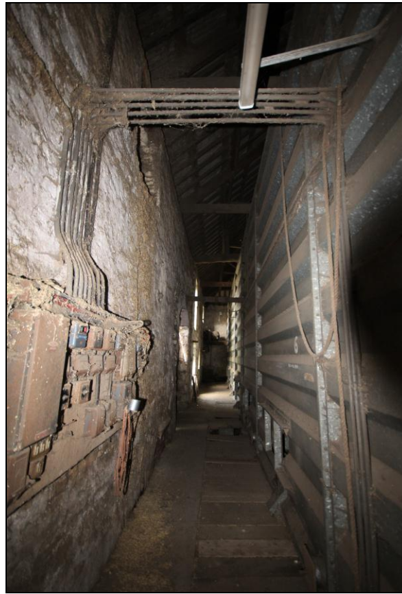
Figure 56: View of the interior of building L, facing north.
