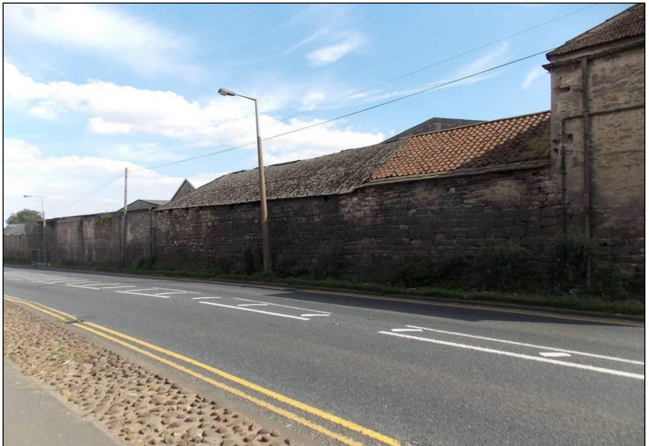
Figure 49: North elevation of Building K, looking south-east in 2012.
