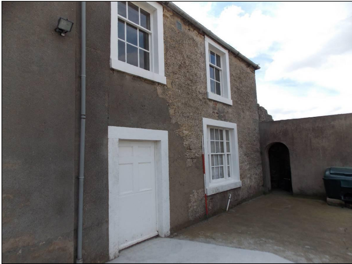
Figure 4: North elevation of Building B, looking south-west, 2m scale.
