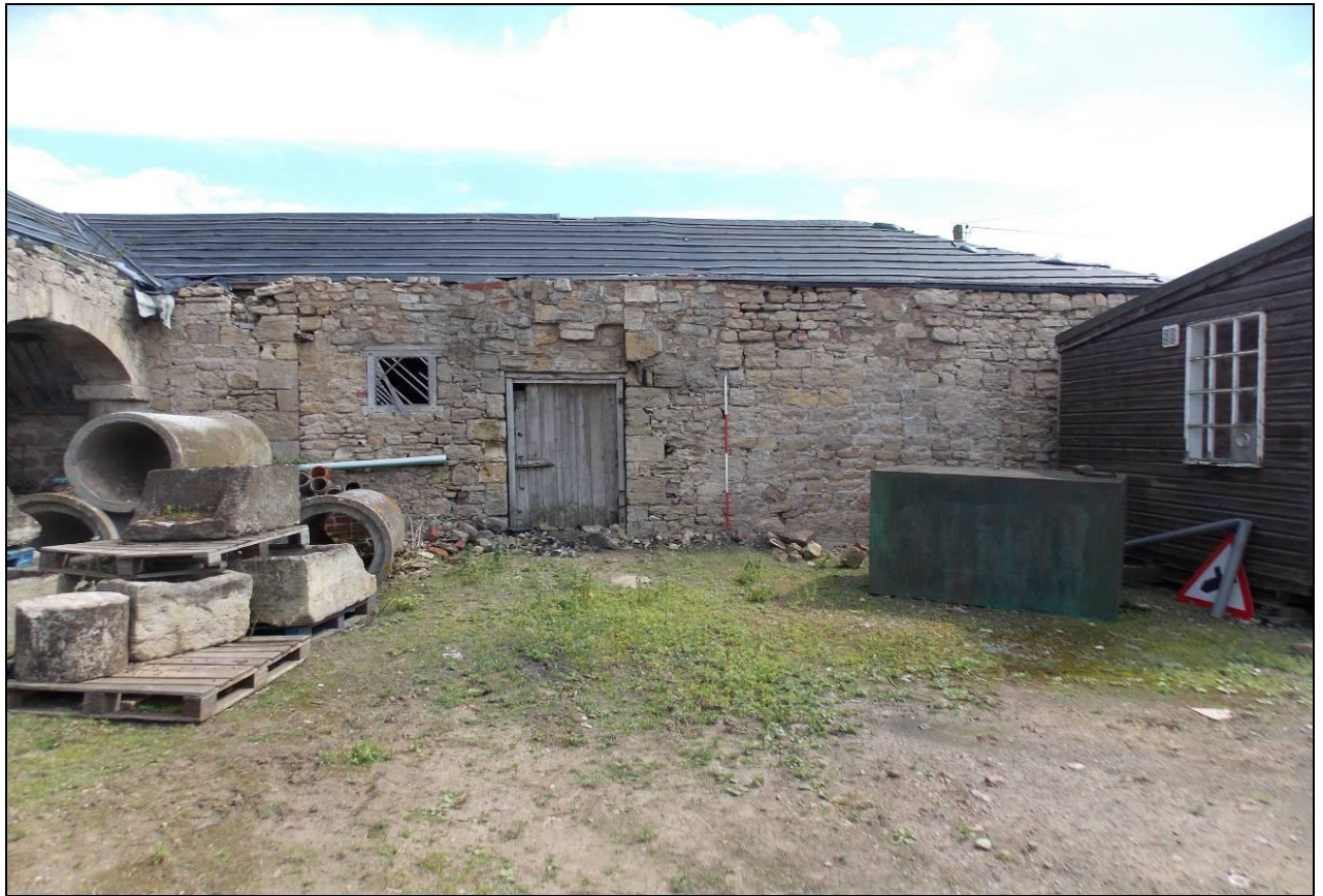
Figure 24: West elevation of Building E in 2012, 2m scale.
