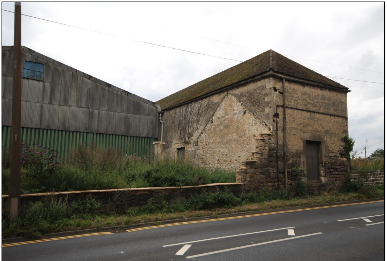
Figure 51: Currently all that remains is the outline of the former western gable.
