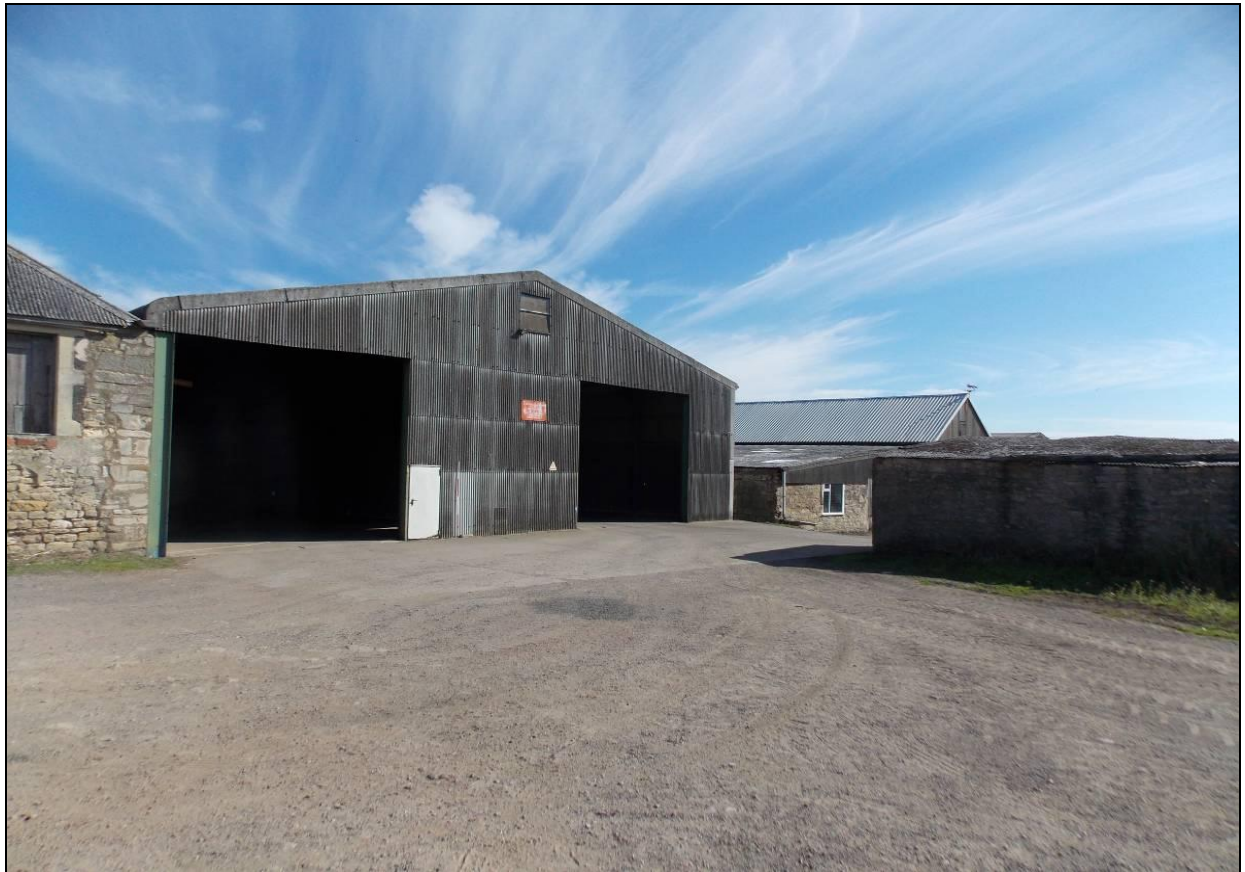
Figure 46: Front elevation of Building J, looking north-east, 2m scale.
