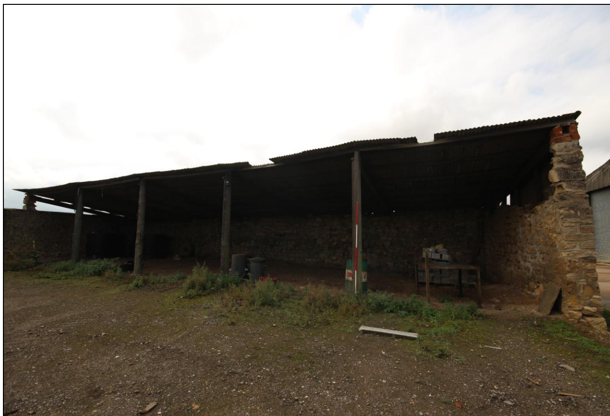
Figure 61: Building N, looking south-west, 2m scale.
