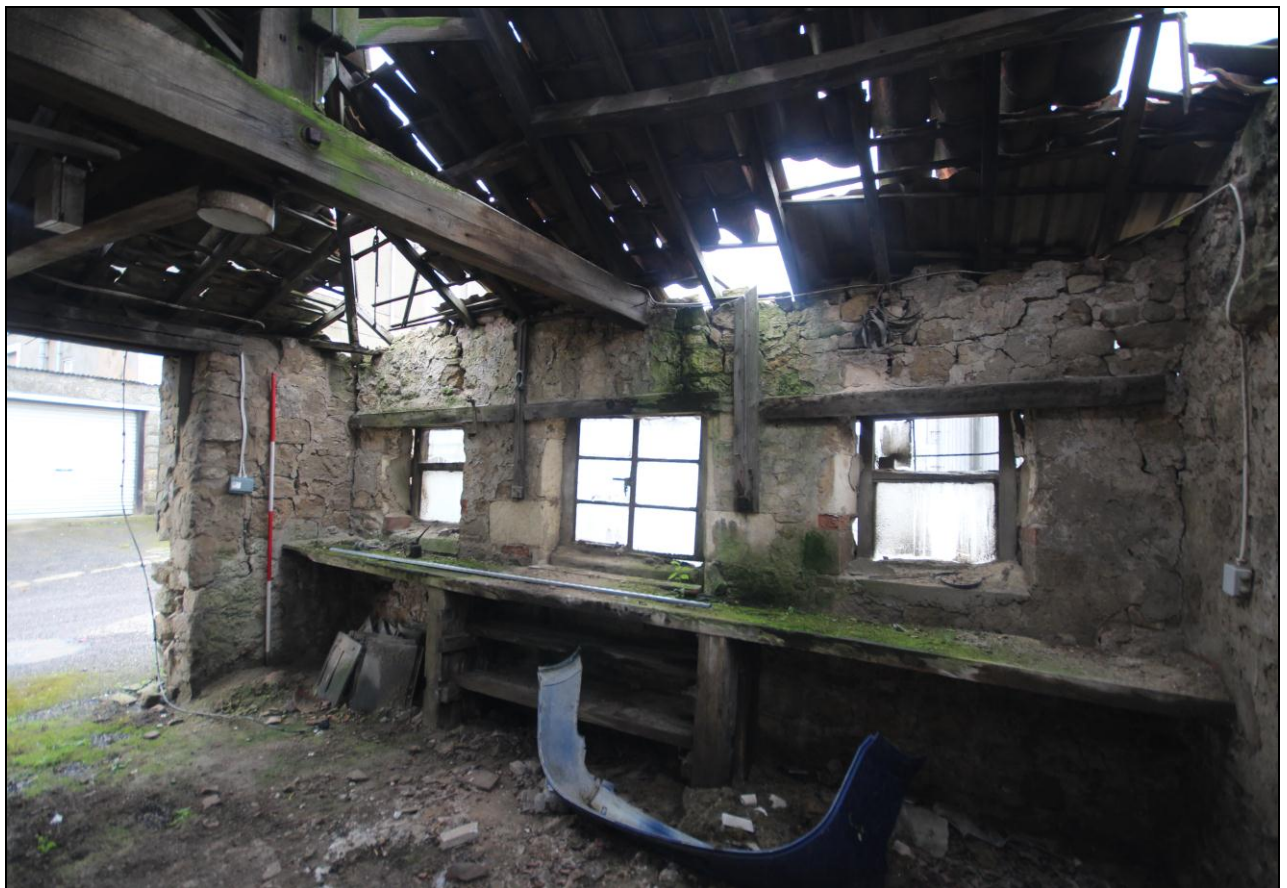
Figure 17: view of the interior of building D, 2m scale.
