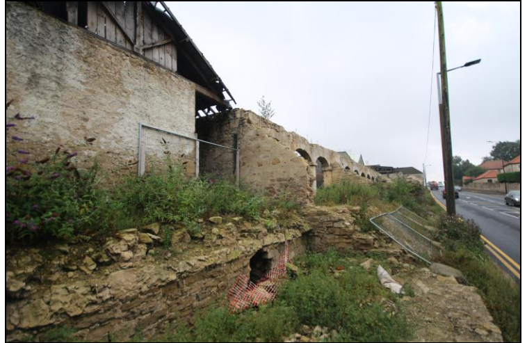
View of the buildings bordering the site to the north of the complex.
