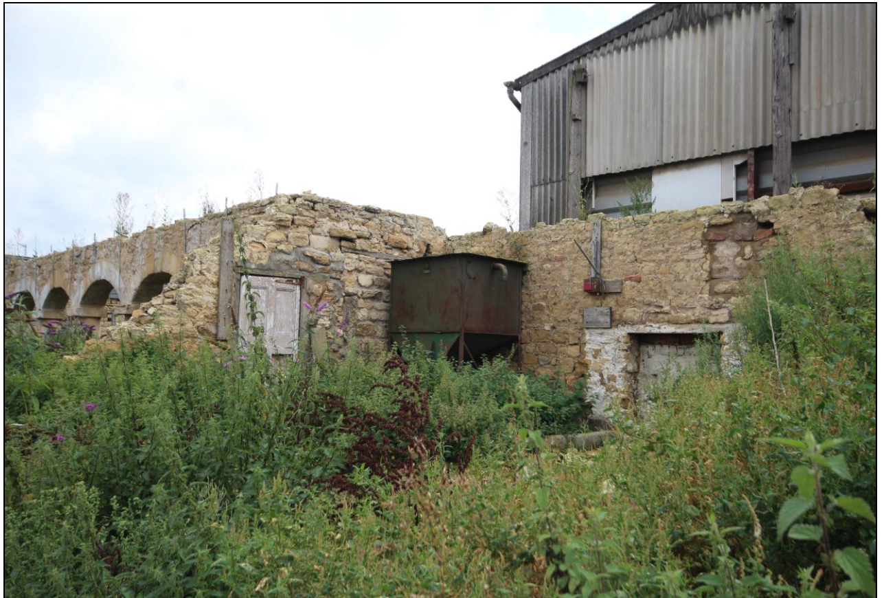
Figure 38: View of the interior of building G was has succumbed to vegetation.
