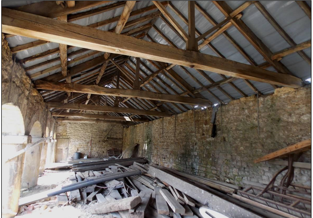
Figure 31: Internal view of Building F, looking west in 2012, 2m scale.
