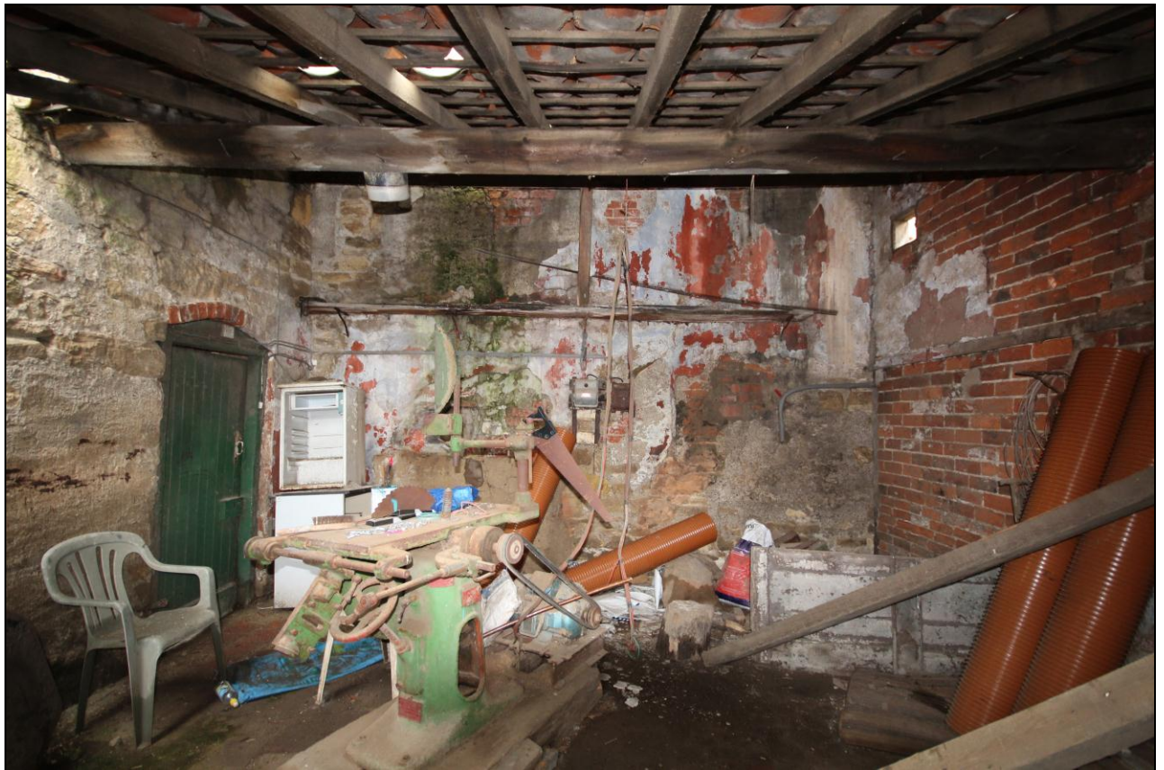
Figure 13: View of the interior of the brick section of building C.
