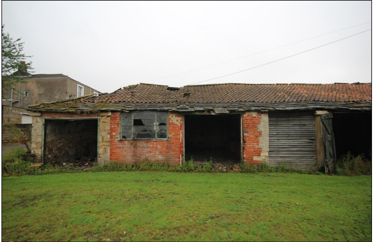
Figure 16: View of the exterior of building D, 2m scale.
