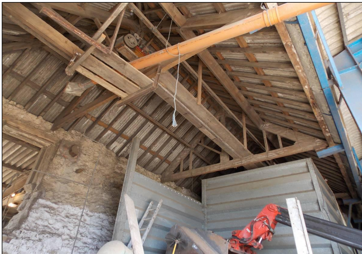
Figure 58: Roof structure of Building L, looking north in 2012.
