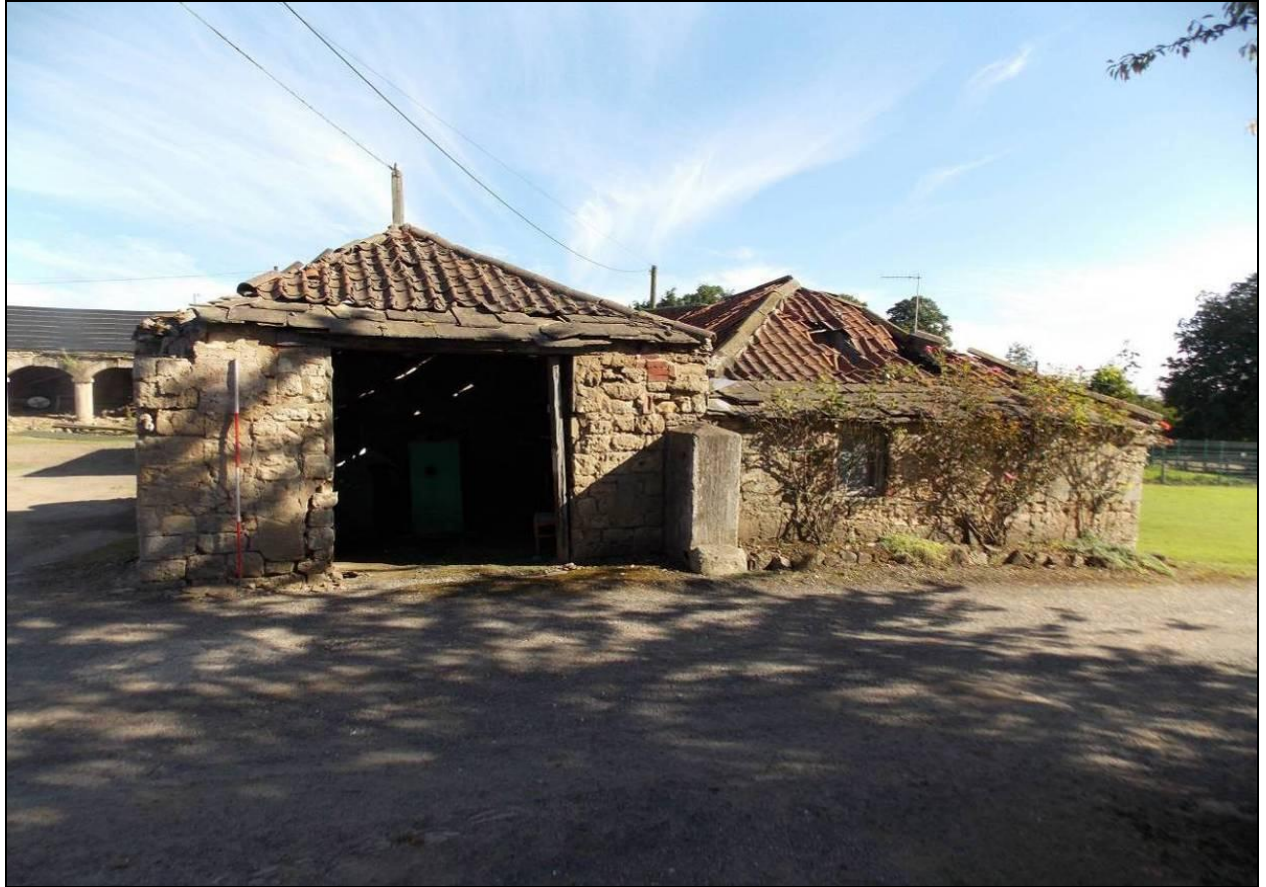
Figure 14: South elevation of Building D in 2012, 2m scale.
