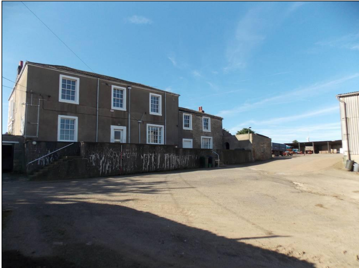
Figure 3: General view of Building B adjoining the main farmhouse (Building A), looking south-west.
