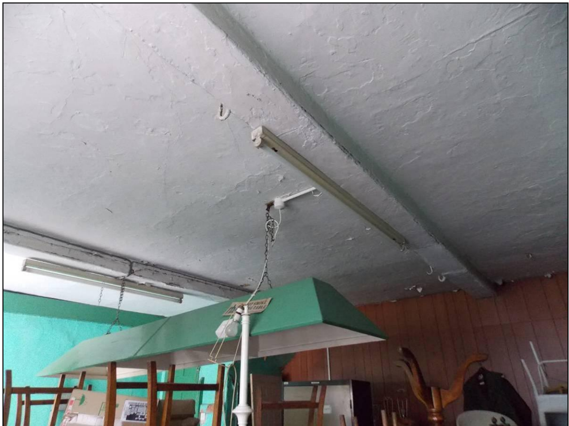
Figure 7: Ceiling beam with iron hooks.
