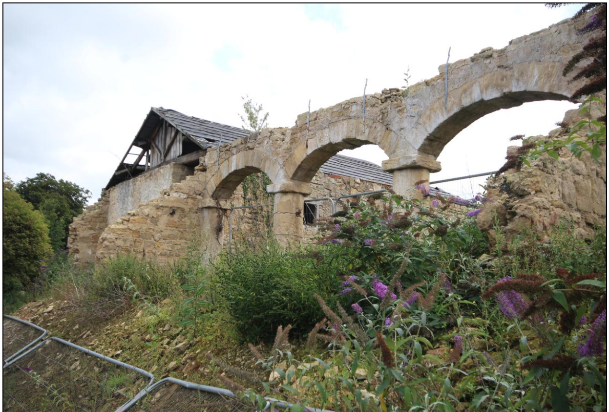
Figure 32: View of the colonnade of building F.
