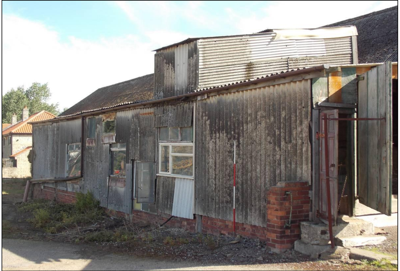
Figure 59: West elevation of Building M, looking north-east in 2012, 2m scale.
