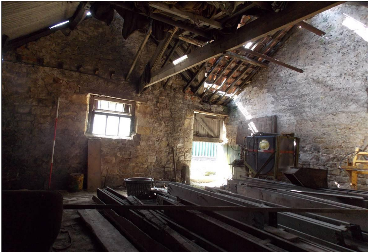
Figure 50: Inside the easternmost cross-wing, looking south in 2012, 2m scale 2m.
