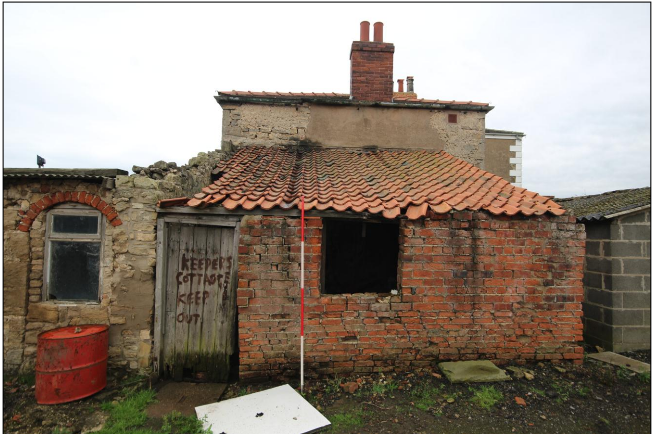
Figure 10: View of the brick section of building C, 2m scale.
