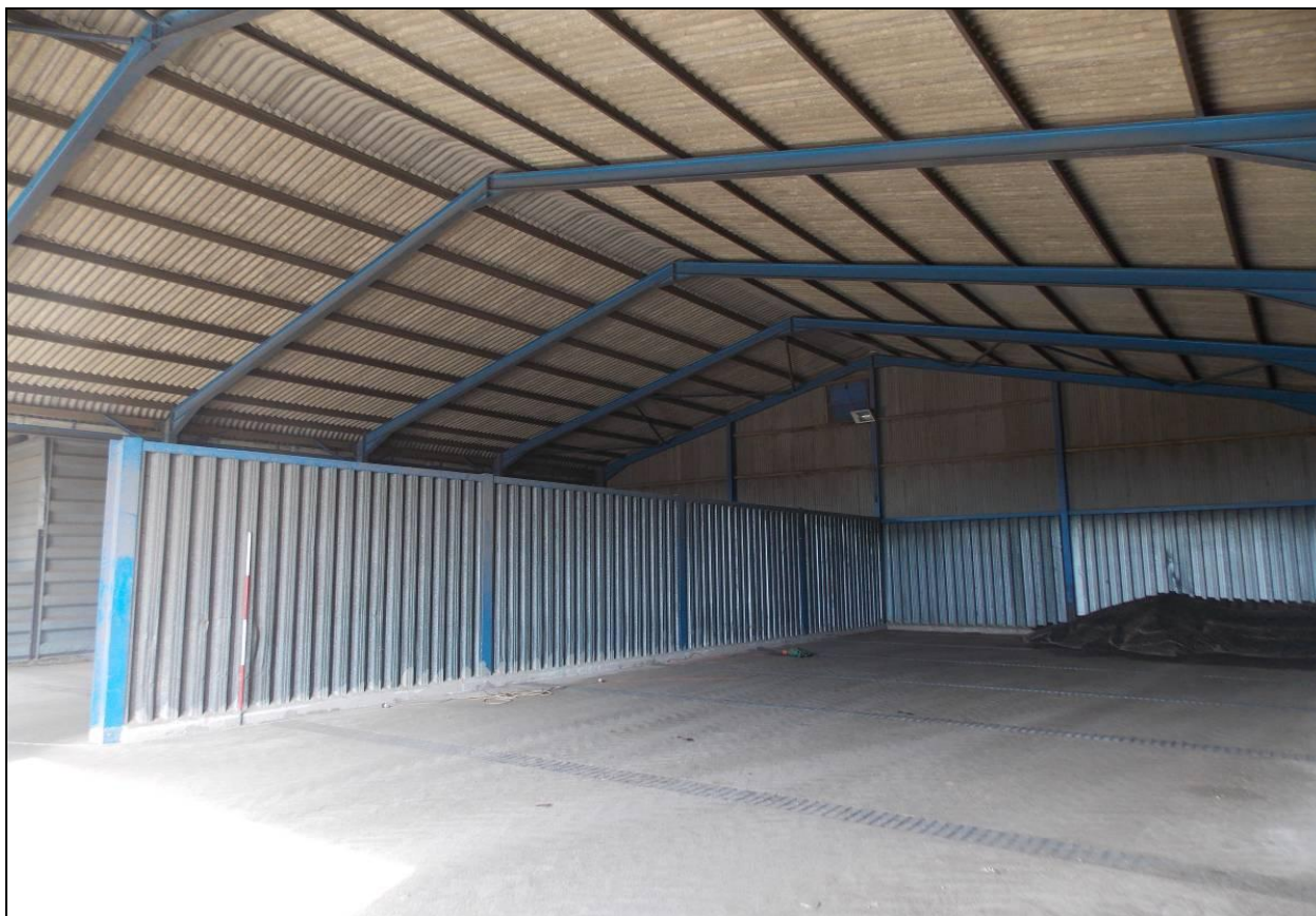
Figure 47: Internal view of Building J, looking north, scale 2m.
