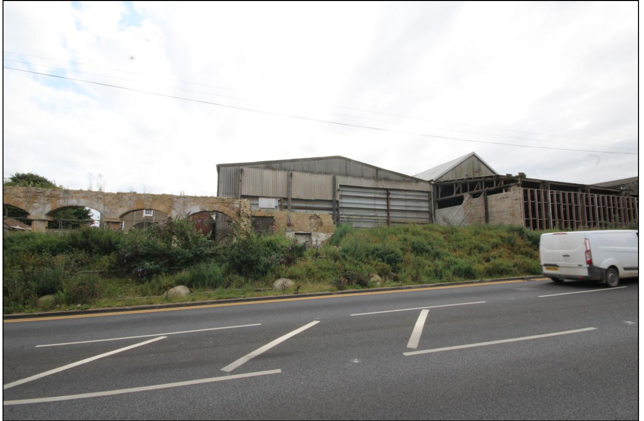
Figure 33: View of the dilapidated building F, represented by a single elevation.
