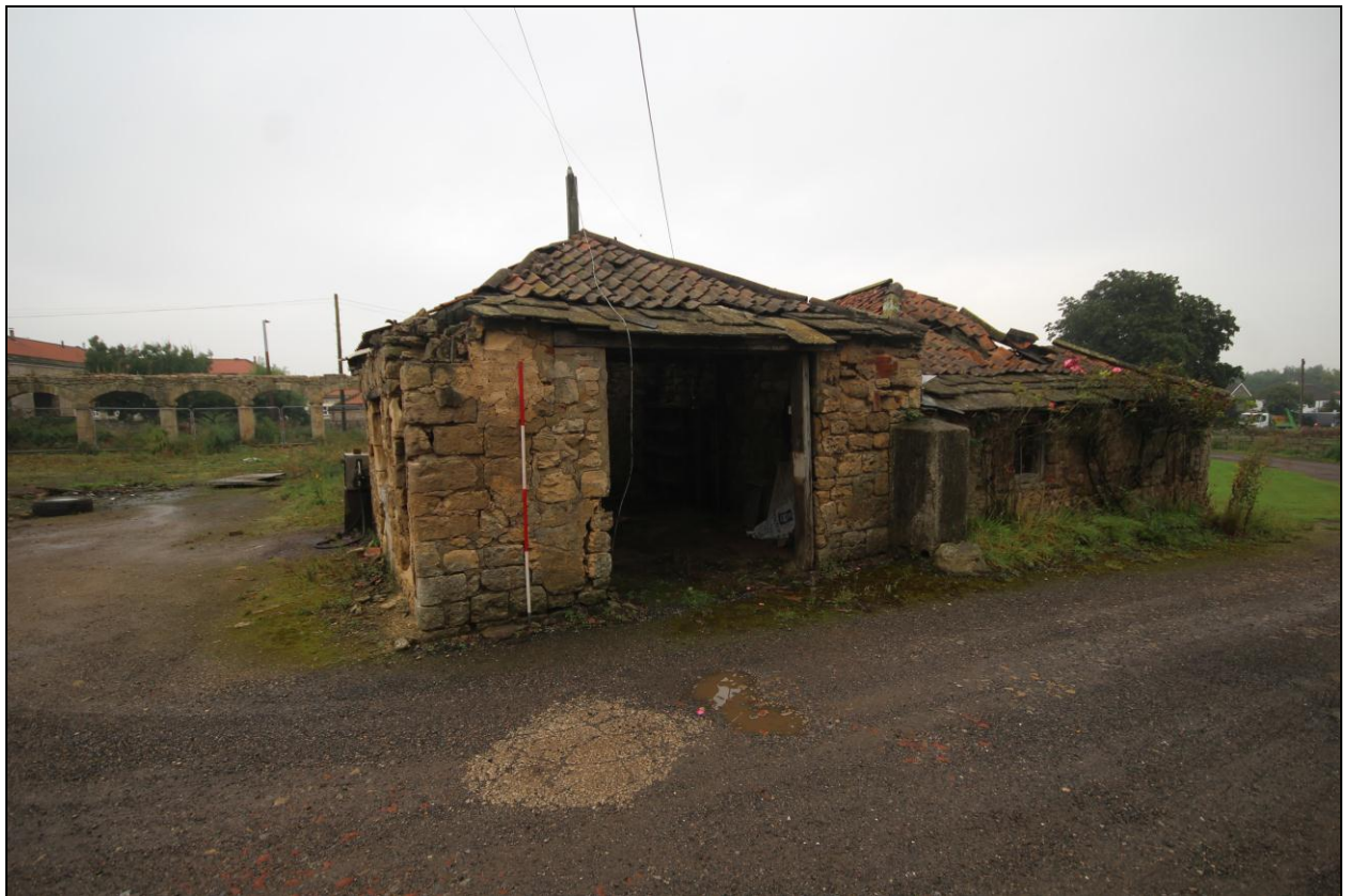
Figure 15: View of the exterior of building D, 2m scale.
