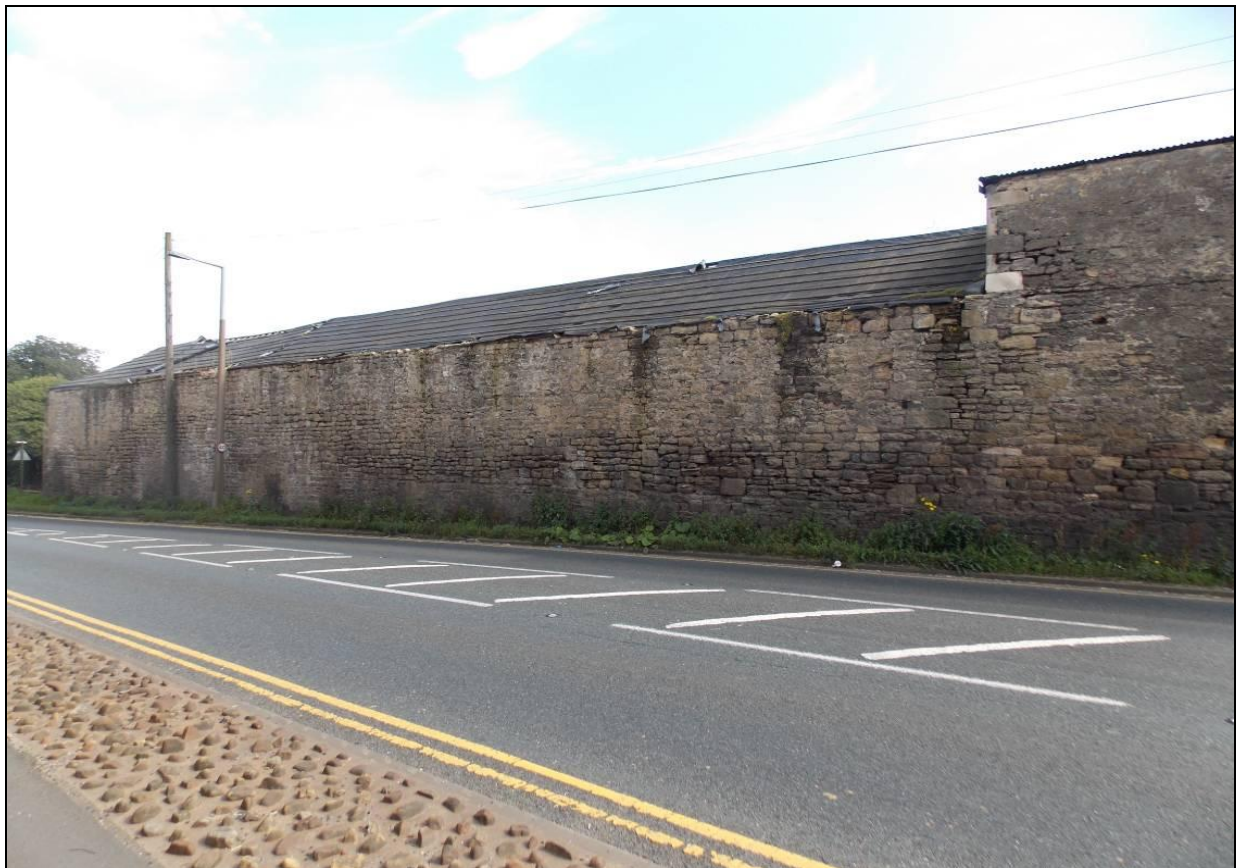
Figure 30: North elevation of Building F along Barnsley Road, looking south-east in 2012.
