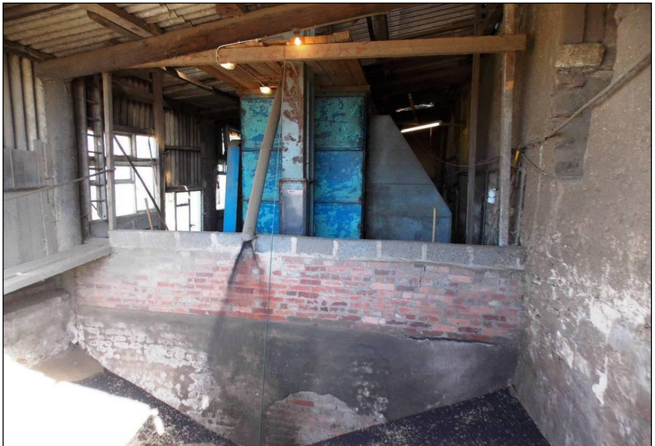
Figure 60: in pit inside Building M, looking north in 2012.
