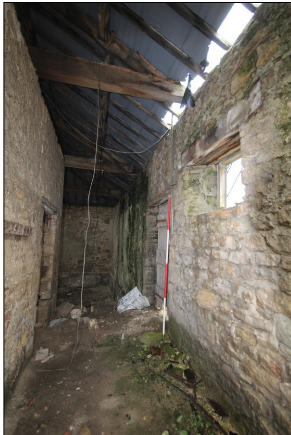
Figure 27: View of the interior of part of building E, 2m scale.
