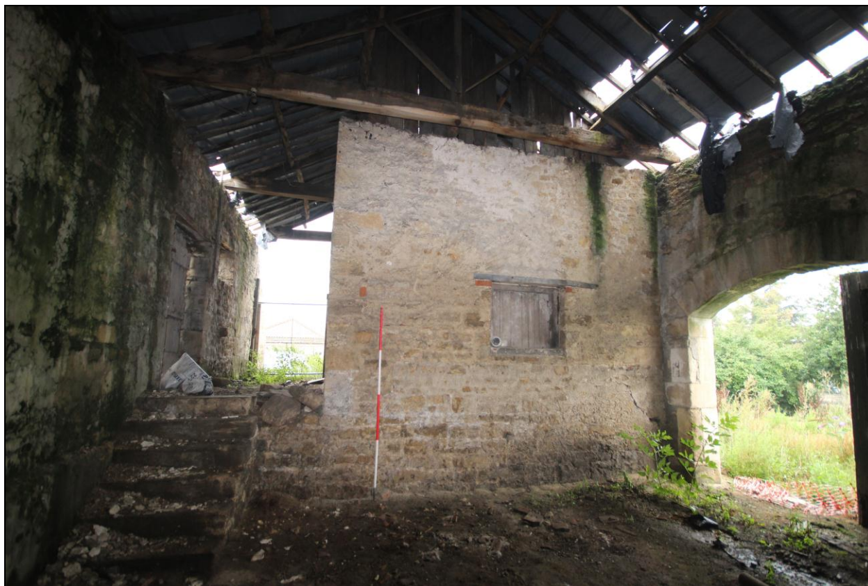
Figure 28: View of the interior of building E, facing northwards, 2m scale.
