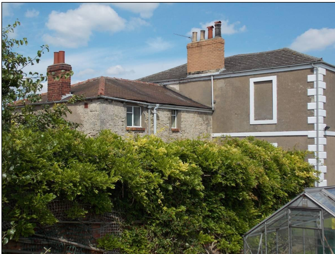
Figure 5: South elevation of Building B abutting the main farmhouse (Building A), looking north-east.
