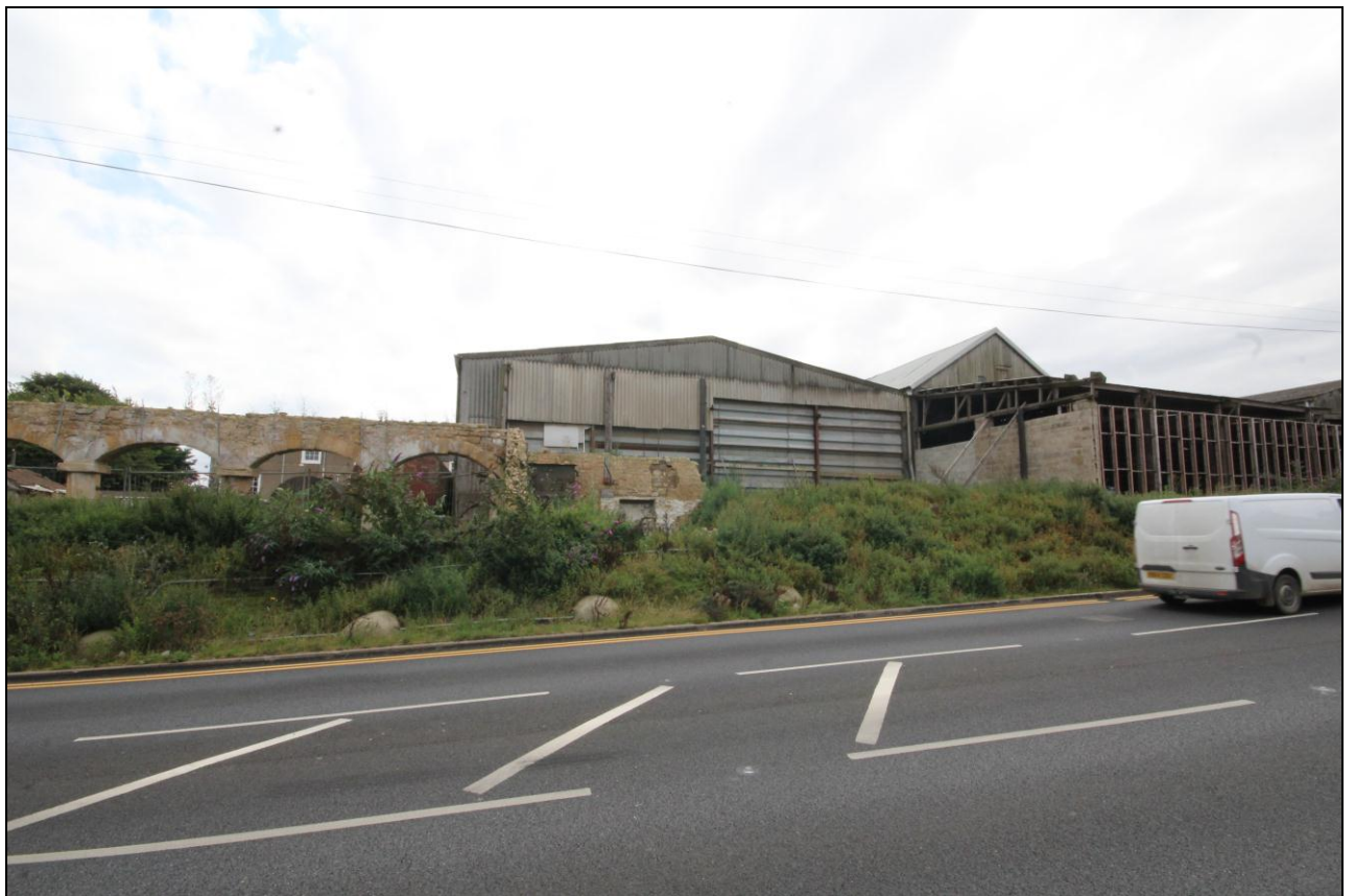
Figure 37: View of the dilapidated building G, which has nearly disappeared.
