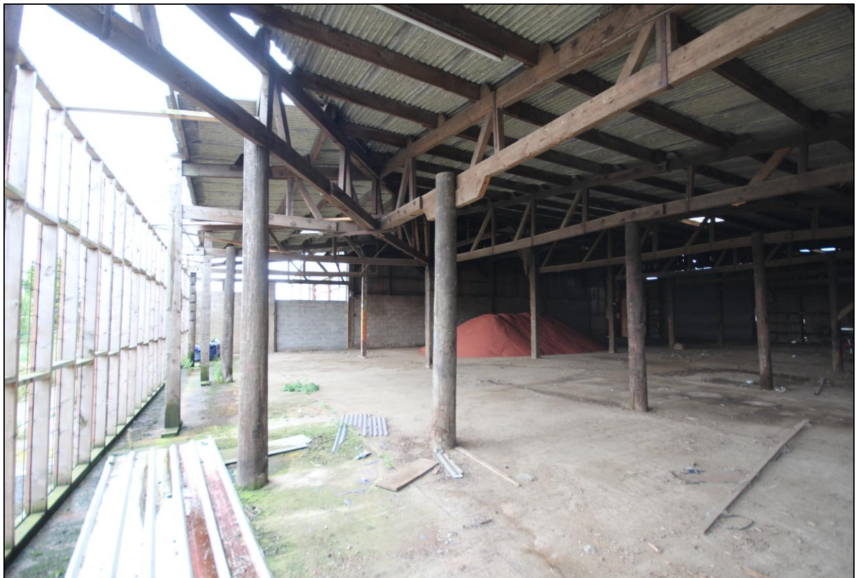
Figure 43: View of the interior of building I, facing east.
