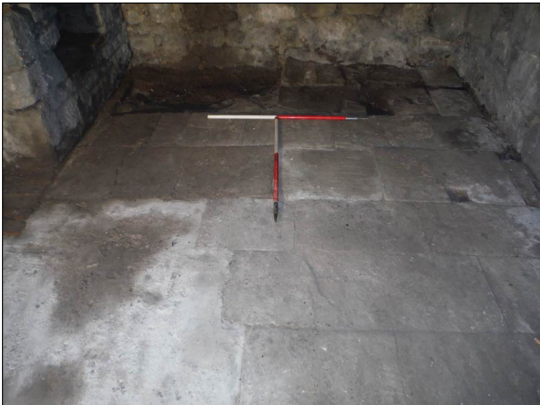
Figure 7. the flooring within the recess behind the stairs on the pele tower's ground floor. Scales = 2 x 1m.
