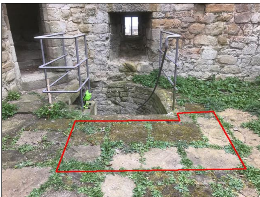
Figure 3. Location and extent of Test Pit 2.
