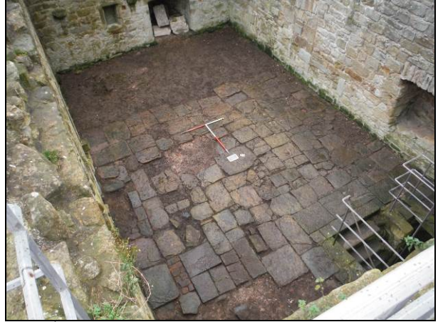
The 1 st floor of Cresswell Pele Tower, prior to the excavation of the test pits.
