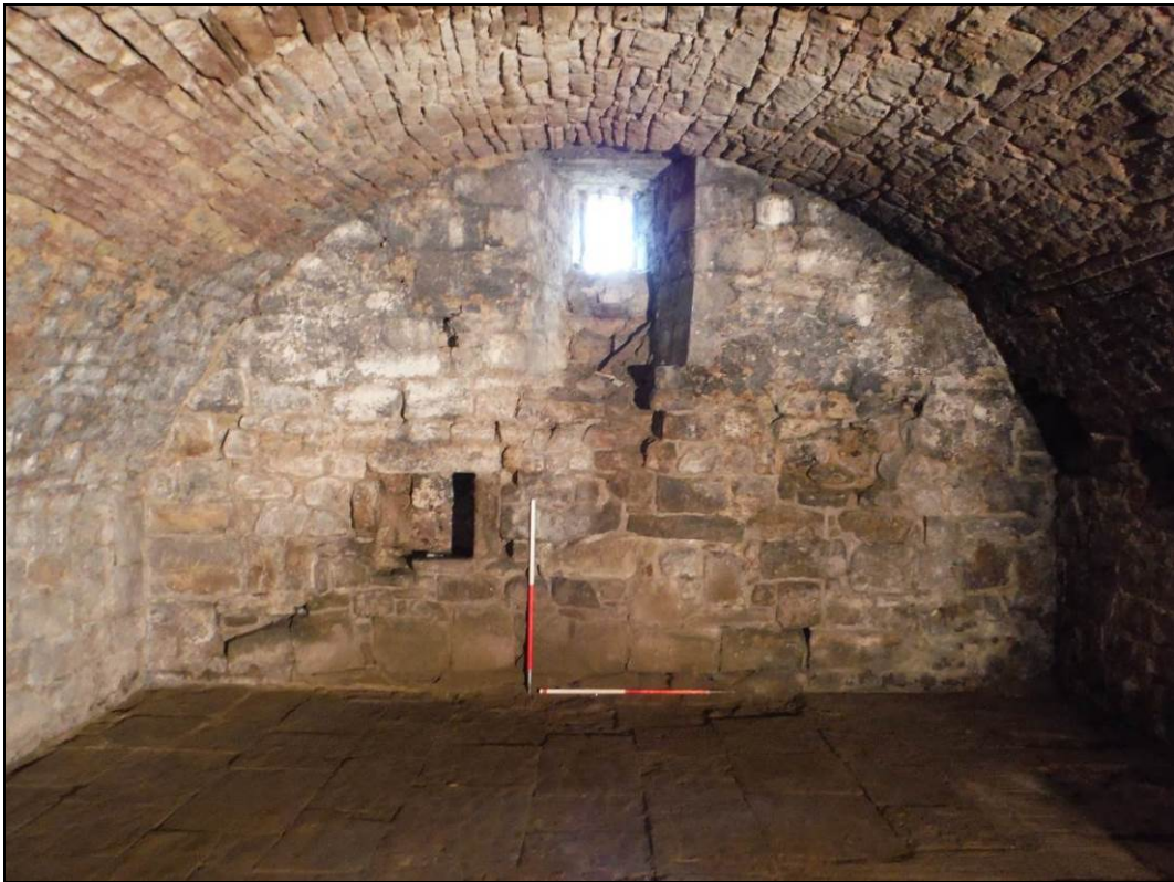
Figure 4. The south-western elevation of the pele tower's ground floor. Scales = 2 x 1m.
