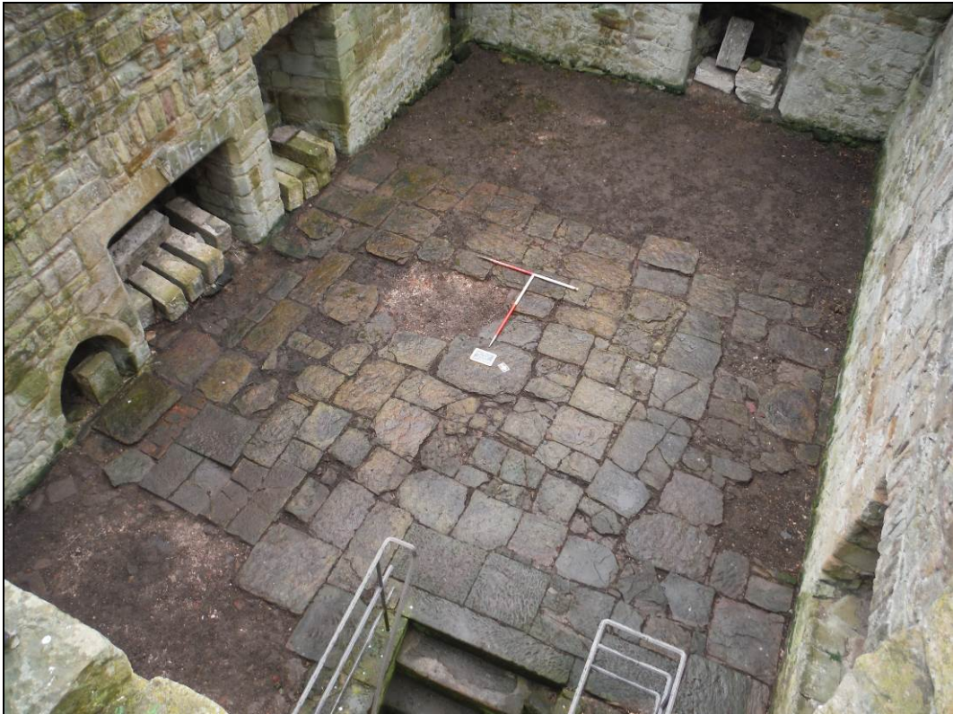
Figure 16. The first floor of the pele tower prior to excavation. Scales = 2 x 1m.
