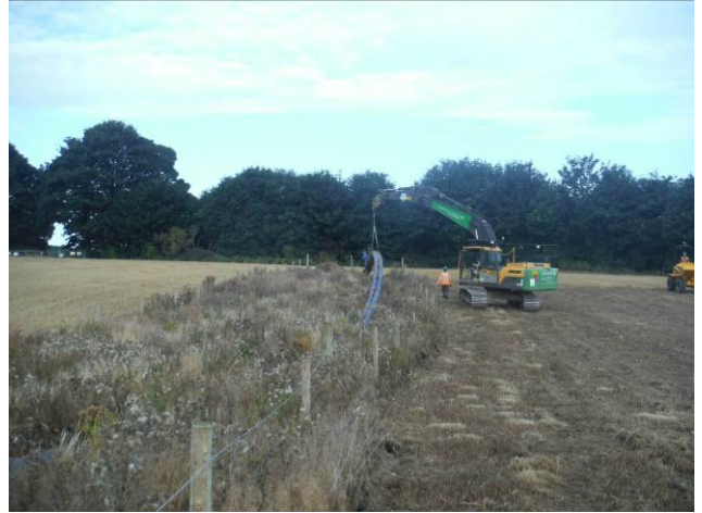
View north-west of the lifting of the temporary pipe replacement
