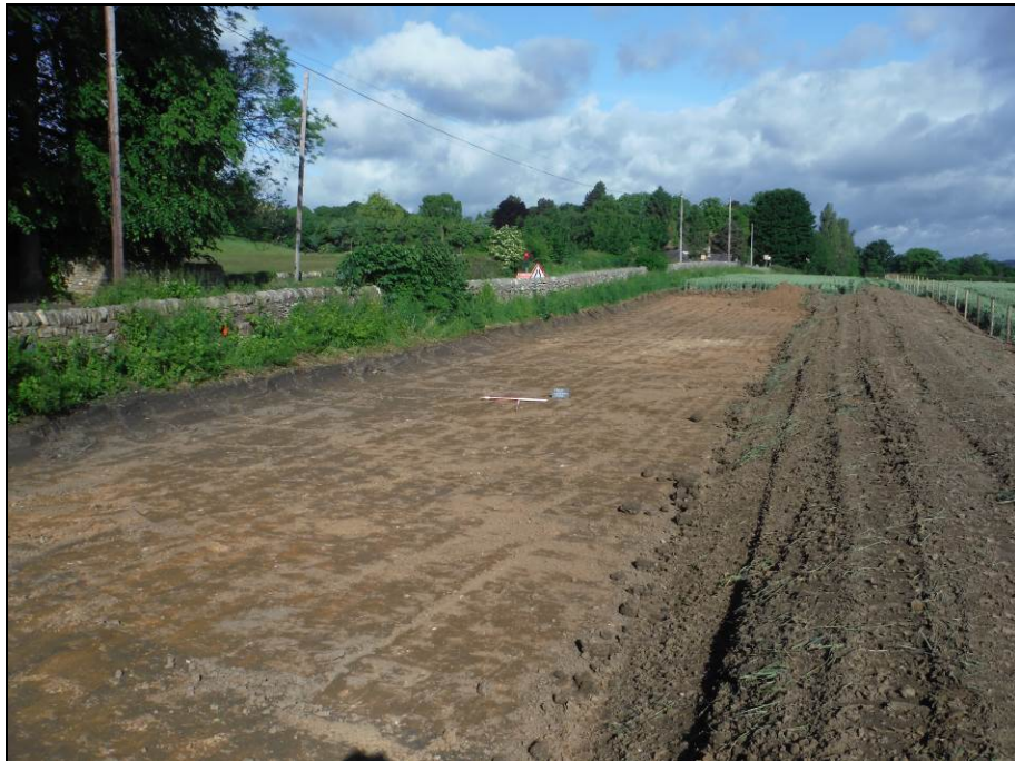
Figure 13. Overview of partially stripped area adjacent to road (scale = 0.5m graduations).
