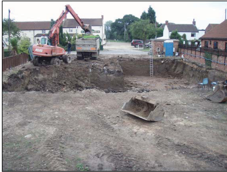
Fig. 5 View of the total area of the trench looking east.
