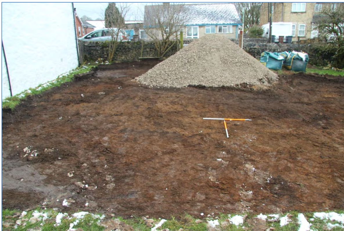
Figure 29: Footprint of excavation after removal of topsoil for siting sales cabin
