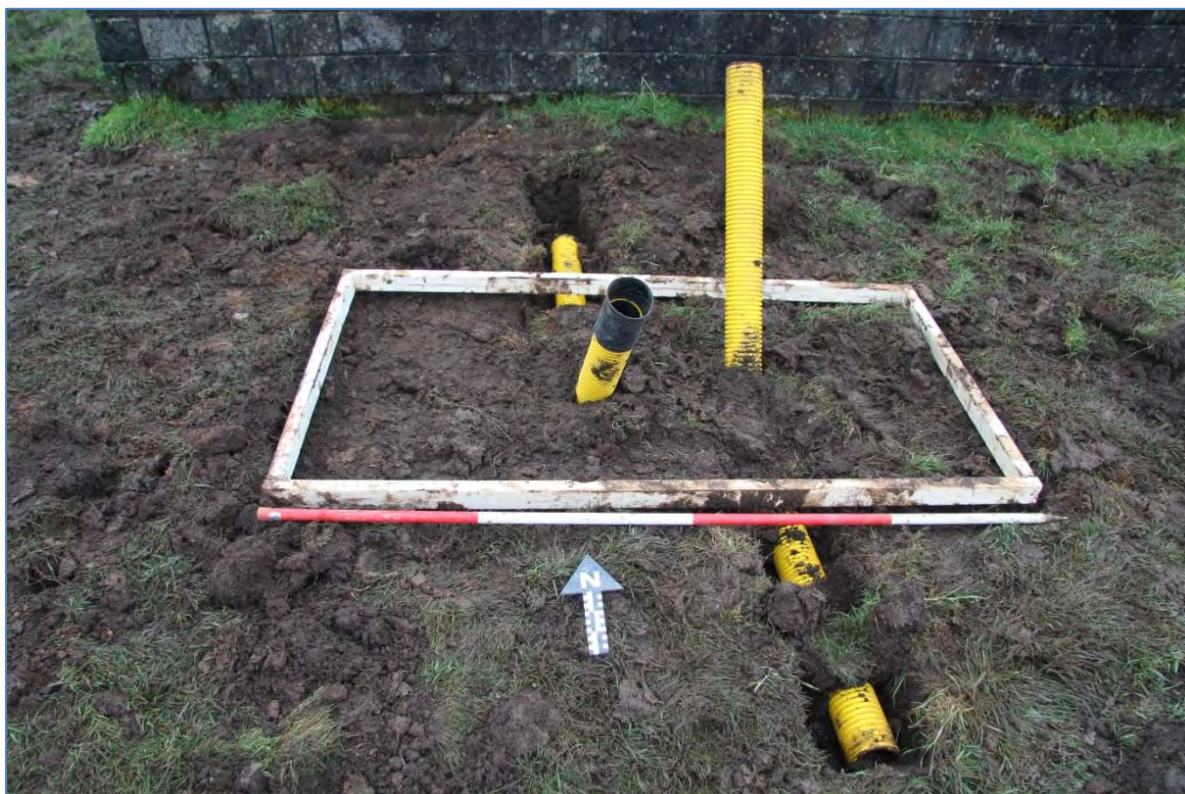
Figure 30: Excavations for Electricity Cable looking west
