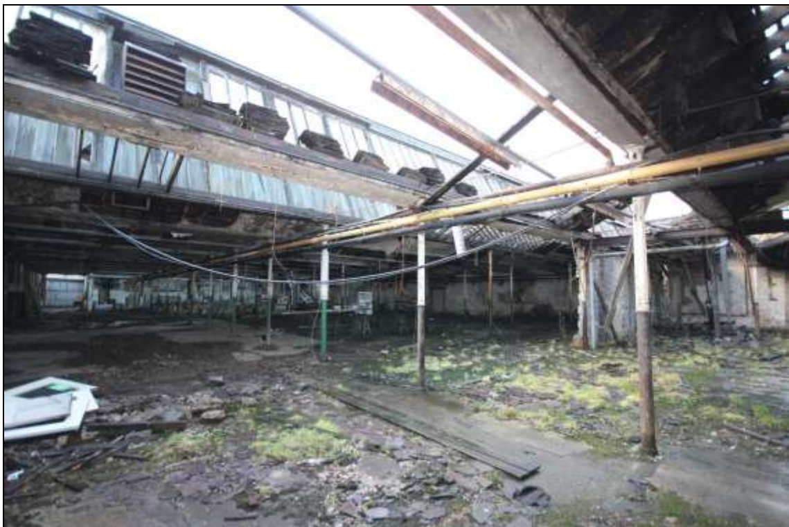
Figure 37: View of the former mule spinning shed, facing south west.
