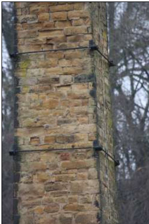
Figure 124: View of the southern elevation of the chimney.
