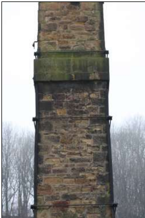
Figure 110: View of the northern elevation of the chimney.
