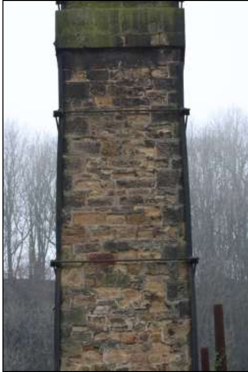
Figure 109: View of the northern elevation of the chimney.
