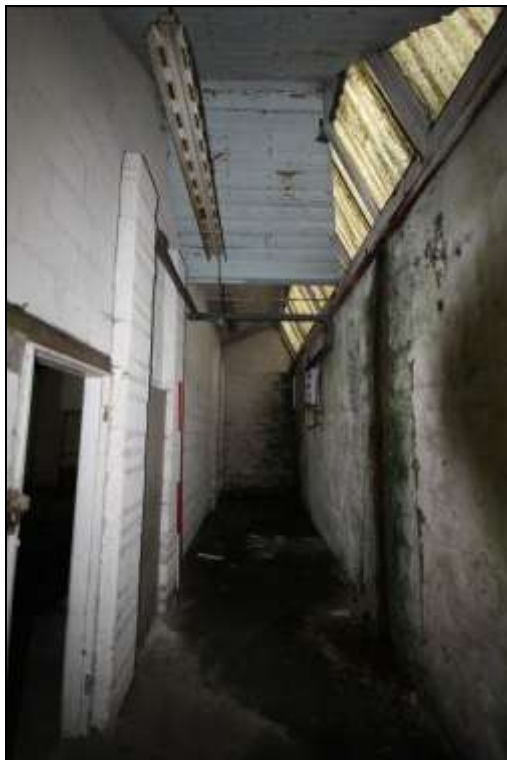
Figure 67: The insertion of a concrete breeze block wall has provided a separate room in the north east corner of the former mule spinning shed, 2m scale.
