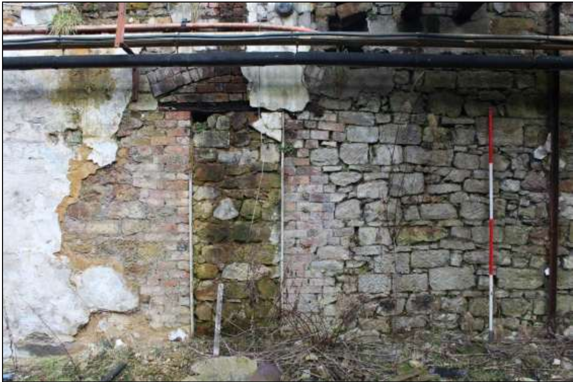
Figure 68: View of a modified aperture along the northern wall of the western section of the former mule spinning shed, 2m scale.
