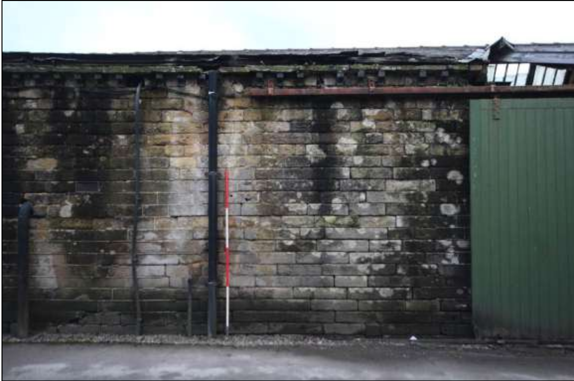
Figure 20: View of the coursed sandstone south elevation, 2m scale.
