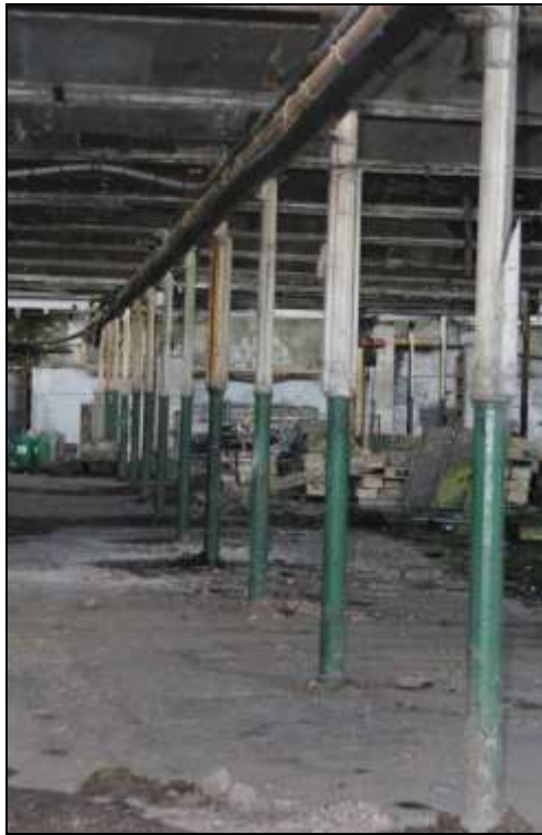
Figure 34: View of the cast-iron columns in the former mule spinning shed.
