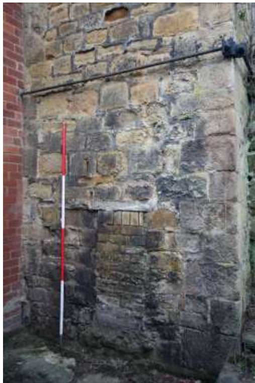
Figure 120: View of the southern elevation of the chimney, 2m scale.
