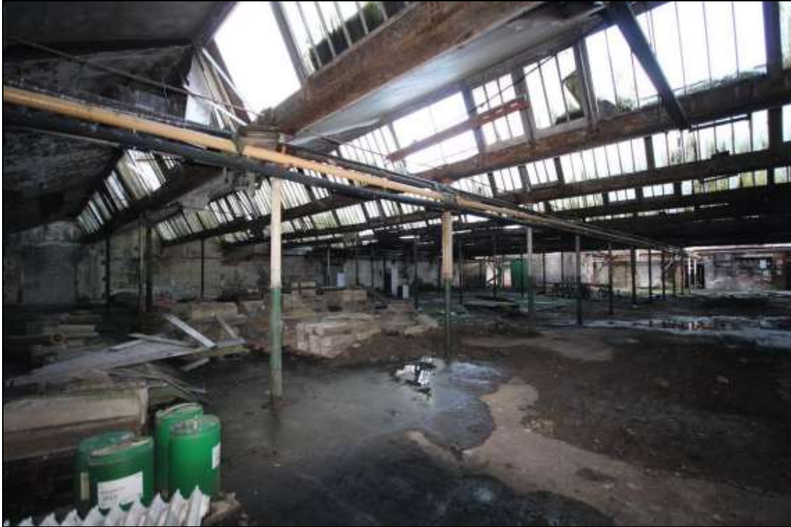
Figure 32: View of the former mule spinning shed, facing north west.
