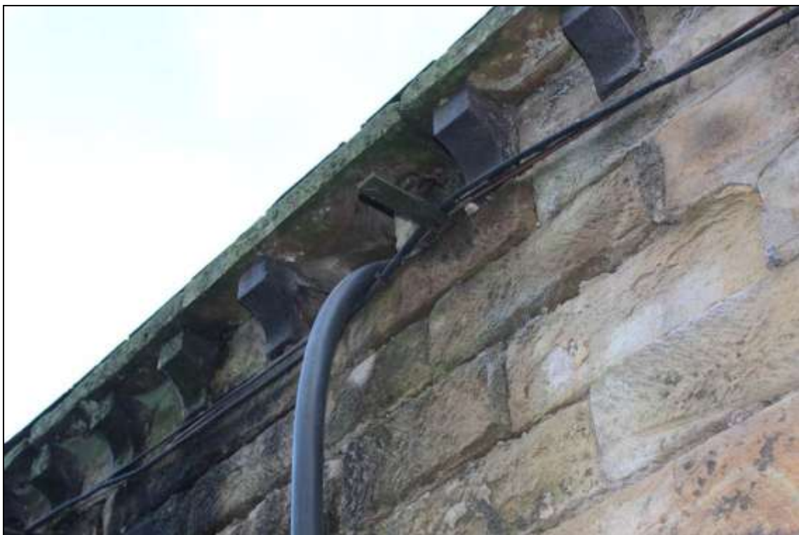
Figure 19: View of the dentilled verge along the southern elevation of the former mule spinning shed.
