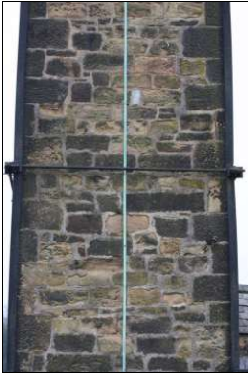
Figure 115: View of the eastern elevation of the chimney.
