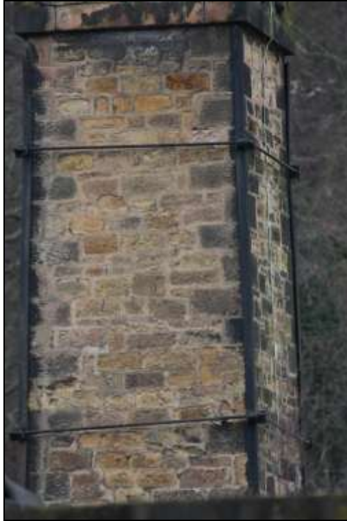
Figure 121: View of the southern elevation of the chimney.
