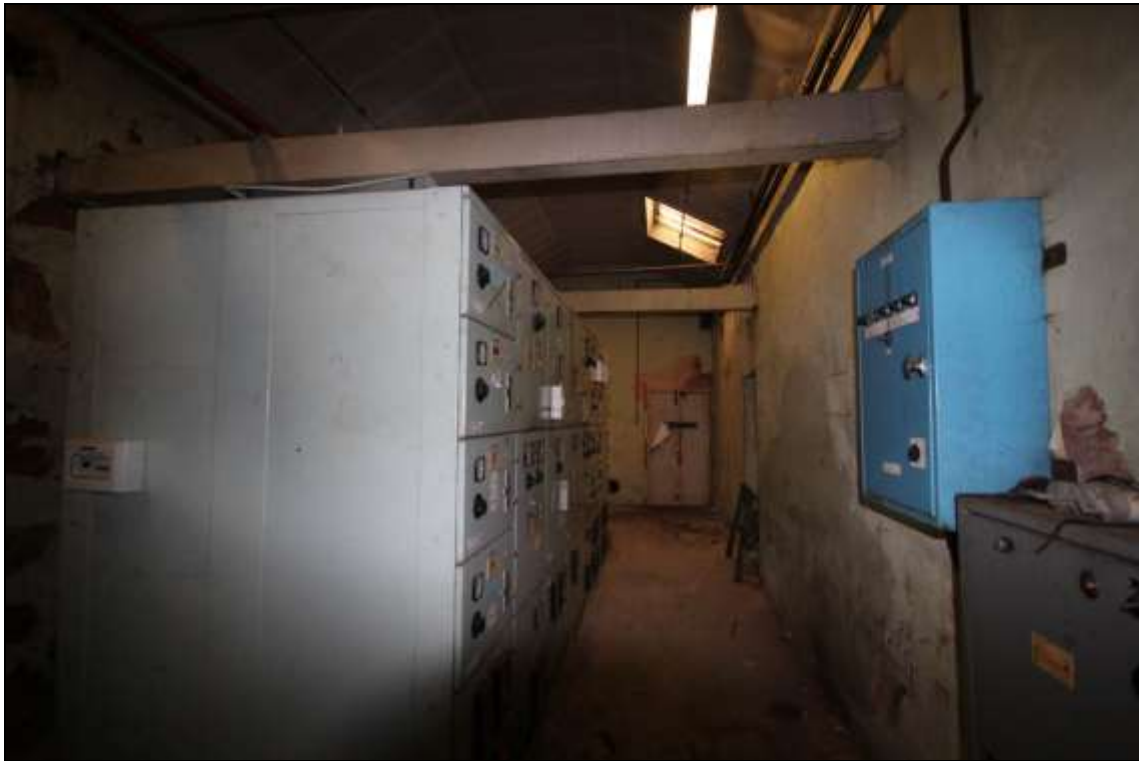
Figure 58: View of a western room adjacent to the mule spinning shed.
