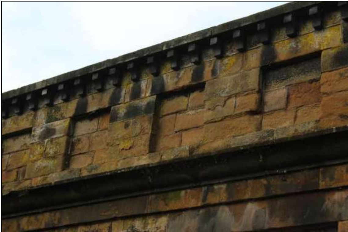
Figure 10: Detail of the squared blind recessed niches and blue dentilled brick verges.
