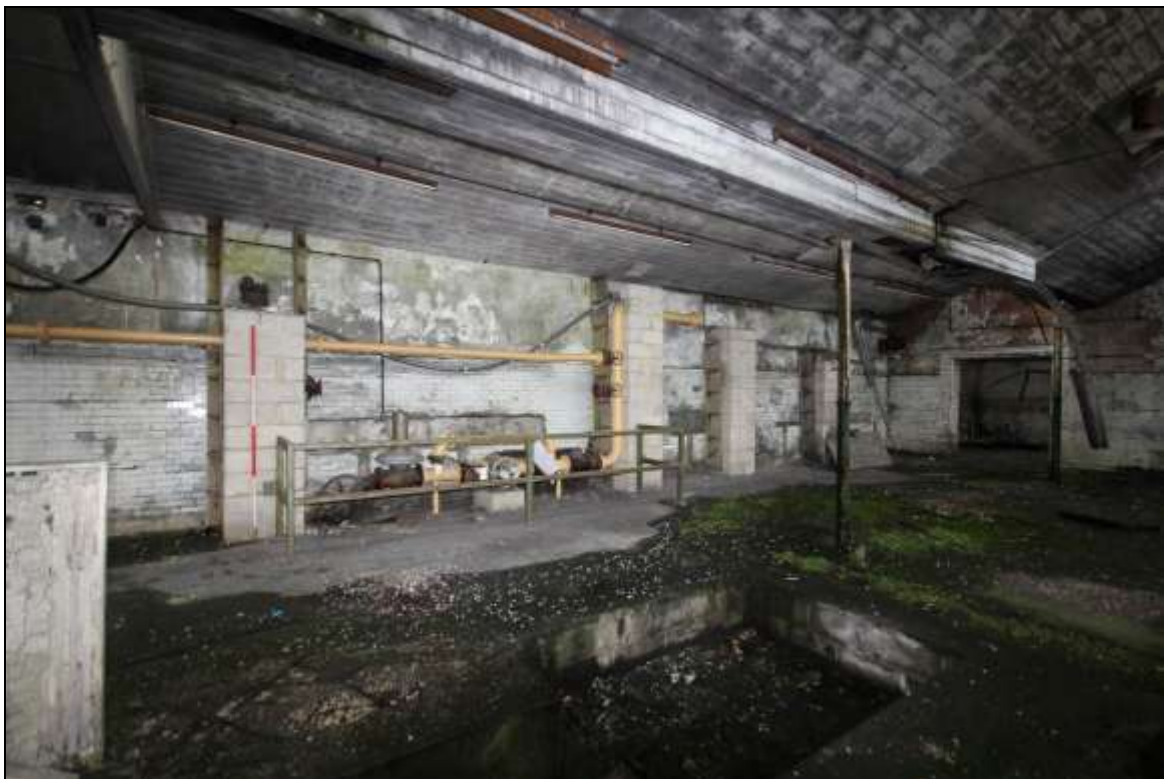
Figure 83: View of a section of the southern wall consisting of stone and a layer of glazed tiles, 2m scale.
