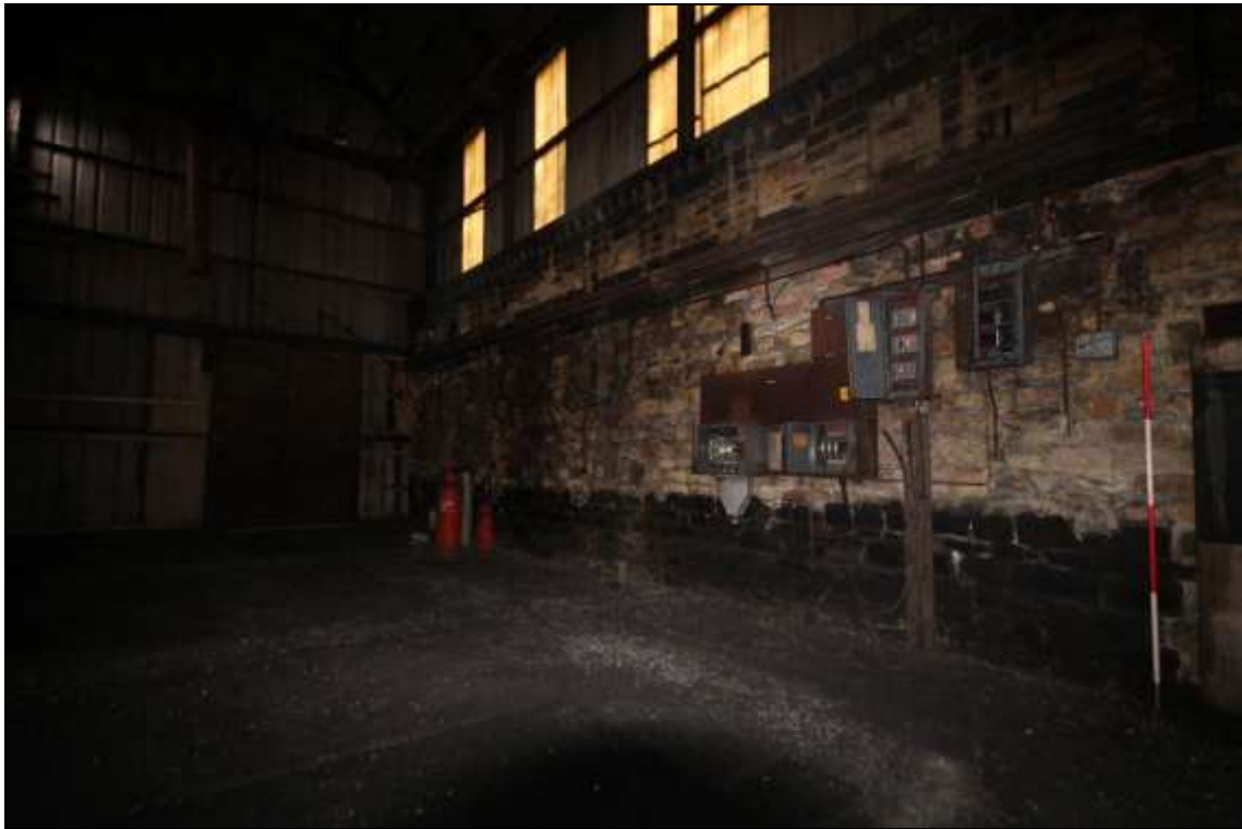
Figure 26: View of the western wall, facing north east, 2m scale.
