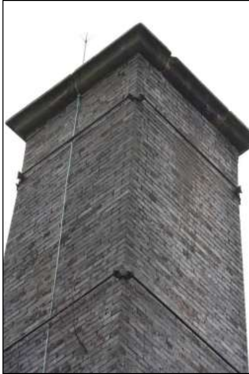
Figure 136: View of the western and southern elevations of the brick chimney.
