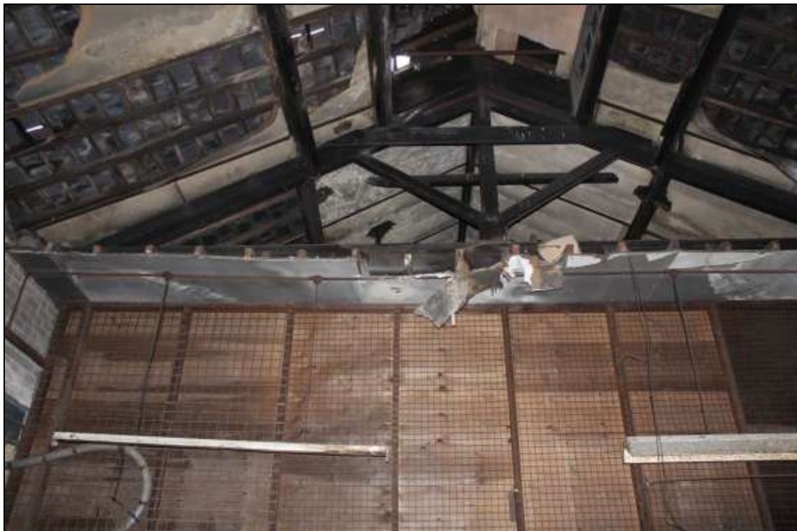
Figure 97: View of the internal roof structure of the retort house.
