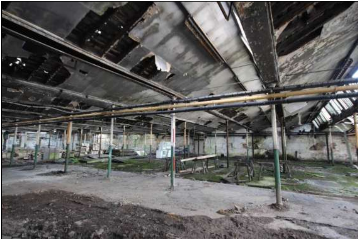
Figure 38: General view of the interior of the former mule spinning shed.
