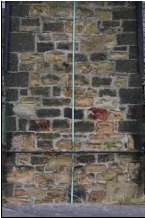
Figure 113: View of the eastern elevation of the chimney.
