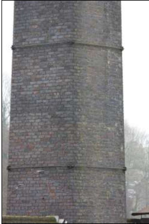
Figure 138: View of the north and east elevations of the brick chimney.
