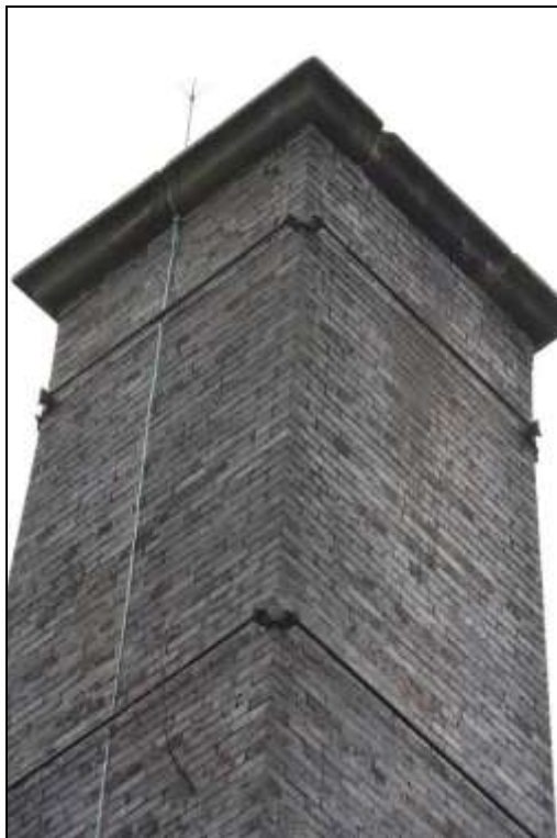
Figure 129: View of the west and south elevations of the brick chimney.
