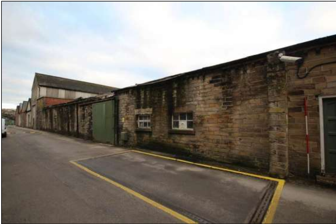
Figure 14: View of the southern elevation of the mule spinning shed, 2m scale.
