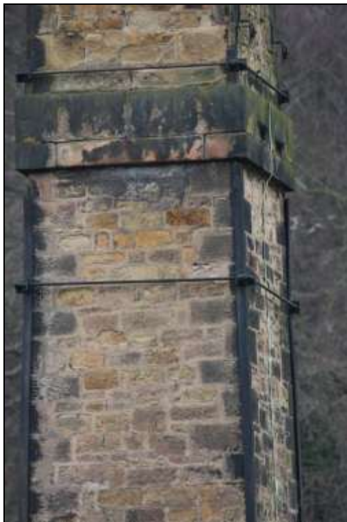
Figure 122: View of the southern elevation of the chimney.
