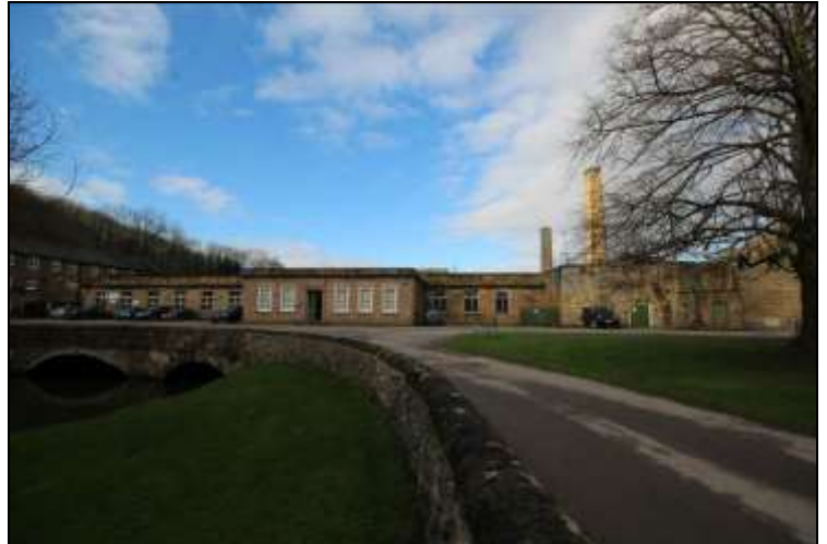
General view of the eastern façade of the former mule spinning shed and two chimneys at Riverside Business Park, Bakewell, Derbyshire.
