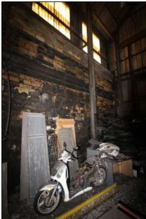
Figure 29: View of the southern section of the western elevation.
