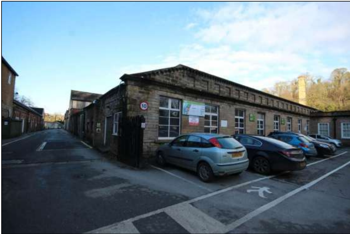
Figure 8: General view of the south eastern side of the former mule shed, facing north west.
