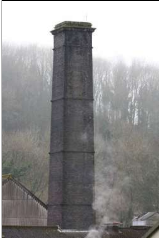
Figure 128: General view of the brick chimney.
