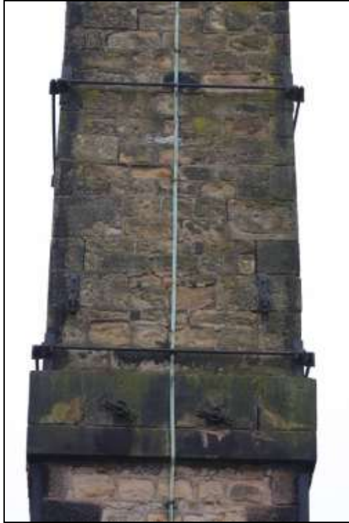
Figure 117: View of the eastern elevation of the chimney.
