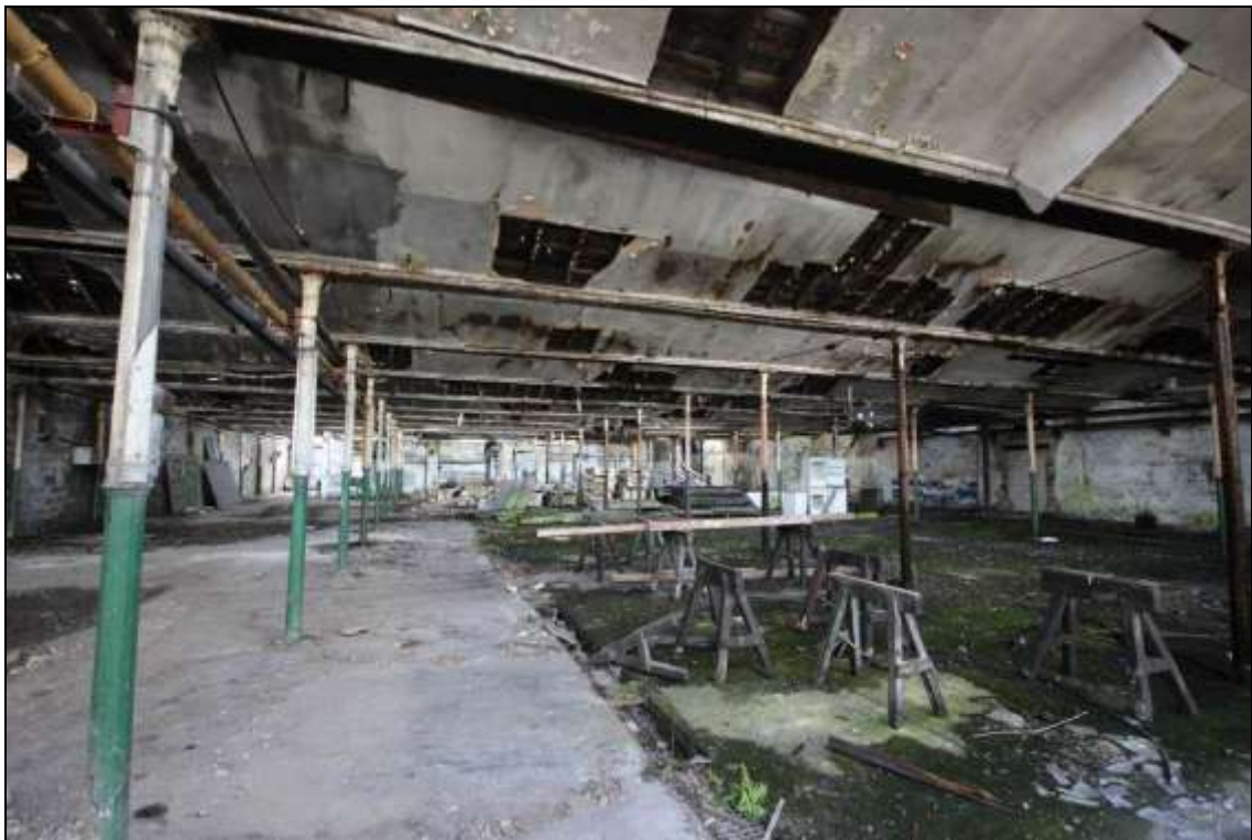
Figure 41: View of the former mule spinning shed, facing north.
