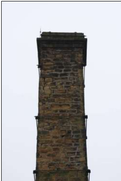
Figure 112: View of the northern elevation of the chimney.
