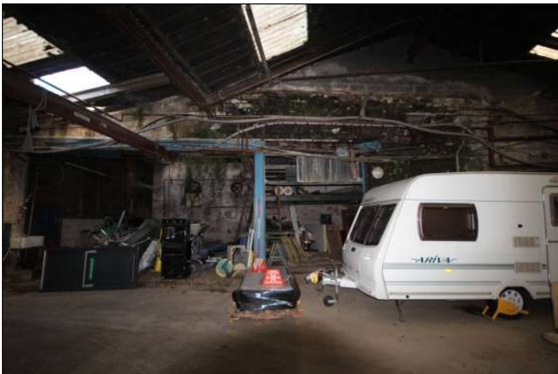
Figure 95: View of the modified western elevation, 2m scale.
