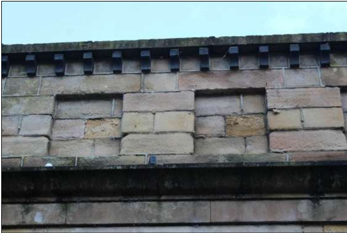
Figure 6: View of the parapet decoration along the eastern elevation.
