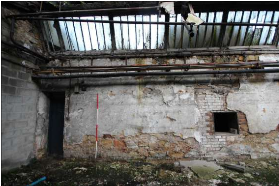
Figure 71: View of modified apertures along the northern wall, 2m scale.
