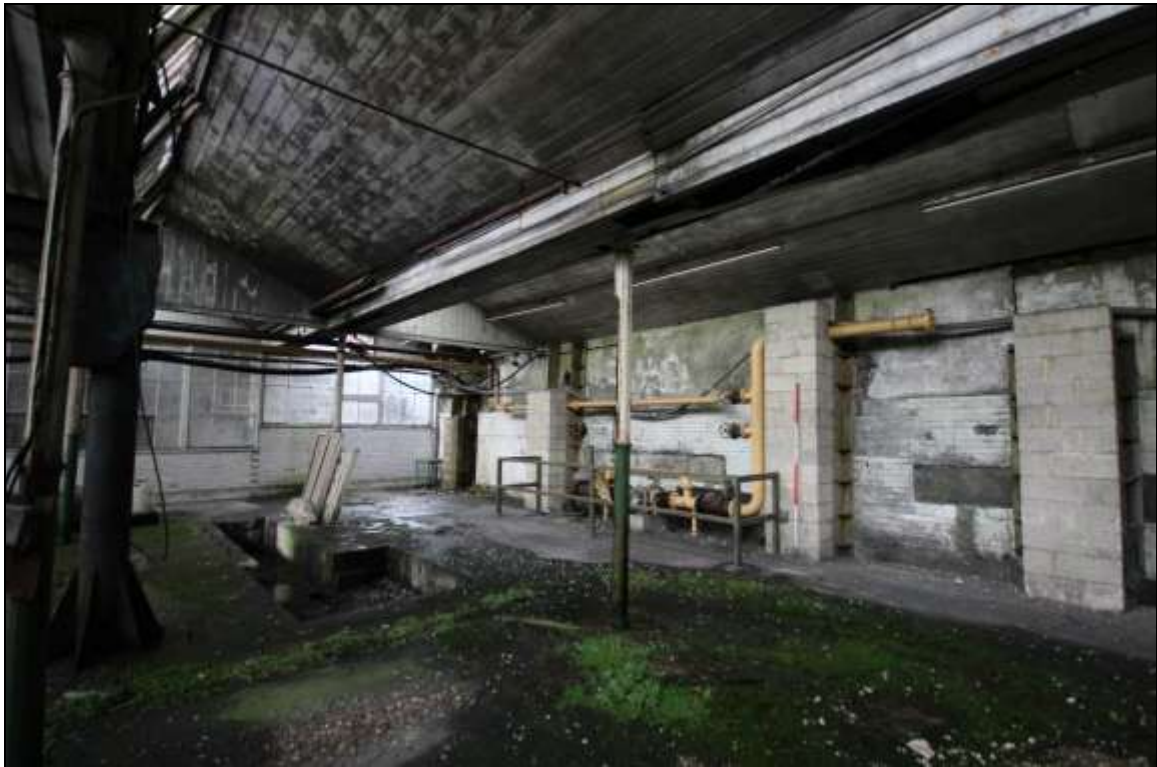
Figure 82: View of the southern wall, facing south east, 2m scale.
