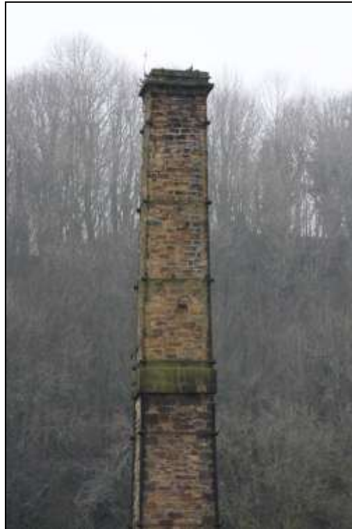
Figure 106: General view of the northern elevation of the stone chimney.
