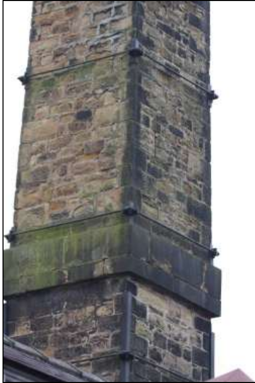
Figure 125: View of the western elevation of the chimney.
