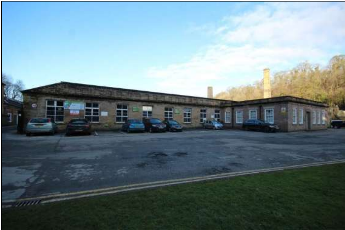
Figure 2: General view of the former mule spinning shed.
