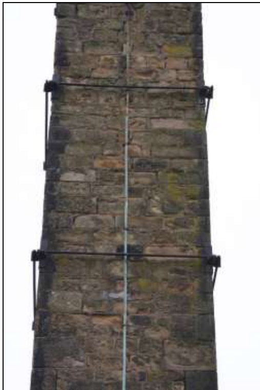
Figure 118: View of the eastern elevation of the chimney.
