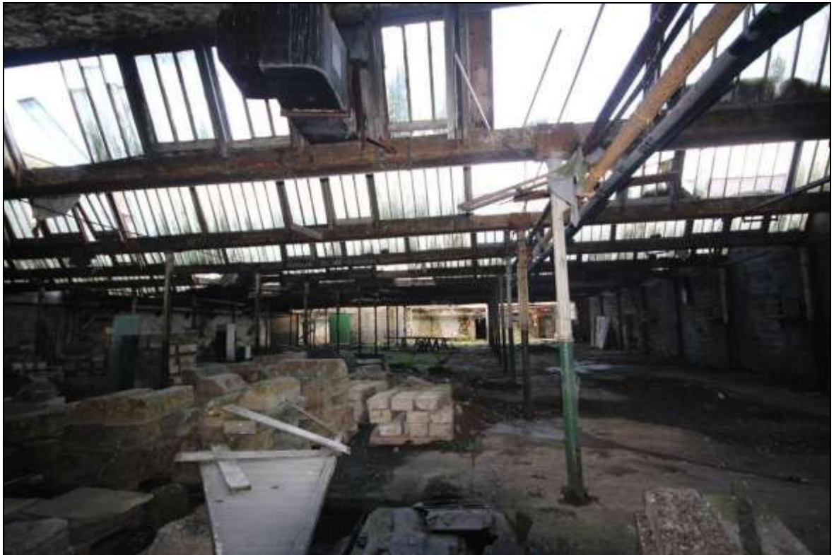
Figure 40: View of the former mule spinning shed facing north.
