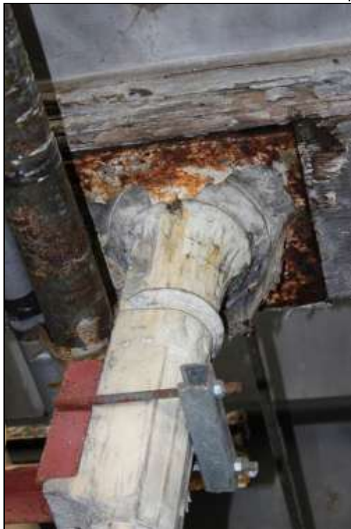
Figure 45: View of a capital of one of the cast-iron columns.
