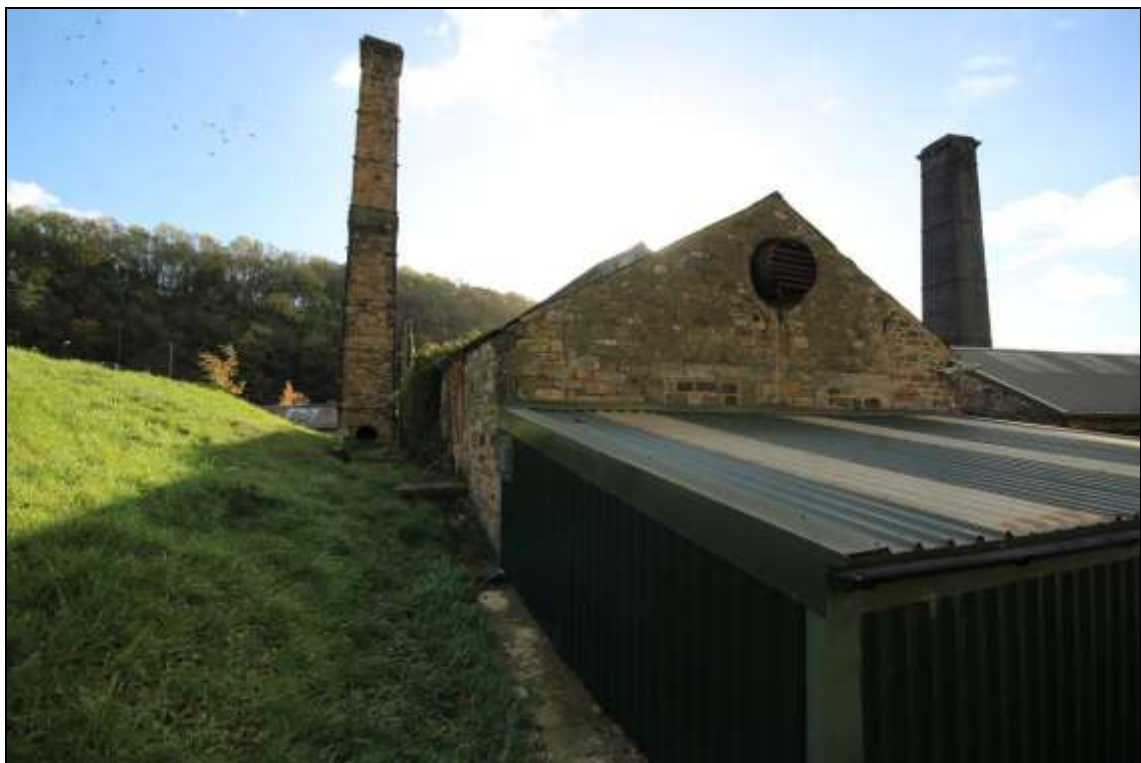
Figure 87: General view of the retort house, facing south west, 2m scale.
