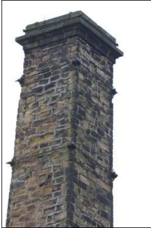
Figure 127: View of the western elevation of the chimney.
