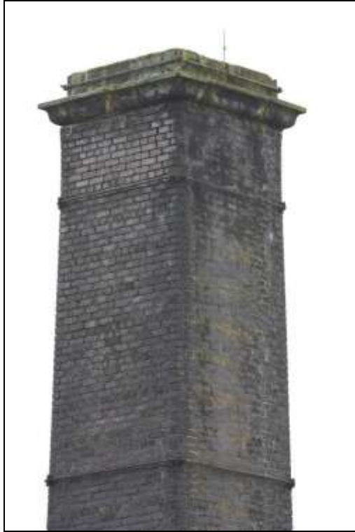
Figure 140: View of the brick chimney at Riverside Business Park, Bakewell.
