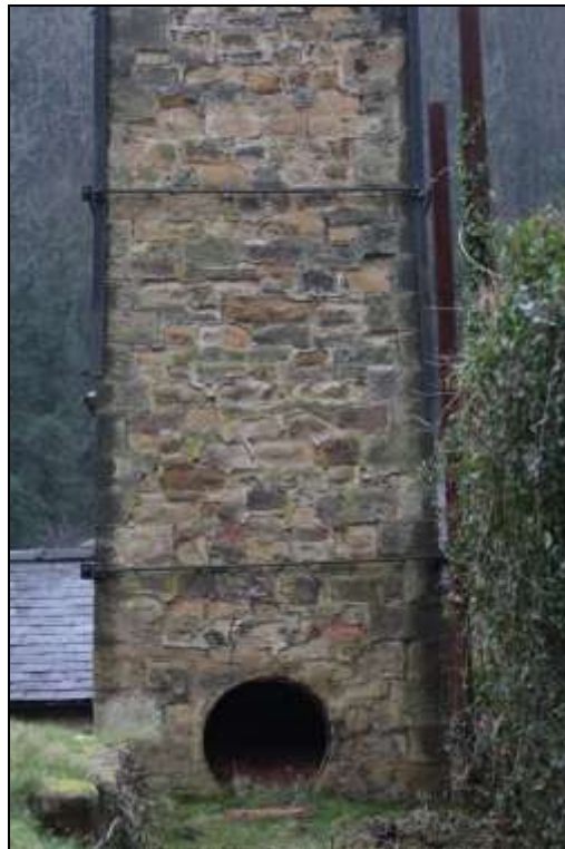
Figure 107: View of the northern elevation of the chimney.
