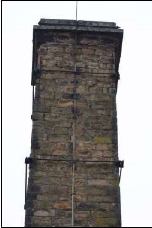
Figure 119: View of the eastern elevation of the chimney.
