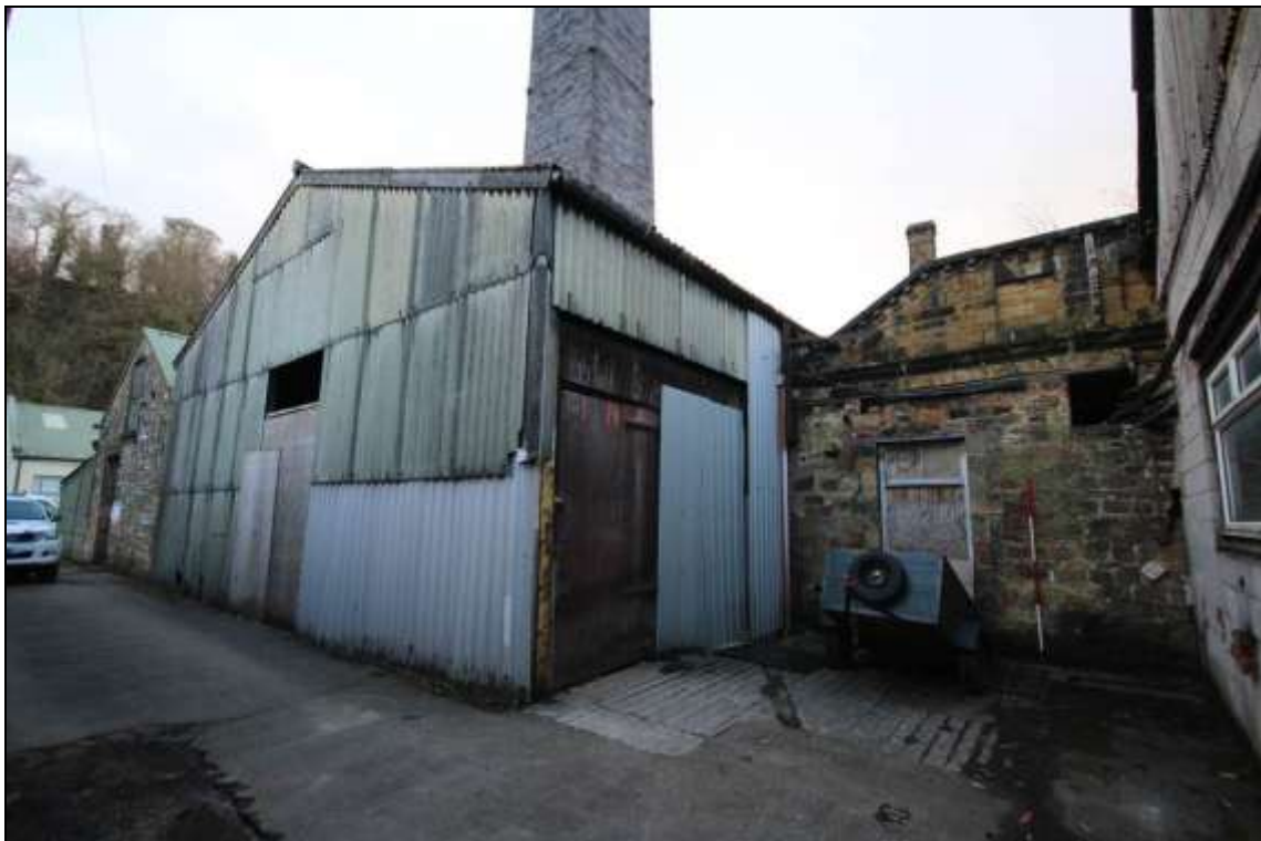
Figure 23: View of a segment of the western elevation of the former mule spinning shed with sloped parapet edge, 2m scale.
