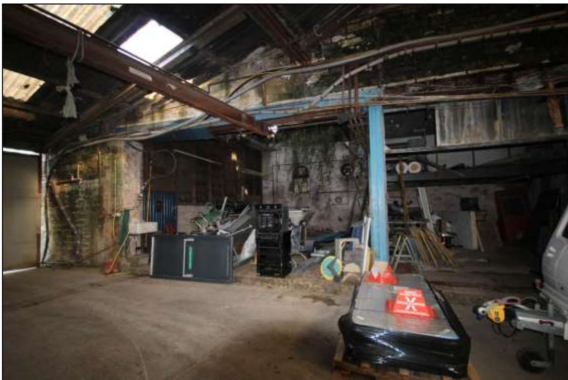
Figure 93: View of the heavily modified western elevation of the retort house.
