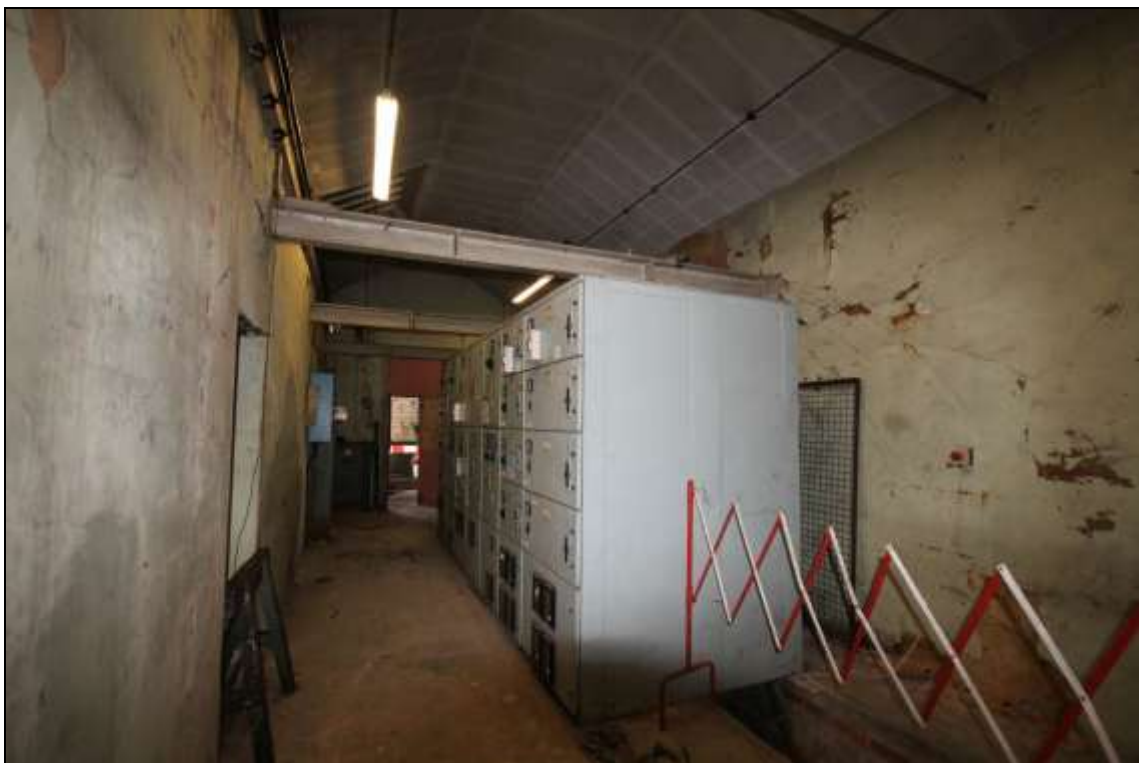
Figure 57: View of a room situated to the west of the former mule spinning shed.
