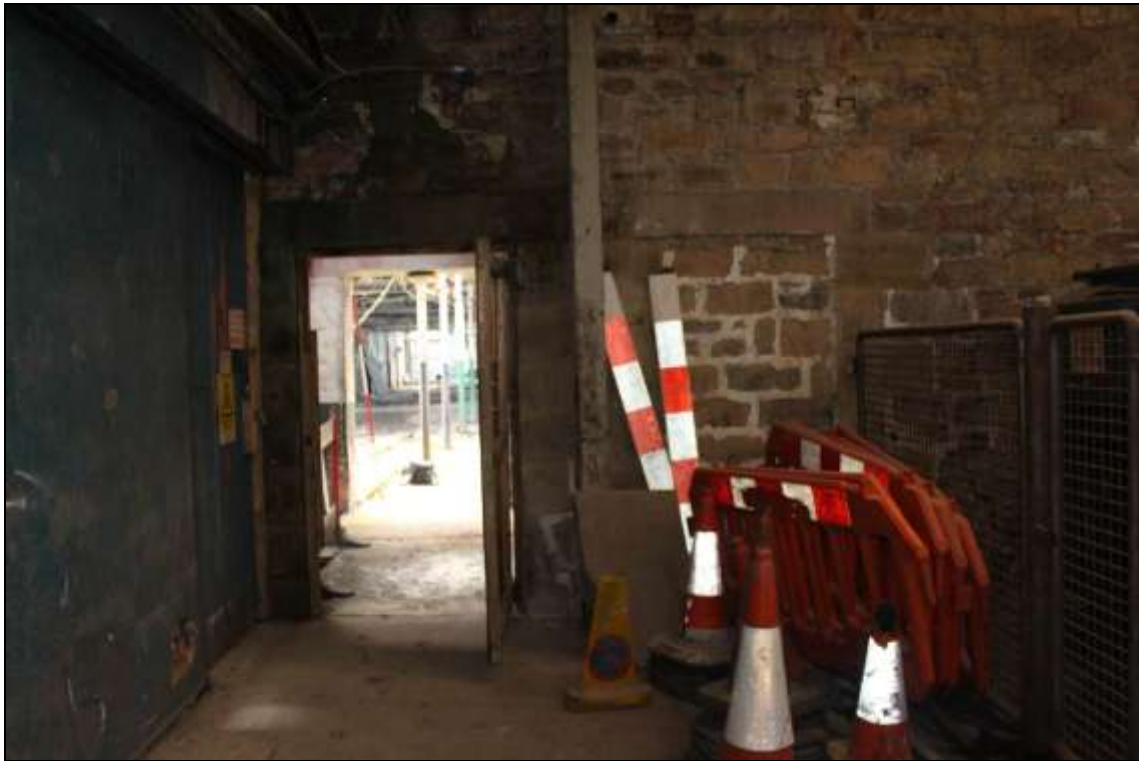
Figure 22: View of a blocked aperture along the northern elevation.
