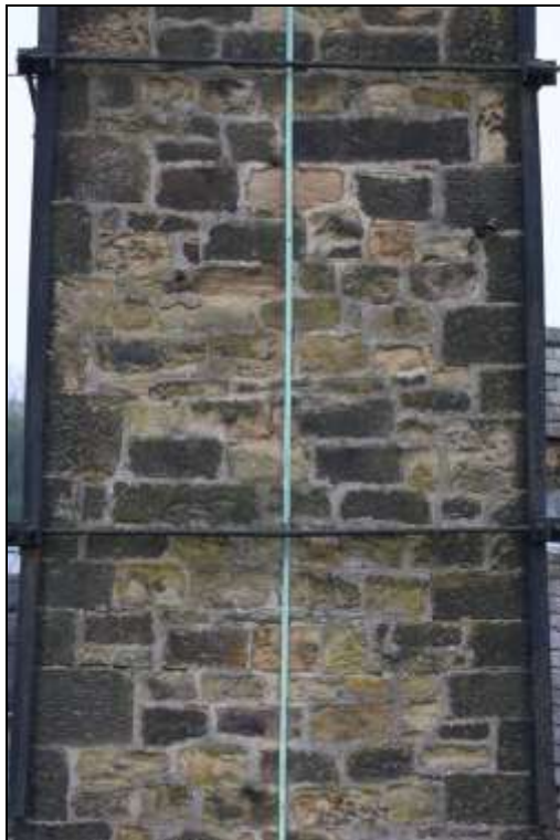
Figure 114: View of the eastern elevation of the chimney.
