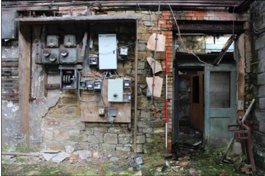
Figure 70: View of later inserted doorway leading into the former plan room, 2m scale.
