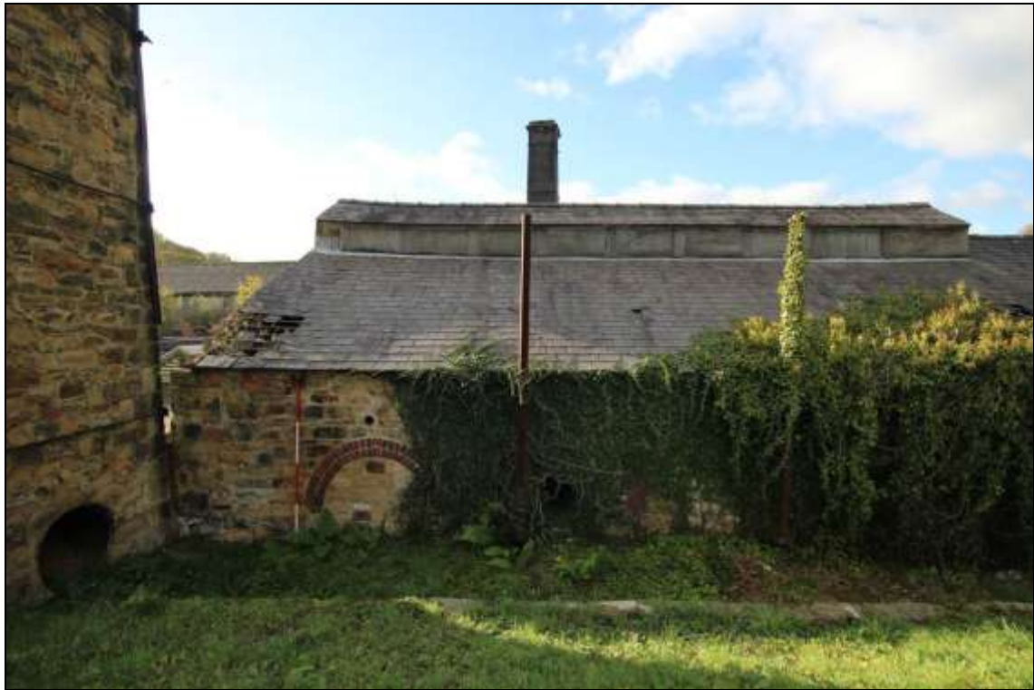
Figure 90: View of the eastern elevation with rounded brick arch, 2m scale.
