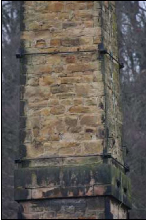
Figure 123: View of the southern elevation of the chimney.
