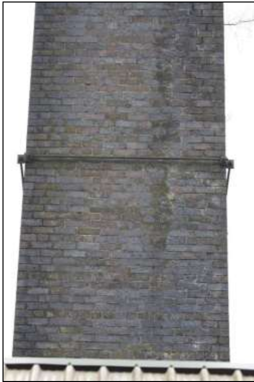
Figure 134: View of the northern elevation of the brick chimney.
