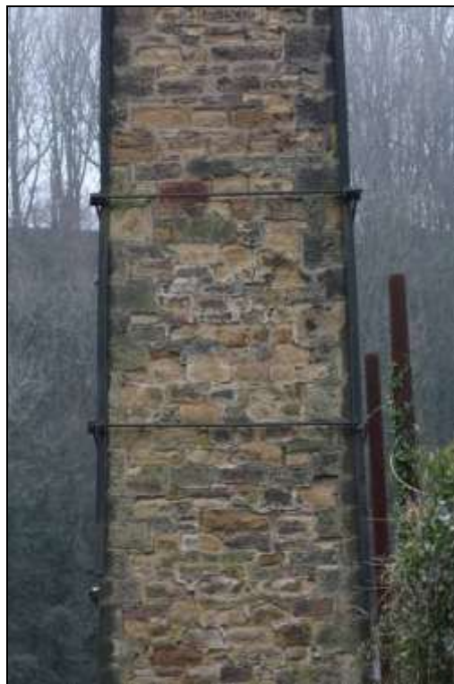
Figure 108: View of the northern elevation of the chimney.
