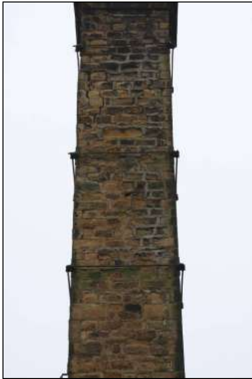
Figure 111: View of the northern elevation of the chimney.
