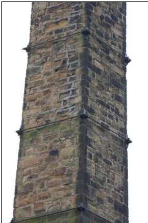
Figure 126: View of the western elevation of the chimney.
