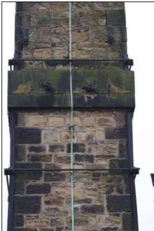
Figure 116: View of the eastern elevation of the chimney.
