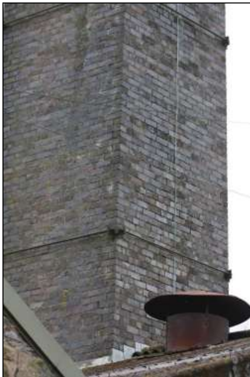
Figure 137: View of the western and northern elevations of the brick chimney.
