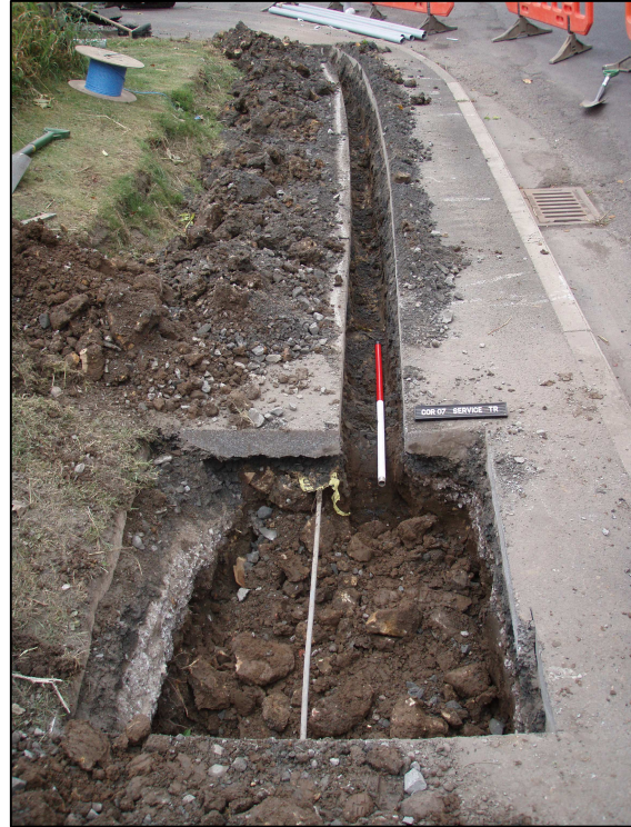
General shot of trench, looking west
