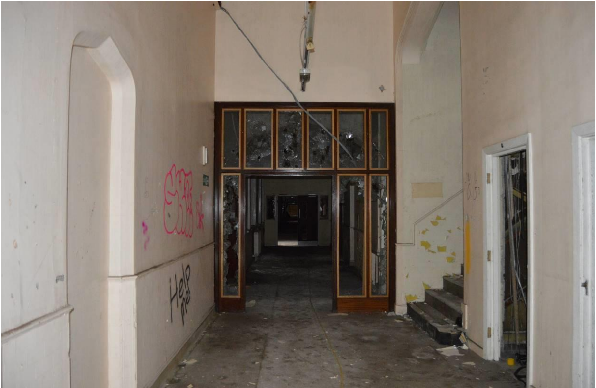
Plate 91.1: Tudor arch entrances to east pavilion ward, ground floor lobby facing south west.
