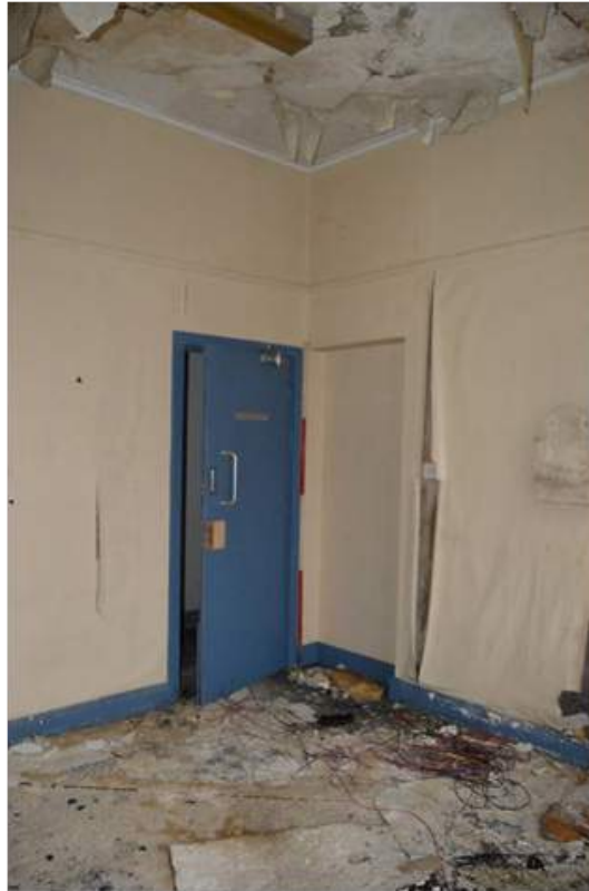
Plate 43.4: Late doorway next to blocked original opening. Scale 2m.
