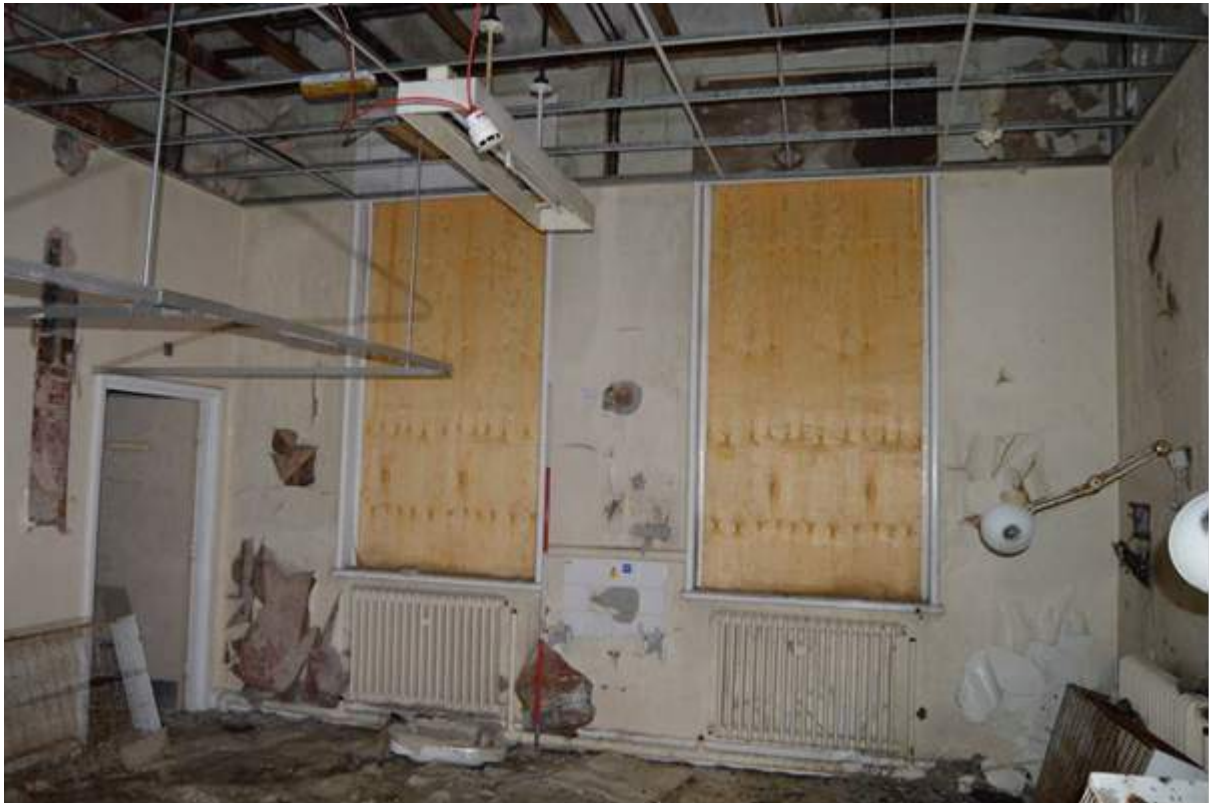
Plate 86.2: Front elevation of the board room. Scale 2m.
