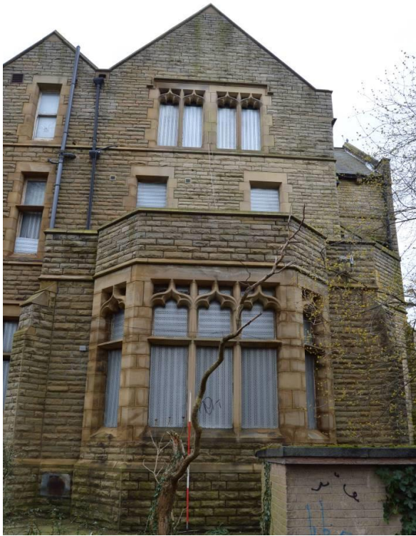
Plate 100.3: View of east elevation section, facing south west. Scale 2m.
