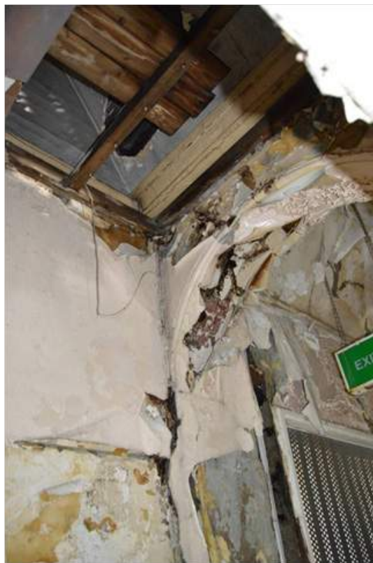
Plate 59.2: Remains of light well above lobby.
