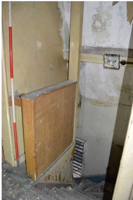
Plate 68: View towards staircase to section of second floor accommodation. Scale 2m.
