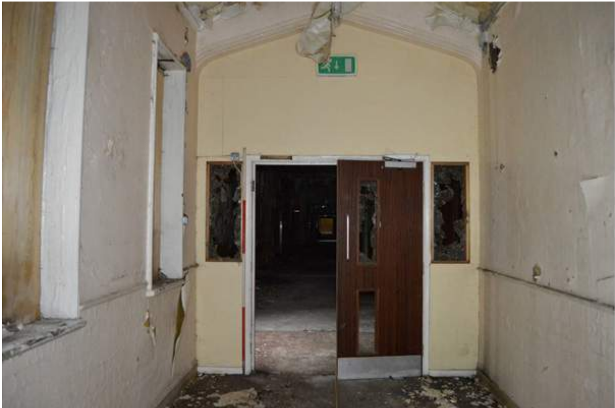
Plate 88.2: Blocked in Tudor style arch, view facing west in axial corridor. Scale 2m.
