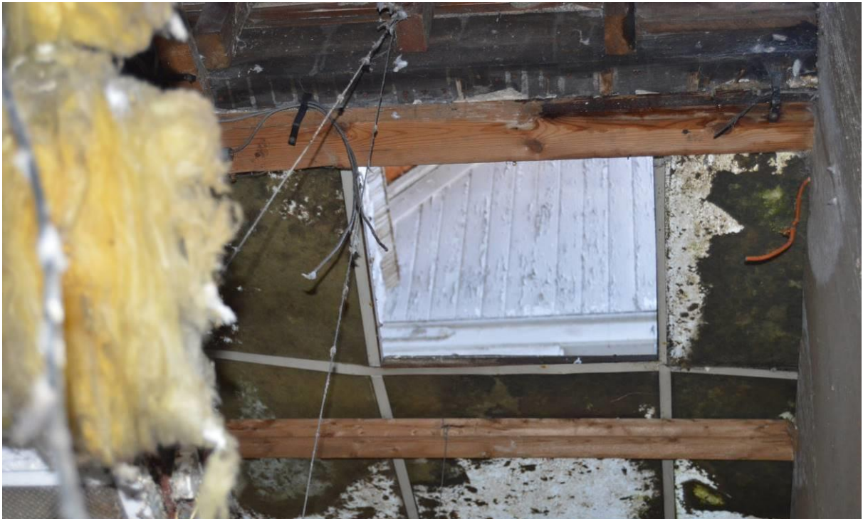
Plate 89.3: Operating theatre skylight in situ above later suspended ceiling (facing north west).
