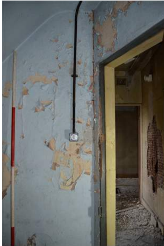
Plate 68.7: View from within room S10. Scale 2m.
