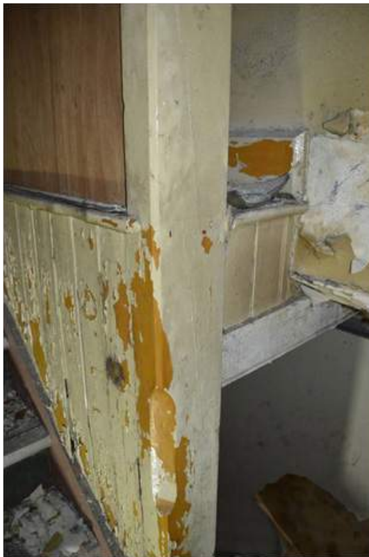
Plate 52.4: Stairs to the west of the nurses' accommodation.
