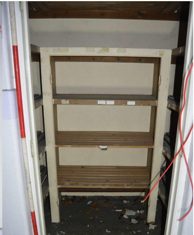
Plate 104.10: Airing cupboard off X-ray corridor (facing south east). Scale 2m.
