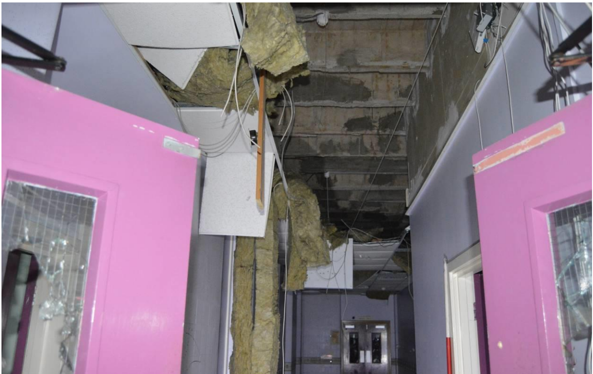
Plate 105.11: The Ann Canning Childs' ward was constructed of cast re-enforced concrete and steel framing (facing south west).
