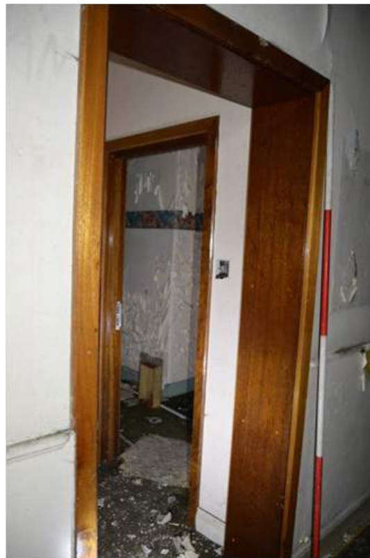
Plate 26: Modern doorway into matron's room G4. Scale 2m.
