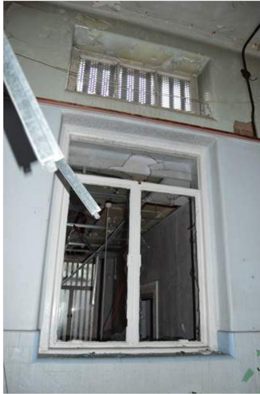
Plate 104.7: Detail of X-ray corridor window with internal and upper lights.
