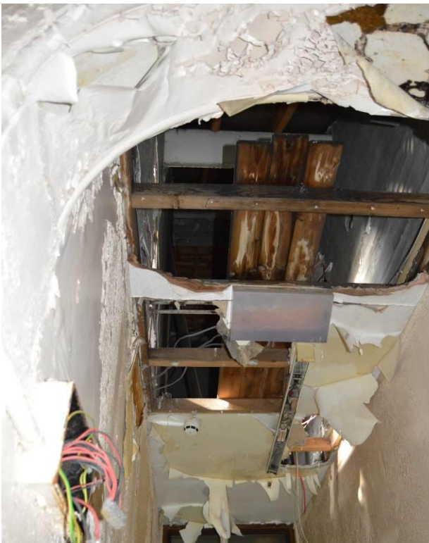
Plate 59.3: View through the later ceiling of the lobby. Facing north west.
