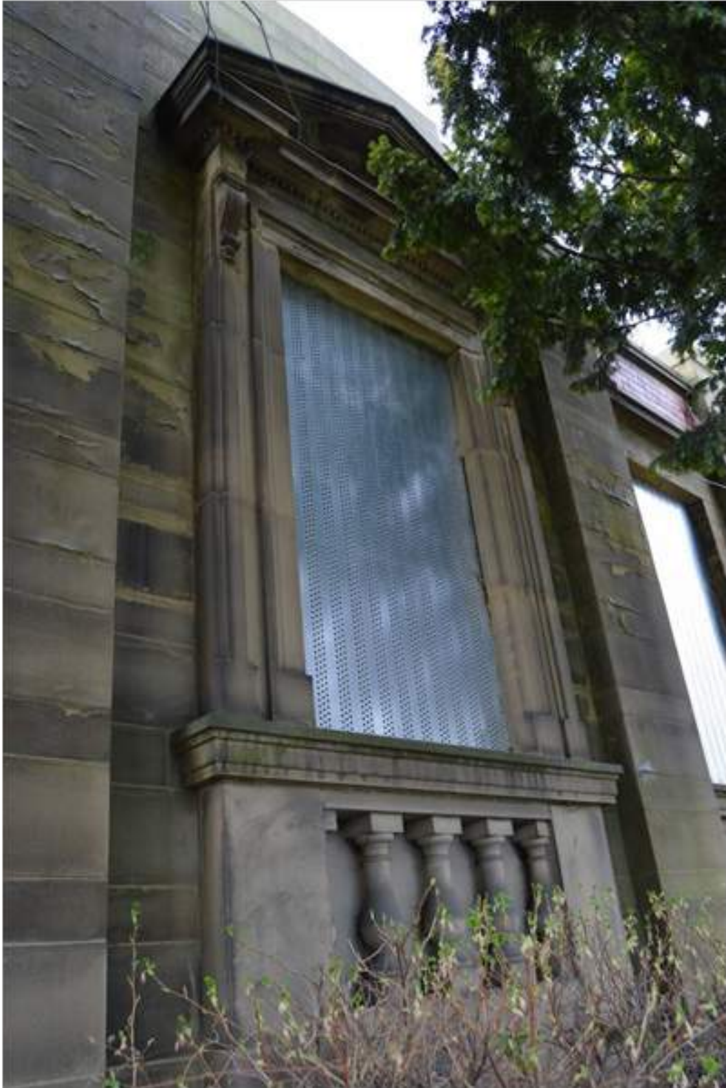
Plate 104: Stone façade pediment window surround to X-Ray wing.
