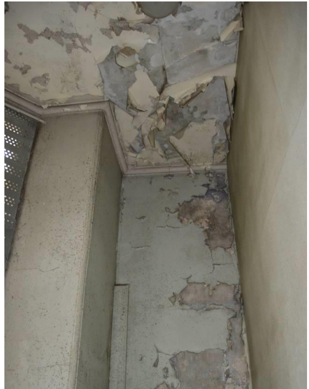
Plate 38.2: Retained beaded cornice above modern partitions. Facing north east.
