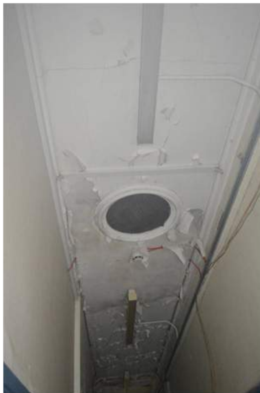
Plate 46: View of nurses' corridor ceiling vent.
