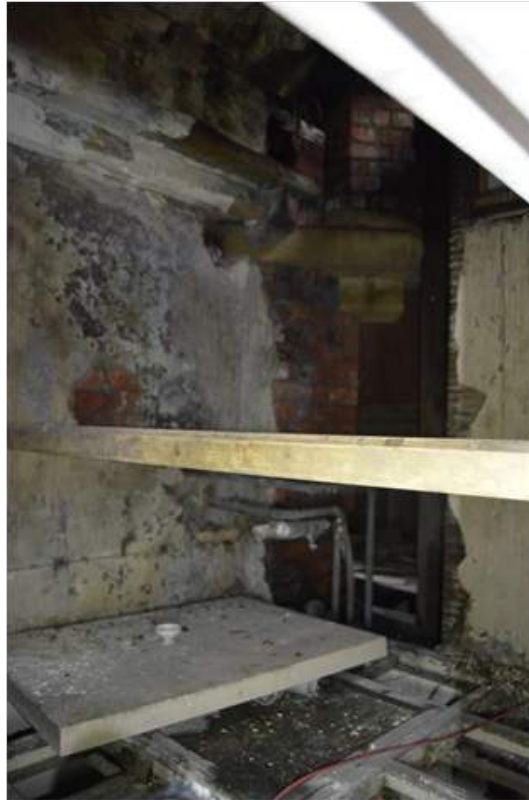
Plate 61.6: Chamfered timber handrail.
