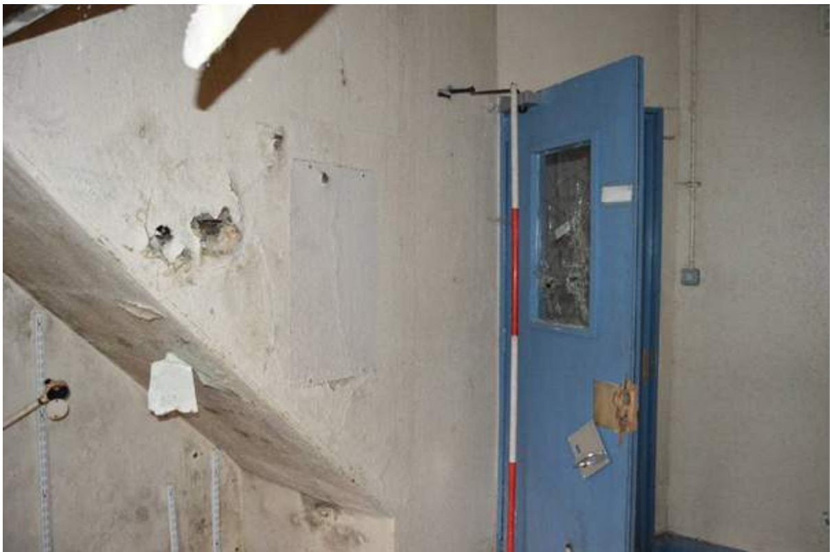
Plate 55.2: Inserted stair enclosure in F13. Scale 2m.
