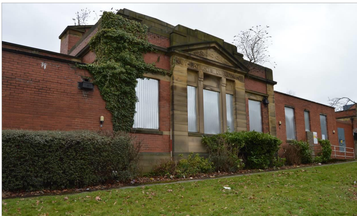
Plate 102: East façade to Out-patients Department, facing west. Scale 2m.
