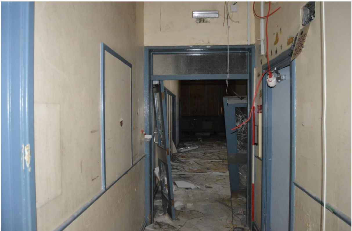
Plate 92.2: Lobby prior entry to the ward (facing south east). Scale 2m.
