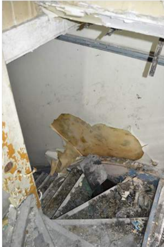
Plate 52.3: Stairs to the west of the nurses' accommodation.
