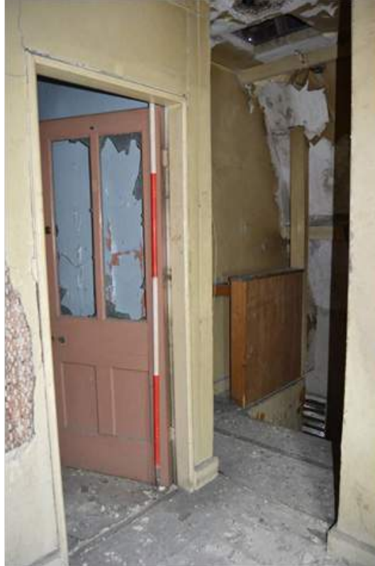
Plate 68.9: Half-glazed door to room S12. Scale 2m.
