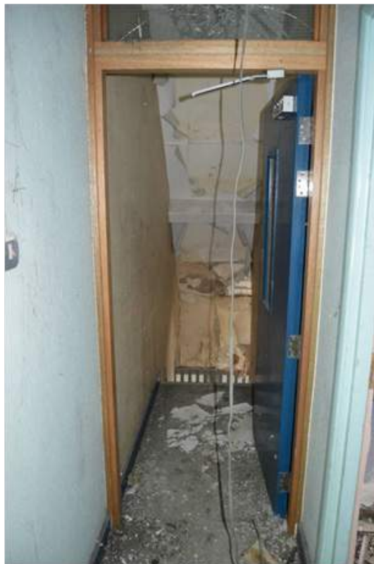
Plate 67.2: Modern fire door inserted into S4.
