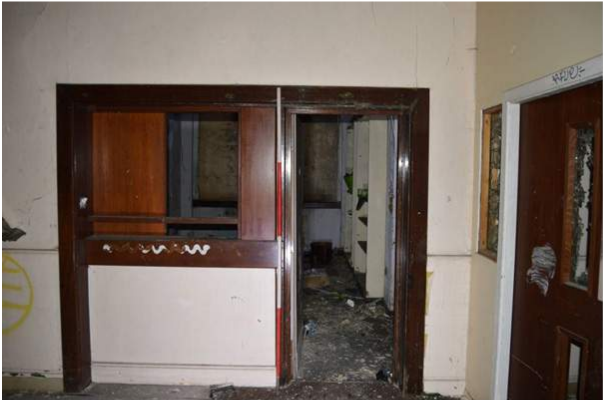
Plate 32: Counter/hatch and entrance from corridor into room G8. Scale 2m.
