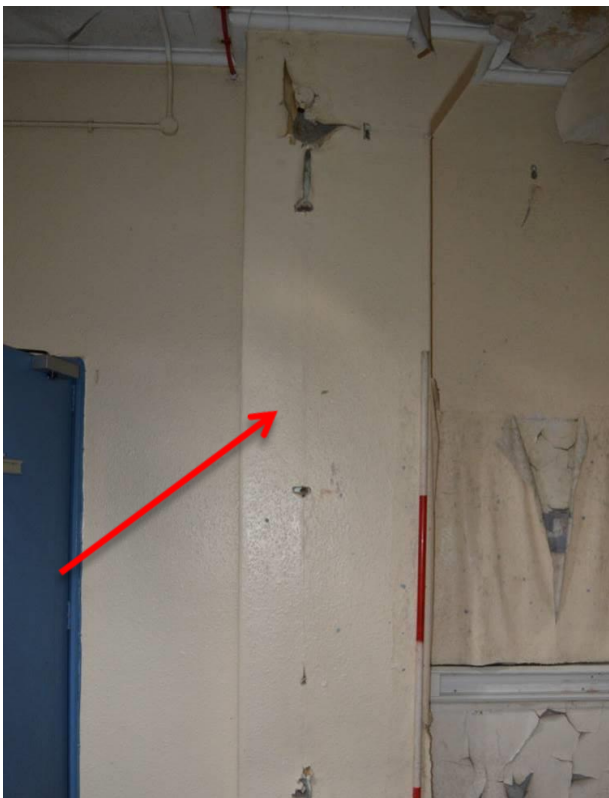
Plate 57.3: Flue from assistant surgeon's sitting room fireplace. Scale 2m. Facing north west.
