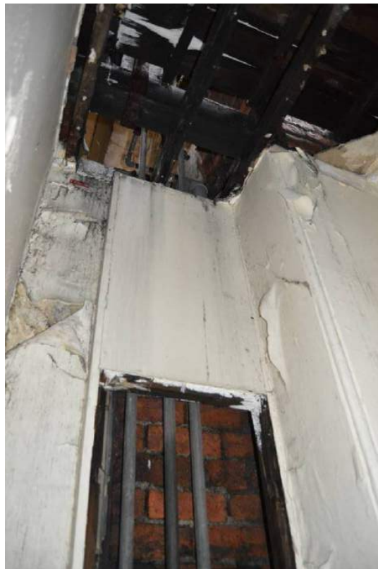
Plate 42.1: View of remaining plaster finish.
