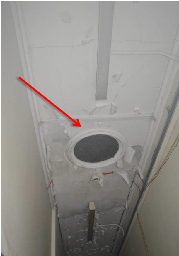
Plate 46: View of nurses' corridor ceiling vent. Facing north east.
