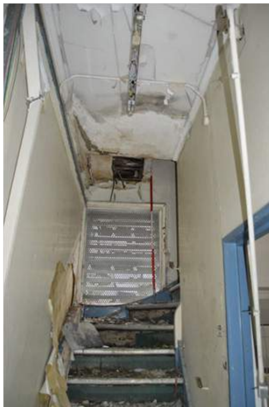
Plate 52.2: Stairs to the west of the nurses' accommodation. Scale 2m.
