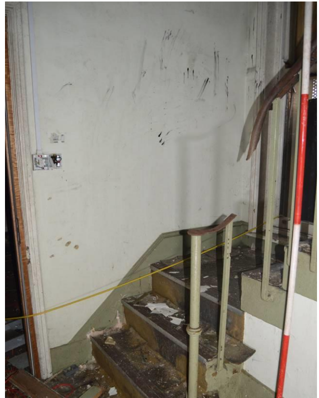
Plate 101.4: Shaw nurses' home side stairs (facing north west). Scale 2m.
