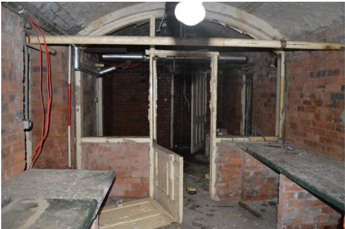
Plate 71: Original wine cellar features in situ. Scale 2m.
