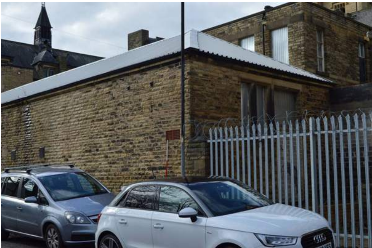
Plate 99.1: South east corner of the laundry building. Scale 2m.
