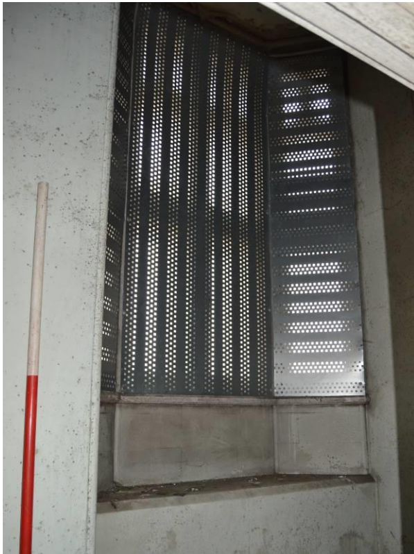
Plate 38.1: Recess for the bay window. Scale 2m. Facing north.
