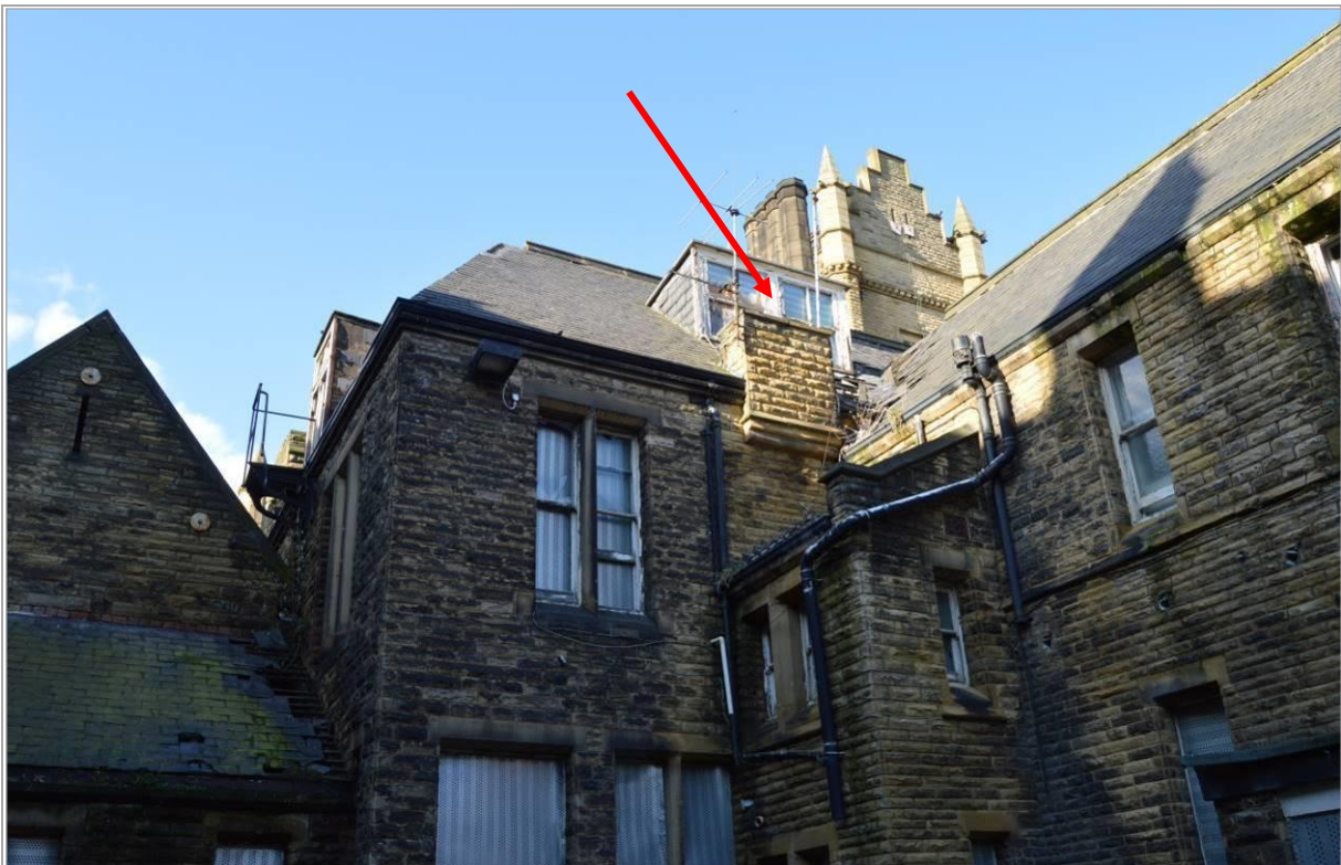
Plate 17: Rear view of the administration range looking north west. Note again a truncated and capped chimney flue along the line of the eaves. Facing north.
