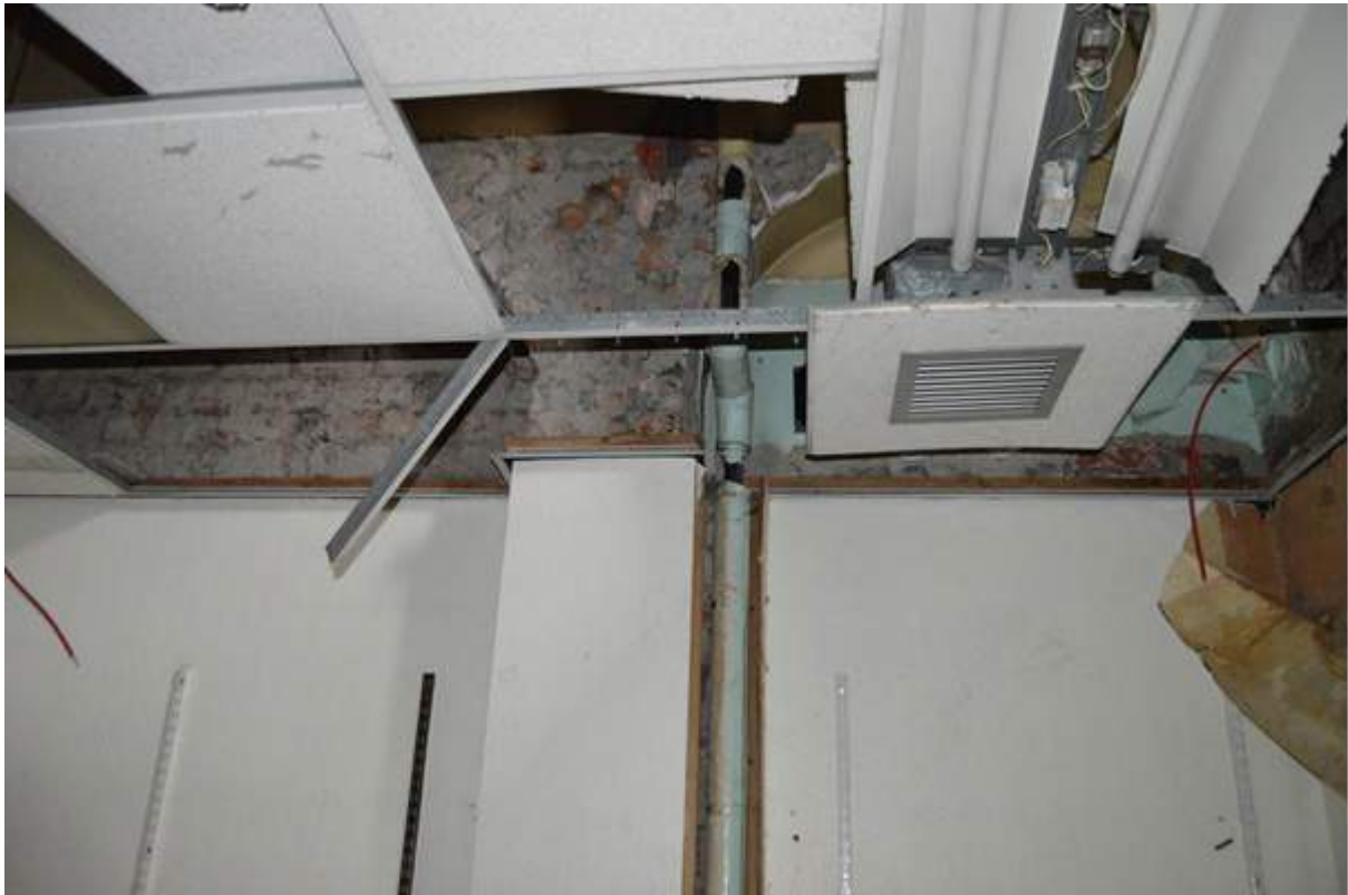
Plate 91.5: Relieving arches, with some early plaster and paint schemes, from the original dispensary areas.
