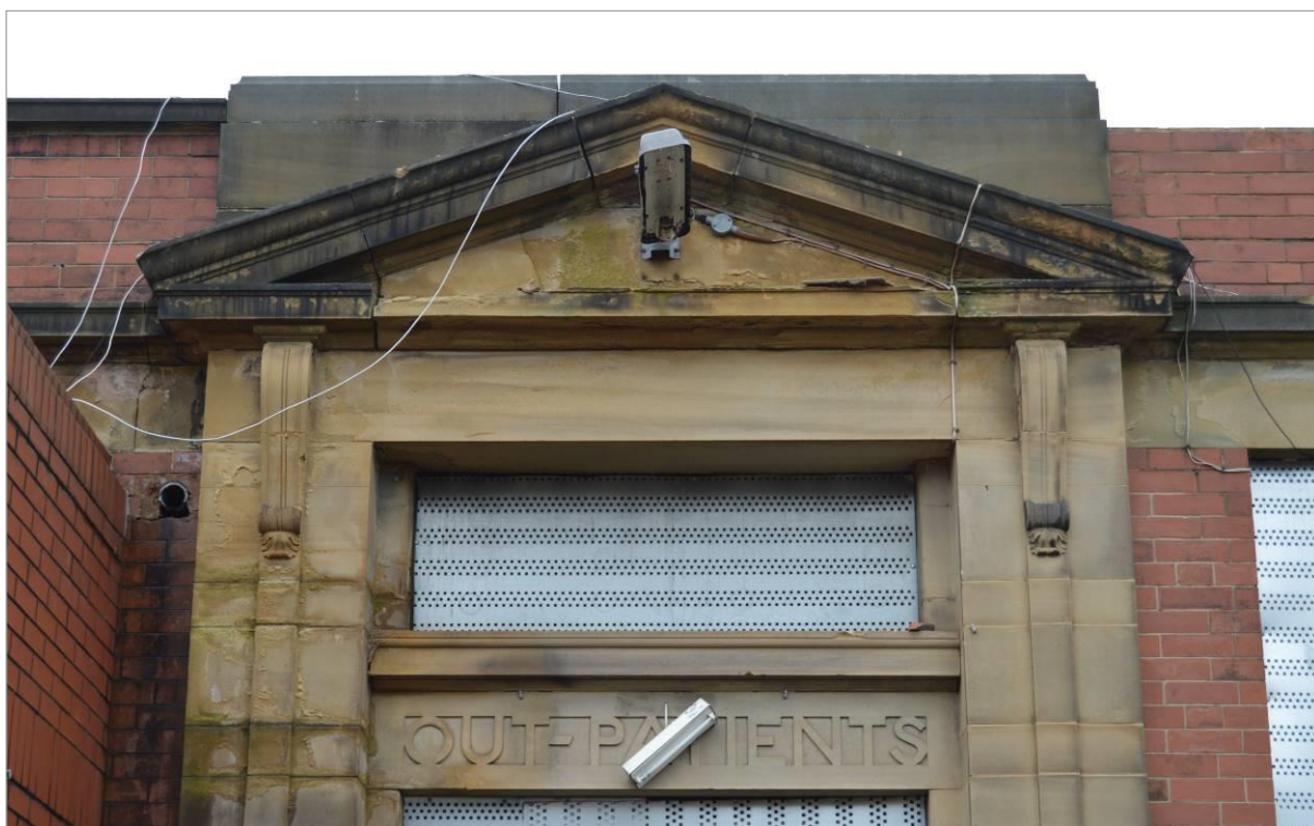
Plate 102.2: South entrance to Out-patients Department, facing north west.
