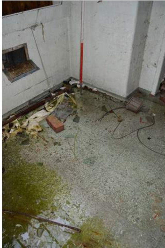
Plate 105.6: Terrazzo floor of the operating theatres. Scale 2m.
