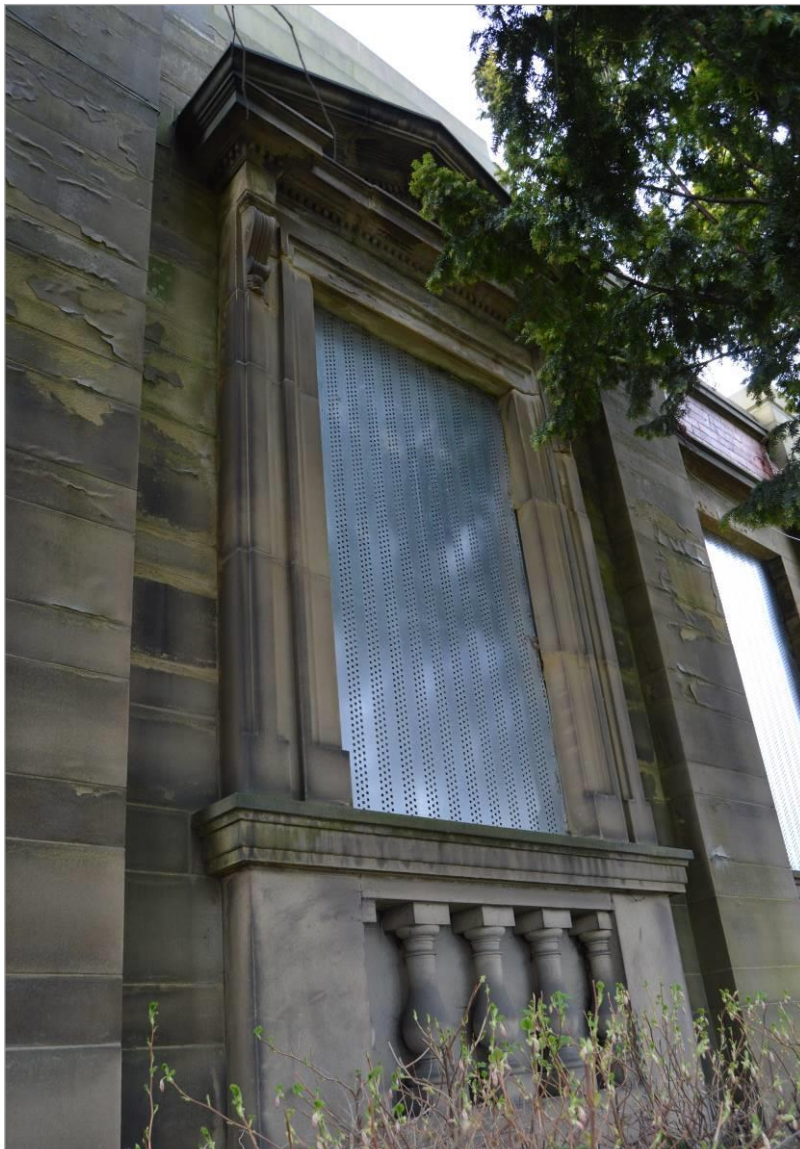
Plate 104: Stone façade pediment window surround to X-Ray wing, facing west.
