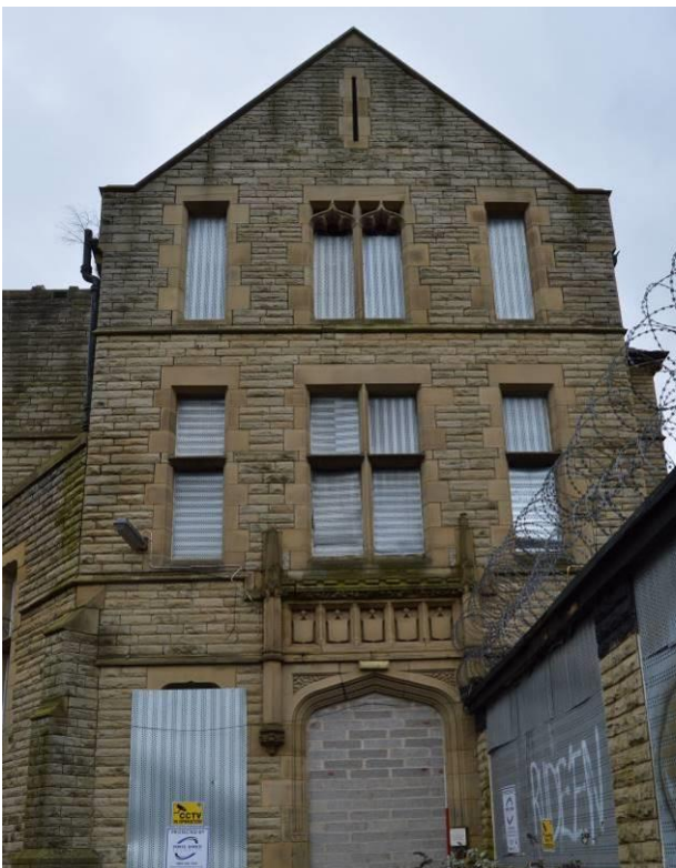
Plate 100.1: View of nurses' Home north facing elevation (facing south east).
