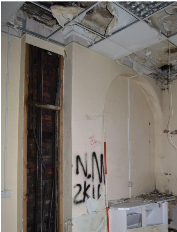
Plate 28.3: Alcove to room G6 with cornice above. Scale 2m. Facing west.
