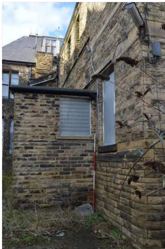
Plate 72.4: Flat roofed single storey extension to east of service wing. Scale 2m.
