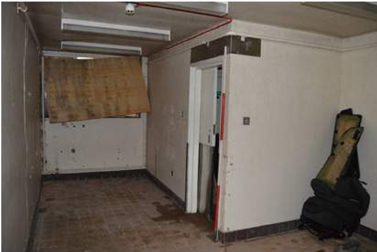
Plate 80.6: Reverse view in room G12.8. Scale 2m.
