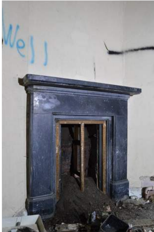
Plate 28.1: Corner fireplace to room G6.
