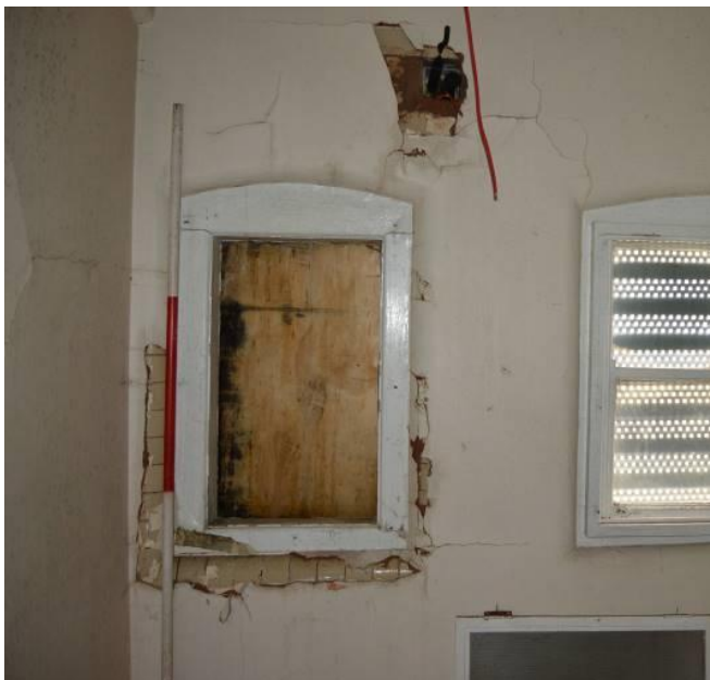
Plate 79.1: Detail of windows to G11.6. Scale 2m. Facing north east.
