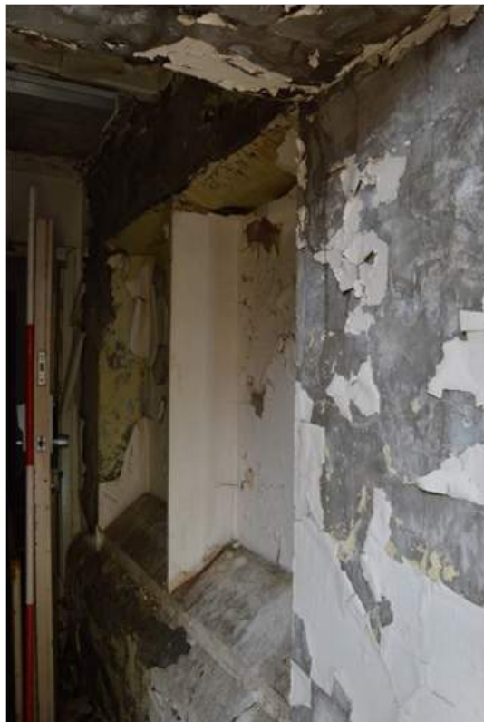
Plate 91.21: Blocked windows of the original building exterior wall.
