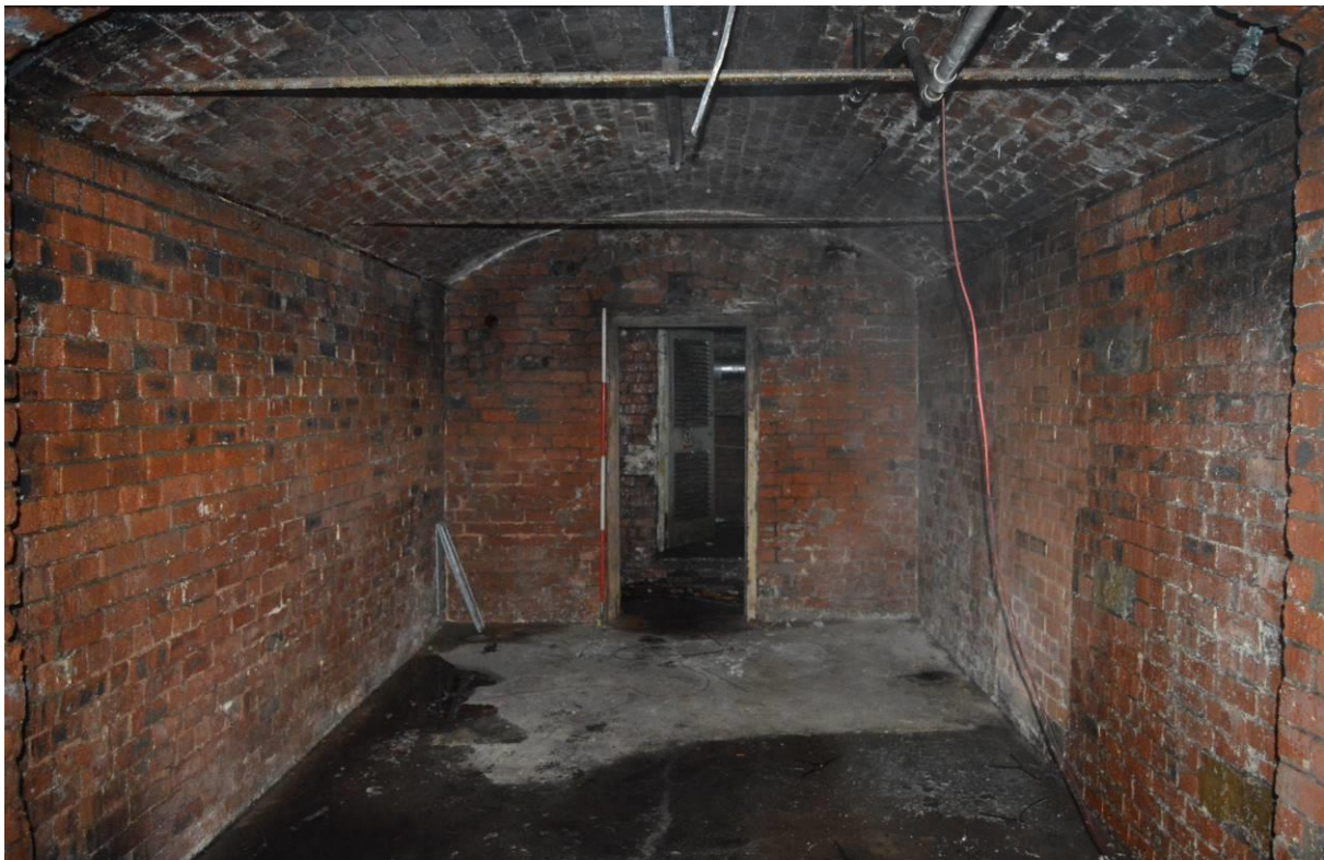
Plate 70.4: Cellar room. Scale 2m. facing north west.
