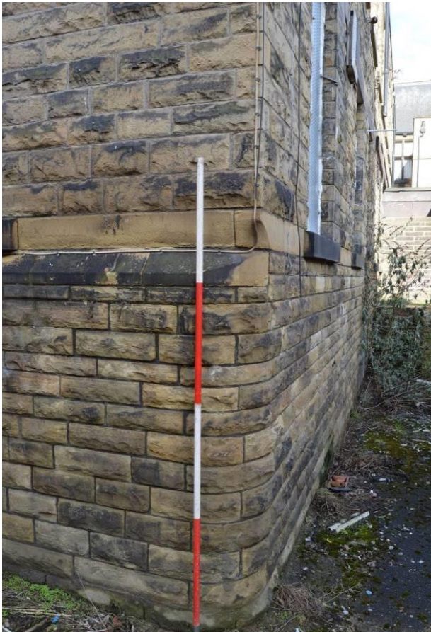
Plate 72.3: Filleted corner to south east corner of service wing extension. Scale 2m. Facing north east.
