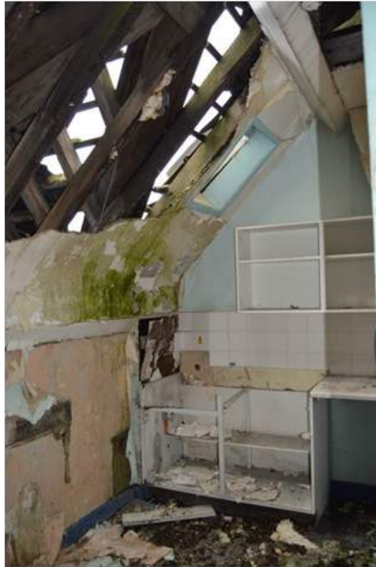
Plate 67.5: Room S5, with sloping ceiling with skylight.
