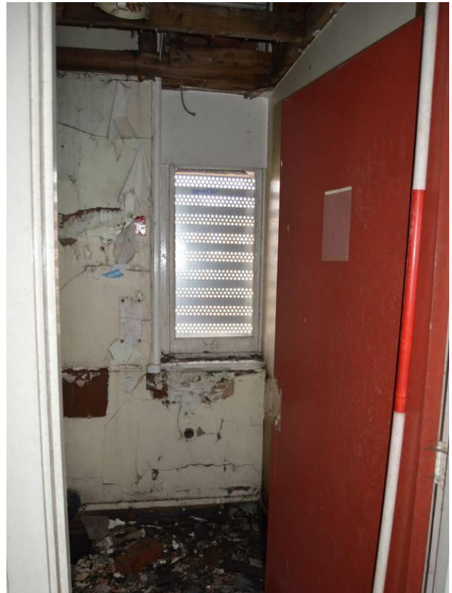
Plate 41: View into the rearranged surgeons' bathroom. Scale 2m. Facing north west.
