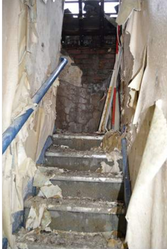
Plate 56.2: Half-landing/dog-leg of the stairs to the second floor. Scale 2m.
