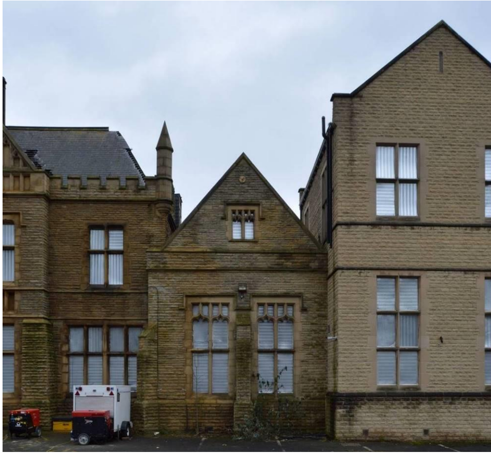
Plate 83: Exterior of linking range incorporating the board room, facing south east.
