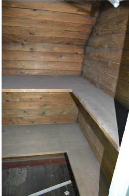
Plate 67.7: Tongue and groove cladding and shelving in airing cupboard.
