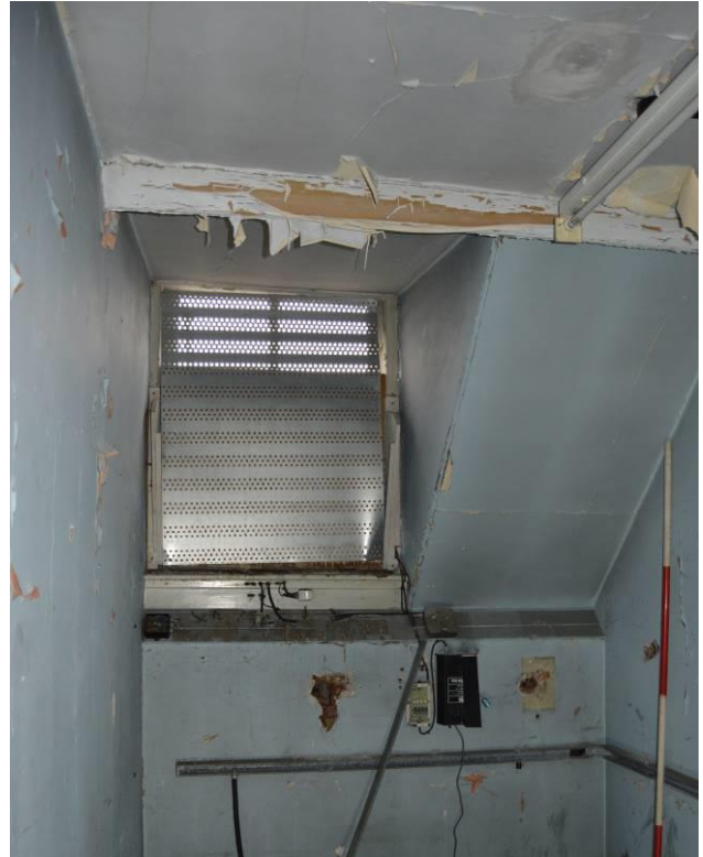
Plate 68.11: Dormer window to room S12. Scale 2m. Facing south east.
