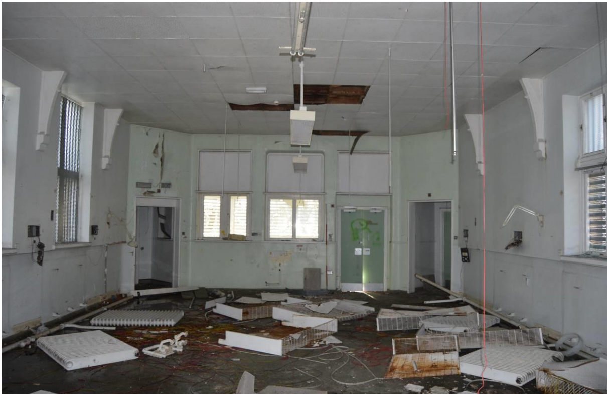
Plate 92.6: Western pavilion ward first floor facing south. Scale 2m.
