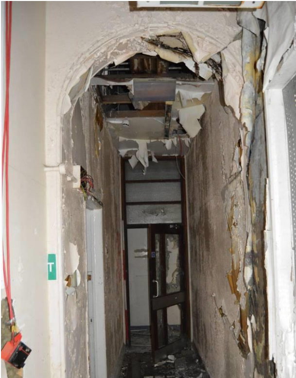
Plate 59.1: View facing north of the lobby. Scale 2m. Facing north west.
