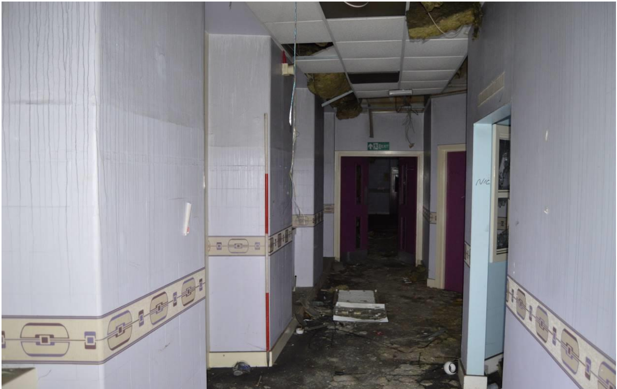
Plate 105.10: The Ann Canning Childs' Building in the part which was originally an open ward. Note the thick embrasures in the right belonging to the original window openings (facing SW). Scale 2m.
