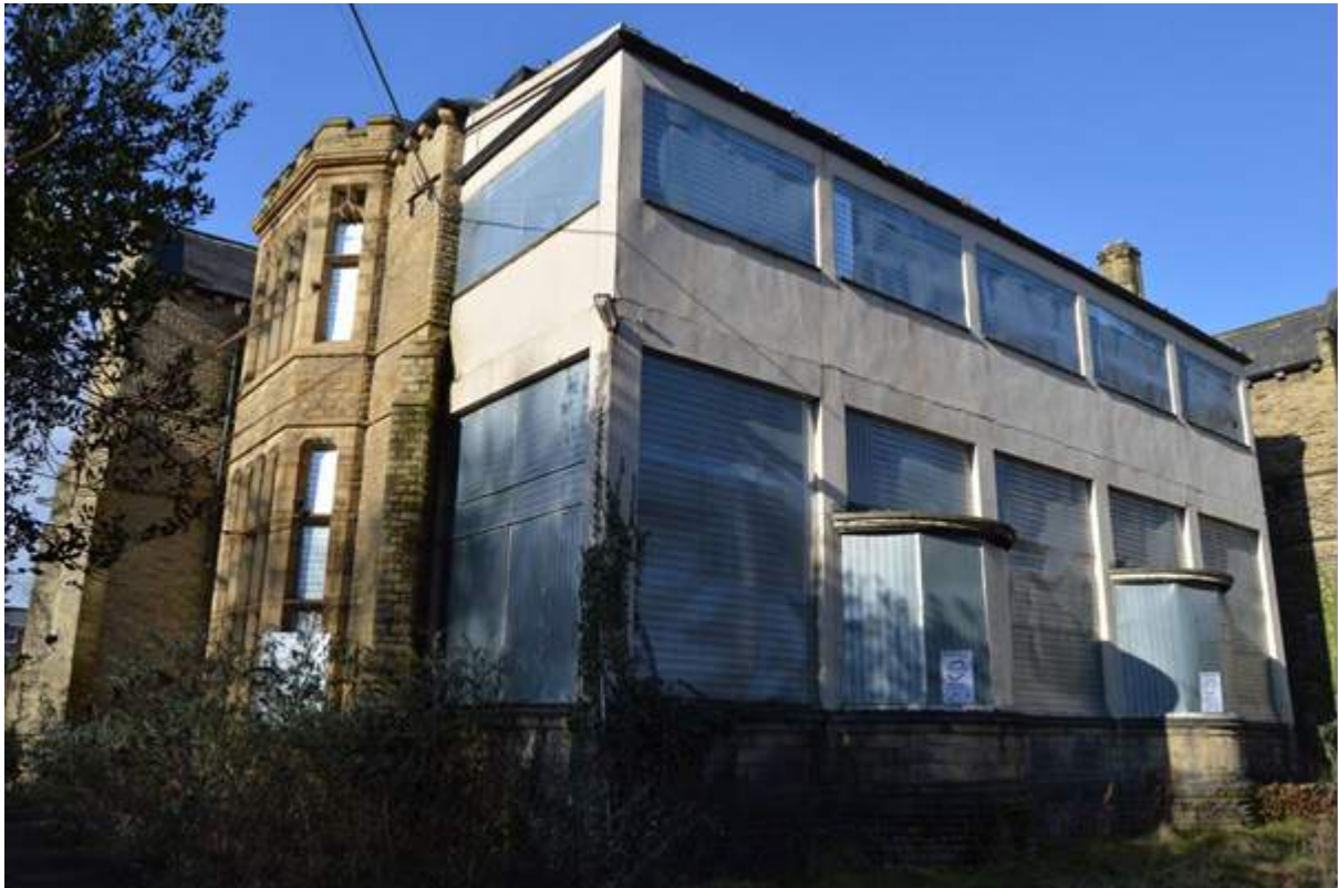
Plate 98: Veranda extension to children's ward. Scale 2m.
