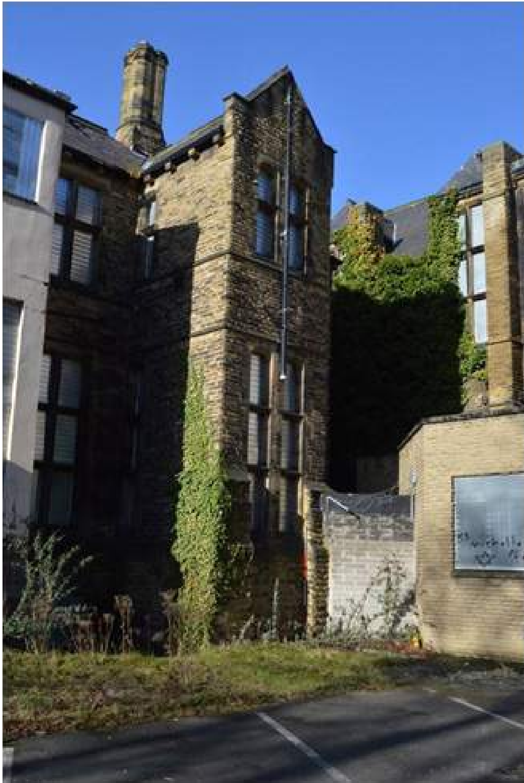
Plate 95: North facing elevation of the special ward. Scale 2m.
