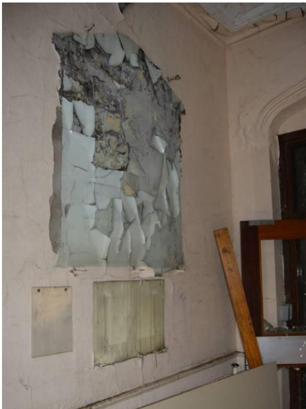
Plate 19.1: Visitor's hall dedication plaque location. Facing east.
