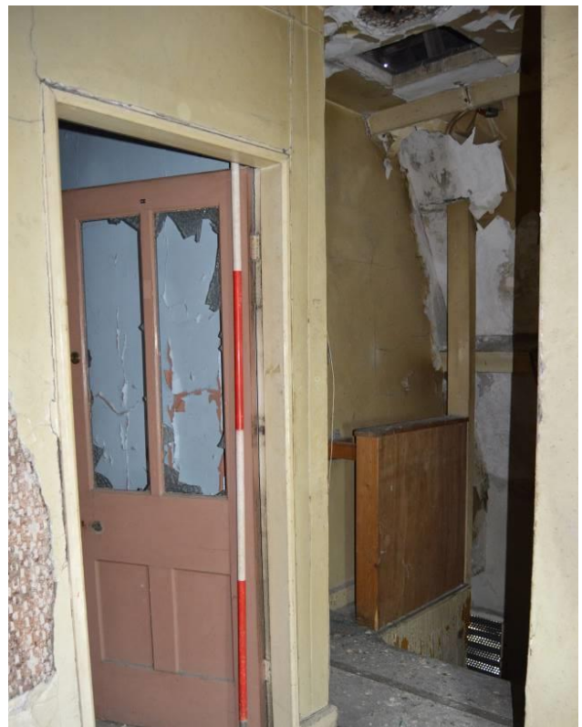
Plate 68.9: Half-glazed door to room S12. Scale 2m. Facing south.
