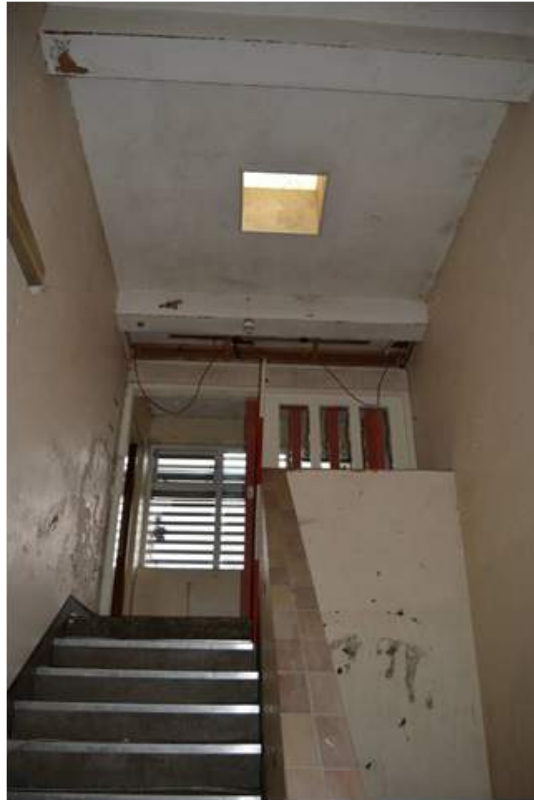
Plate 109.1: Landing in the modern extension to the Canning wards. Scale 2m.
