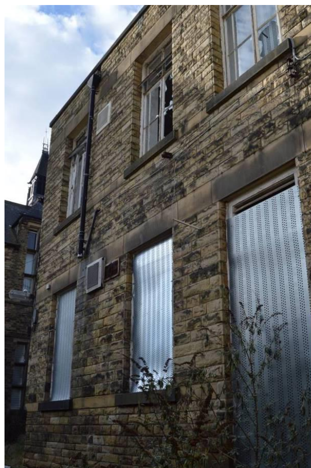
Plate 72.2: South elevation of the service wing extension, looking north east.
