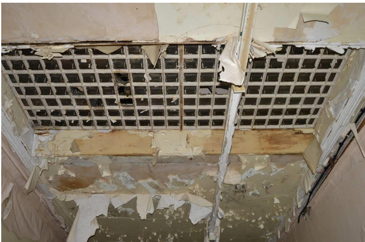
Plate 24: Glass tiled ceiling/floor above the axial corridor. Facing north east.
