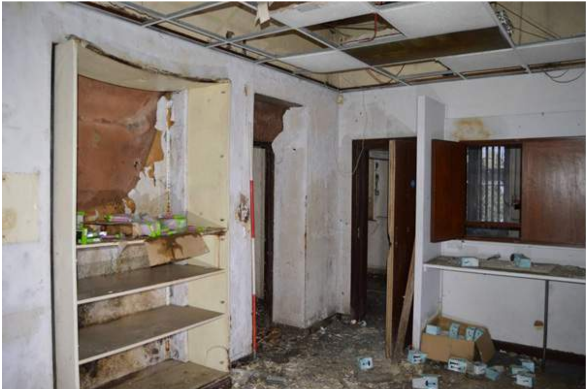
Plate 33.2: Reverse view in room G8. Scale 2m.
