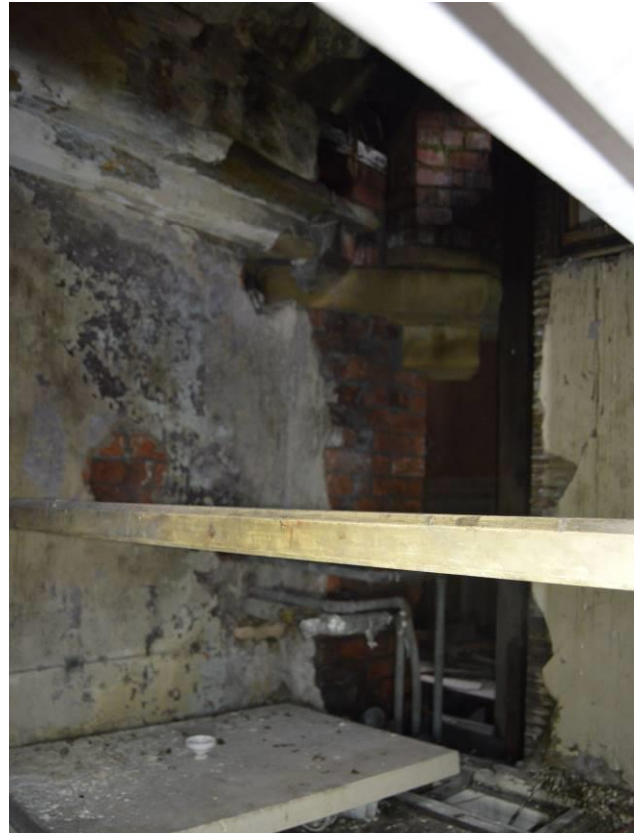
Plate 61.6: Chamfered timber handrail. Facing north.
