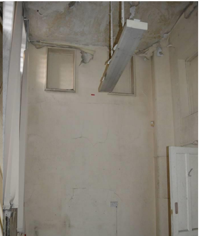
Plate 91.14: Blocked windows in converted W.C. room (facing south west).
