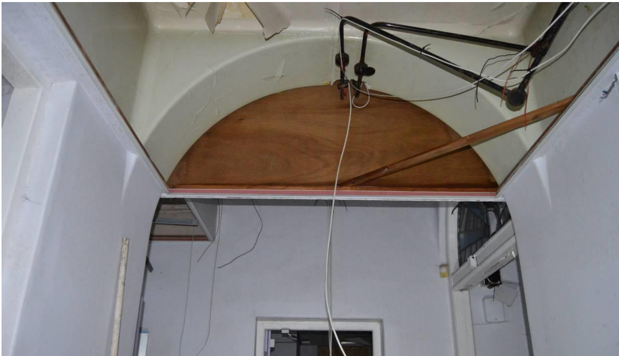
Plate 104.4: Archway at corridor junction in X-Ray wing, facing north west.
