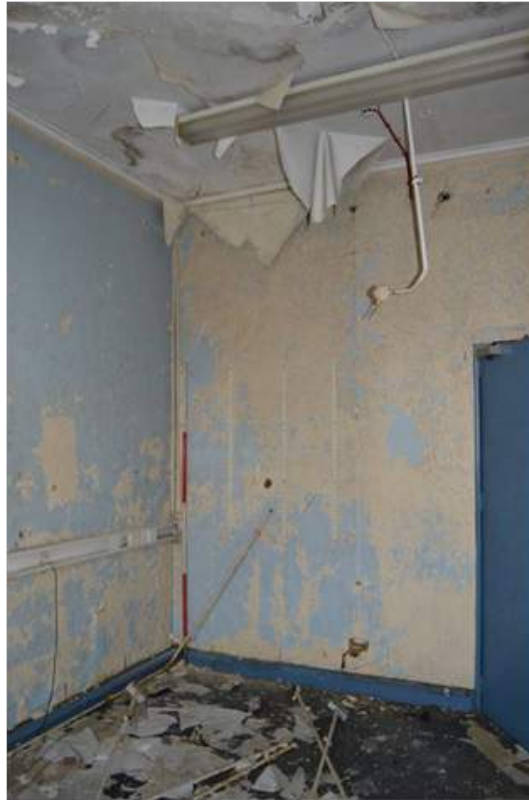
Plate 48.4: View of room F7 with coving in situ. Scale 2m.
