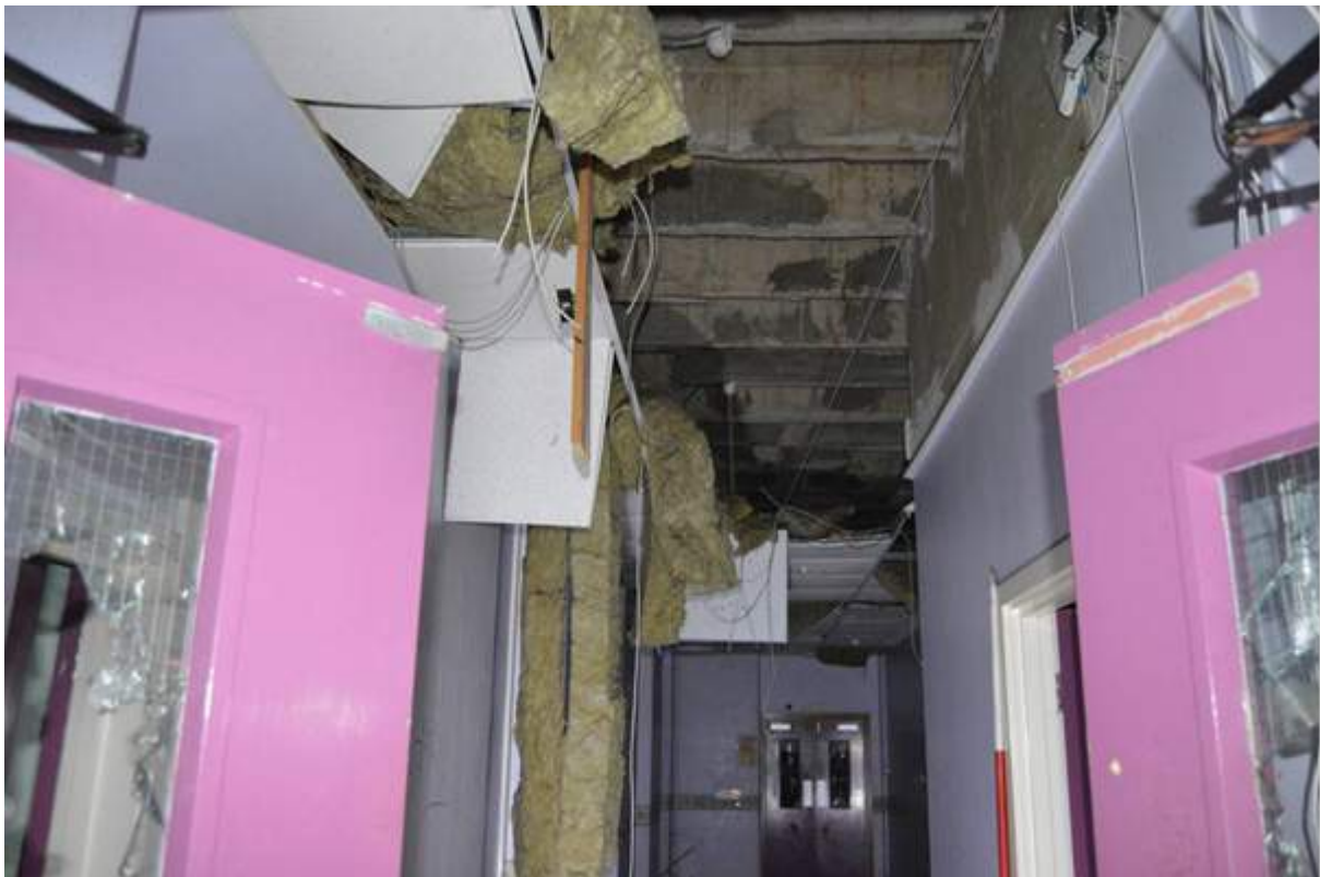
Plate 105.11: The Ann Canning Childs' ward was constructed of cast re-enforced concrete and steel framing.
