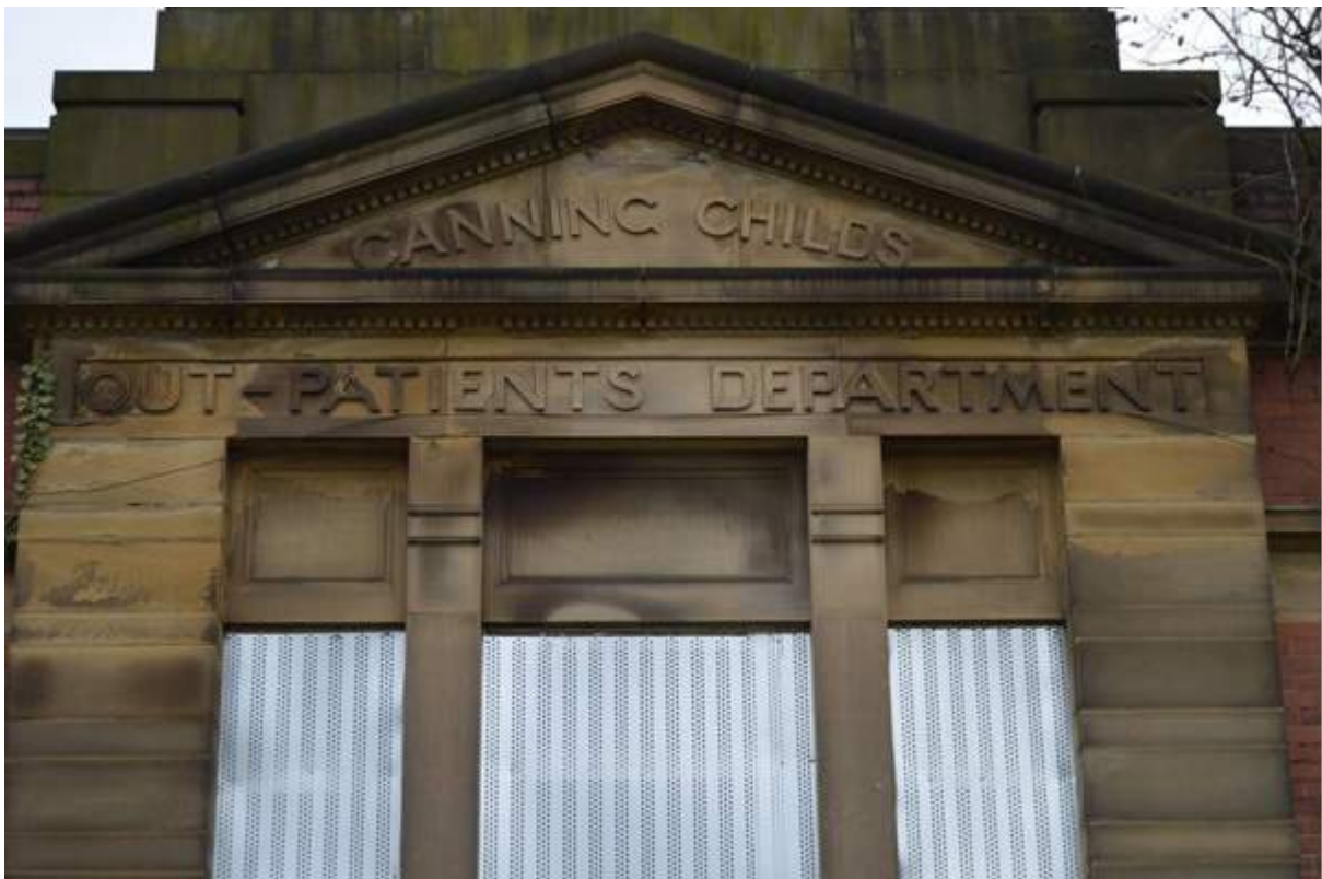
Figure 102.1: Canning Childs Out-patients' pediment over façade.
