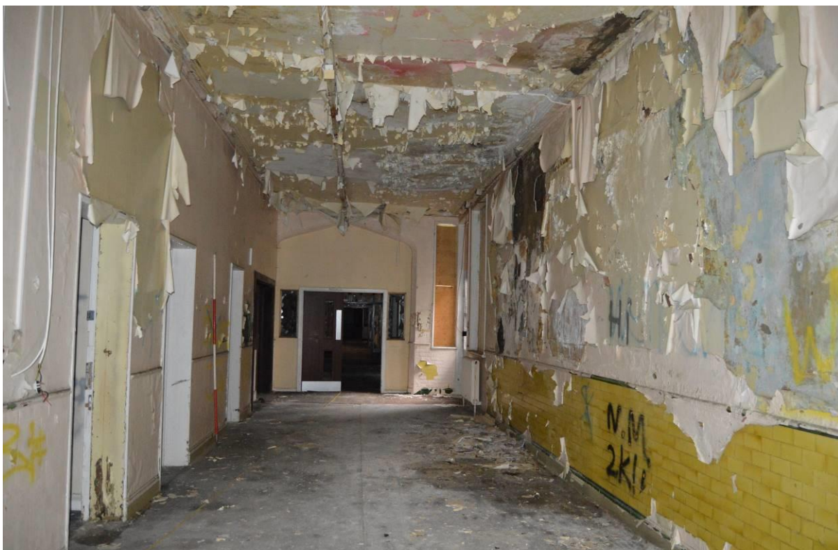
Plate 23: View of the administration range corridor. Scale 2m. Facing north east.
