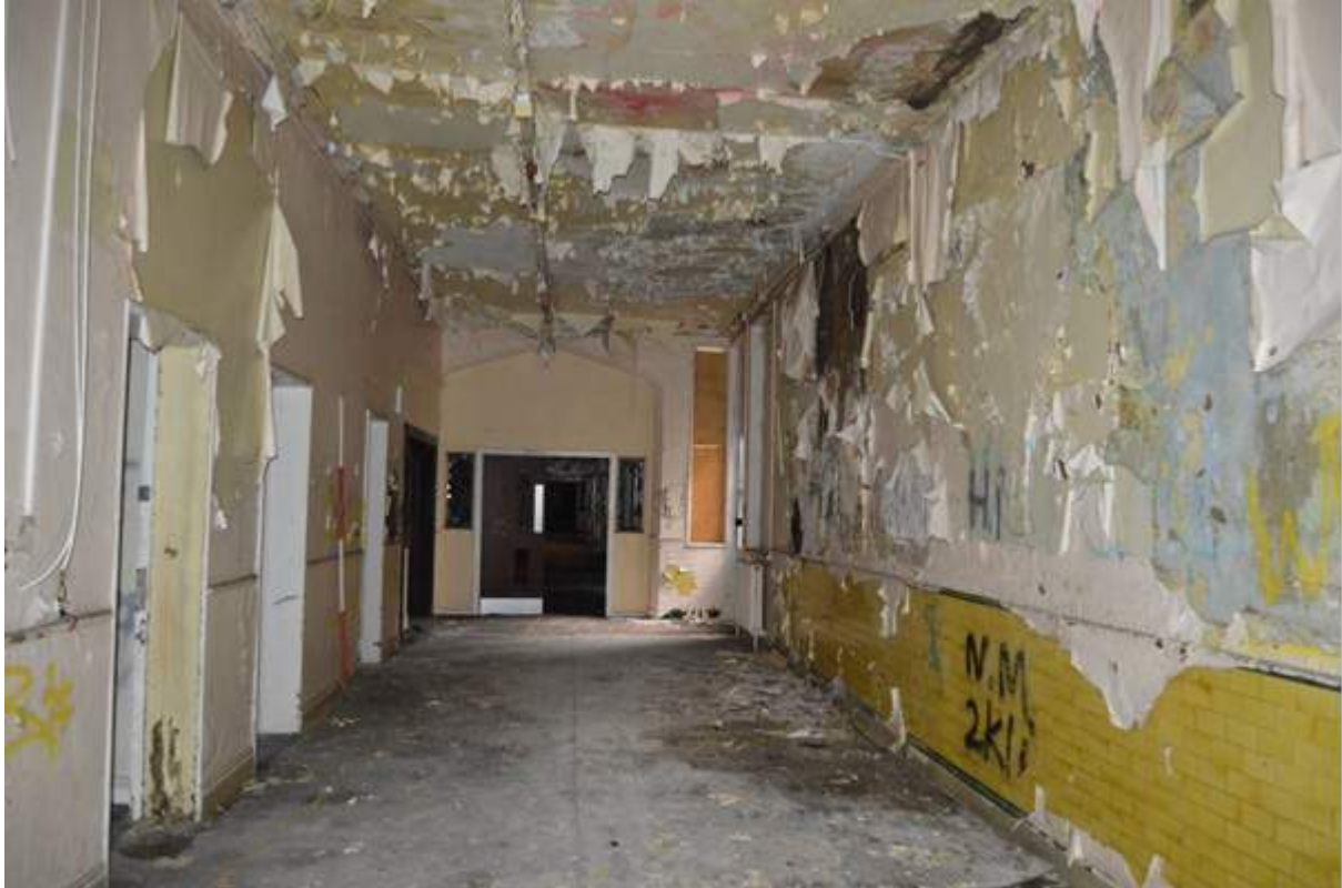
Plate 23: Oblique view of the administration range. Scale 2m.
