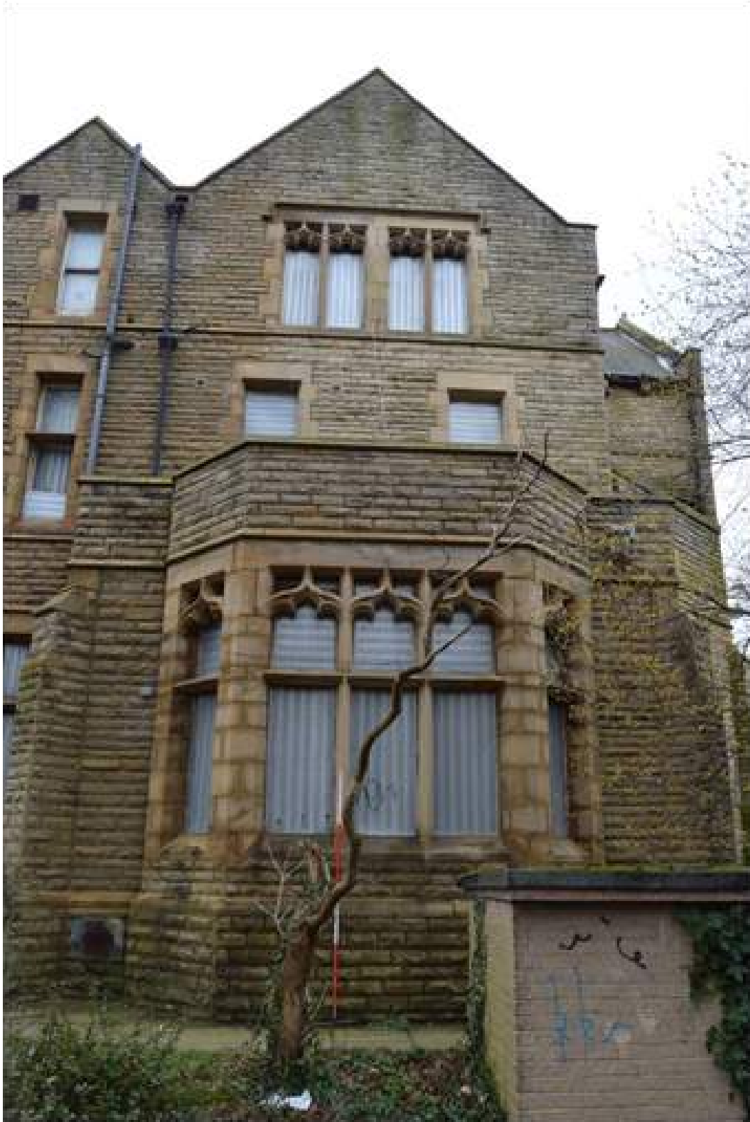
Plate 100.3: View of east elevation section.
