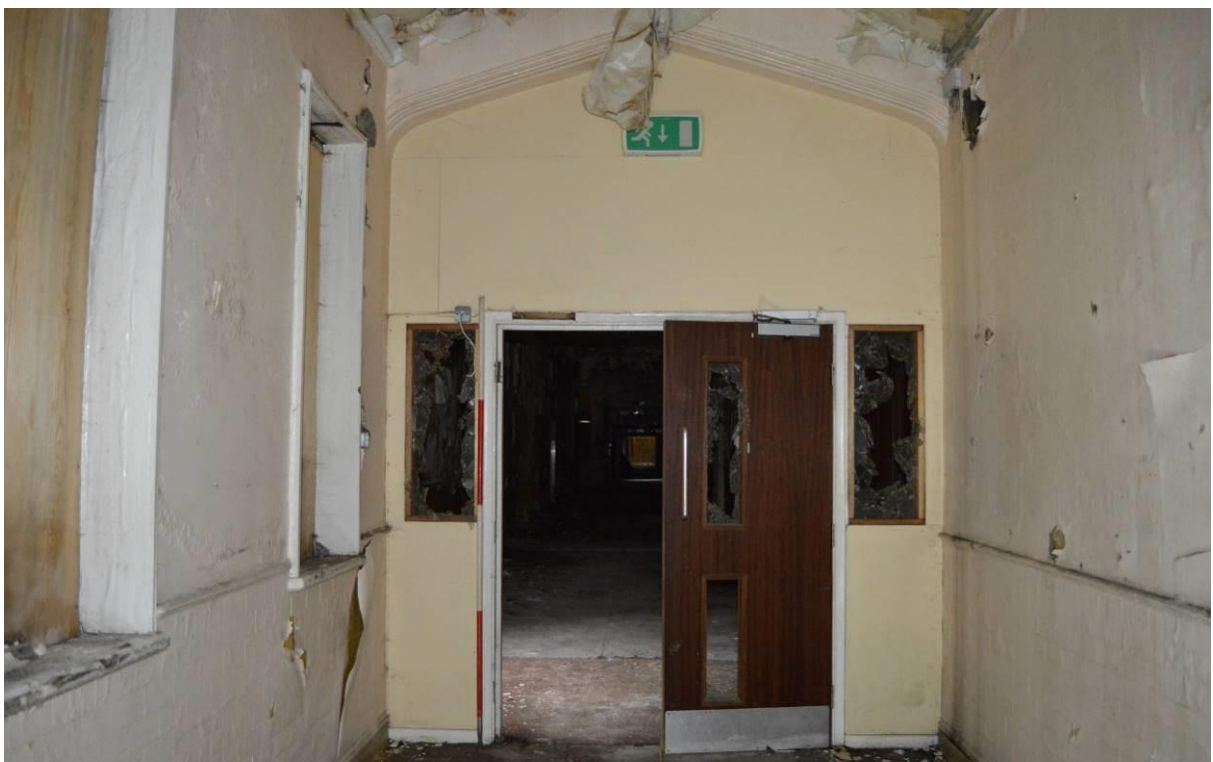
Plate 88.2: Blocked in Tudor style arch, view facing west in axial corridor. Scale 2m.
