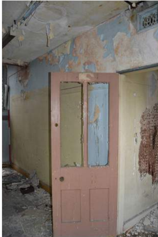
Plate 69.1: Half-glazed door to room S13. Scale 2m.
