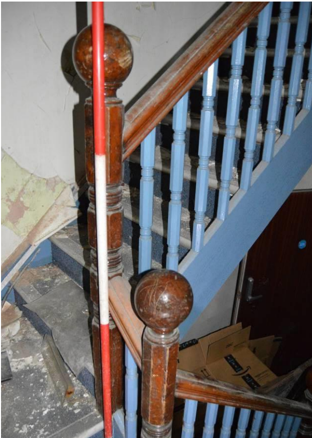
Plate 22.2: Newels and spindles to stairs in room G3. Scale 2m. Facing north.
