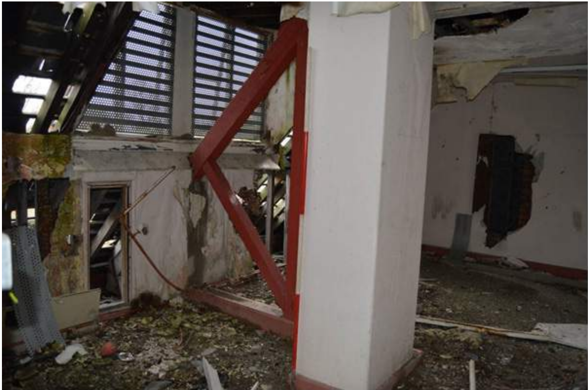
Plate 66: View facing south east in room S3. Scale 2m.
