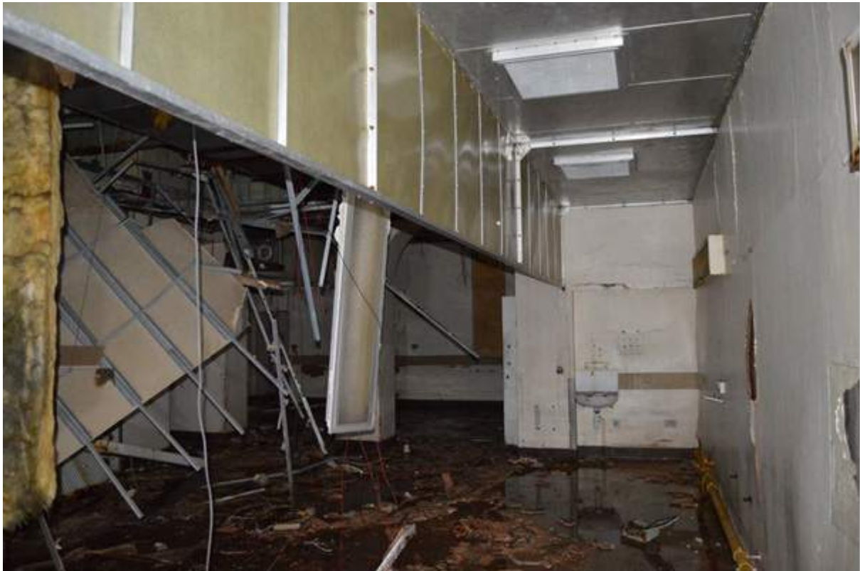
Plate 77: View of the modernised kitchen area.
