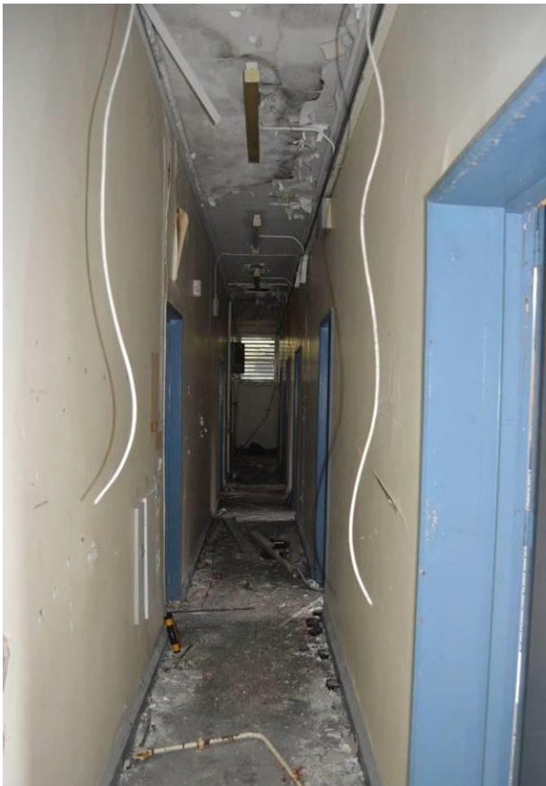
Plate 44: View along nurses' corridor. Facing north east.
