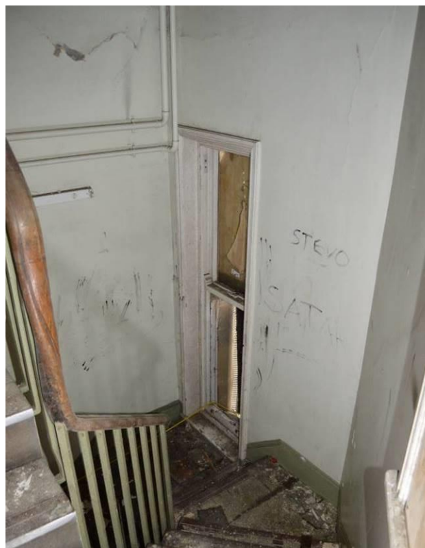
Plate 101.6: View down the stairs to half-landing, facing north.
