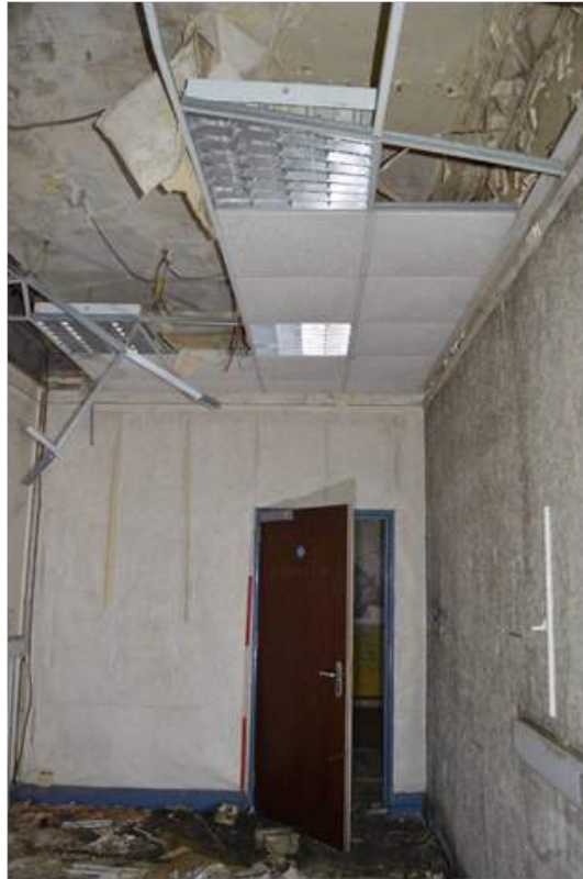
Plate 29.2: Modern door and suspended ceiling but with features above. Scale 2m.
