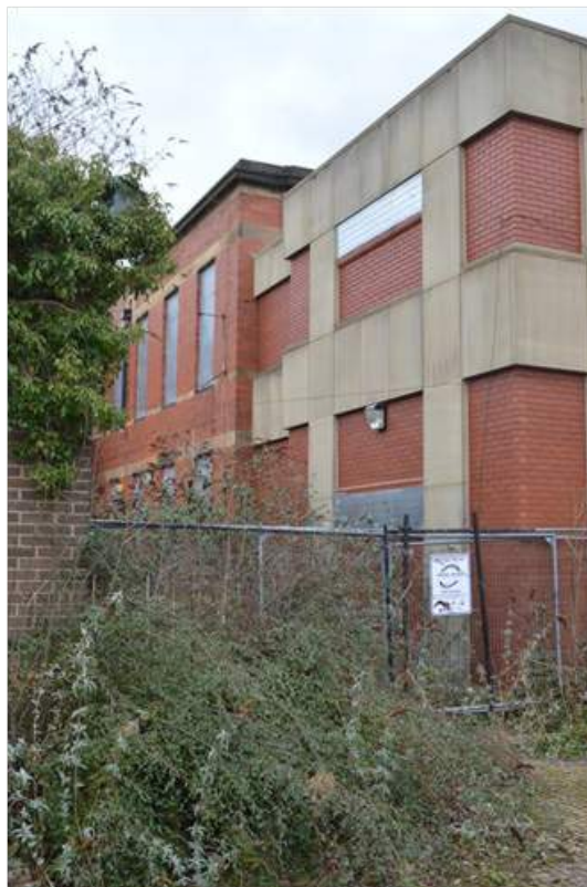
Plate 108.4: North elevation of the modern extension to the Canning wards.
