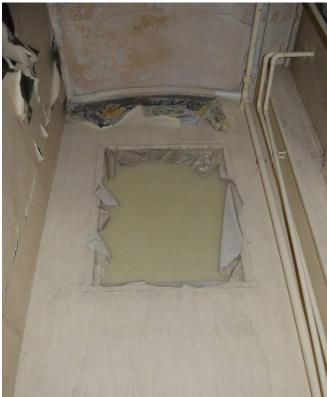
Plate 91.13: Interior window to lobby of west sanitary wing (facing south).
