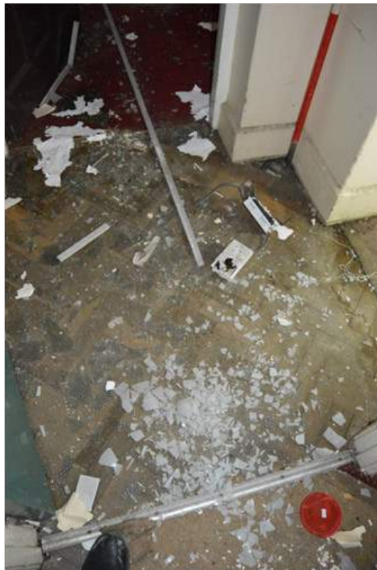
Plate 91.10: Parquet flooring to sanitary wing lobby . Scale 2m.
