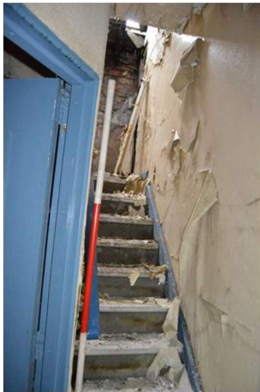
Plate 56.1: View facing up the stairs in room F13. Scale 2m.
