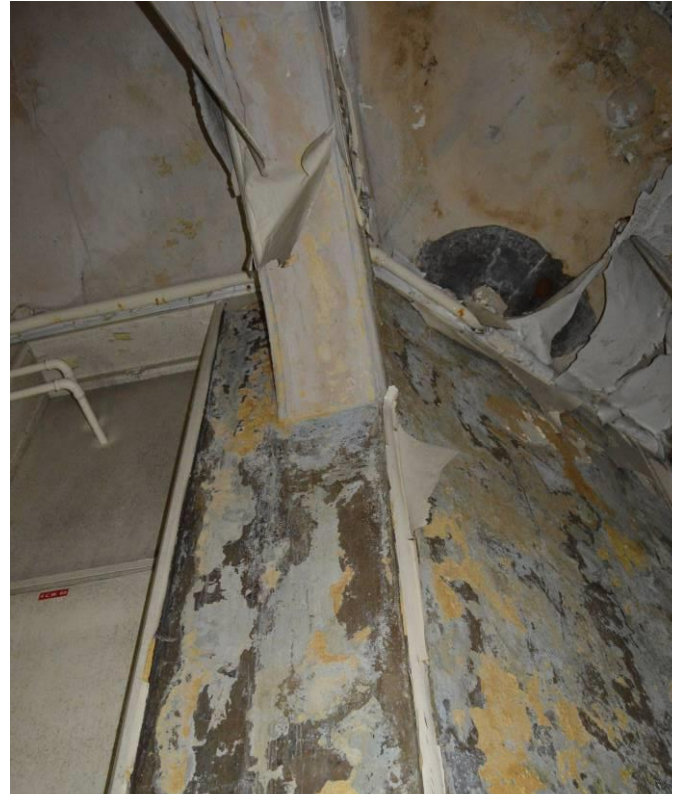
Plate 91.12: Original plaster finishes to west sanitary wing area (facing south west).
