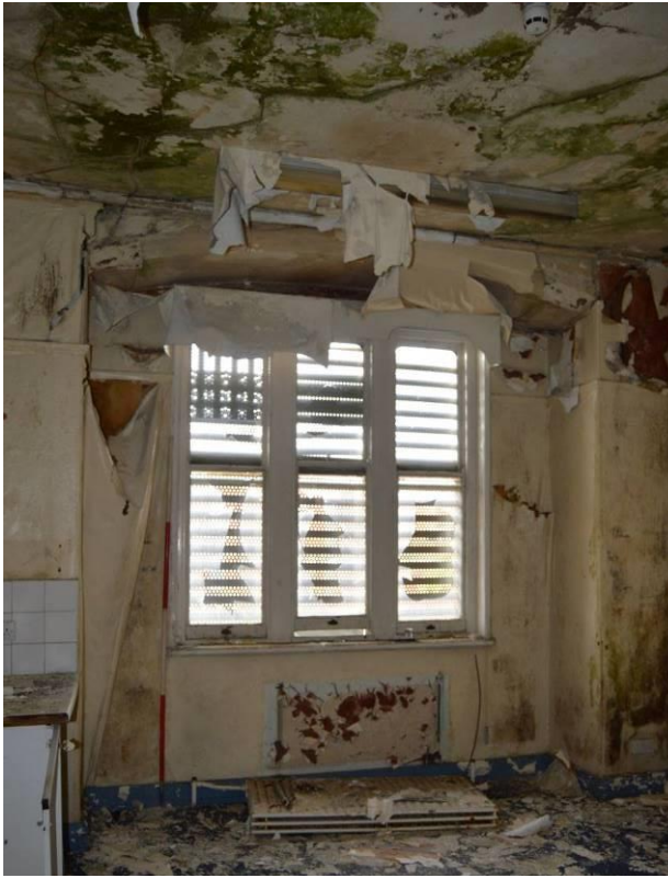
Plate 43.1: Window in room F6. Scale 2m. Facing north west.
