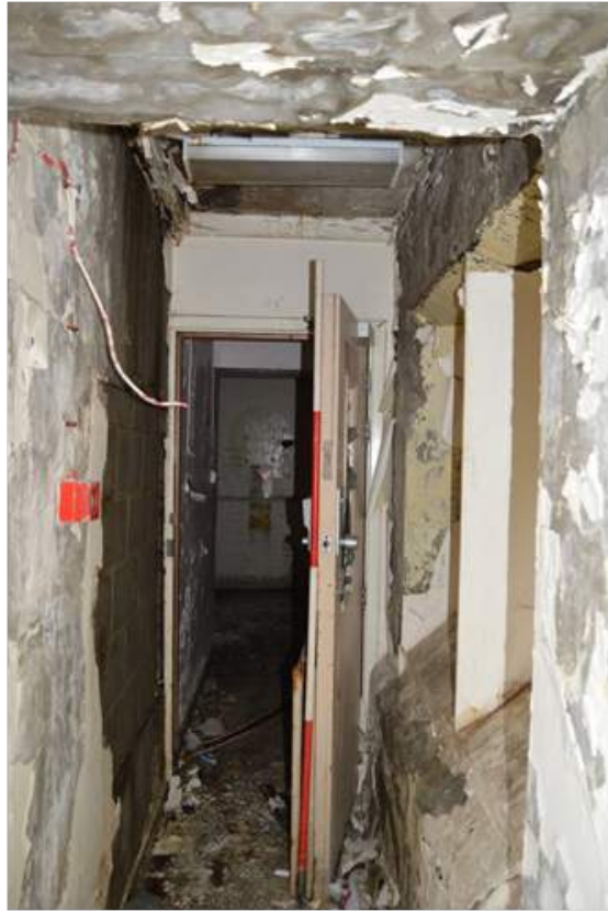
Plate 91.20: Modern corridor returning to the main axial route window. Scale 2m.
