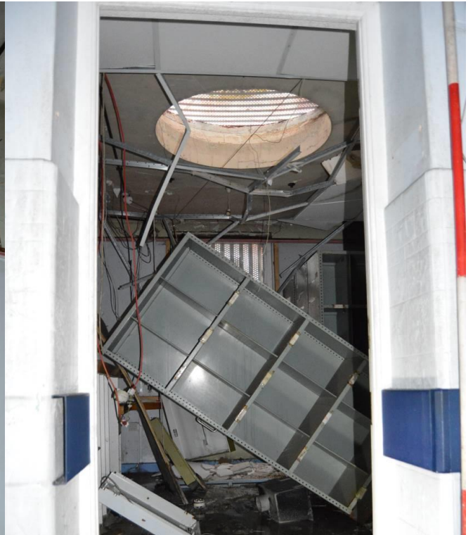
Plate 104.8: Circular skylight to X-ray annex rooms (facing south east).
