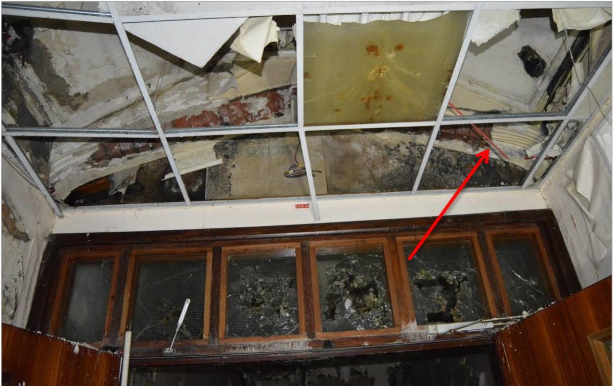
Plate 85.1: Tudor style arch above axial corridor later features (facing south west).
