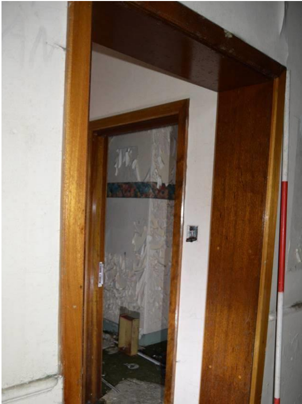
Plate 26: Modern doorway into matron's room G4. Scale 2m. Facing north.
