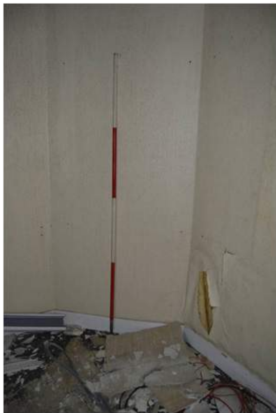
Plate 20.1: Corner chimney breast in visitor waiting room G2. Scale 2m.
