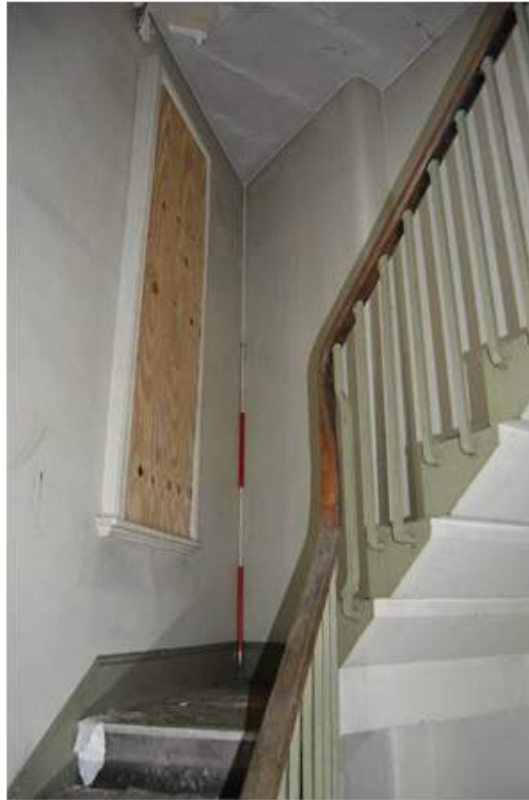
Plate 101.5: Detail of stair banister. Scale 2m.
