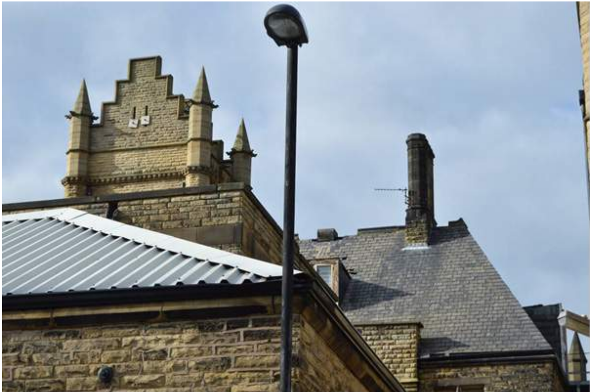
Plate 12: Rear gable of tower, note the plainer style.
