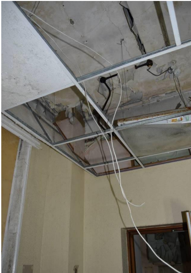
Plate 20.2: View of original plasterwork to room G2. Facing north.
