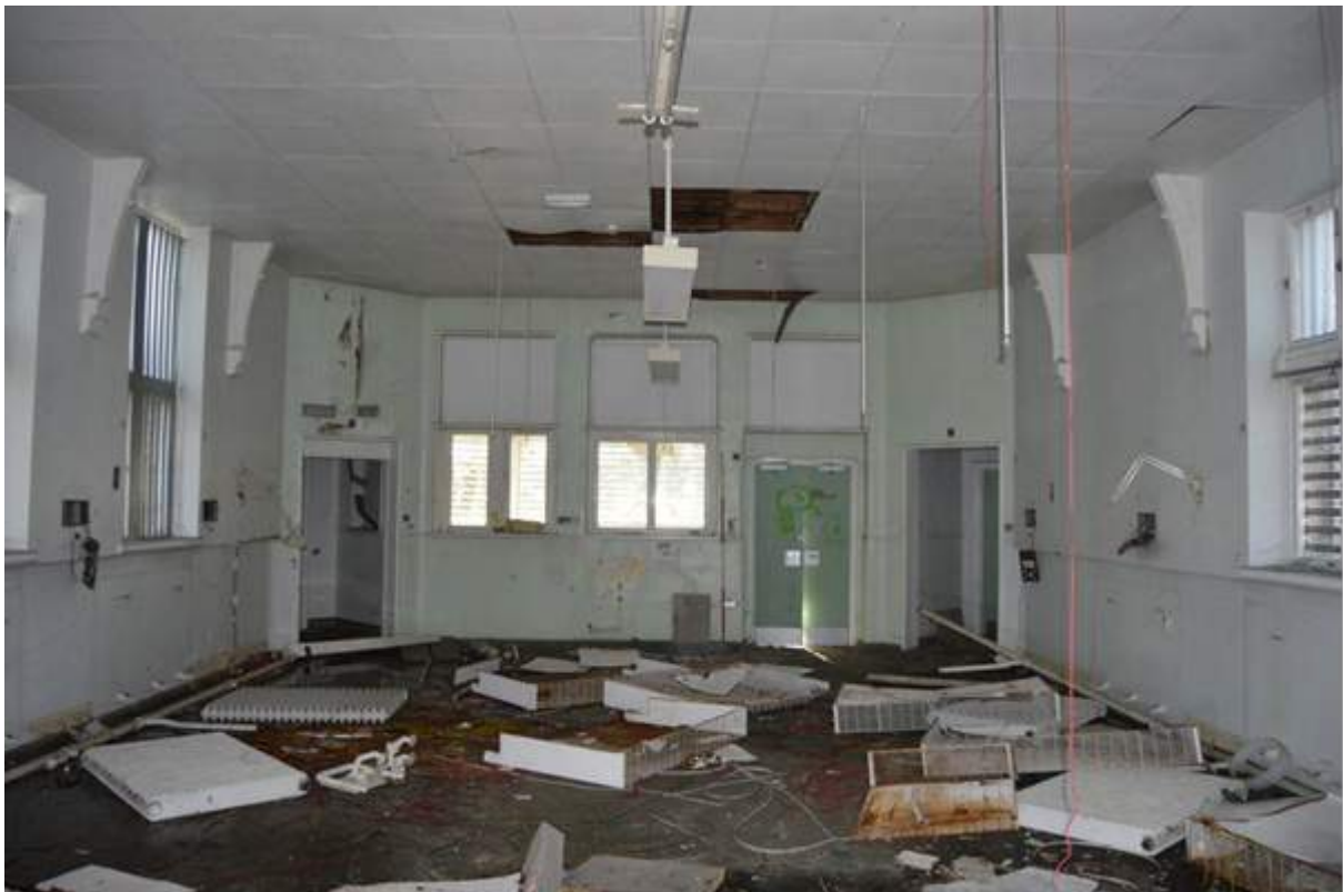
Plate 92.6: Western pavilion ward first floor facing south. Scale 2m.
