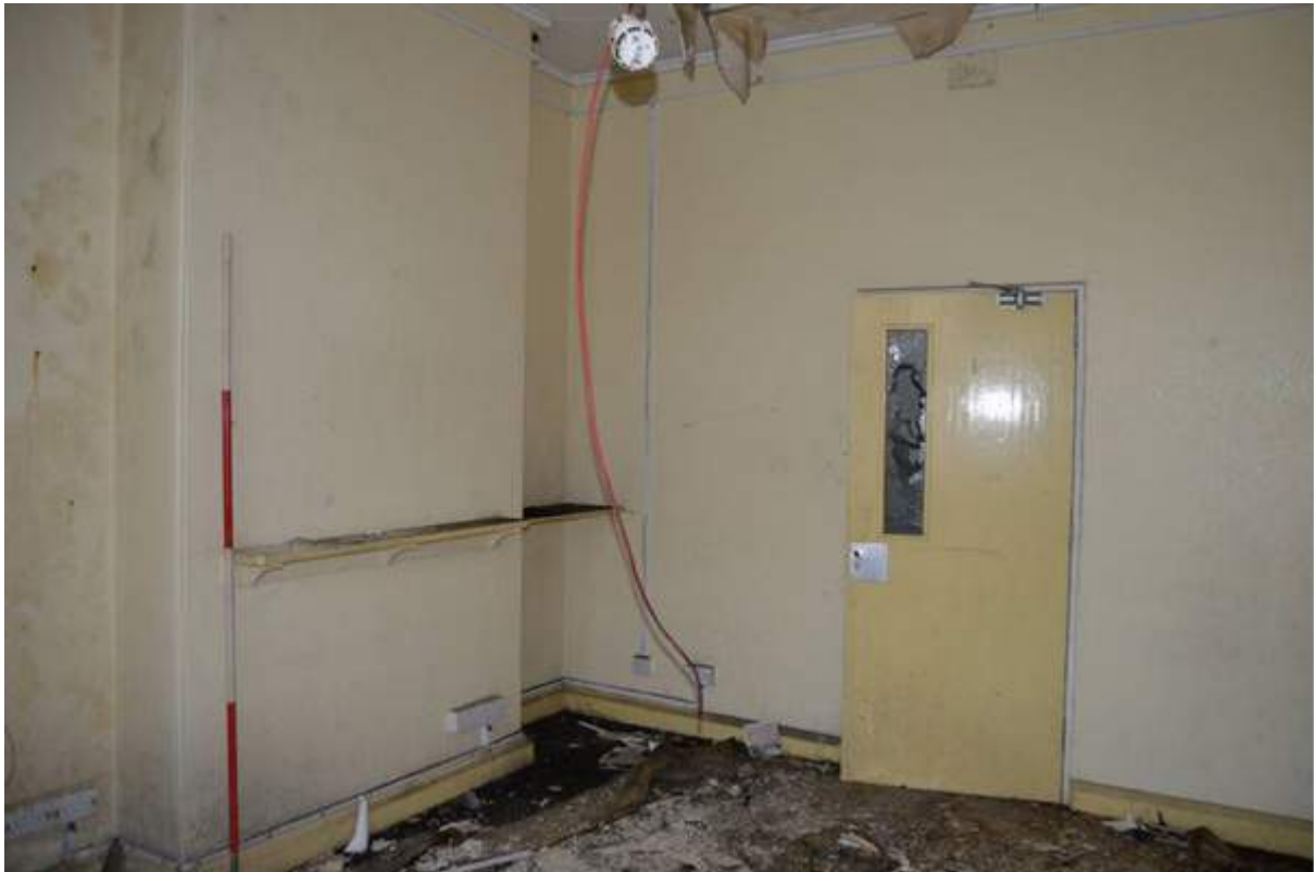
Plate 49.2: Chimney with mantle shelf in matron's bedroom. Scale 2m.
