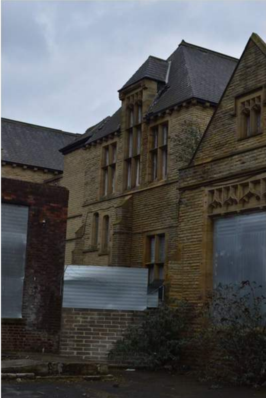
Plate 90: View of the north elevation of the eastern pavilion wing.
