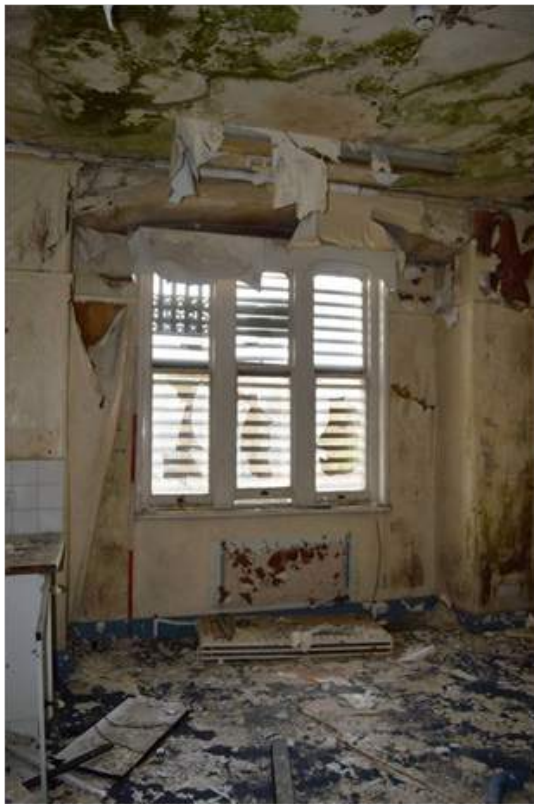
Plate 43.1: Window in room F6. Scale 2m.
