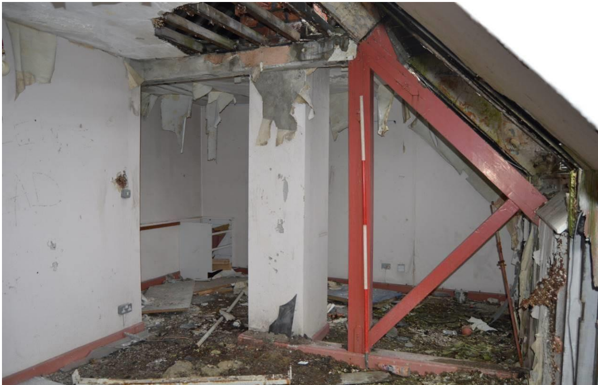
Plate 65.2: Repaired timber truss to room S3. Scale 2m. Facing north east.
