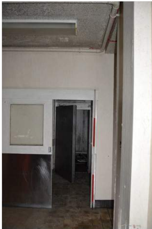
Plate 80.4: View towards cold store in room G12.2. Scale 2m.
