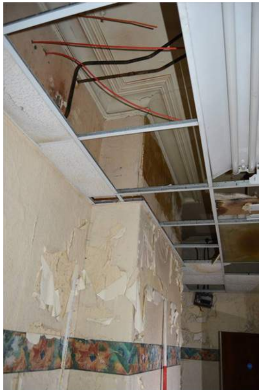
Plate 27.2: Chimney breast and coving.
