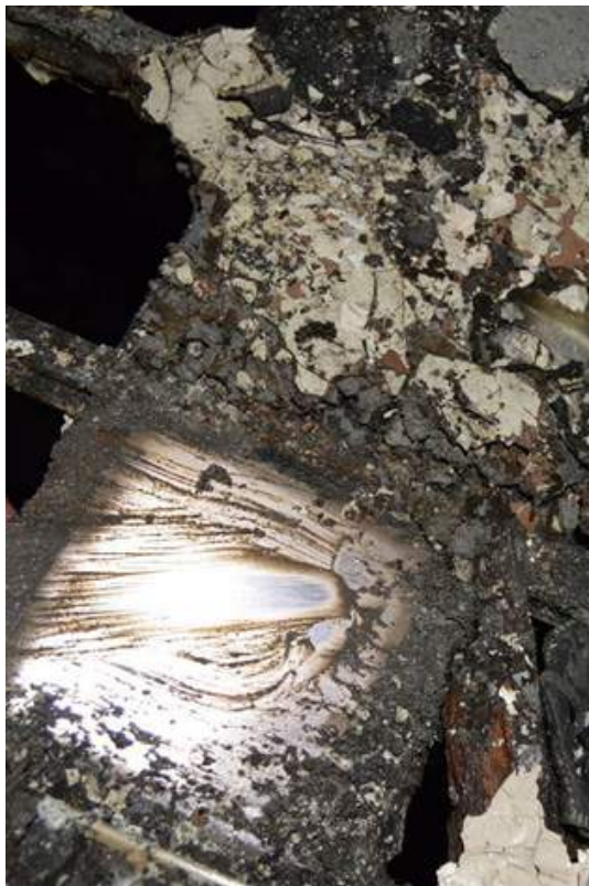
Plate 59.4: Glass tile in metal frame to the floor of the lobby.
