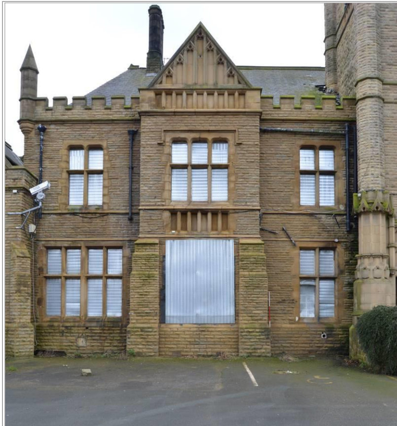
Plate 15: Front elevation view of administrative east range. Scale 2m. Facing south east.
