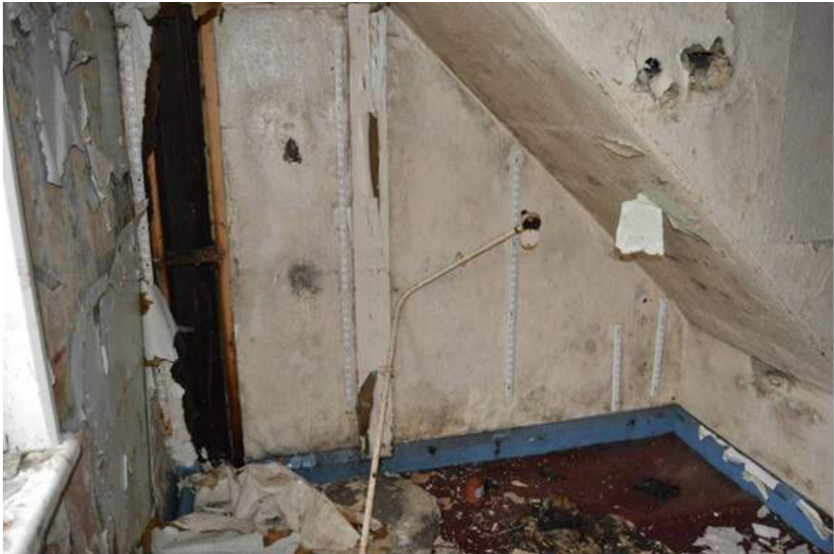
Plate 55.3: View beneath the stairs in room F13.
