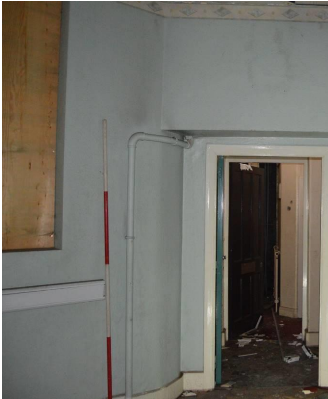
Plate 91.7: View towards the east sanitary wing (facing east). Scale 2m.
