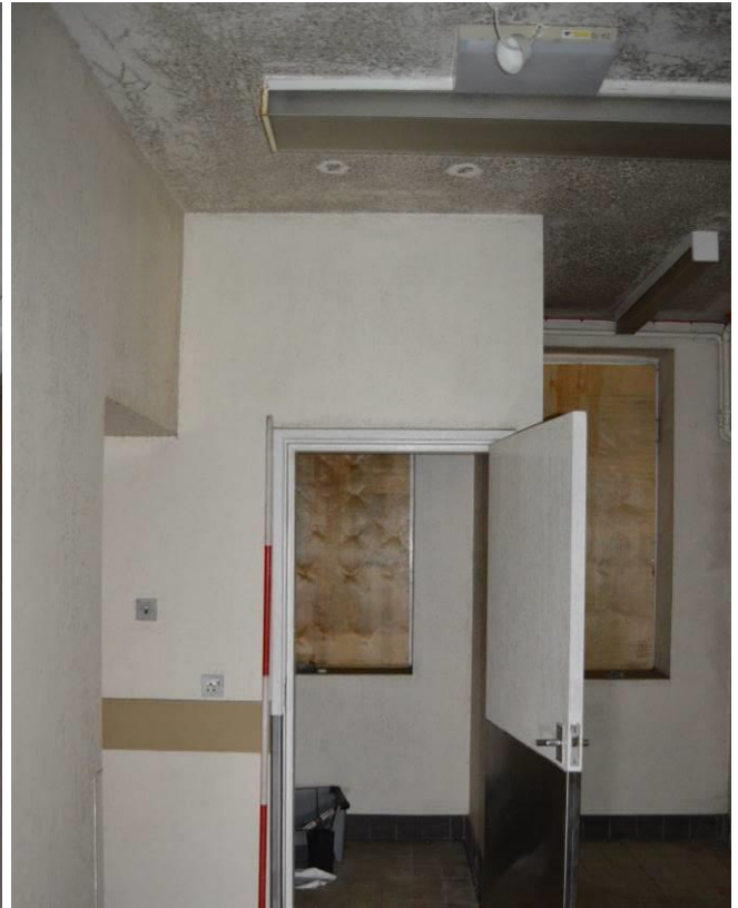
Plate 80.2: Detail into room G12.6 from G12. Scale 2m. Facing east.
