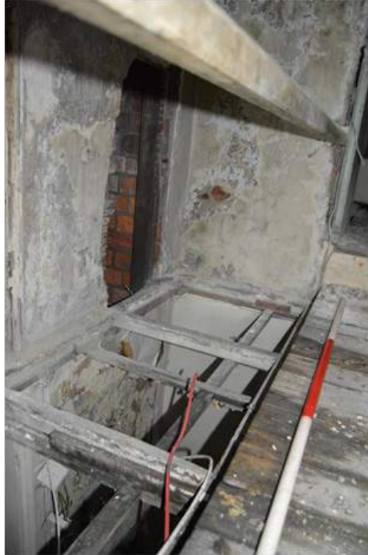
Plate 61.2: View above the landing F1. Scale 2m.
