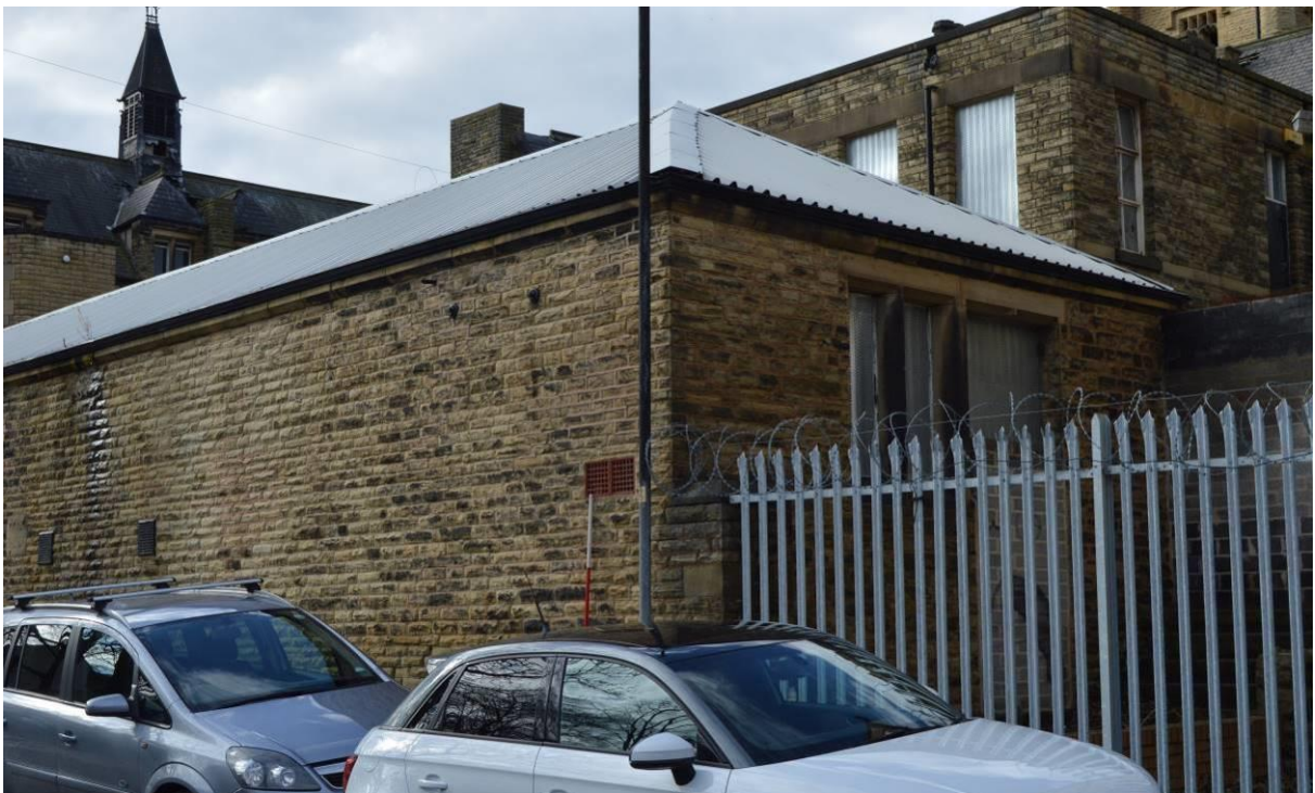
Plate 99.1: South east corner of the laundry building (facing west). Scale 2m.
