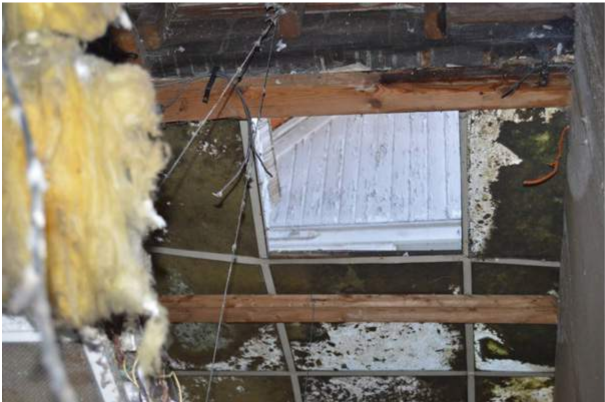
Plate 89.3: Operating theatre skylight in situ above later suspended ceiling.
