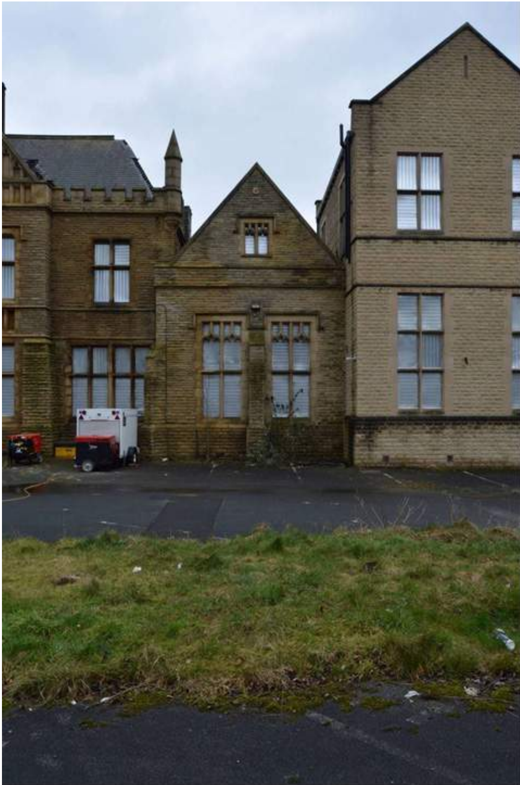
Plate 83: Exterior of linking range incorporating the board room.
