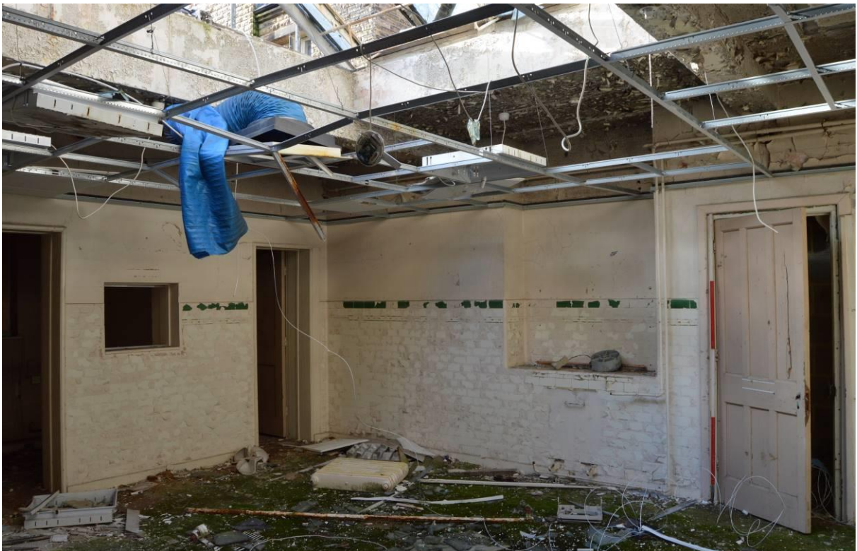
Plate 91.17: Later arrangement of dispensary/out-patients waiting room (facing west). Scale 2m.
