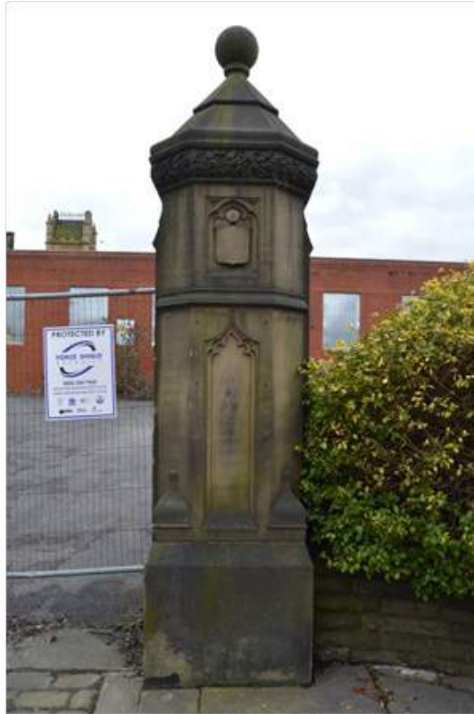
Plate 109.5: East gate, front face of north gate post.
