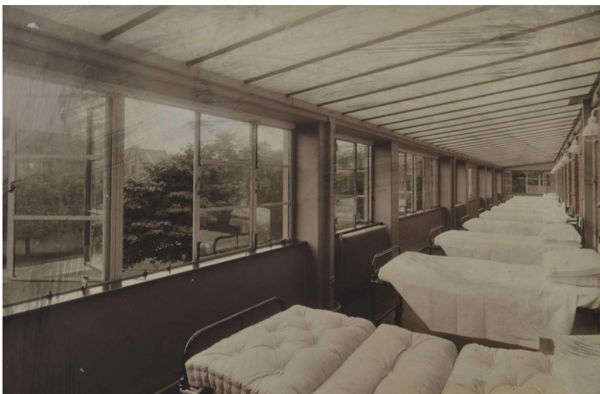
Figure 5: Interior of the sun lounges/verandas as originally set out (Wakefield Archives).
