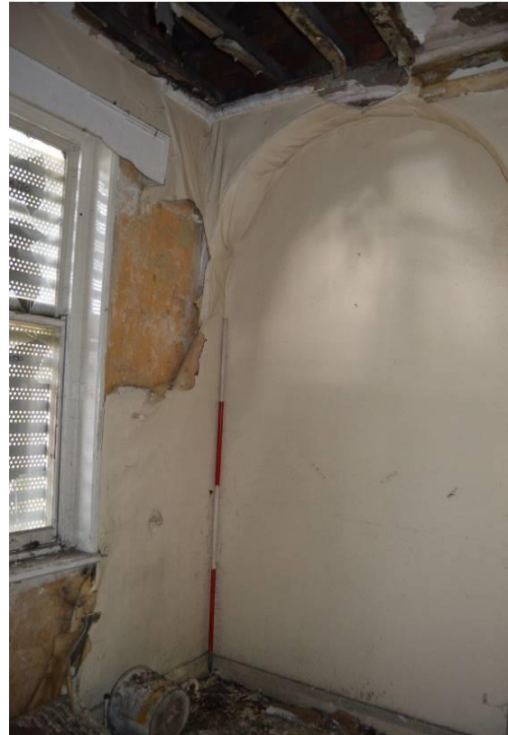
Plate 37.2: Arched recess for shelving and section of window in asst. surgeon's bedroom. Scale 2m. Facing north.
