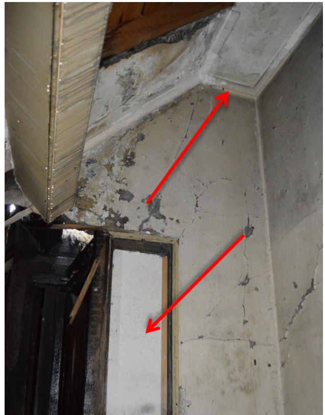
Plate 61.4: View of the lightwell plasterwork. Note the squint type opening in the far wall. Facing north east.
