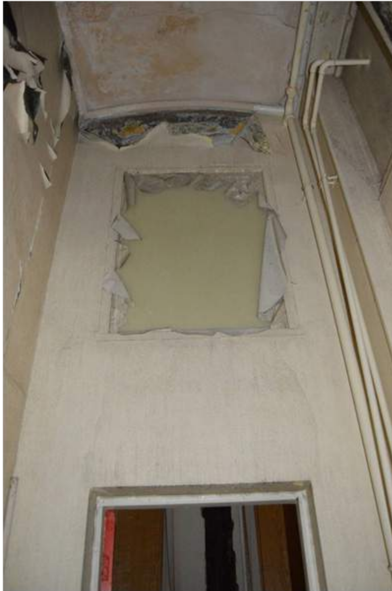
Plate 91.13: Interior window to lobby of west sanitary wing.
