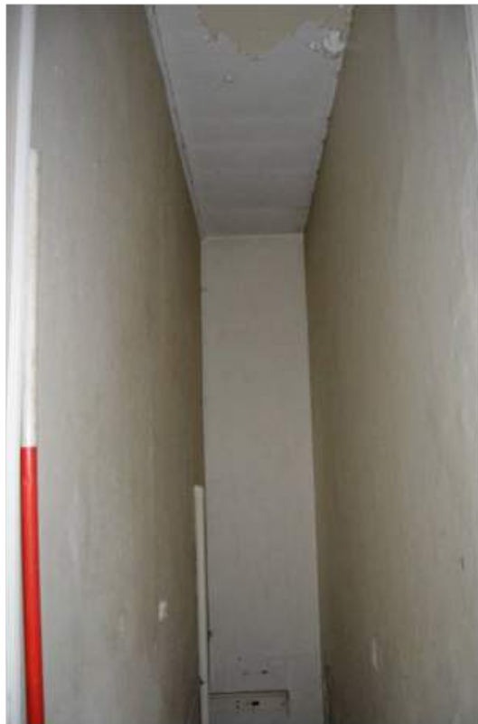
Plate 35.1: Plain ceiling above stair. Scale 2m.
