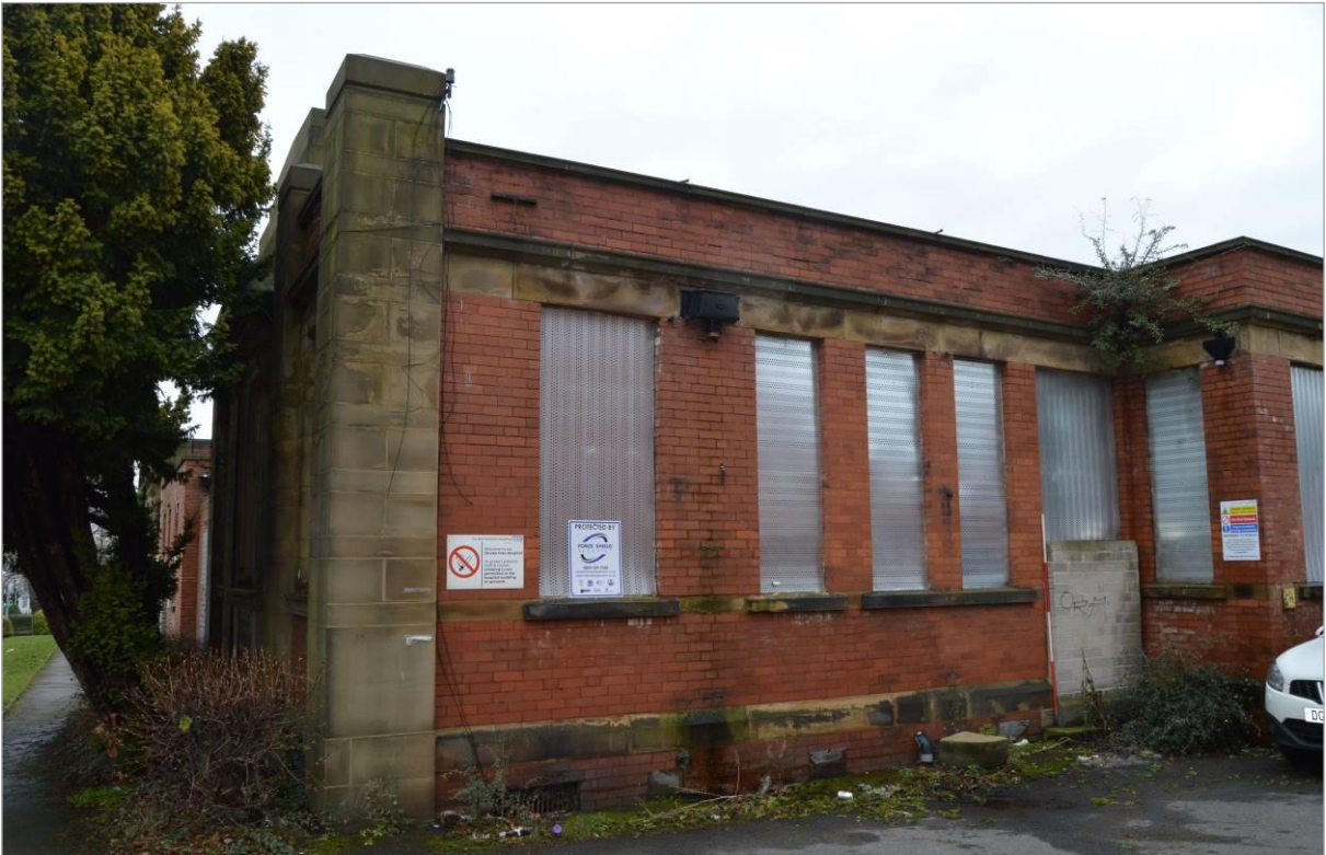
Plate 104.1: Side elevation to X-Ray wing, facing south east. Scale 2m.
