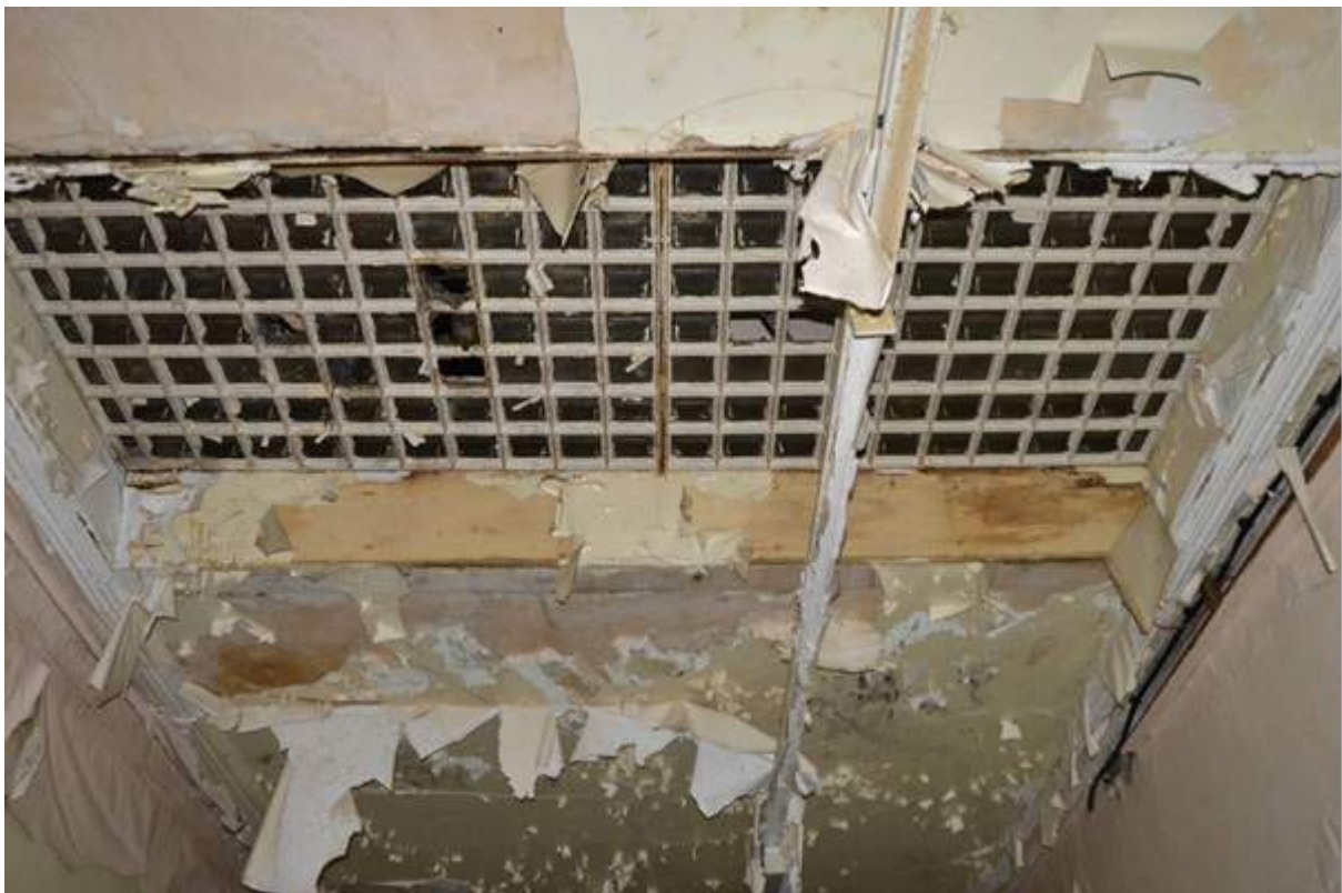
Plate 24: Glass tiled ceiling/floor above the axial corridor.
