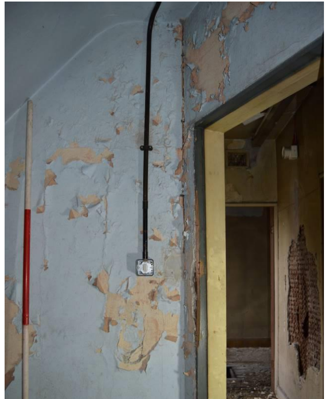
Plate 68.7: View from within room S10. Scale 2m. Facing north.
