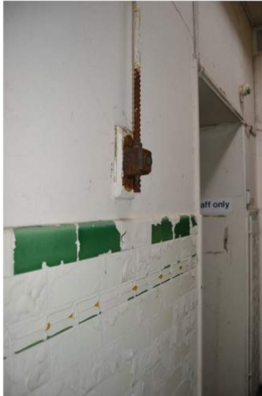
Plate 91.18: Interior fittings to dispensary area.
