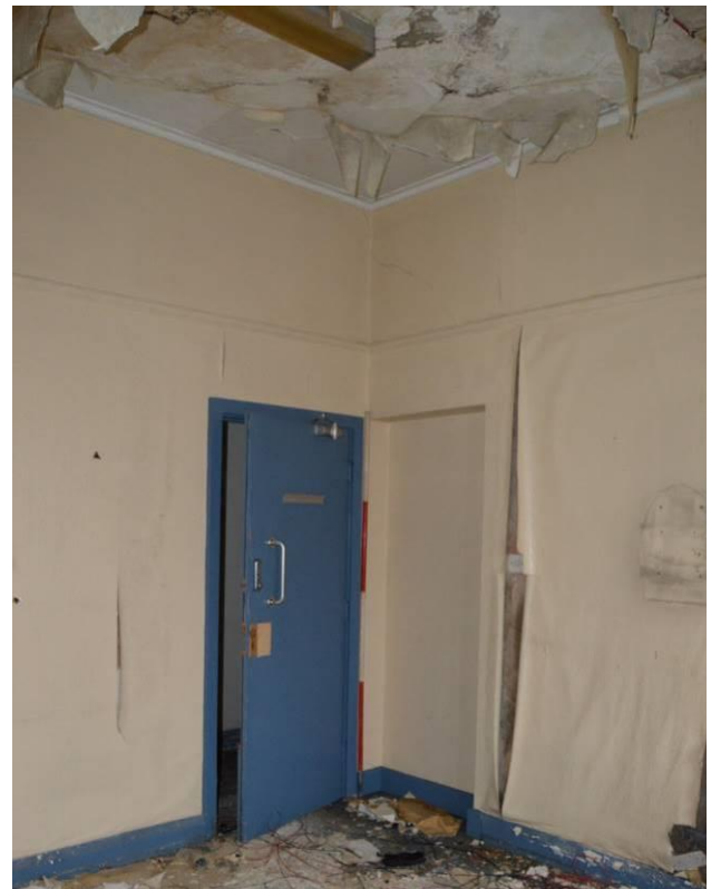
Plate 43.4: Late doorway next to blocked original opening. Scale 2m. Facing south.
