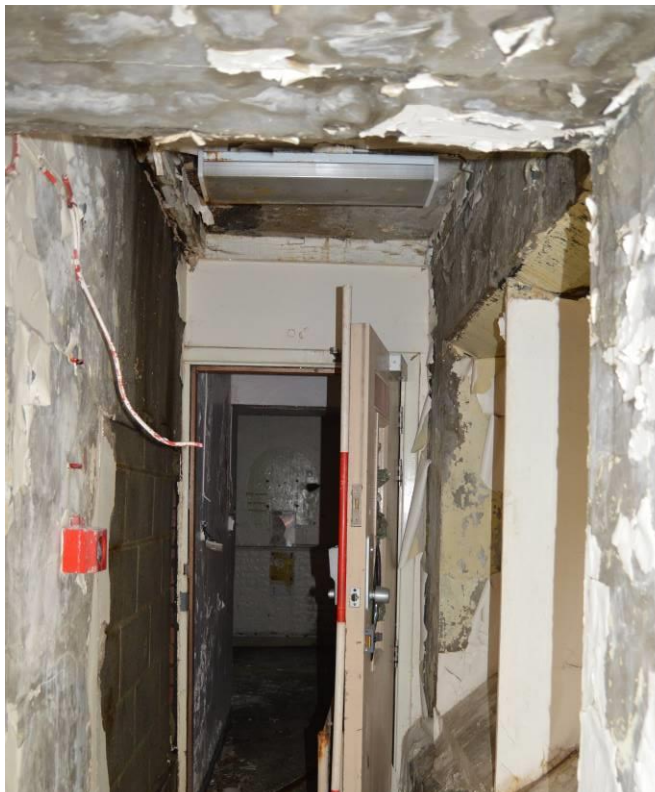
Plate 91.20: Modern corridor returning to the main axial route window (facing north west). Scale 2m.
