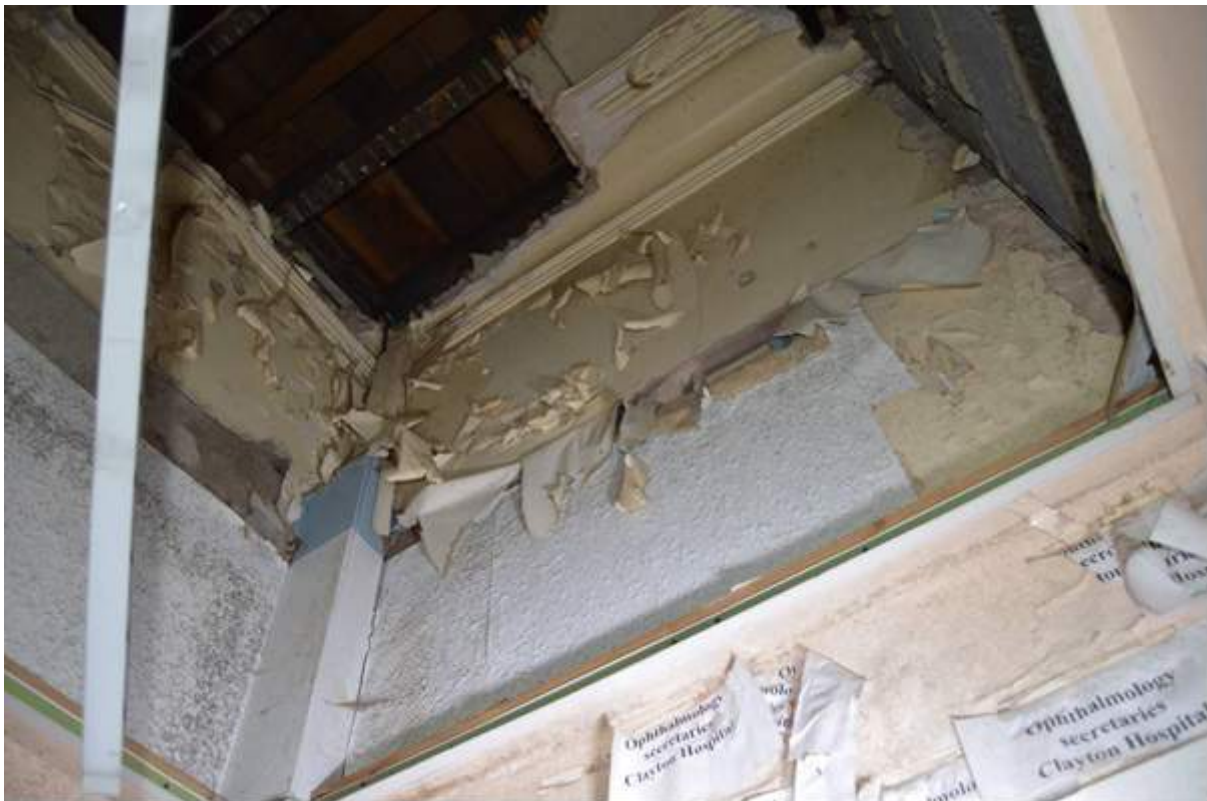
Plate 31: Surgeon's sitting room cornice in place above modern dumb waiter enclosure.
