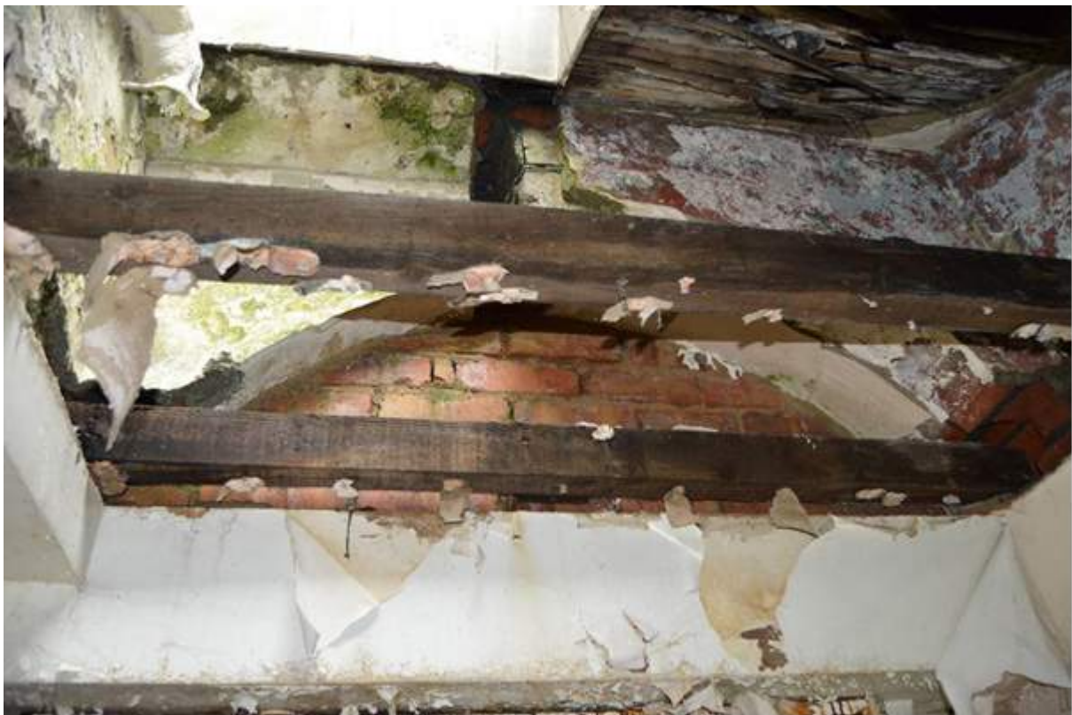
Plate 82: Arch above the half-landing of the nurses' stair half-landing.
