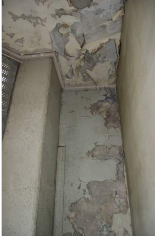
Plate 38.2: Retained beaded cornice above modern partitions.
