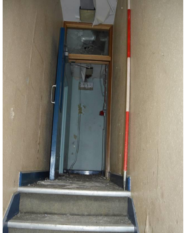
Plate 67.1: The corridor giving access to S3 and other rooms in the west section of the second floor accommodation. Scale 2m. Facing north west.
