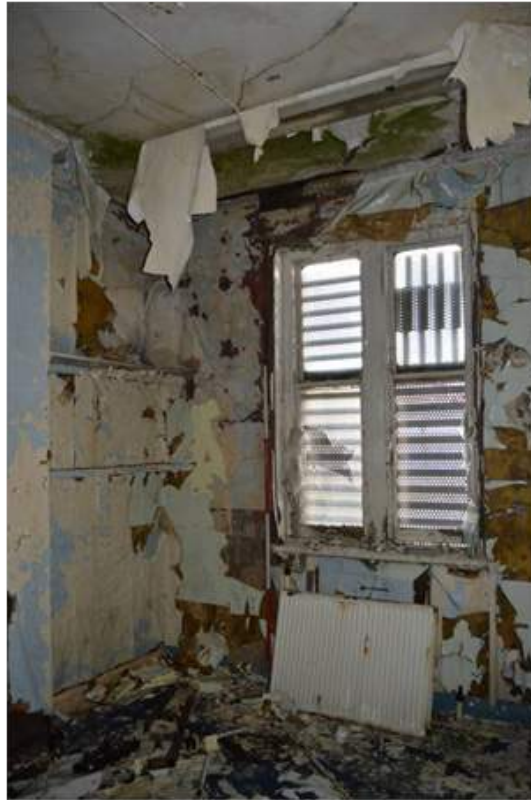
Plate 48.2: Sash window. Scale 2m.
