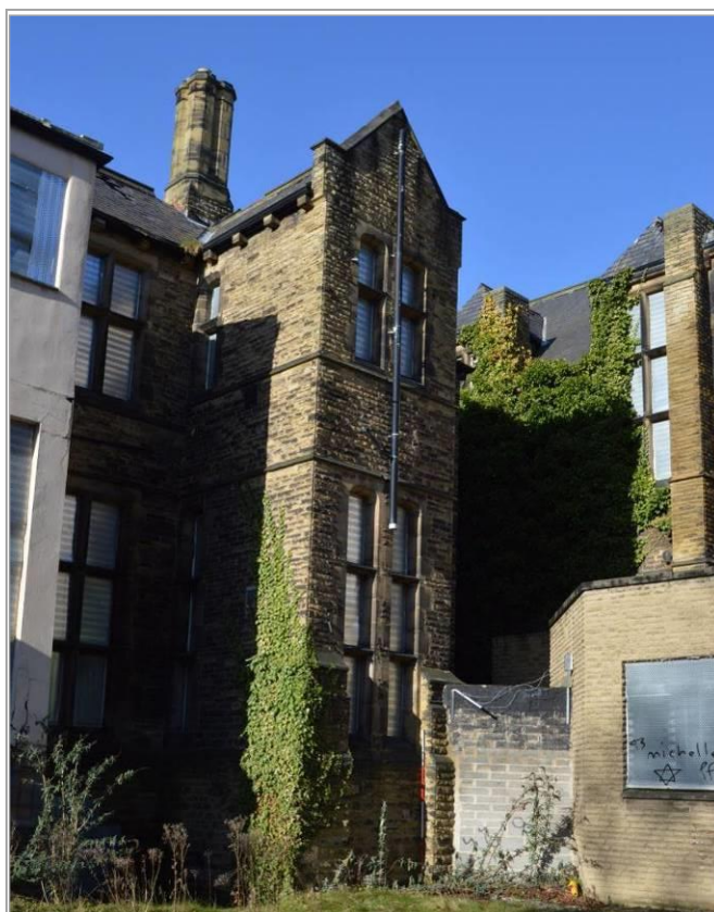
Plate 95: North facing elevation of the special ward (facing north). Scale 2m.
