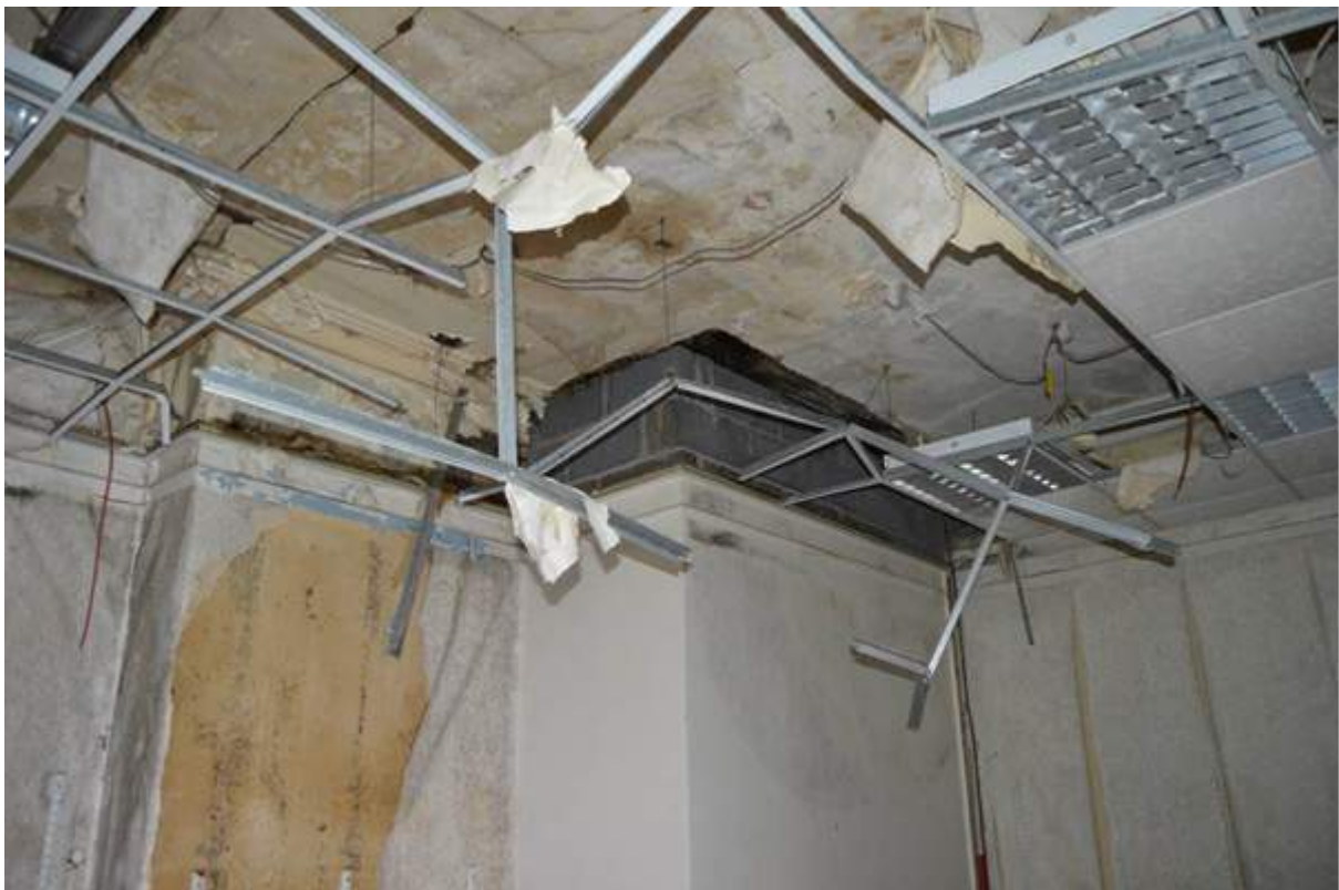
Plate 29.1: Later dumb waiter shaft inserted in room G7.
