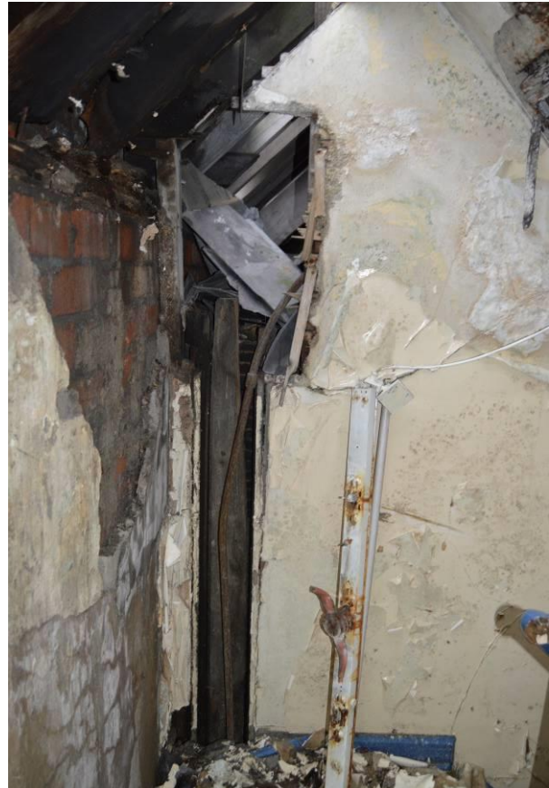
Plate 56.4: Corner of half-landing. Facing east.
