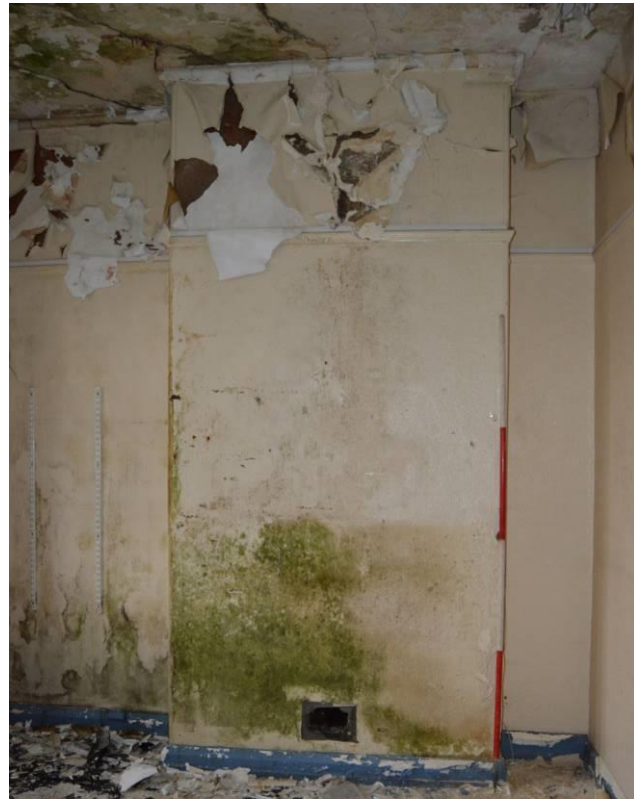
Plate 43.2: Chimney in room F6. Scale 2m. Facing north east.
