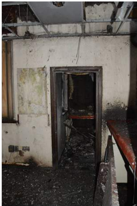
Plate 89.1: View through the theatre.
