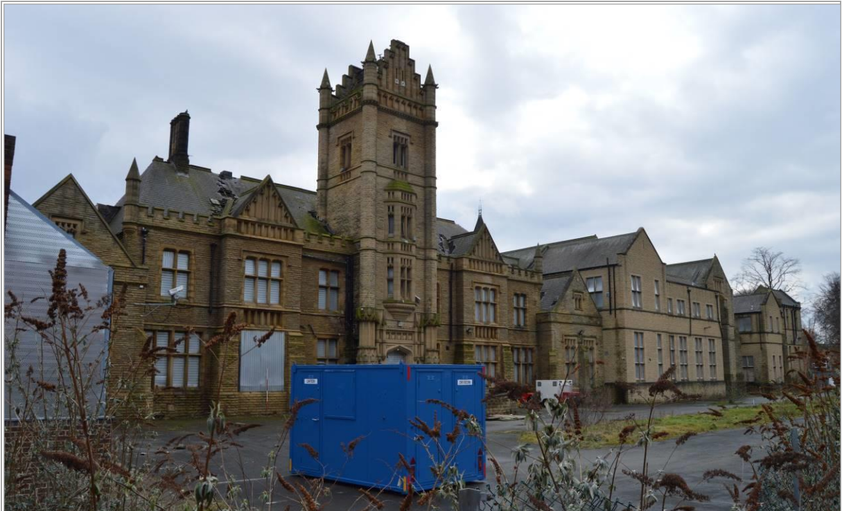
Plate 2: View administration range facing south. Facing south west. Scale 2m.
