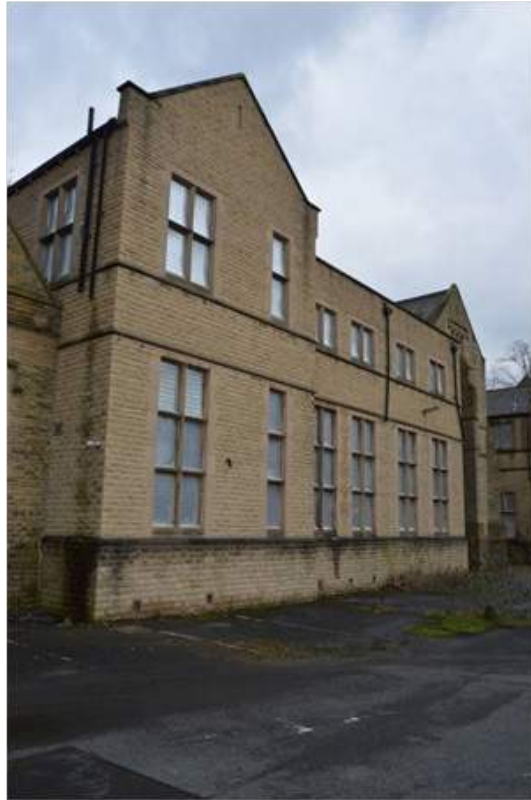
Plate 93: Modern extension to the north face of the original building. Scale 2m.
