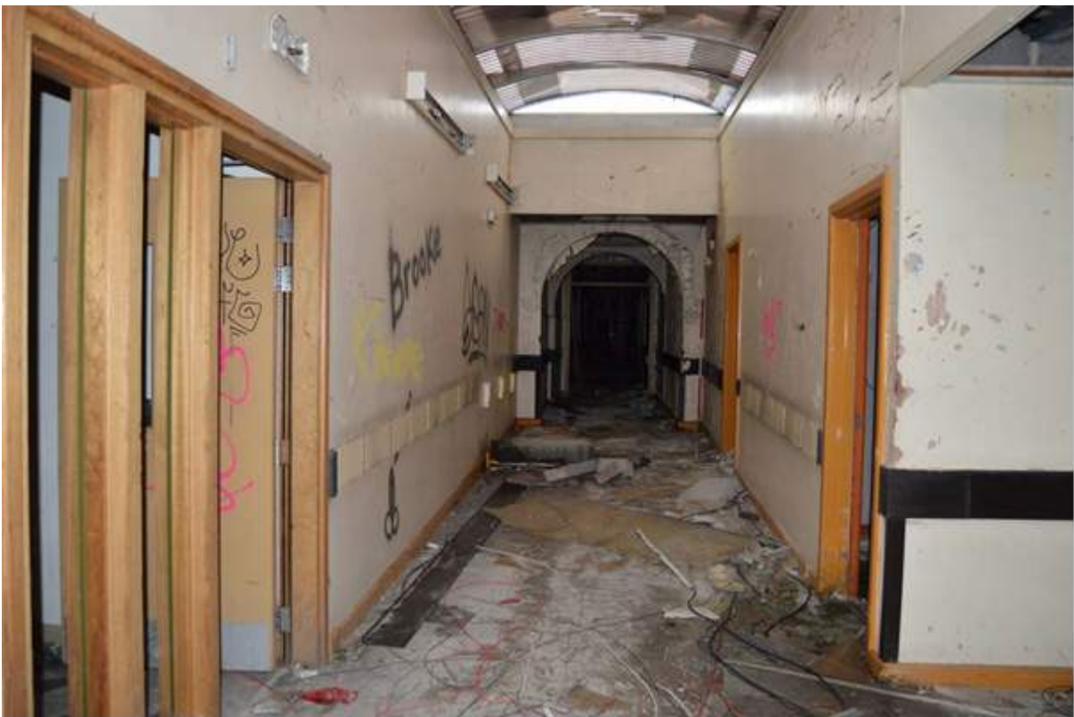
Plate 101.8: View of the later linking corridor. Scale 2m.
