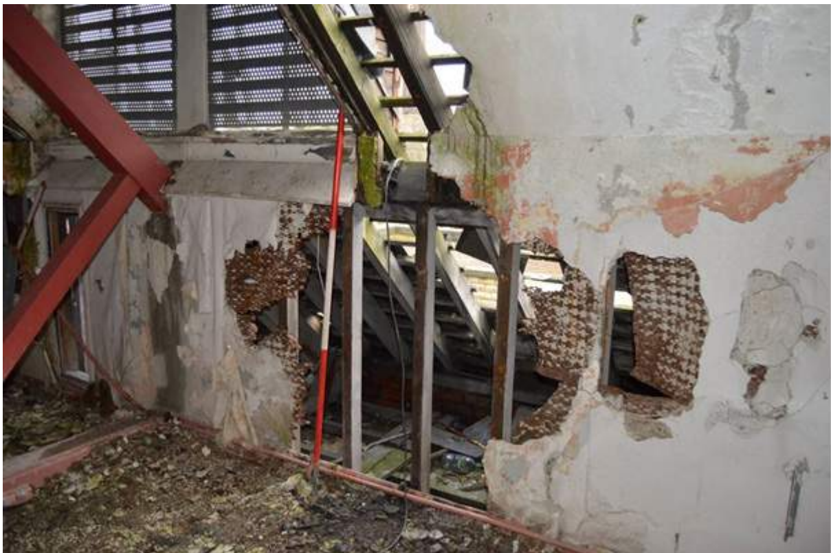
Plate 66.1: Room S3 with mesh and plaster wall construction. Scale 2m.
