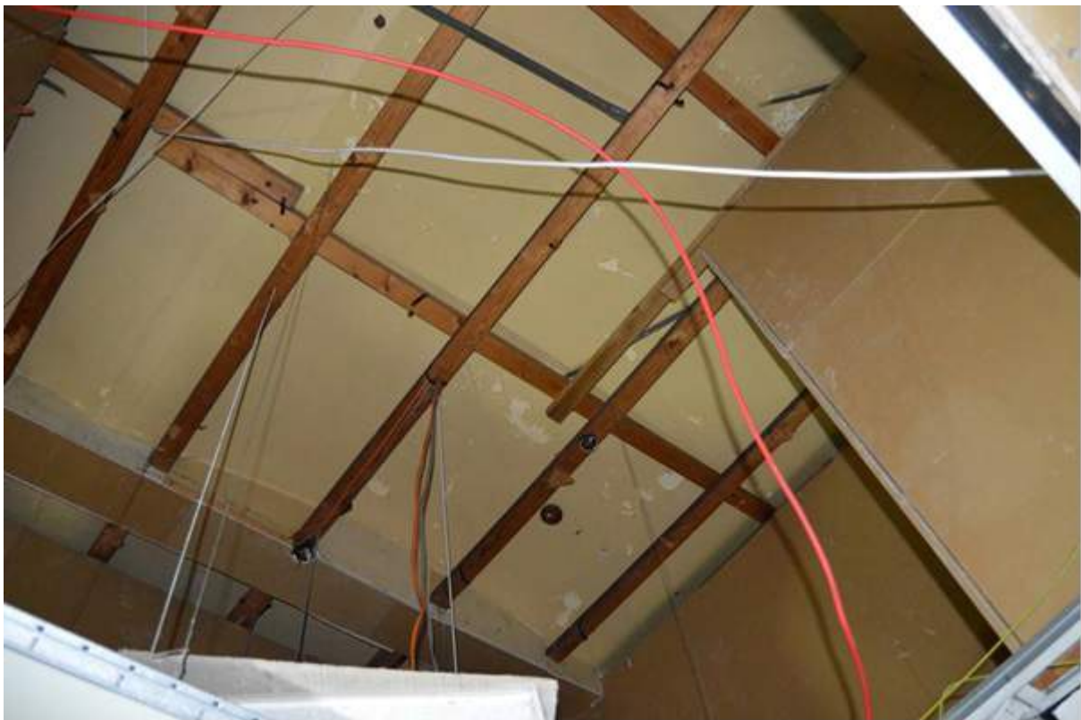
Plate 91.6: Original barrel vaulted plaster ceilings to dispensary/out-patients' consulting areas.
