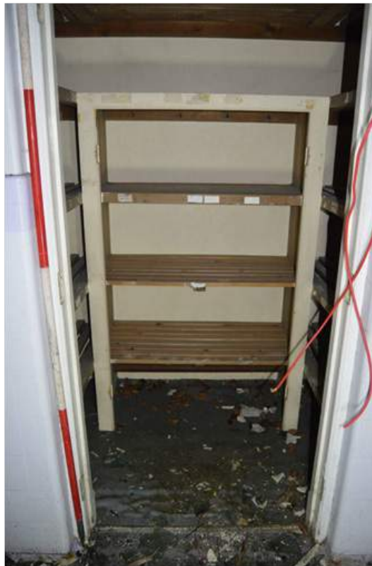
Plate 104.10: Airing cupboard off X-ray corridor. Scale 2m.
