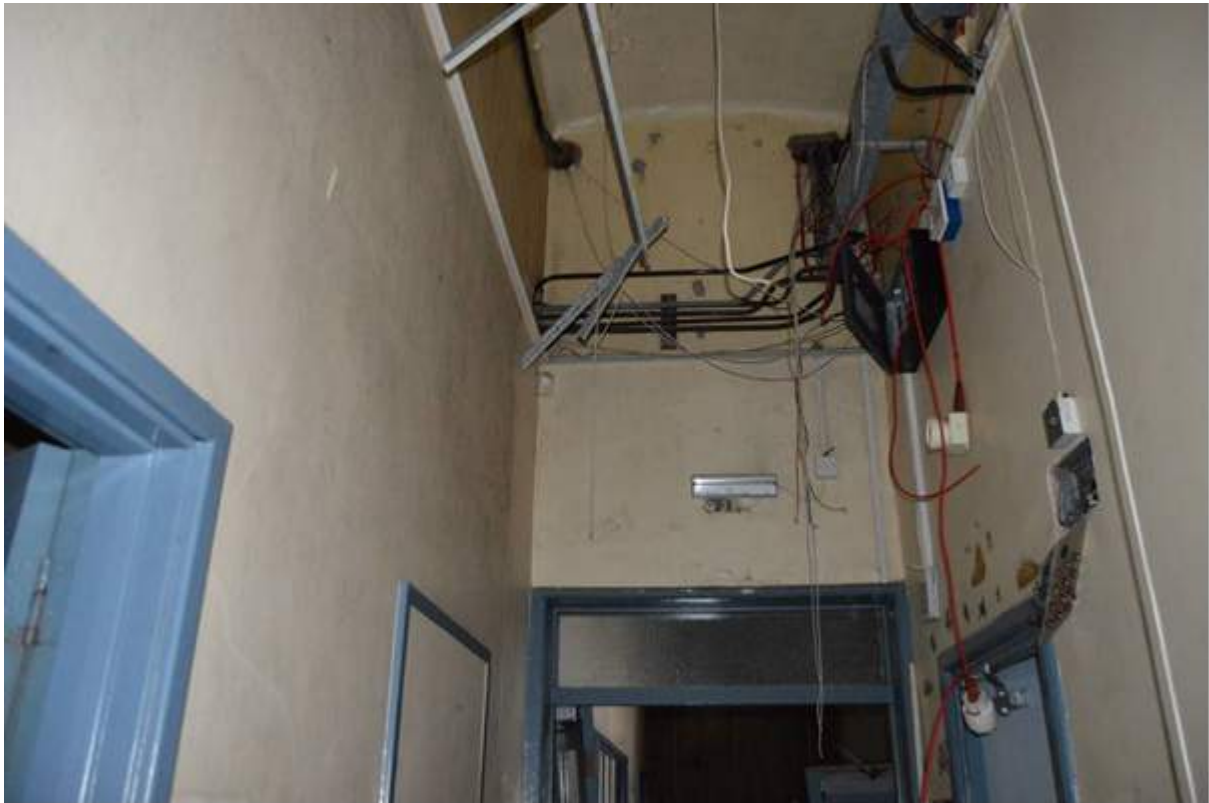
Plate 92.3: View of the barrel vaulted ceiling, an original feature of the ward lobby.
