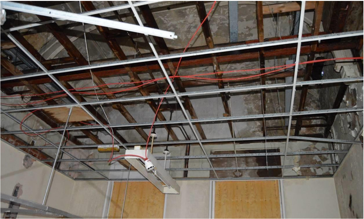
Plate 86.3: View of the ceilings above the board room (facing west).
