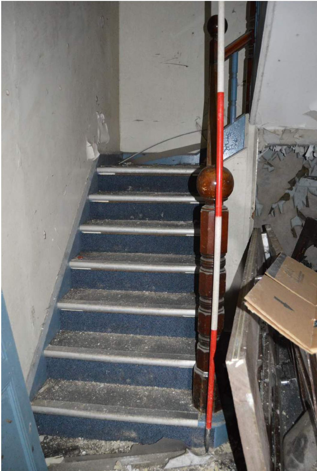
Plate 22.1: Stairs to first floor of administration range. Scale 2m.
