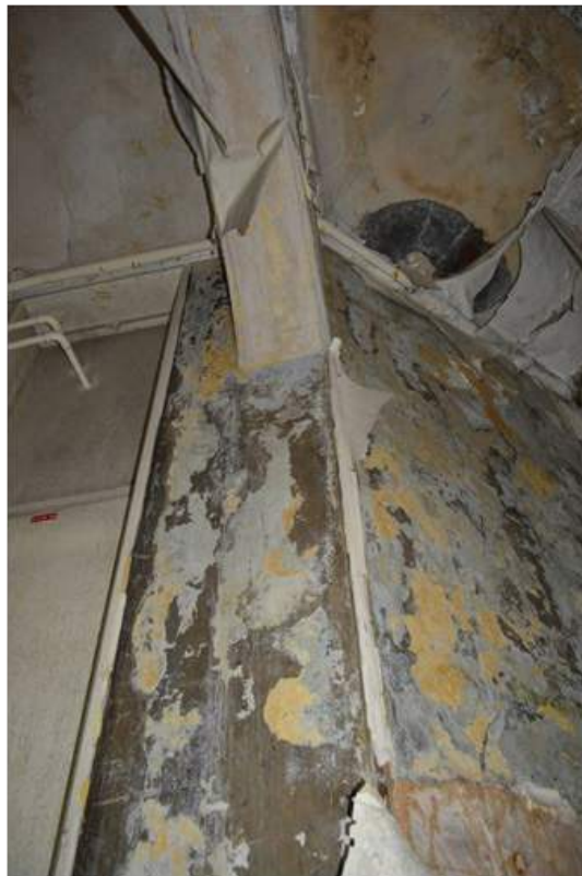
Plate 91.12: Original plaster finishes to west sanitary wing area.
