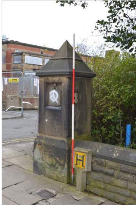
Plate 109.9: West gate, front face of north gate post. Scale 2m.
