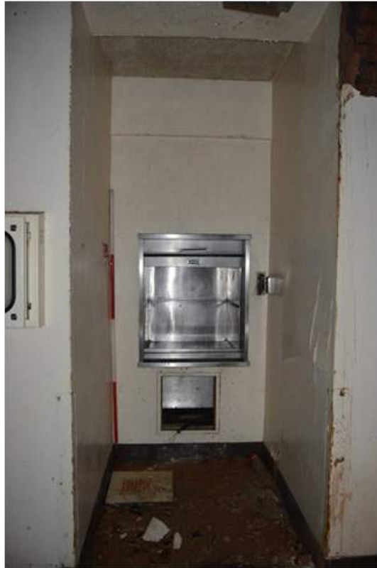
Plate 79.3: Detail of modern dumb waiter in room G11.1. Scale 2m.
