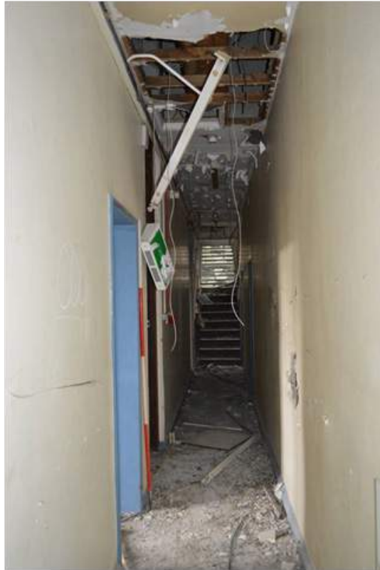
Plate 47: View along nurses' corridor with light well to ceiling. Scale 2m.
