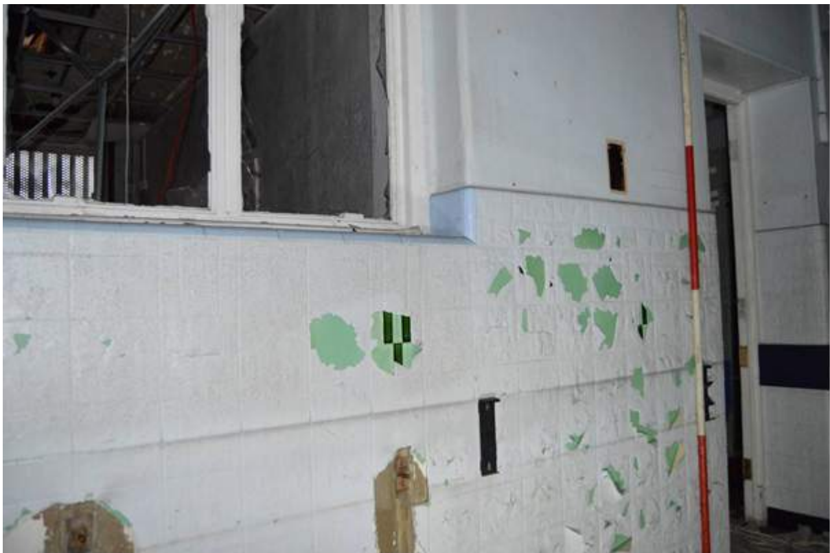
Plate 104.6: Tiled wall finish to X-Ray wing corridor. Scale 2m.
