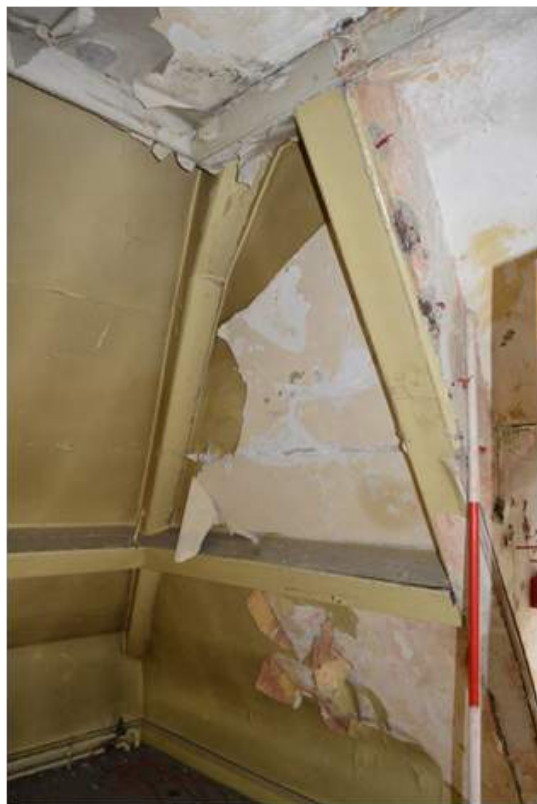
Plate 68.6: Trusses supporting the eastern hip incorporated into the interior space. Scale 2m.
