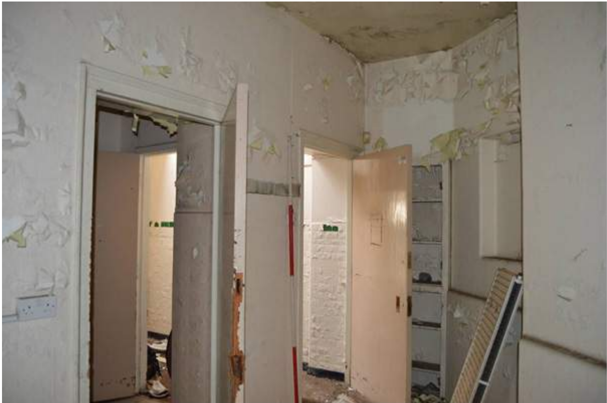
Plate 91.16: Room G26 formed by a later extension added to original east pavilion ward ground floor. Scale 2m.
