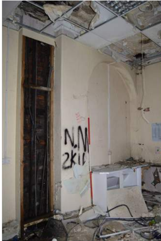
Plate 28.3: Alcove to room G6 with cornice above. Scale 2m.
