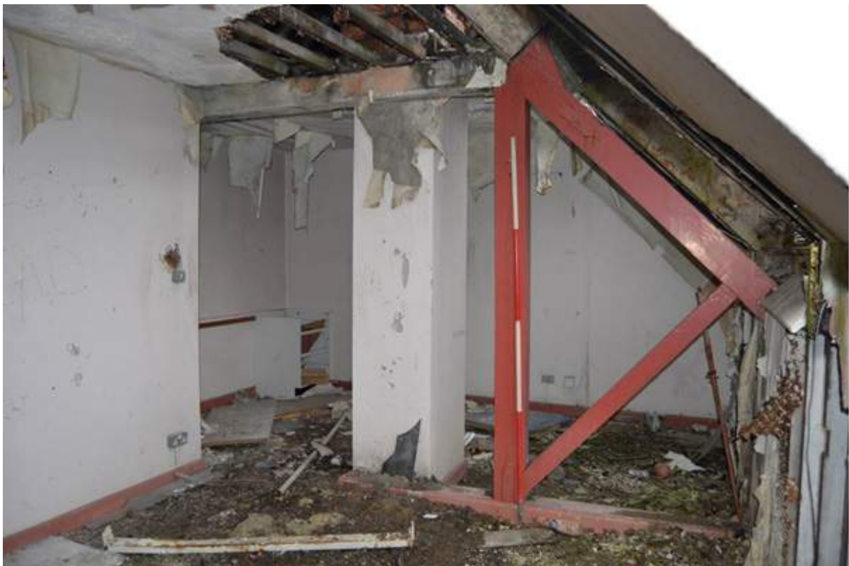
Plate 65.2: Repaired timber truss to room S3. Scale 2m.
