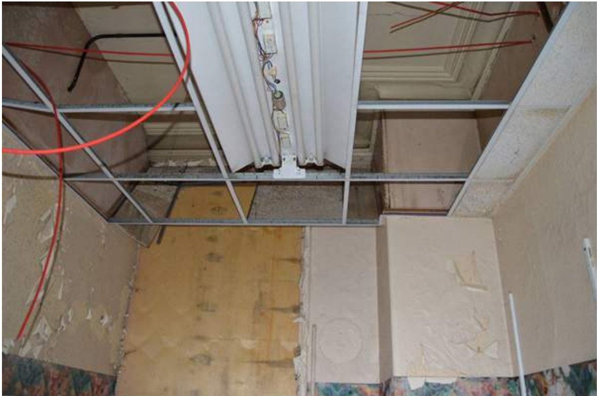
Plate 25: Plaster corning retained to G4/Matron's room.
