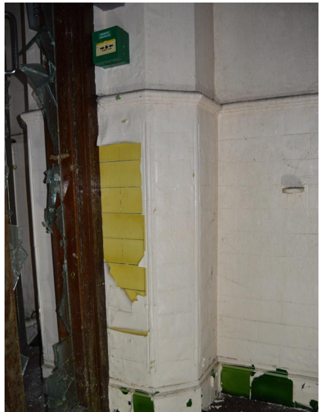
Plate 19.6: Surviving tiling scheme in visitor's hall. Facing north.
