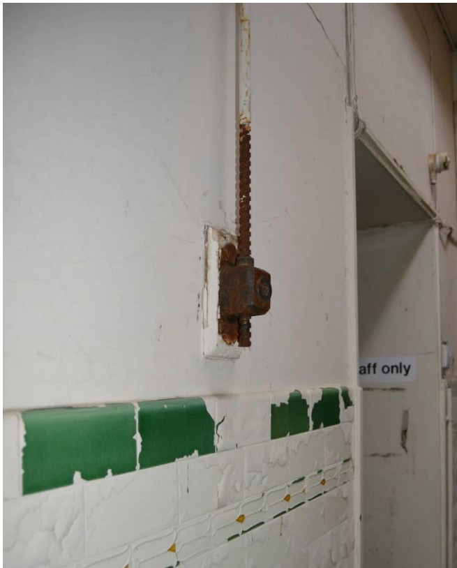
Plate 91.18: Interior fittings to dispensary area (facing south east).
