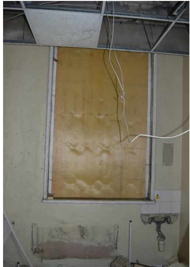
Plate 20.3: View of window in room G2. Facing north west.
