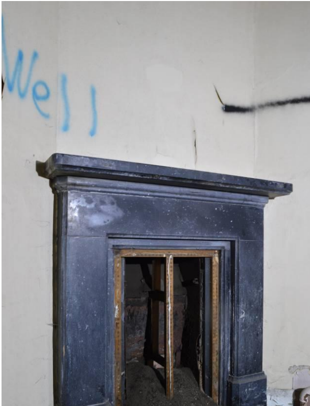
Plate 28.1: Corner fireplace to room G6. Facing south.
