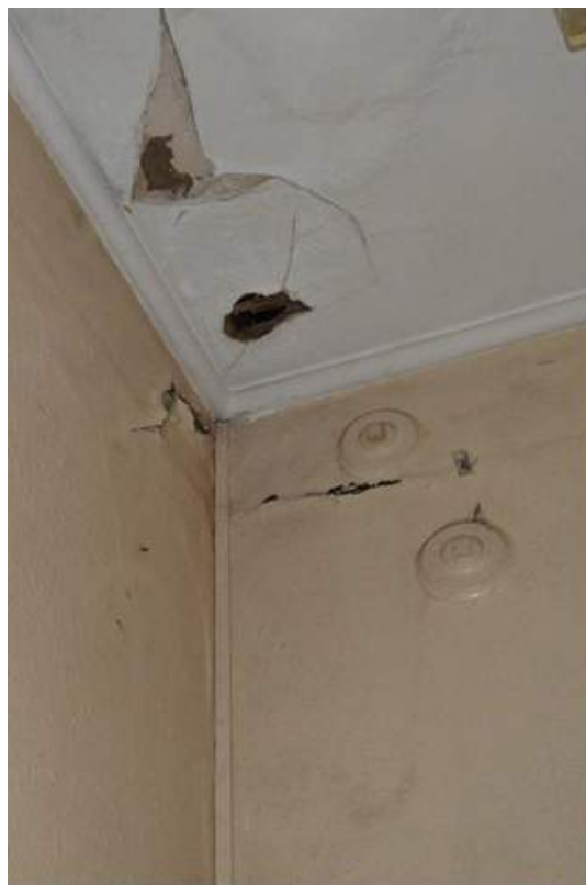
Plate 53.4: View of tie plate fittings to room F11.
