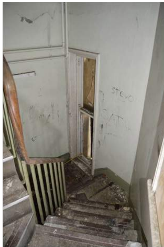
Plate 101.6: View down the stairs to half-landing.
