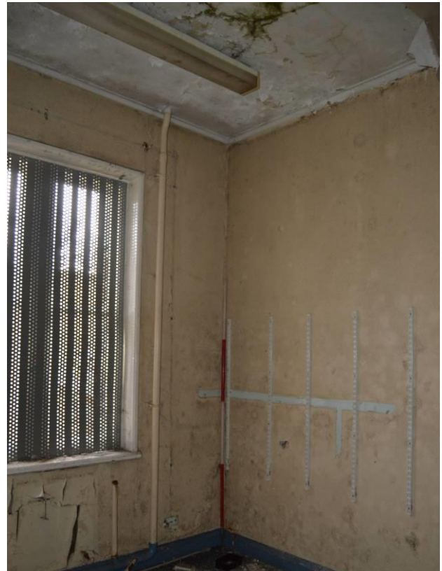
Plate 54.2: Nurse's bedroom, note lack of corner chimney piece. Scale 2m. Facing north.
