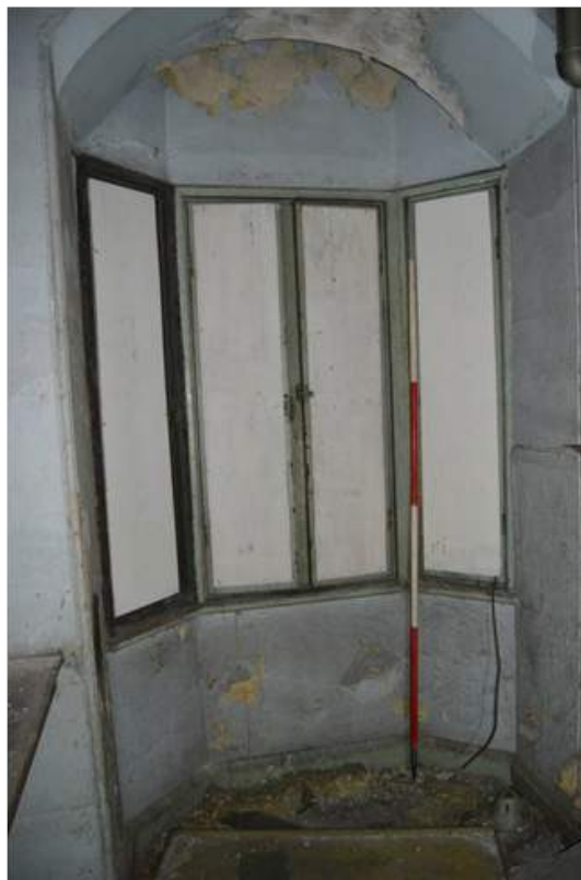
Plate 64.1: Top bay of the oriel window the tower with original shutters. Scale 2m.
