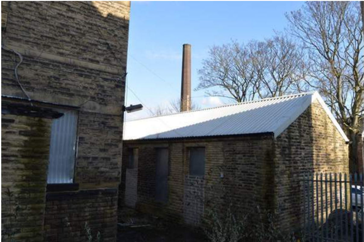
Plate 99.2: North west corner of the laundry range. Note there is a gable at this end. Scale 2m.
