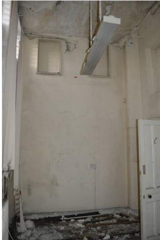
Plate 91.14: Blocked windows in converted W.C. room (G24).
