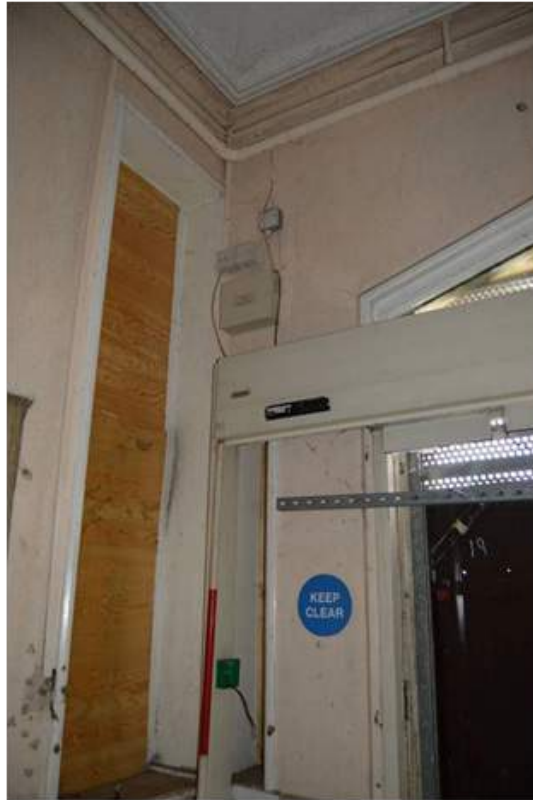
Plate 19.3: Detail of windows and coving to north corners of visitor hall. Scale 2m.
