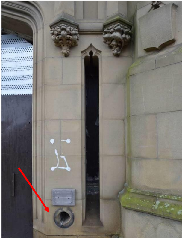
Plate 8: One of the lancet windows either side the entrance. Note, remains for a bell pull. Facing south east.
