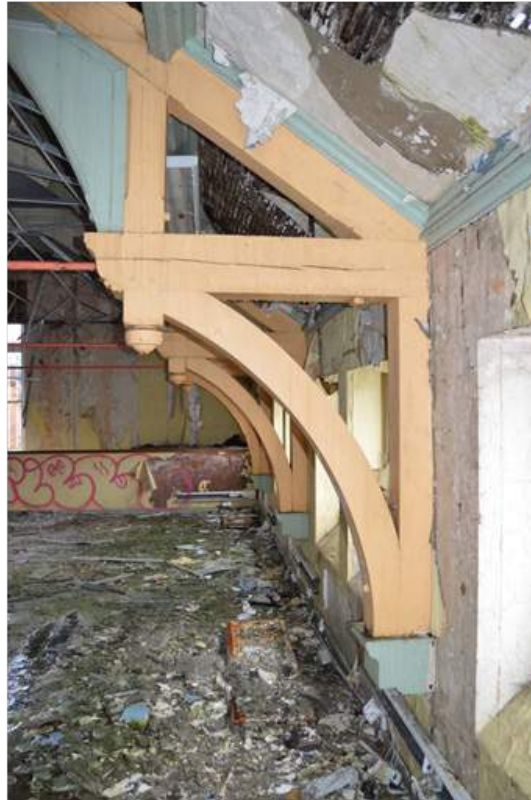
Plate 103: Upper level, retained ceiling features to out-patient's waiting room.
