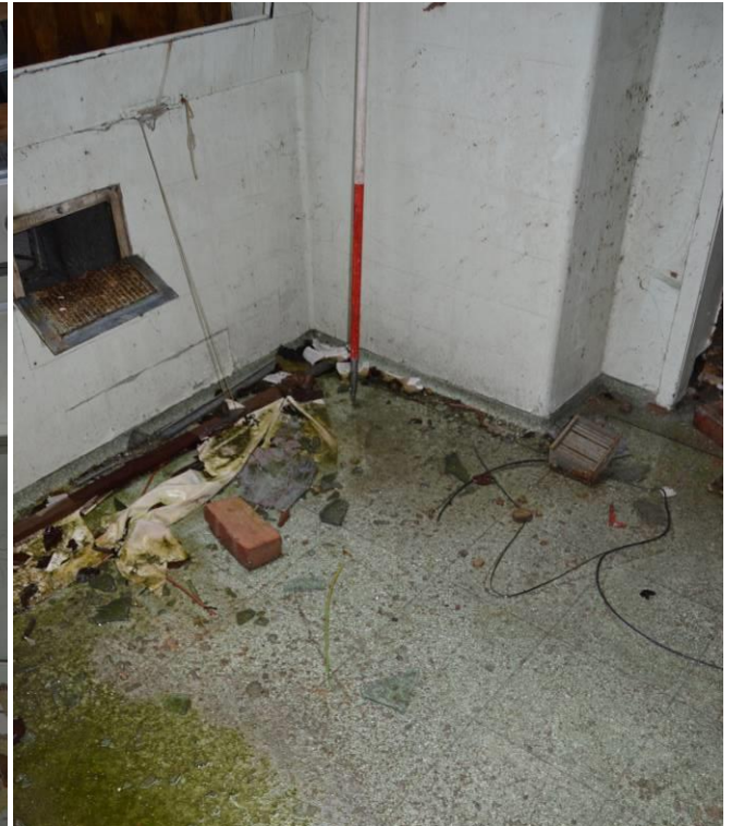
Plate 105.6: Terrazzo floor of the operating theatres (facing north). Scale 2m.
