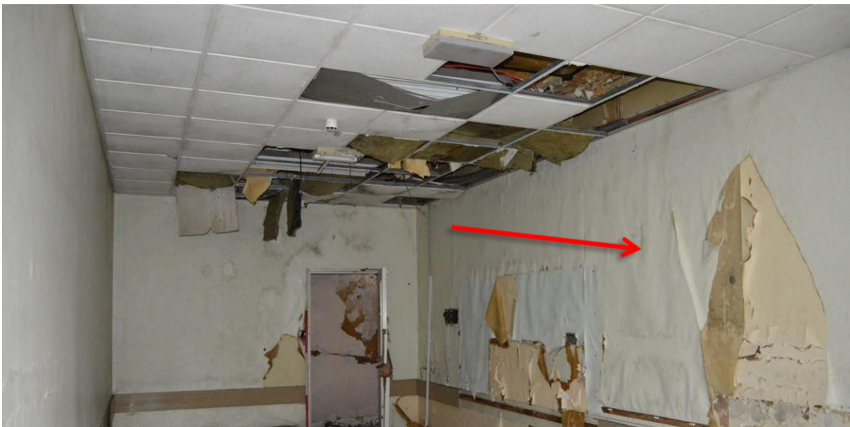
Plate 60.2: View facing east in the nurses' dormitory. Note the rough wall surface where the fireplace would have been located. Facing east.
