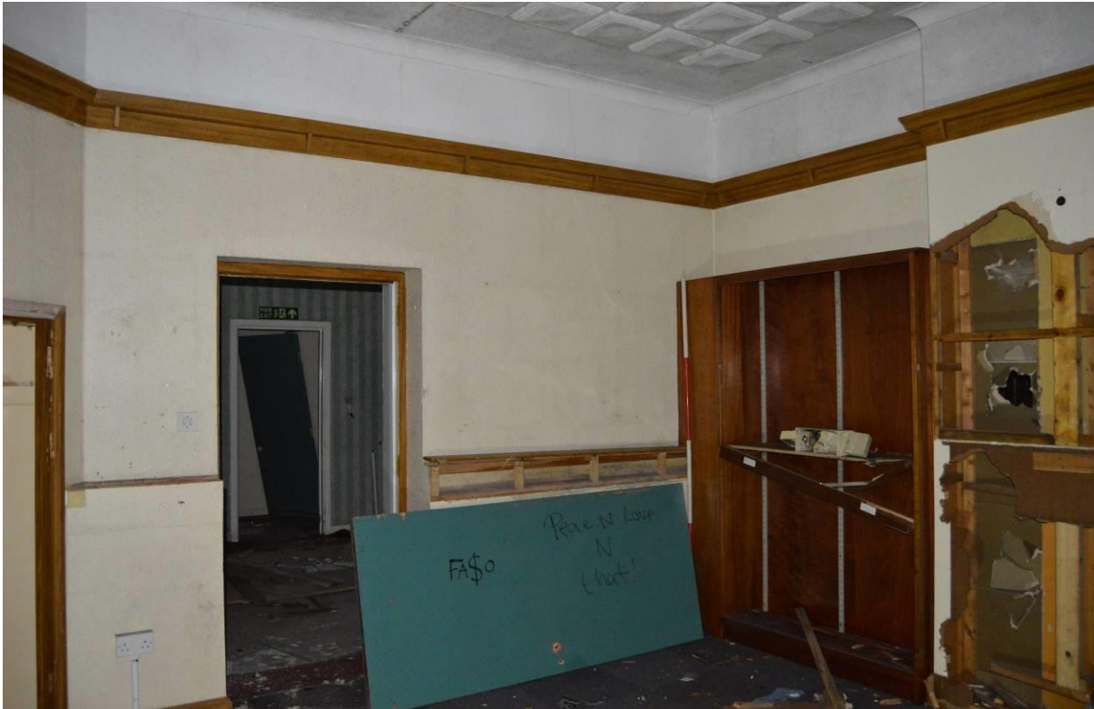
Plate 91.15: Former consulting room G25, now 20 th century office, in extension to east pavilion ward, ground floor (facing north). Scale 2m.
