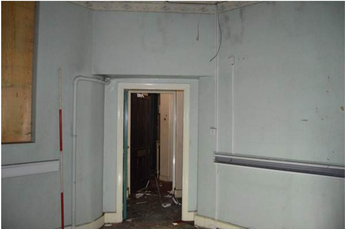
Plate 91.7: View towards the east sanitary wing (from G22). Scale 2m.
