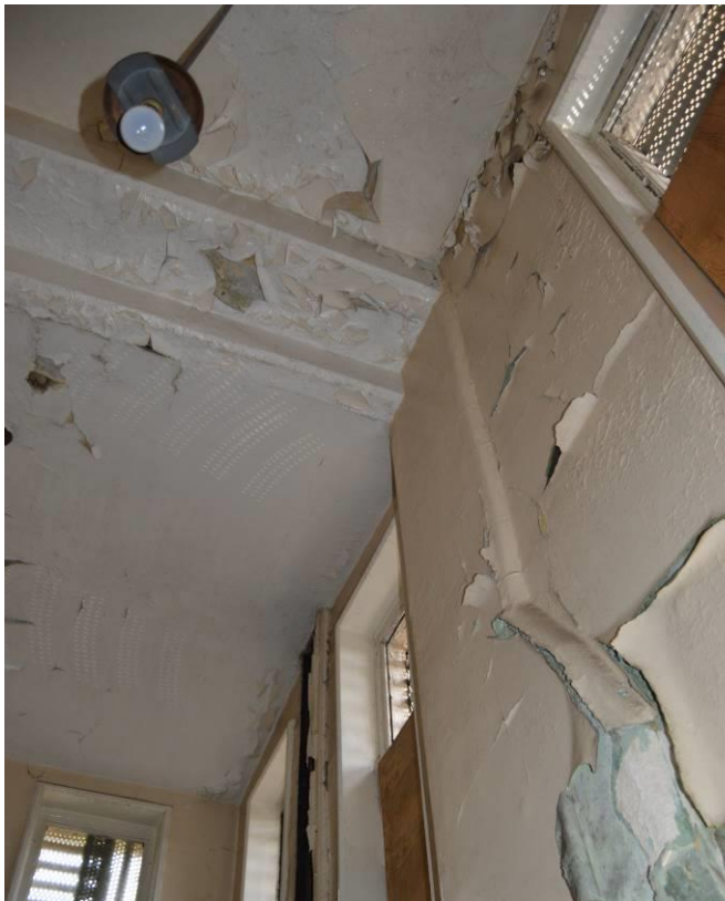
Plate 91.9: East sanitary wing later structural alterations/extension (facing east).
