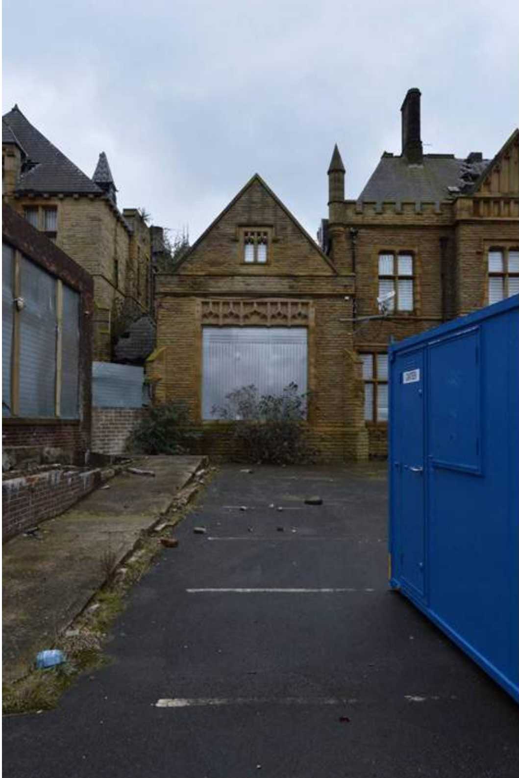
Plate 87: Front elevation of the eastern linking room, the original operating theatre.
