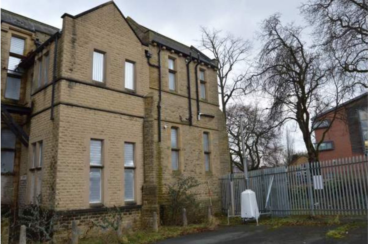
Plate 96.3: Side (north) elevation of the children's ward sanitary wing. Scale 2m.
