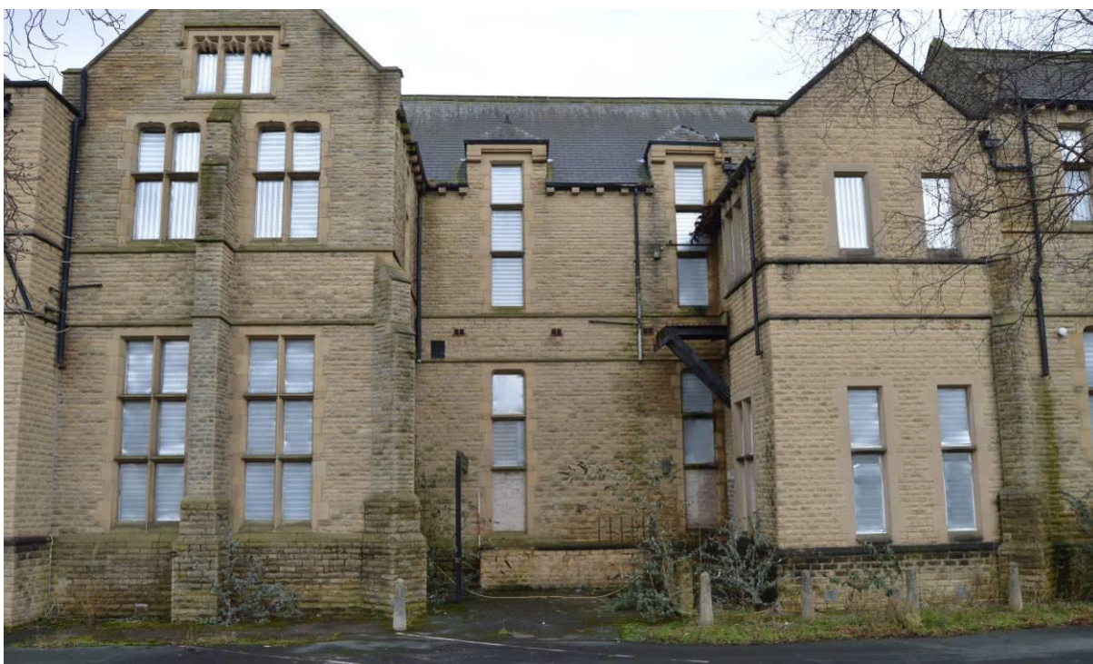
Plate 96.4: Children's ward north elevation between special ward and modern extension, facing south east.
