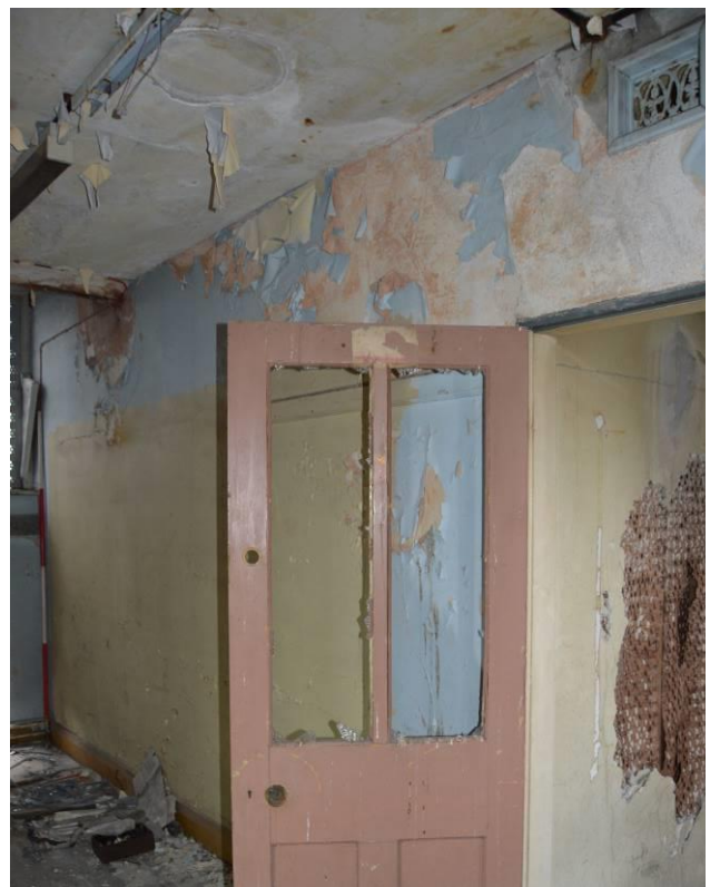
Plate 69.1: Half-glazed door to room S13. Scale 2m. Facing south.
