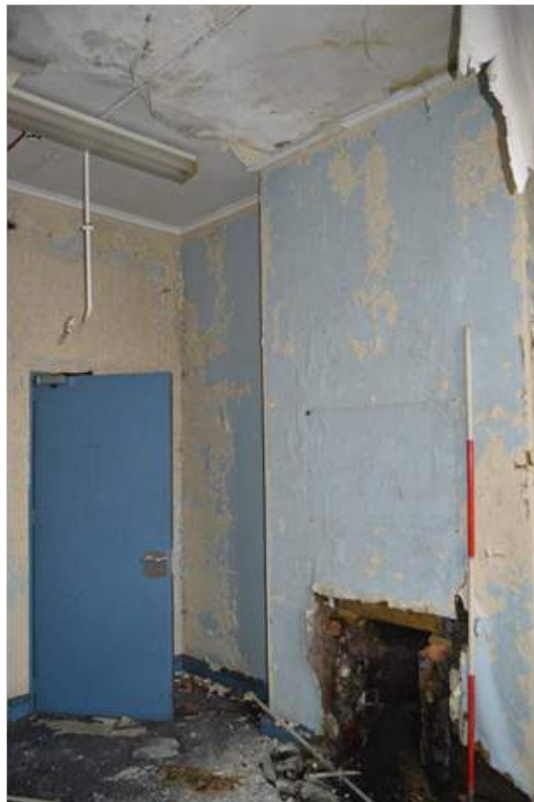
Plate 48.1: Chimney in room F7. Scale 2m.
