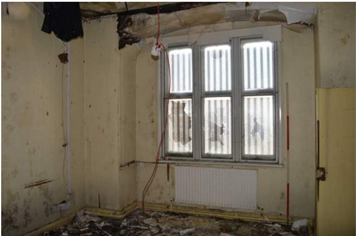
Plate 49.3: Window of the former matron's bedroom. Scale 2m.
