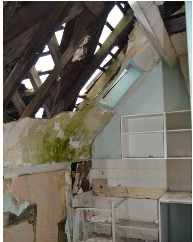
Plate 67.5: Room S5, with sloping ceiling with skylight. Facing north.
