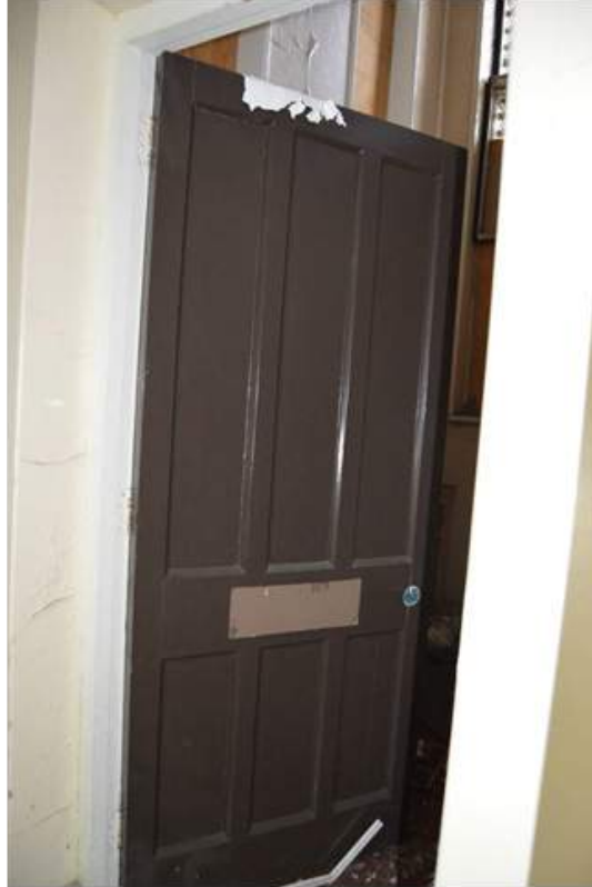
Plate 91.11: Original six panel door to sanitary wing.
