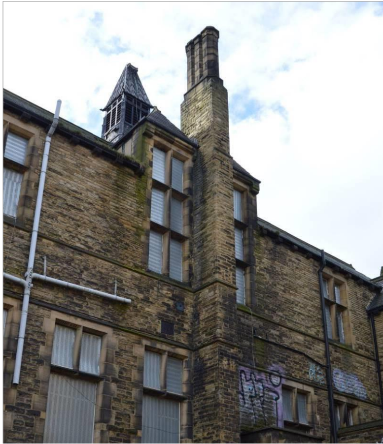
Plate 90.1: View of the eastern pavilion from the south (facing west).
