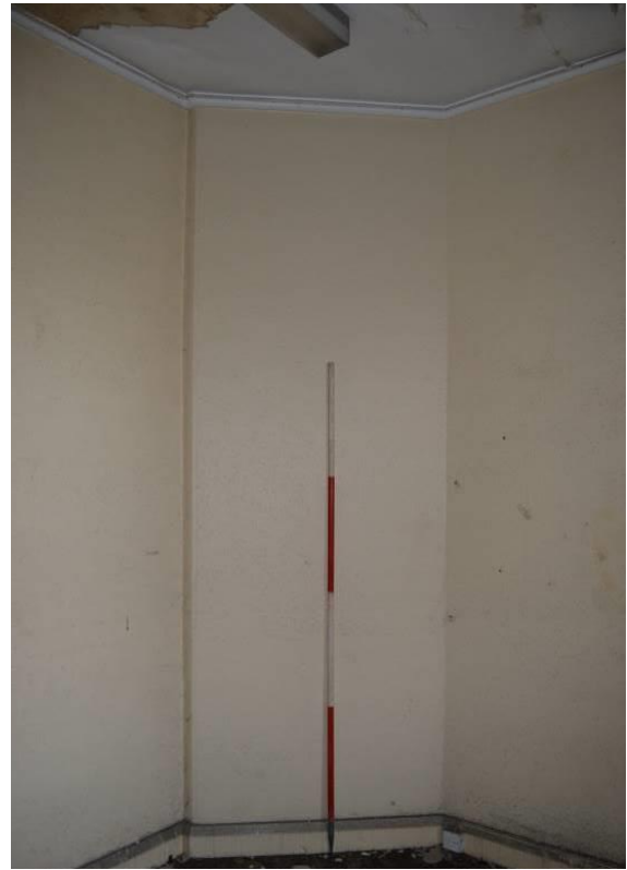
Plate 37.4: View of corner chimney to surgeon's bedroom. Scale 2m. Facing south.
