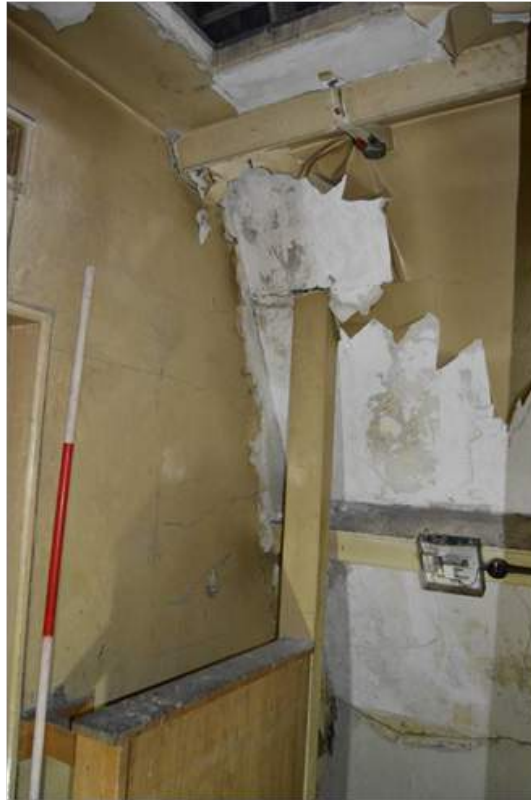
Plate 68.1: Plaster work within the roof space accommodation. Scale 2m.
