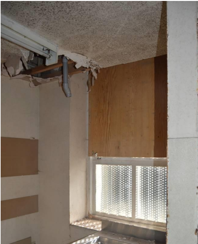
Plate 80.3: Detail in room G12.2. Facing south.
