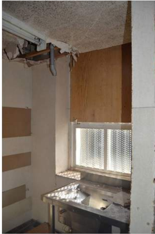
Plate 80.3: Detail in room G12.2.
