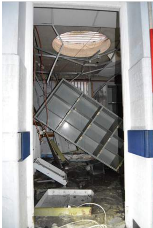
Plate 104.8: Circular skylight to X-ray annex rooms.
