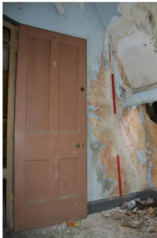
Plate 68.8: View within room S10, with four panel door. Scale 2m.
