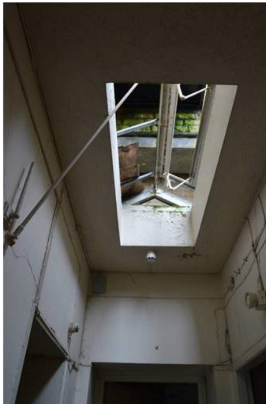
Plate 91.19: Sky light detail of dispensary corridor.
