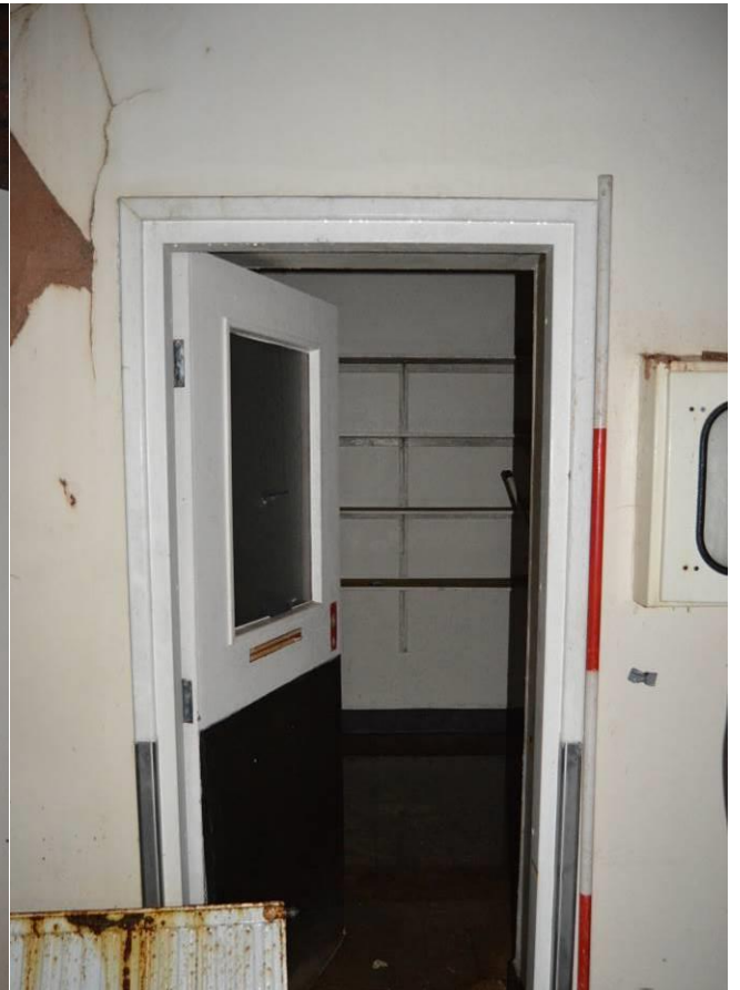
Plate 79.4: Detail into room G11.2. Scale 2m. Facing south east.
