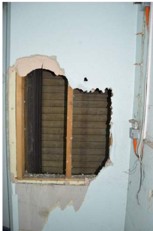
Plate 67.8: Tongue and groove partition behind modern plasterboard.
