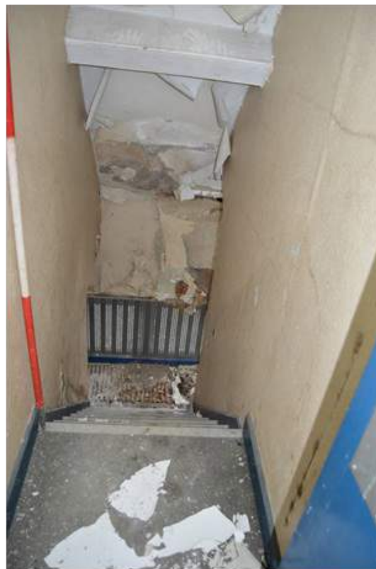
Plate 67: View from the corridor S4 down the stairs. Scale 2m.
