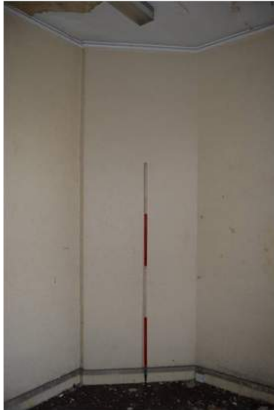
Plate 37.4: View of corner chimney to surgeon's bedroom. Scale 2m.
