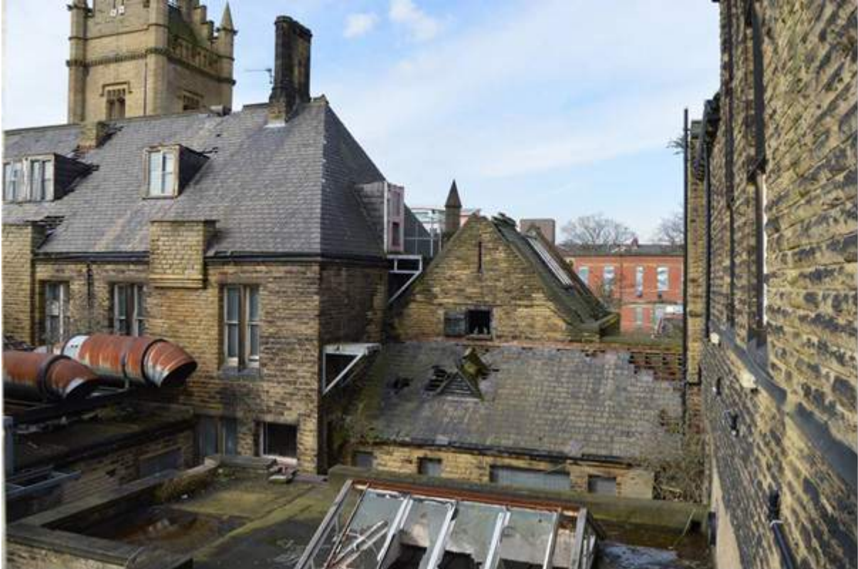
Plate 88: Rear arrangement of the eastern linking range.
