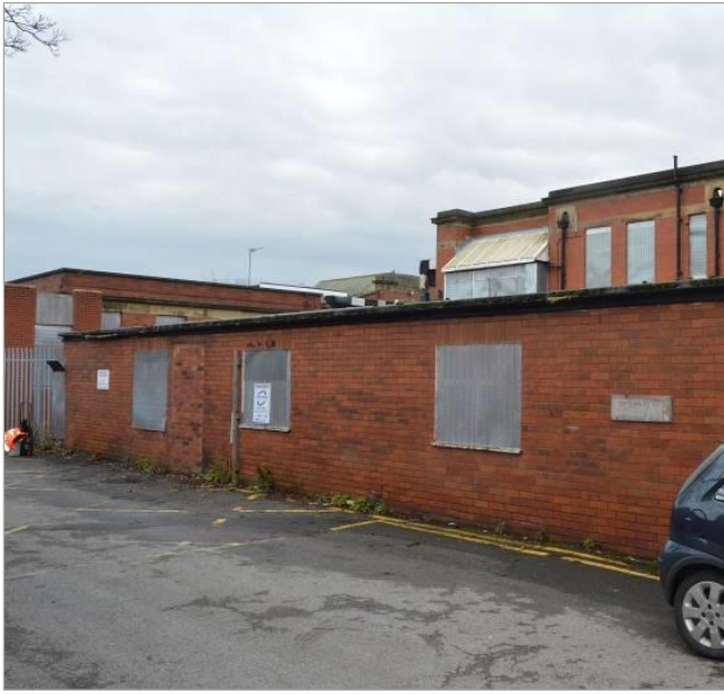
Plate 110.3: Medical stores buildings (facing east).
