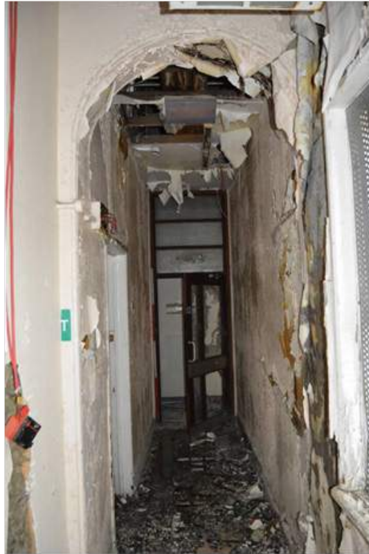
Plate 59.1: View facing north of the lobby. Scale 2m.
