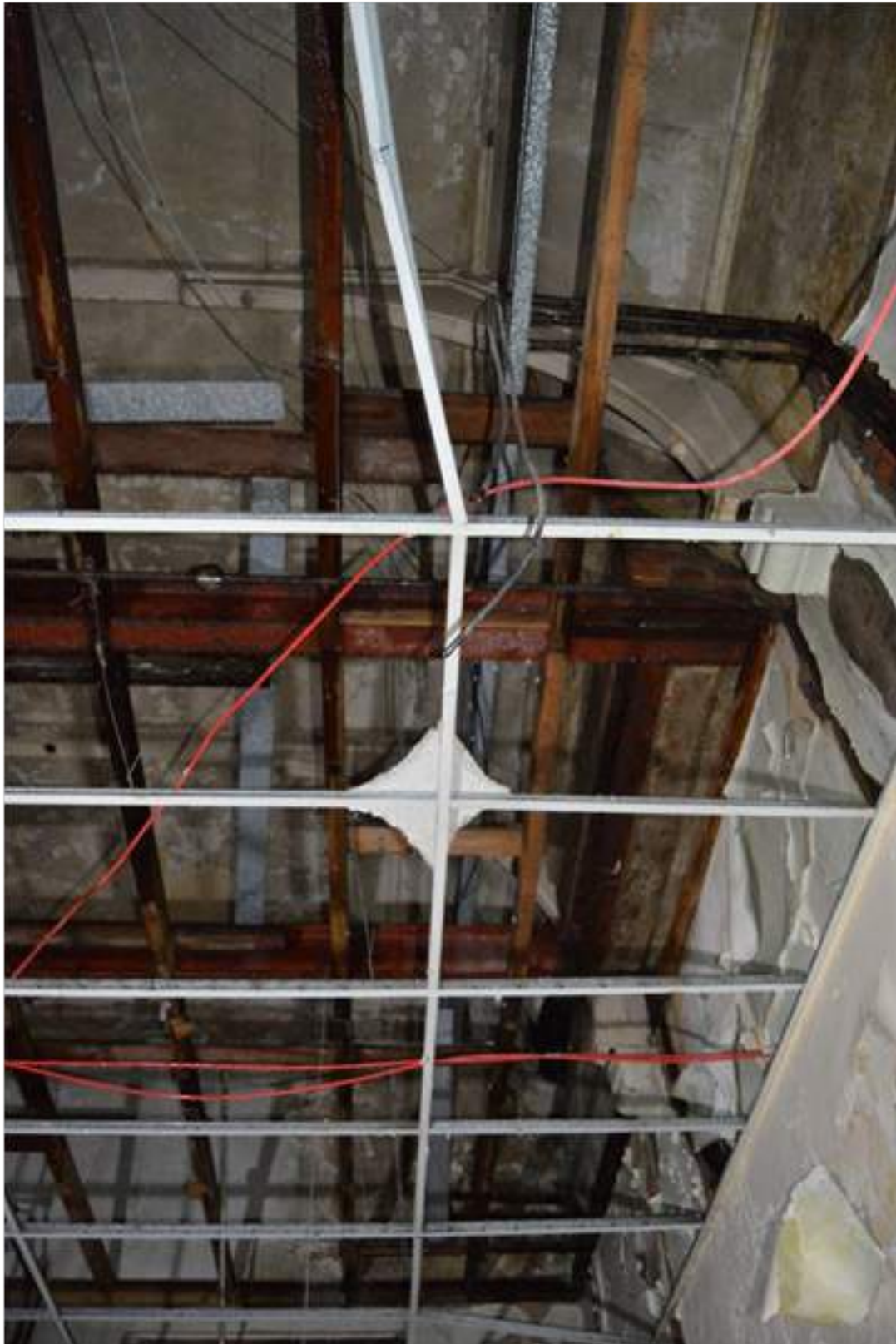
Plate 86.1: View of the board room ornate ceiling with hammer beam details.
