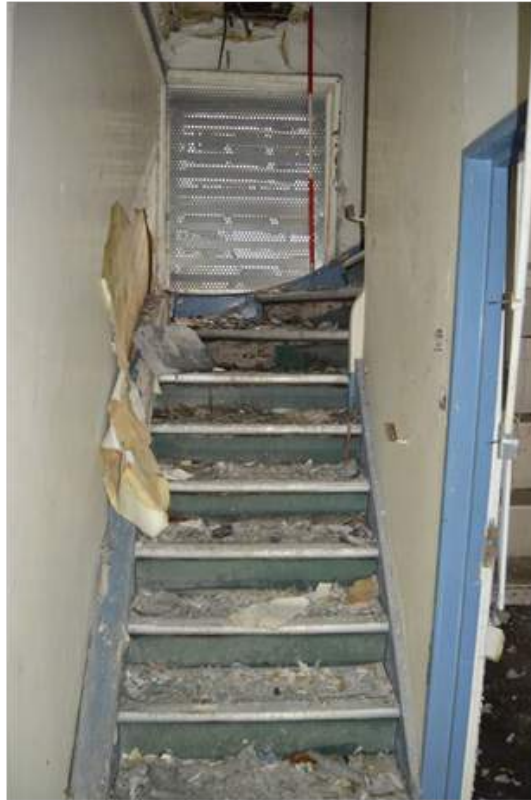
Plate 52.1: Stairs to the west of the nurses' accommodation. Scale 2m.
