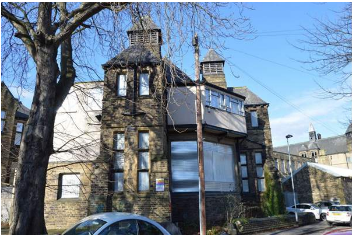
Plate 92: View of the western pavilion south. Scale 2m.
