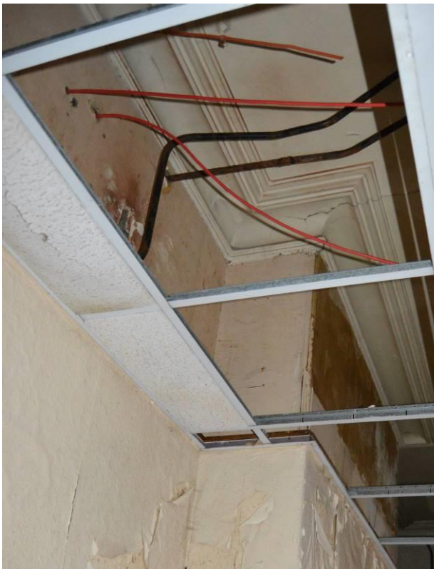
Plate 27.2: Chimney breast and coving. Facing south east.
