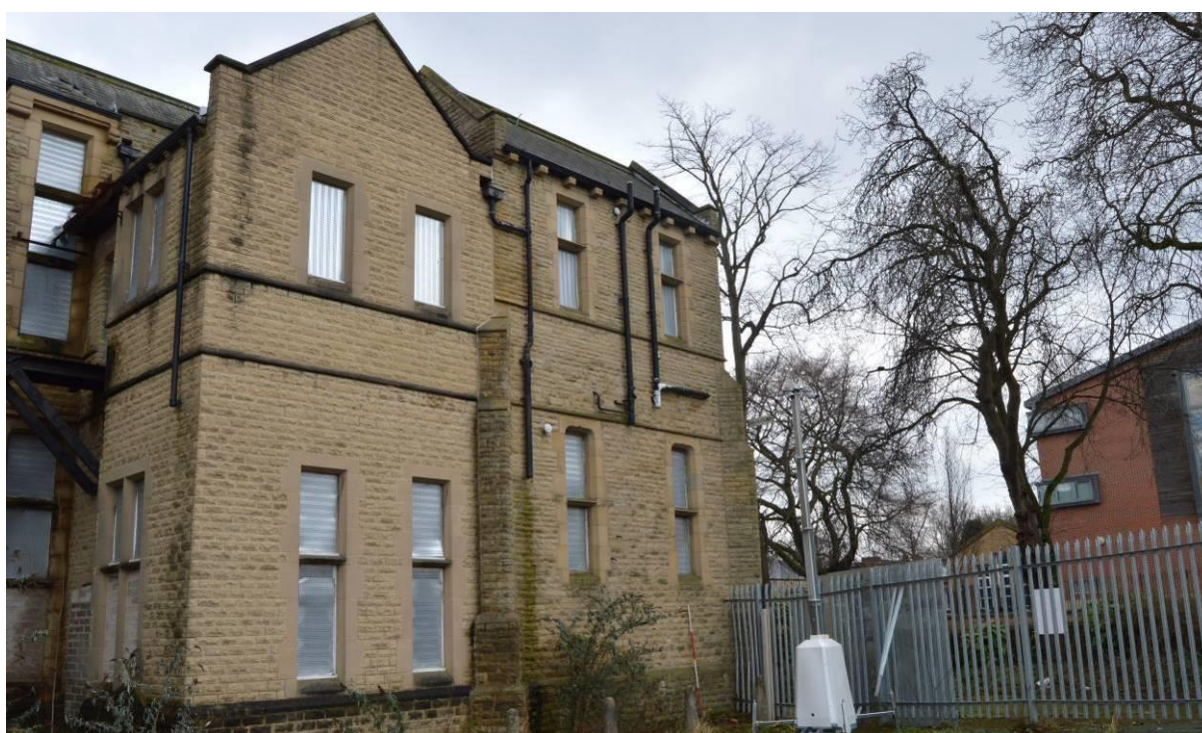
Plate 96.3: Side (north) elevation of the children's ward sanitary wing (facing south). Scale 2m.
