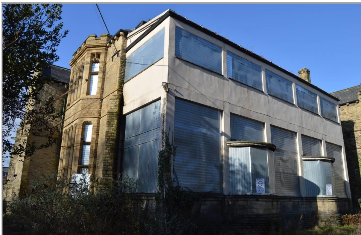
Plate 98: Veranda extension to children's ward, facing north. Scale 2m.
