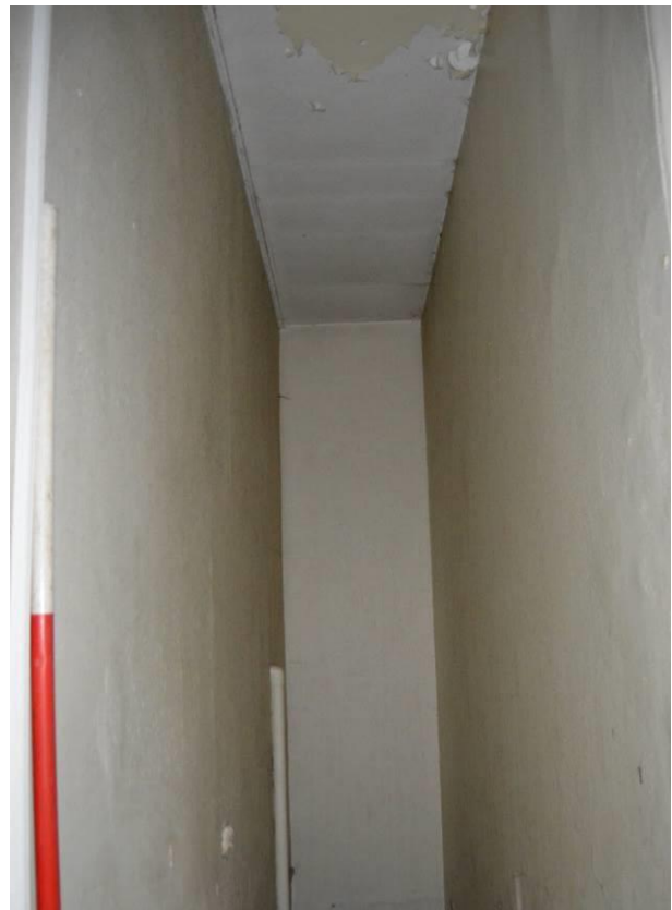
Plate 35.1: Plain ceiling above stair. Scale 2m. Facing south west.
