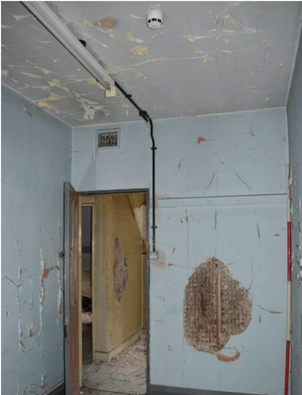
Plate 68.10: View within room S12, note the mesh construction behind the plaster. Scale 2m. Facing north west.
