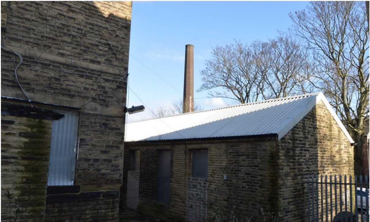
Plate 99.2: North west corner of the laundry range, facing east. Note there is a gable at this end.
