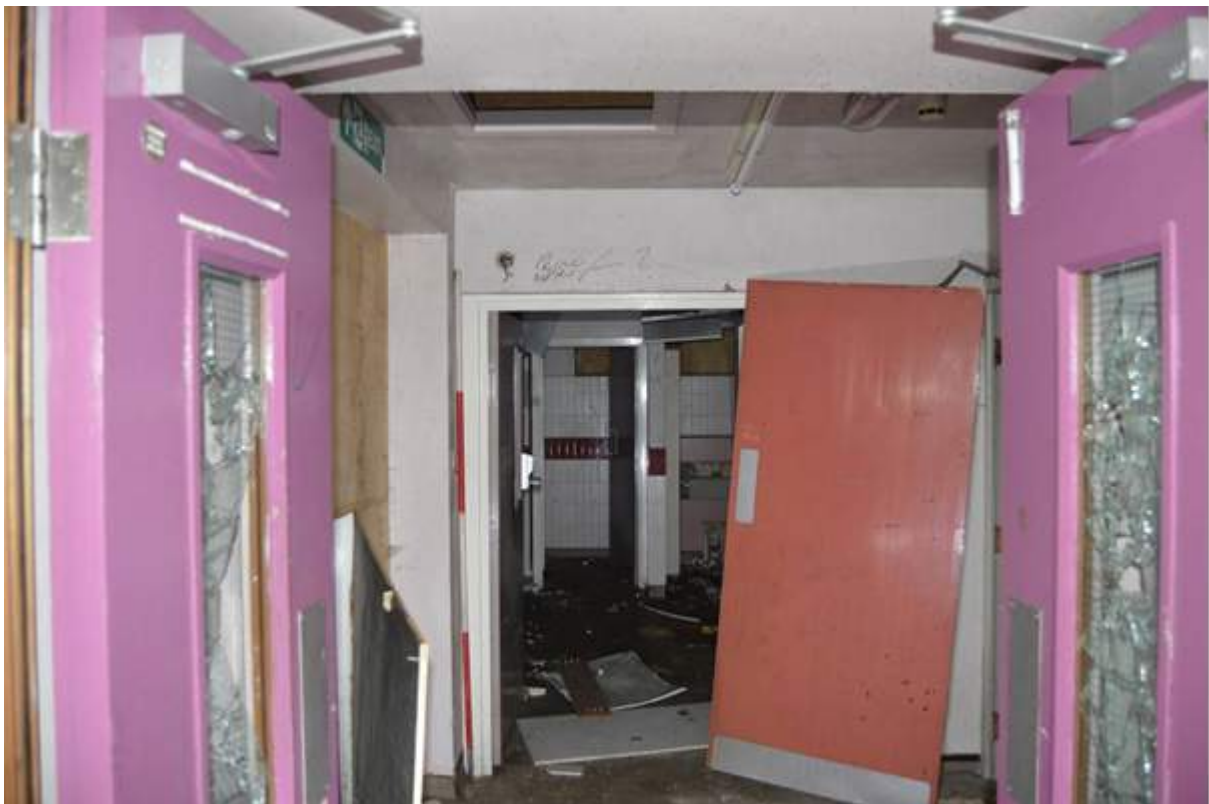
Plate 105.13: The Ann Canning Childs' Building terminated in a later extension to the west. Scale 2m.
