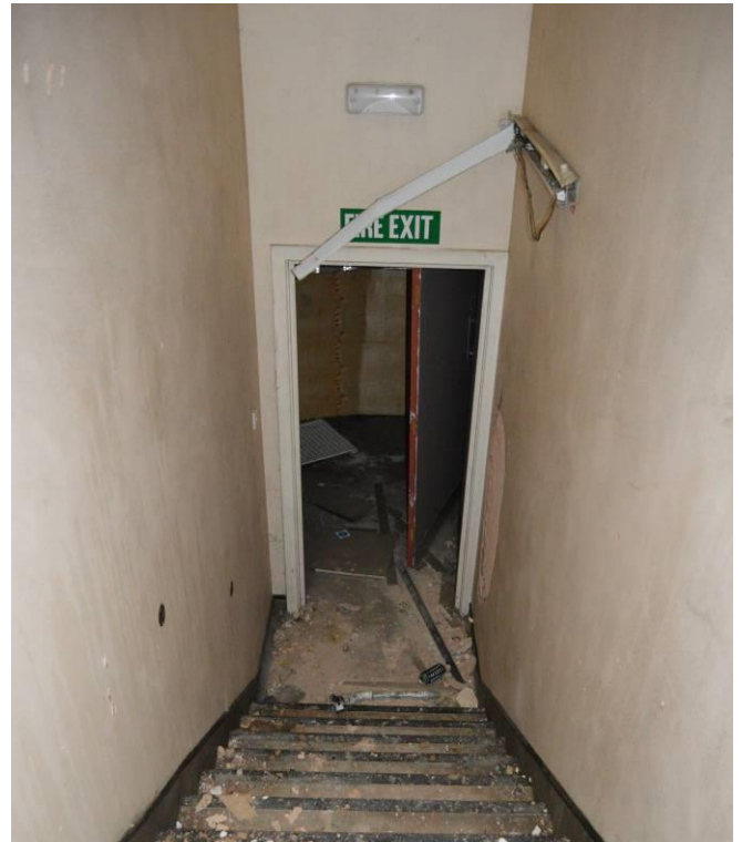
Plate 109.2: Stairs, modern extension with the Canning wards (facing south east).
