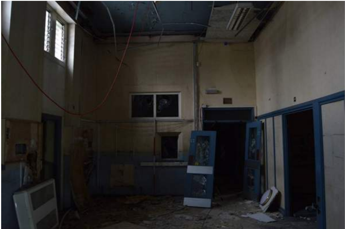
Plate 92.5: Looking back at the ward entry, note the squint style window from the nurse's station (bottom centre). Scale 2m.
