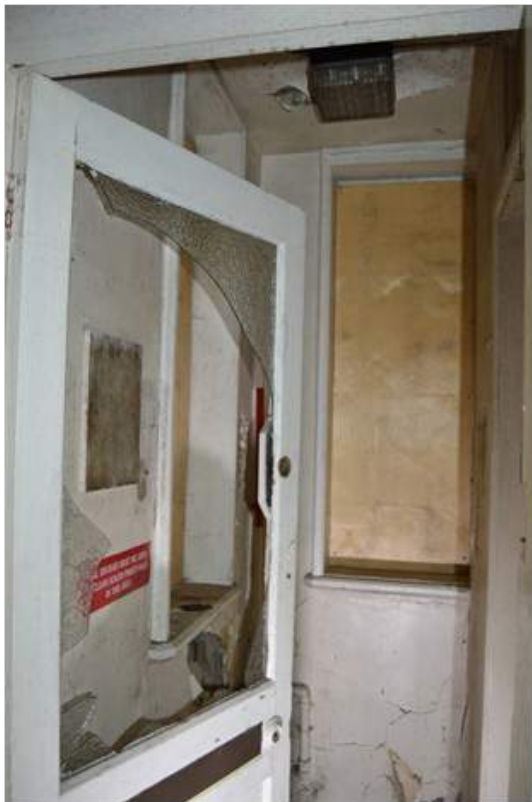
Plate 73.4: Detail of dual aspect windows to W.C..
