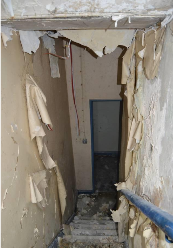
Plate 56.3: Reverse view down the stairs. Facing north west.
