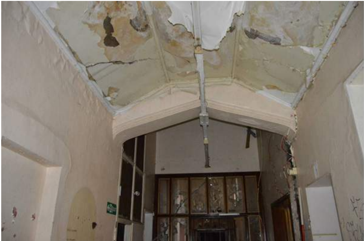
Plate 88.4: Tudor style arch, view facing east in axial corridor.
