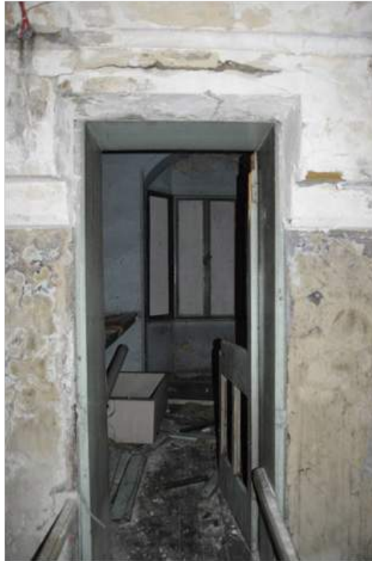
Plate 63: View into second floor tower room. Note the corbelled plasterwork at the door head.
