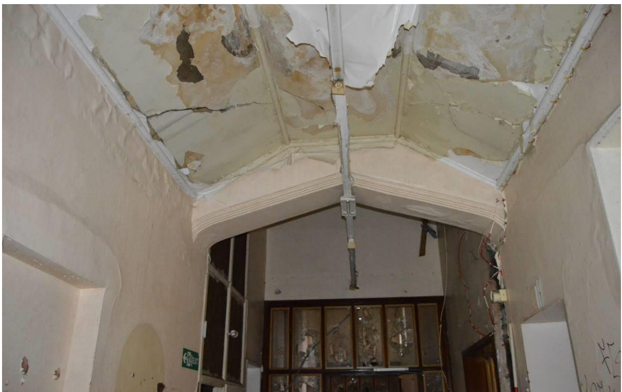
Plate 88.4: Tudor style arch, view facing east in axial corridor.
