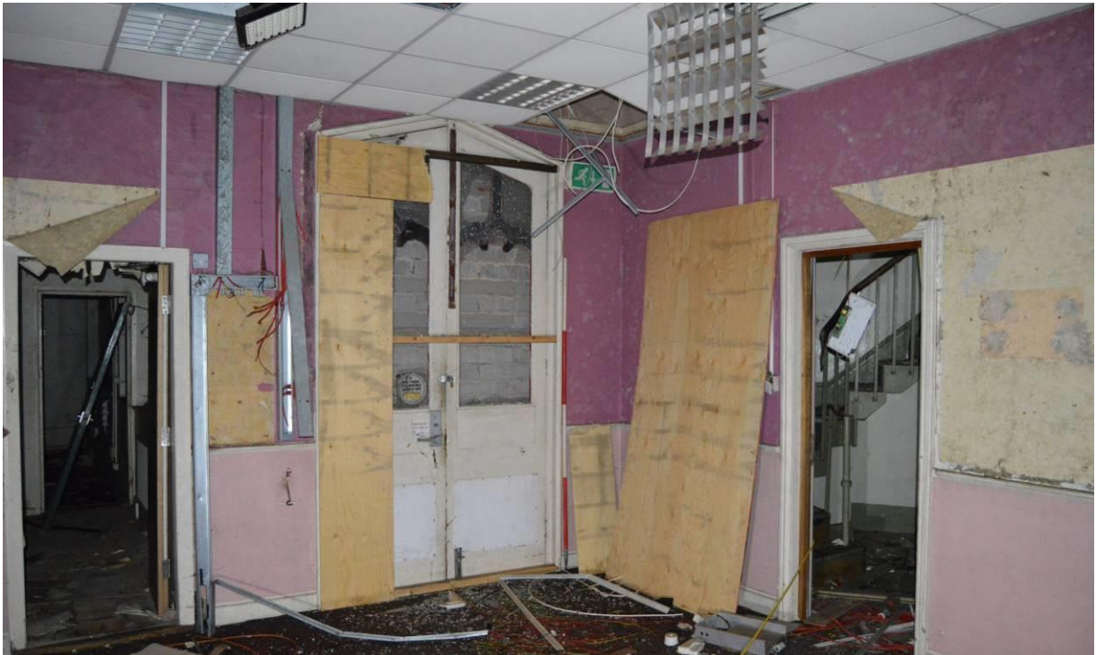
Plate 101.2: Entrance hall of the Nurses' home, facing north. Scale 2m.
