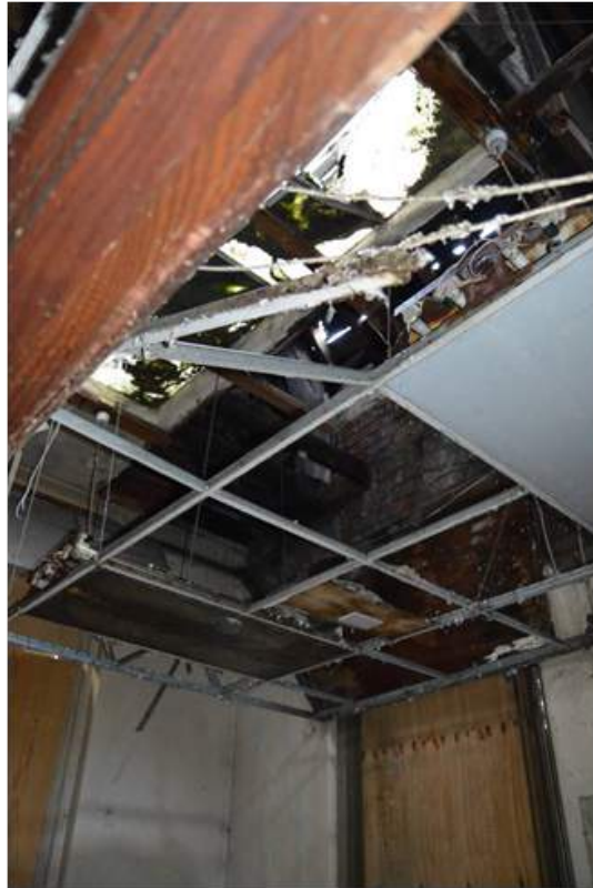
Plate 89.2: Hammer beam above operating theatre.
