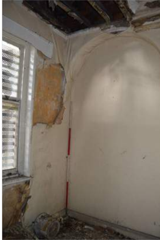
Plate 37.2: Arched recess for shelving and section of window in asst. surgeon's bedroom. Scale 2m.
