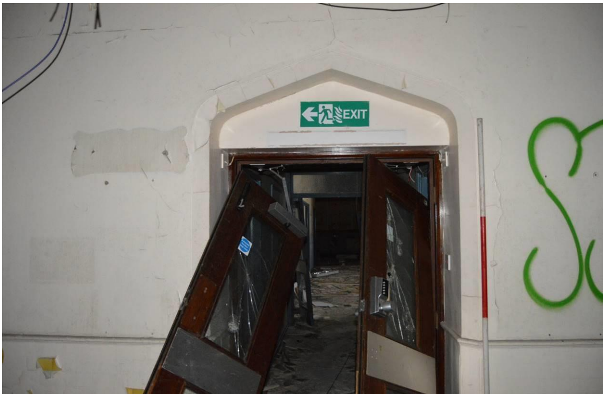
Plate 92.1: Tudor arch entrance retained to west pavilion ward, ground floor (facing south east). Scale 2m.
