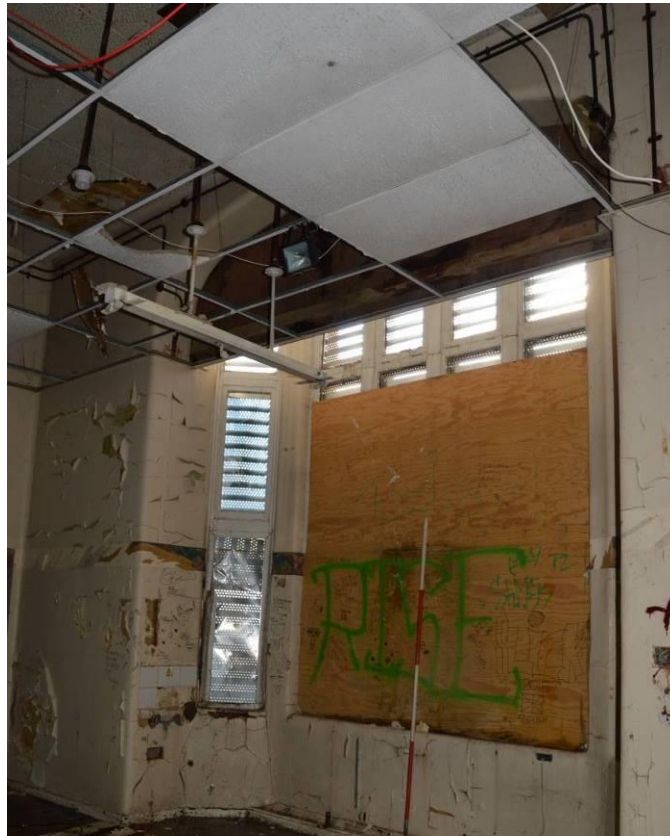
Plate 97.3: Ground floor, bay window to children's ward (facing south). Scale 2m.
