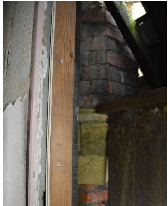
Plate 67.11: Stone corbel below the north east corner turret. Facing west.
