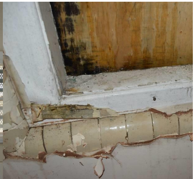
Plate 79.2: Detail to tiling in G11.6. Facing north east.
