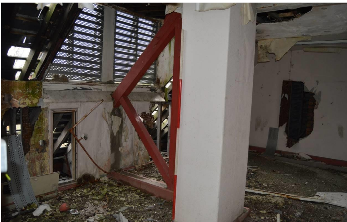
Plate 66: View facing south east in room S3. Scale 2m. Facing south.
