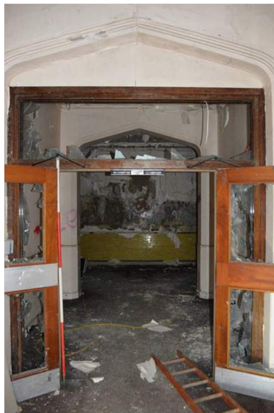
Plate 19: Internal arches in the visitor's hall. Note later insertion of glazed doors. Scale 2m.
