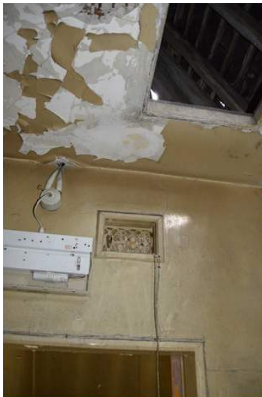
Plate 68.2: Vents above the doors to the rooms of the second floor accommodation.
