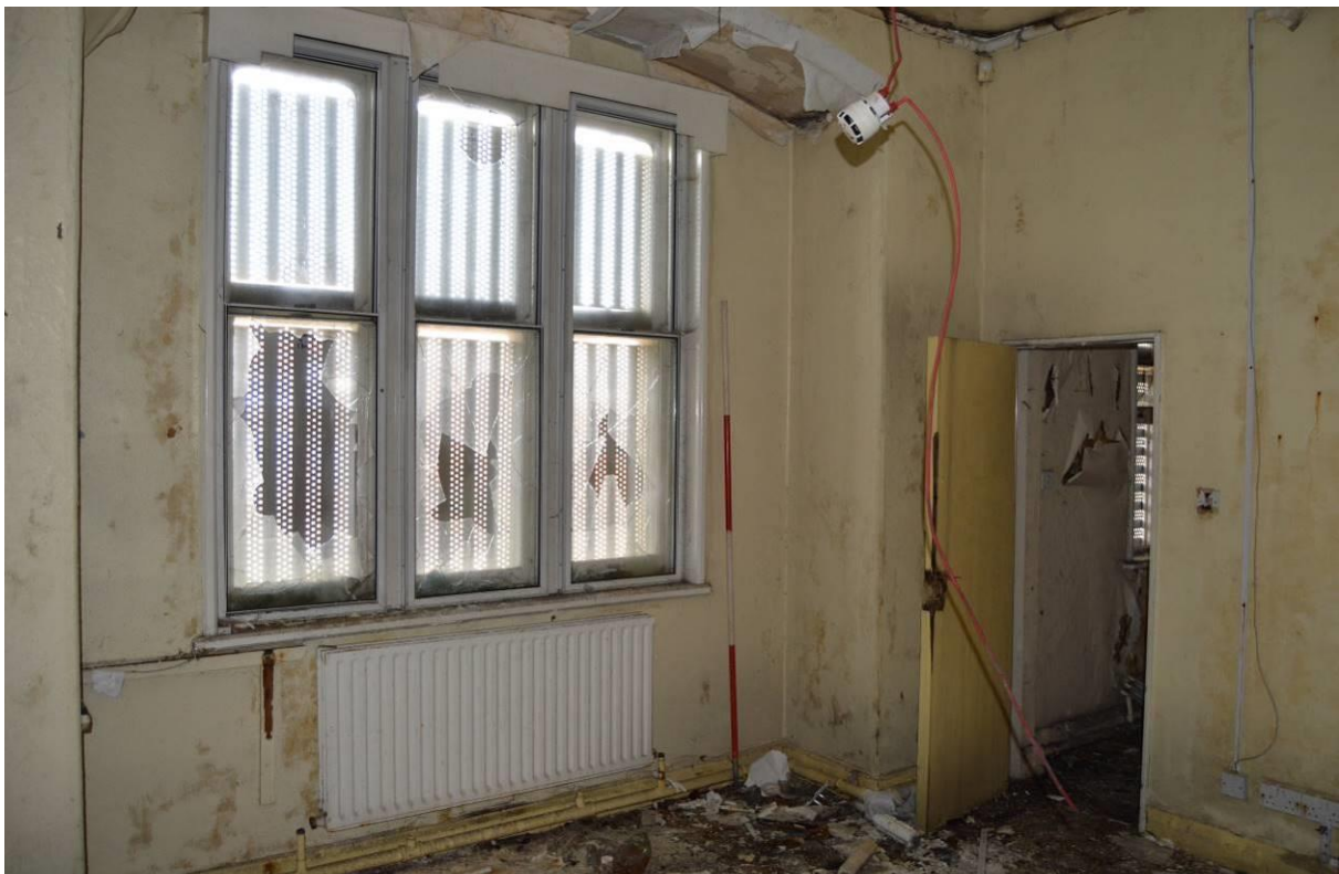
Plate 49.1: Matron's bedroom. Note later door inserted. Scale 2m. Facing north.
