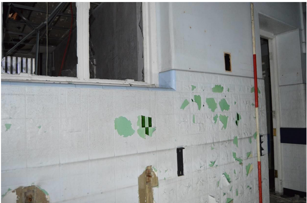
Plate 104.6: Tiled wall finish to X-Ray wing corridor, facing south. Scale 2m.
