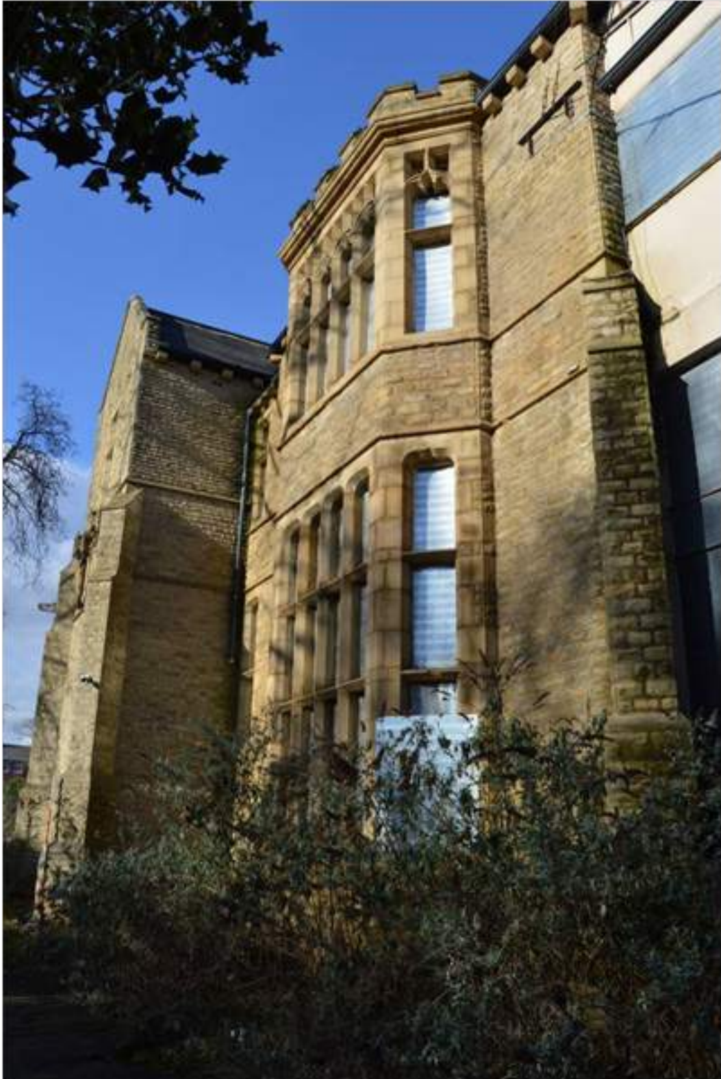
Plate 96.1: View of the children's wards east elevation from the south-west.
