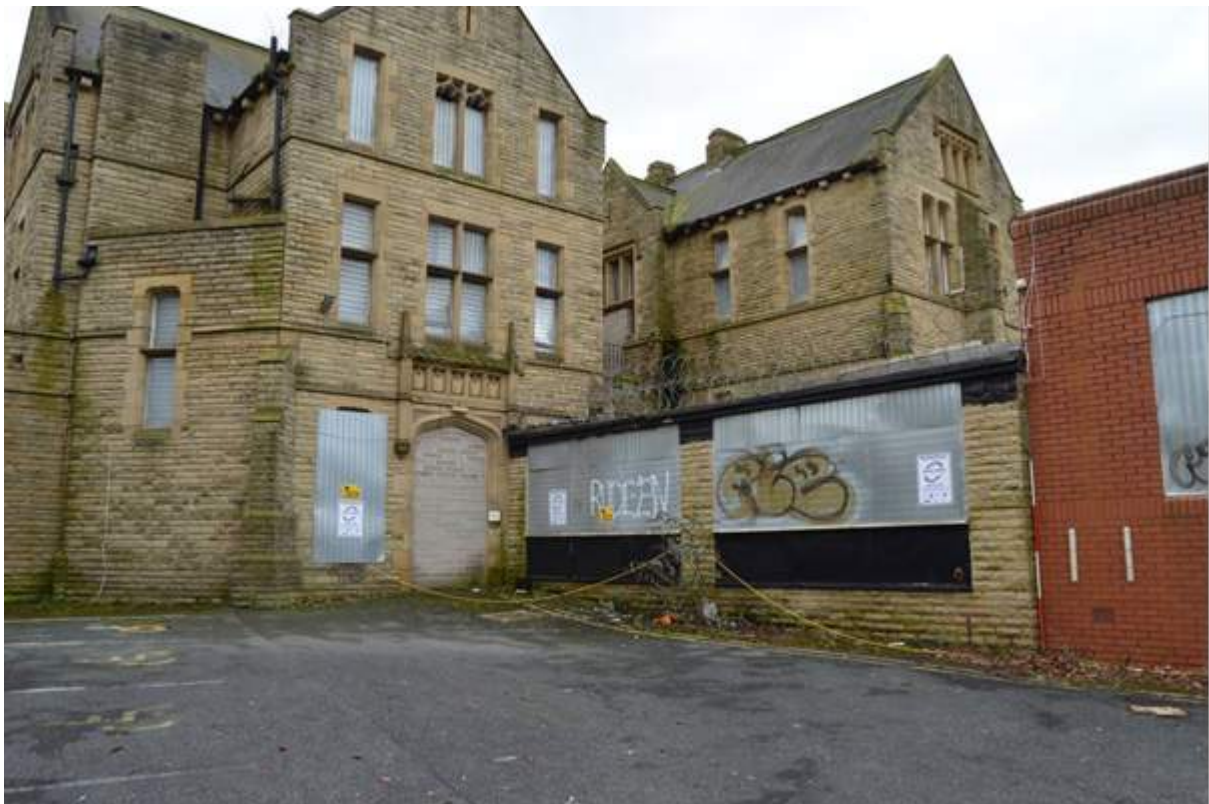
Plate 100: The Nurses' home extension to the east of the original hospital building. Scale 2m.
