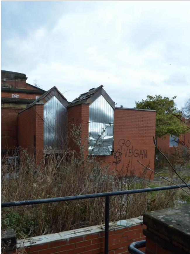
Plate 110.1: Chapel of Rest building (facing east).
