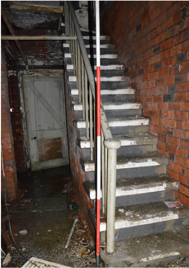
Plate 70.1: Stairs to basement. Scale 2m. Facing south west.
