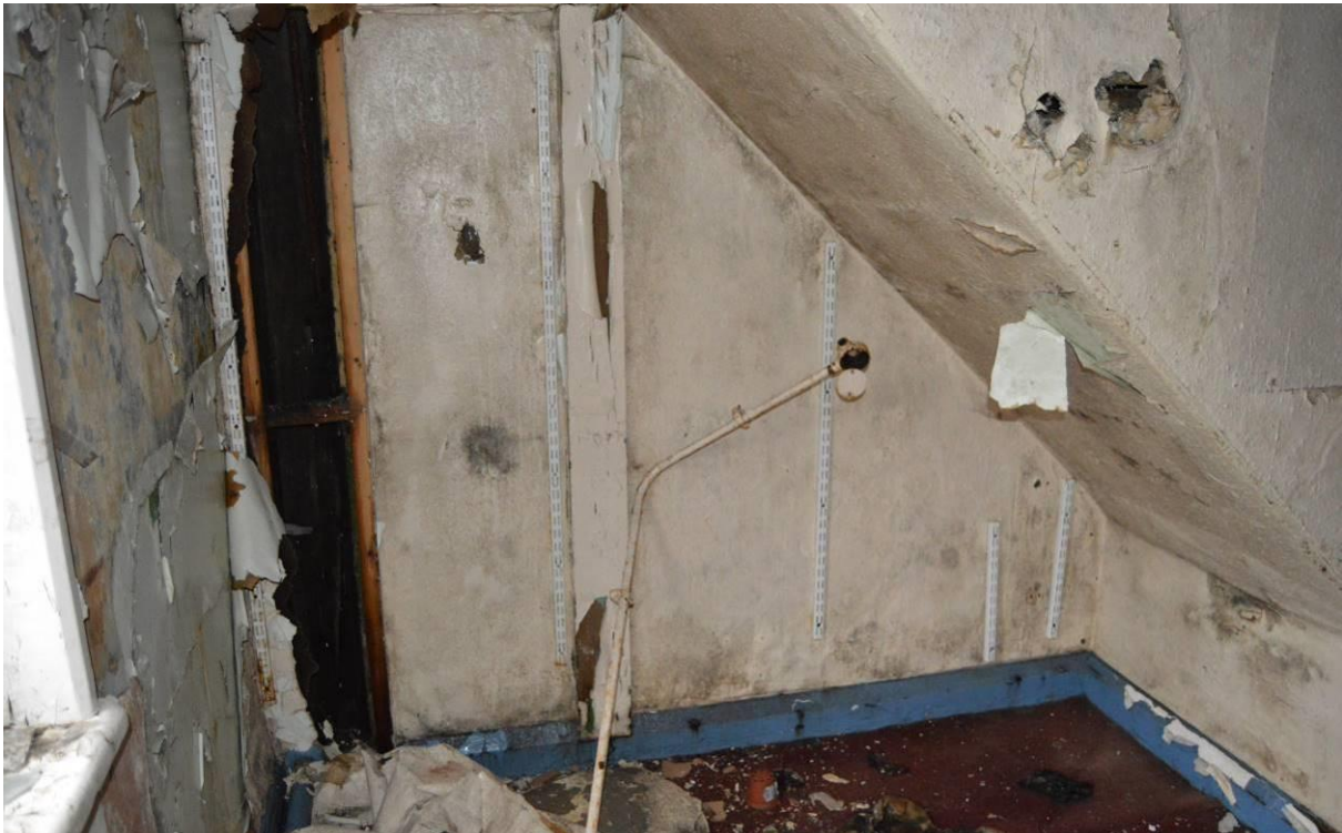
Plate 55.3: View beneath the stairs in room F13. Facing south west.
