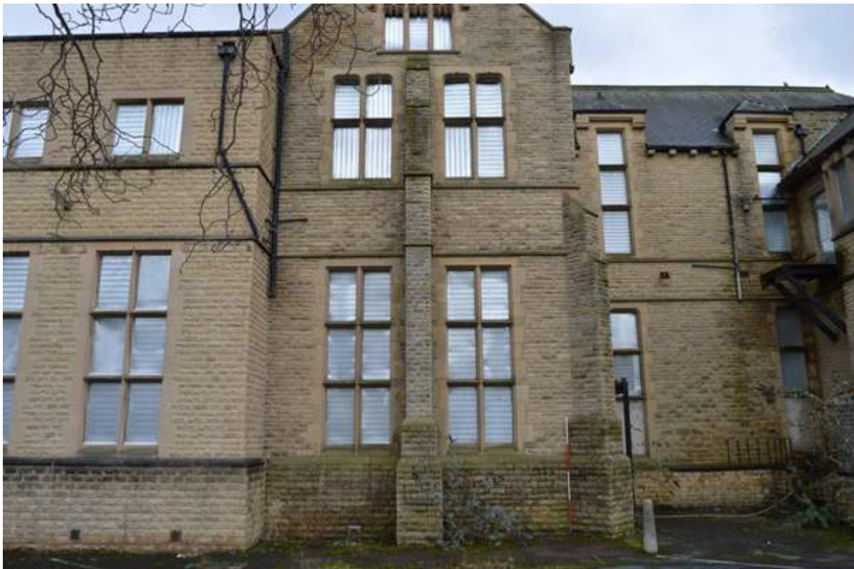
Plate 94: North facing elevation of the special ward. Scale 2m.
