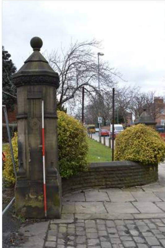
Plate 109.7: East gate, side of north gate post. Scale 2m.
