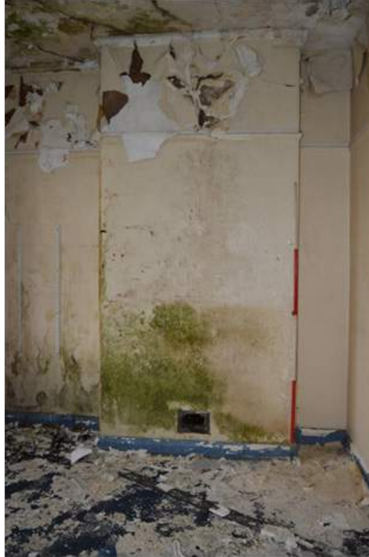
Plate 43.2: Chimney in room F6. Scale 2m.
