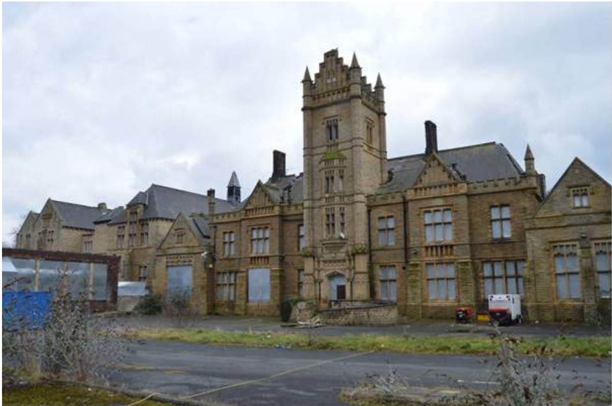
Plate 1: Oblique view of the administration range from the north. Scale 2m.
