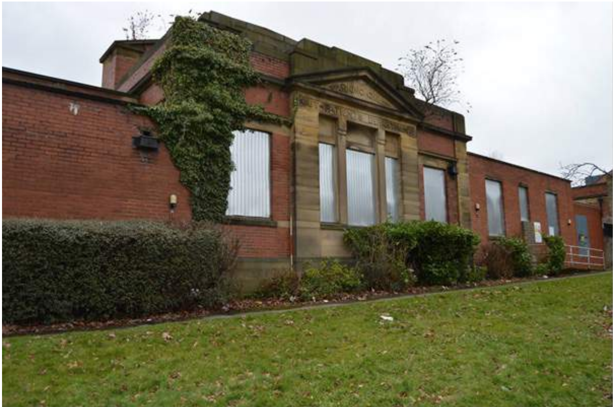
Plate 102: East façade to Out-patients' Department. Scale 2m.
