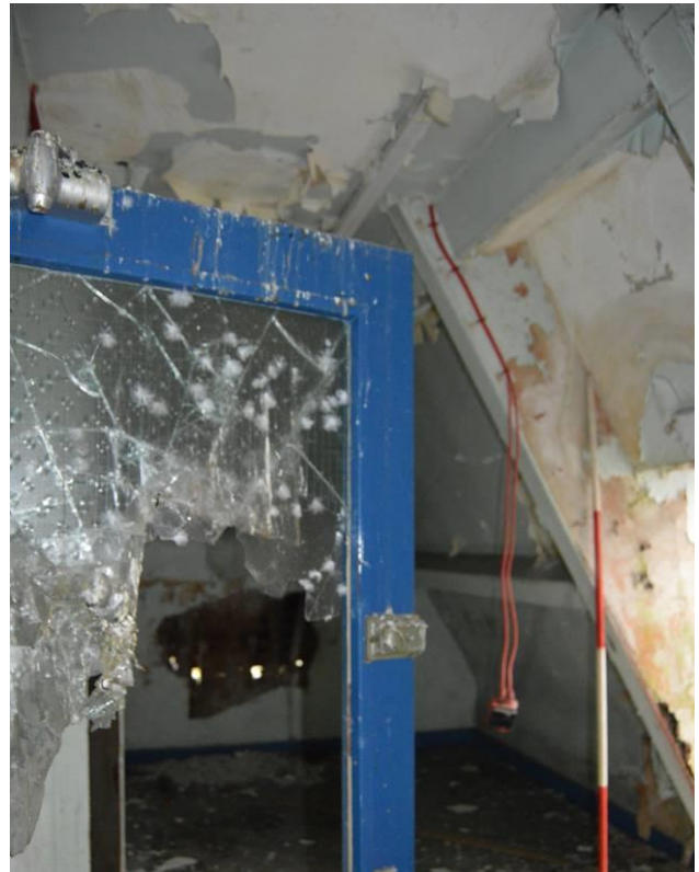
Plate 67.9: View through door into room S8. Scale 2m. Facing north.
