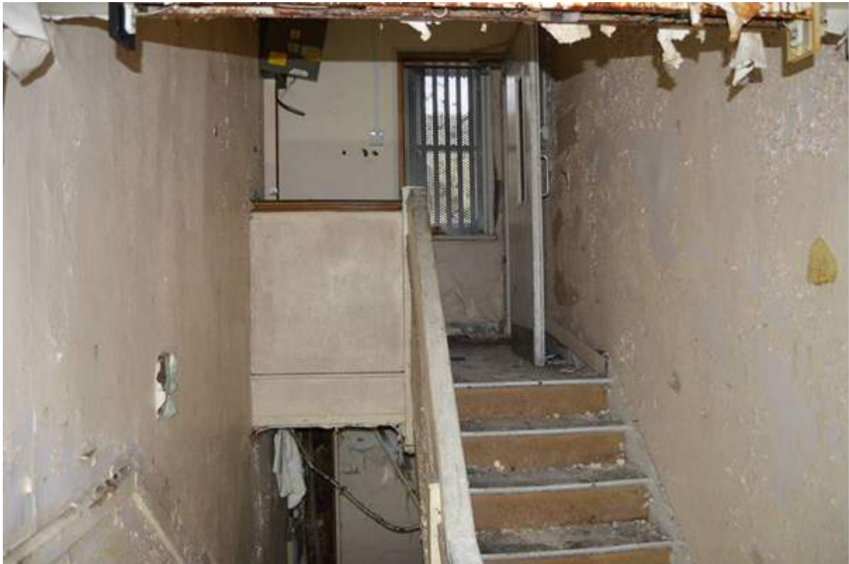
Plate 81: View of the service range staff stairwell/landing.
