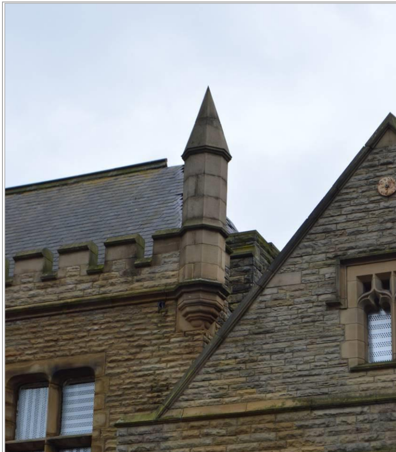
Plate 14: Decorative tourelle to corner of administrative eastern range. Facing east.
