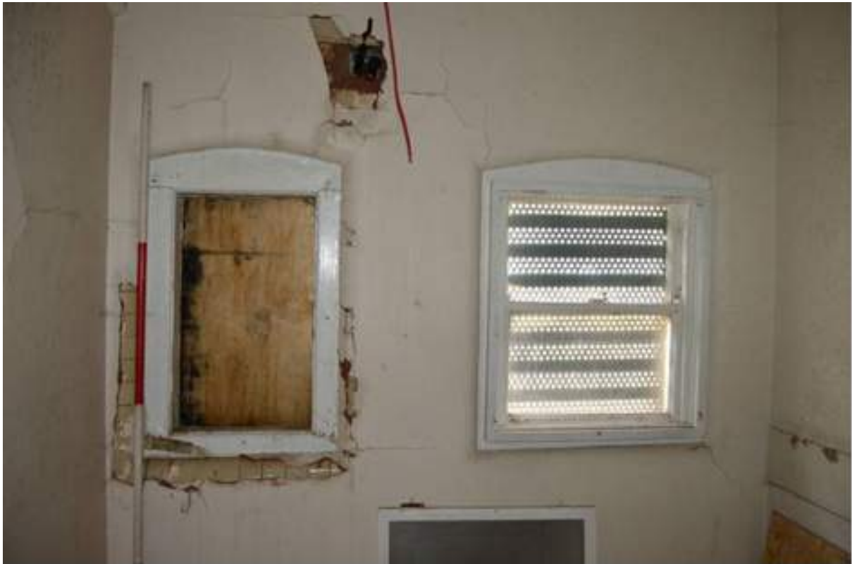
Plate 79.1: Detail of windows to G11.6. Scale 2m.
