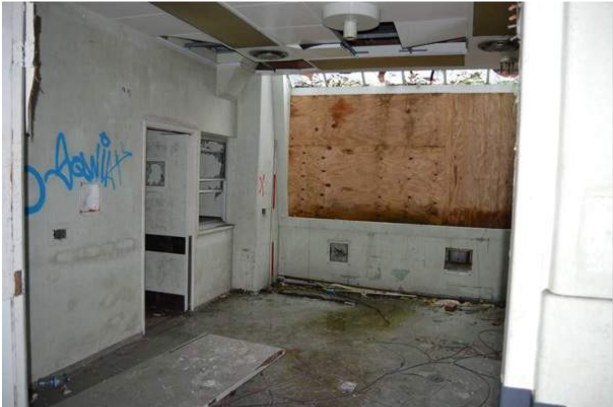
Plate 105.4: Operating theatre. Scale 2m.
