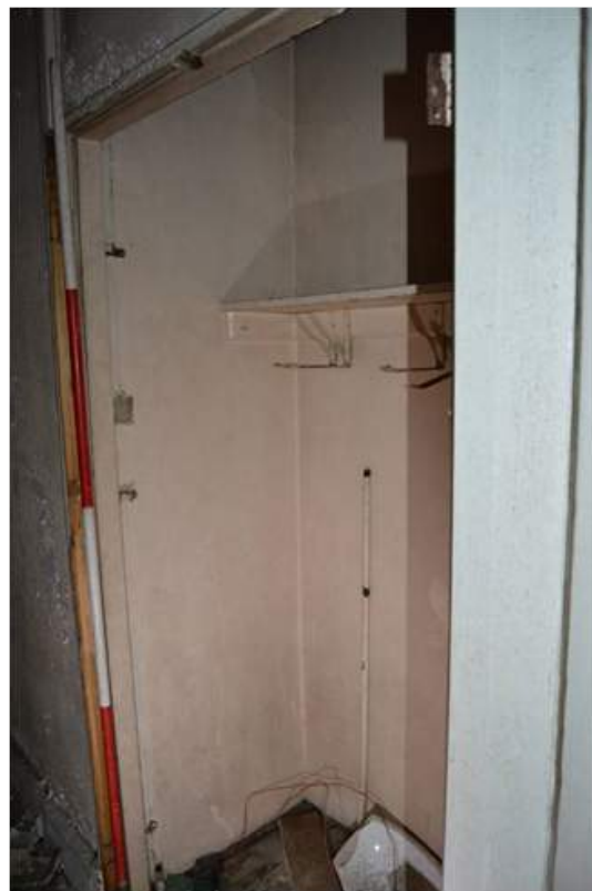
Plate 73.6: View inside the coat cupboard. Scale 2m.
