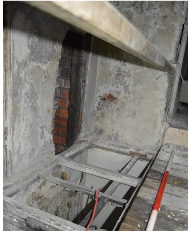
Plate 61.2: View above the landing F1. Scale 2m. Facing north west.
