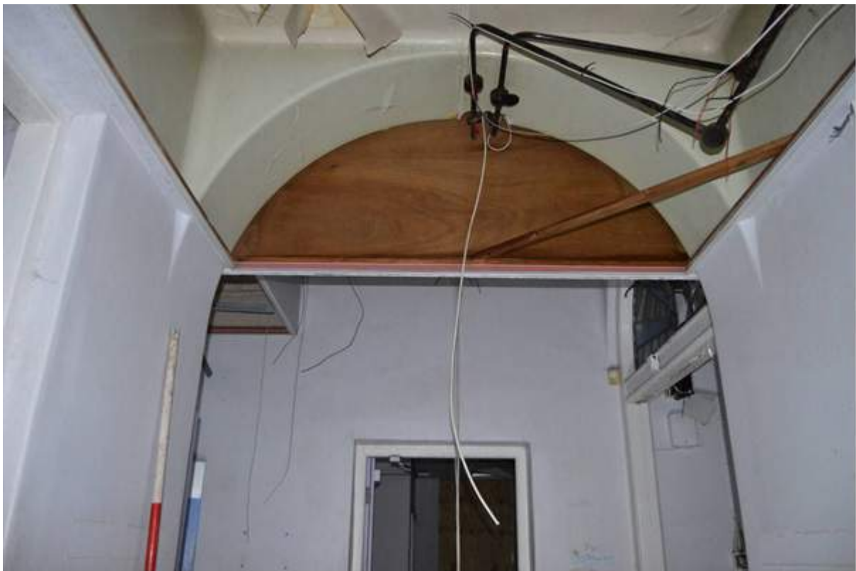
Plate 104.4: Archway at corridor junction in X-Ray wing.
