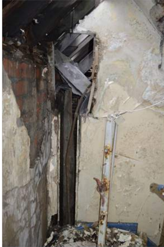
Plate 56.4: Corner of half-landing.
