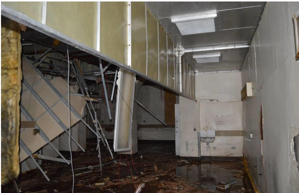
Plate 77: View of the modernised kitchen area. Facing south west.
