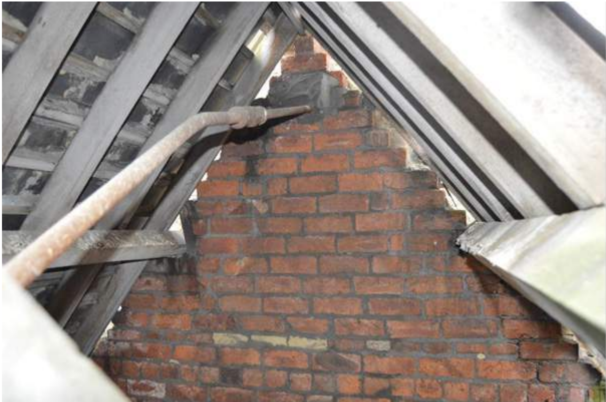
Plate 69.5: Brick construction behind the gable of the projection bay to front.
