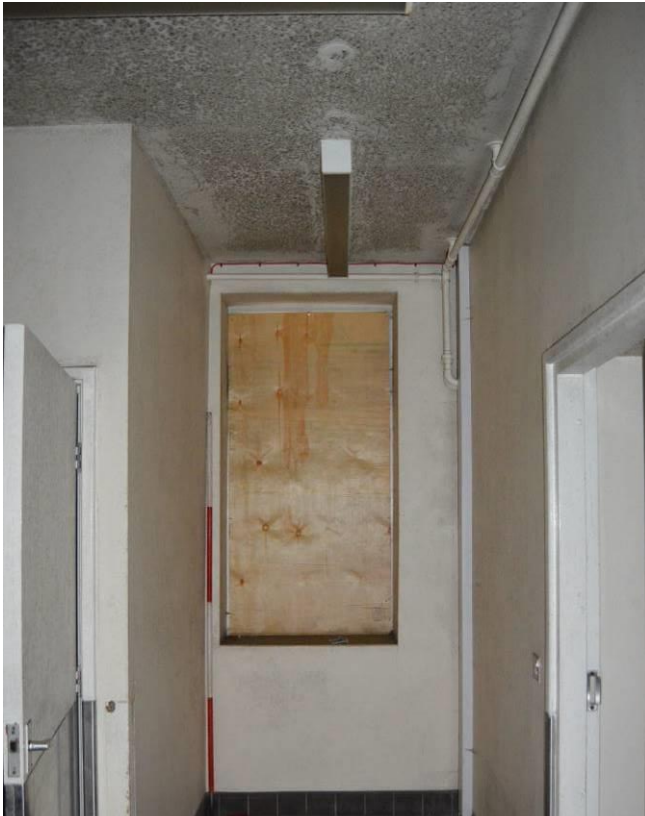
Plate 80.1: Detail in room G12 facing east. Scale 2m. Facing east.
