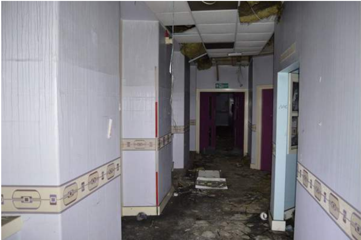
Plate 105.10: The Ann Canning Childs' Building in the part which was originally an open ward. Note the thick embrasures in the right belonging to the original window openings. Scale 2m.
