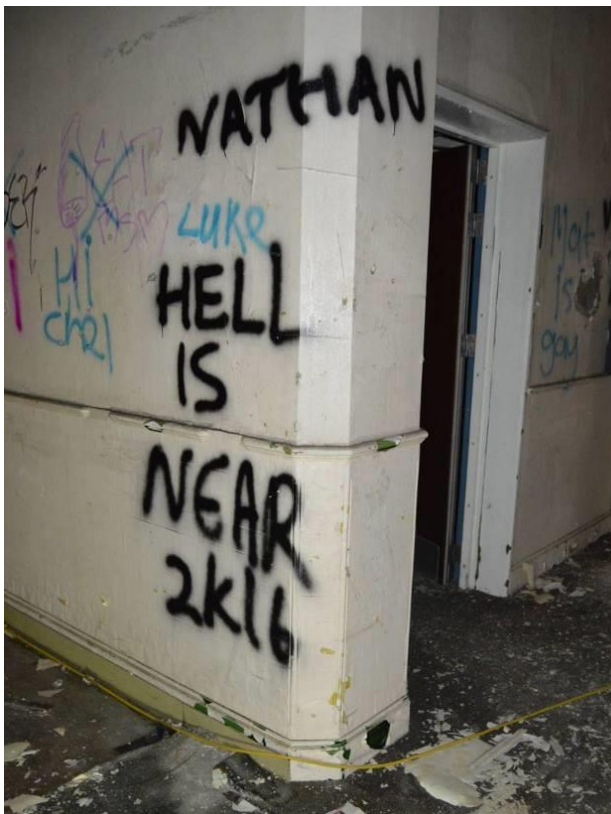
Plate 19.5: Chamfered edge detail to juncture with axial corridor. Facing north.
