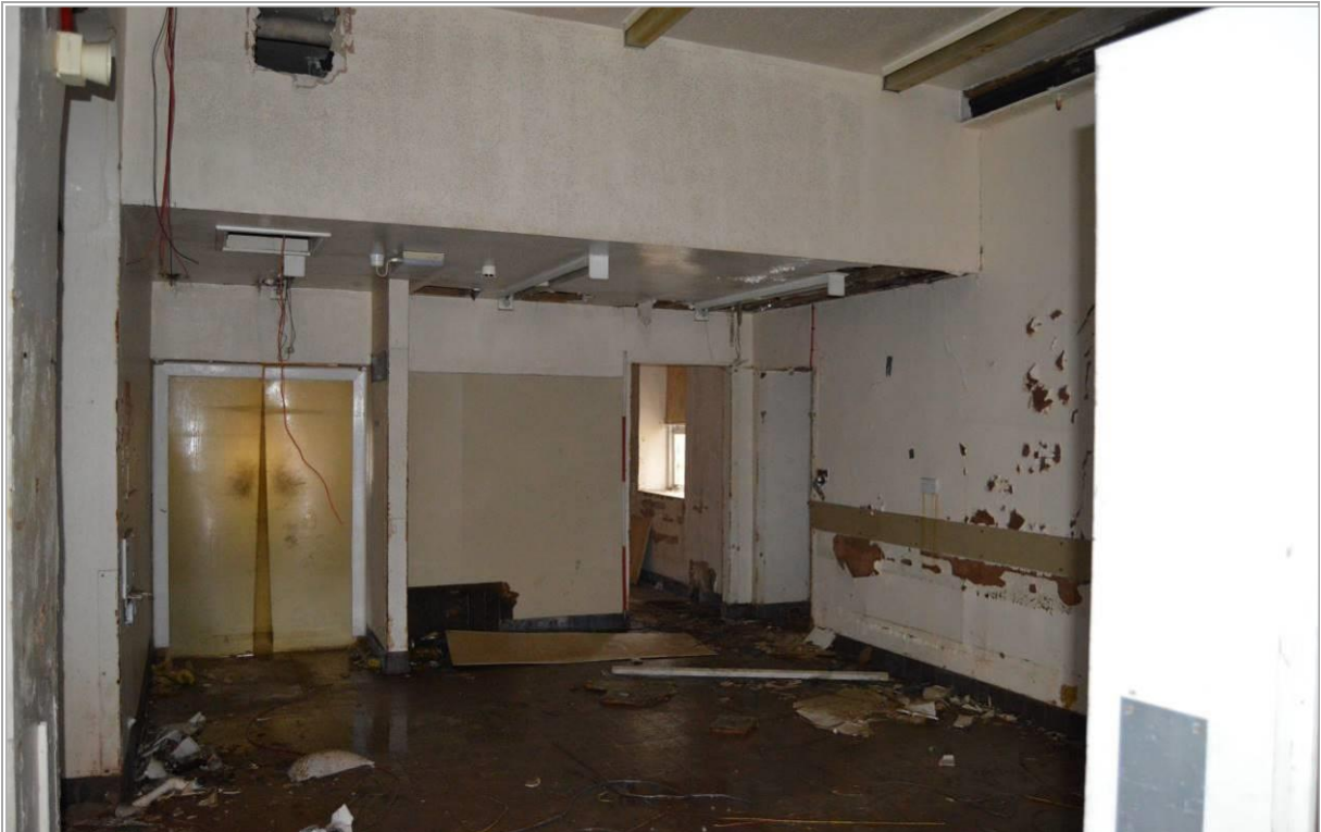
Plate 75: View of the modern kitchen area in the service range, the location of the staff dining room originally. The lowered ceiling is not a structural element, most probably housing modern services and equipment. Scale 2m. Facing south east.
