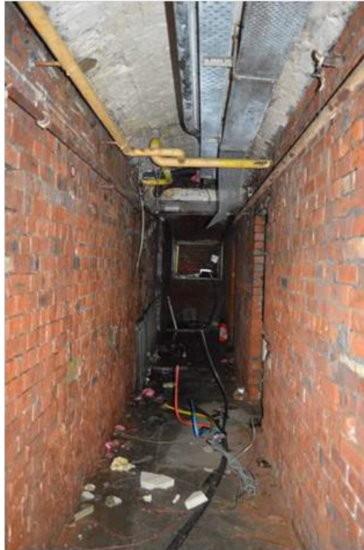
Plate 70.2: Corridor in the basement.
