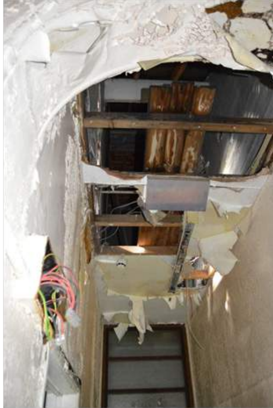
Plate 59.3: View through the later ceiling of the lobby.
