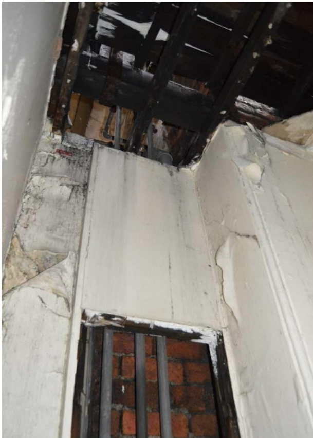
Plate 42.1: View of remaining plaster finish. Facing west.
