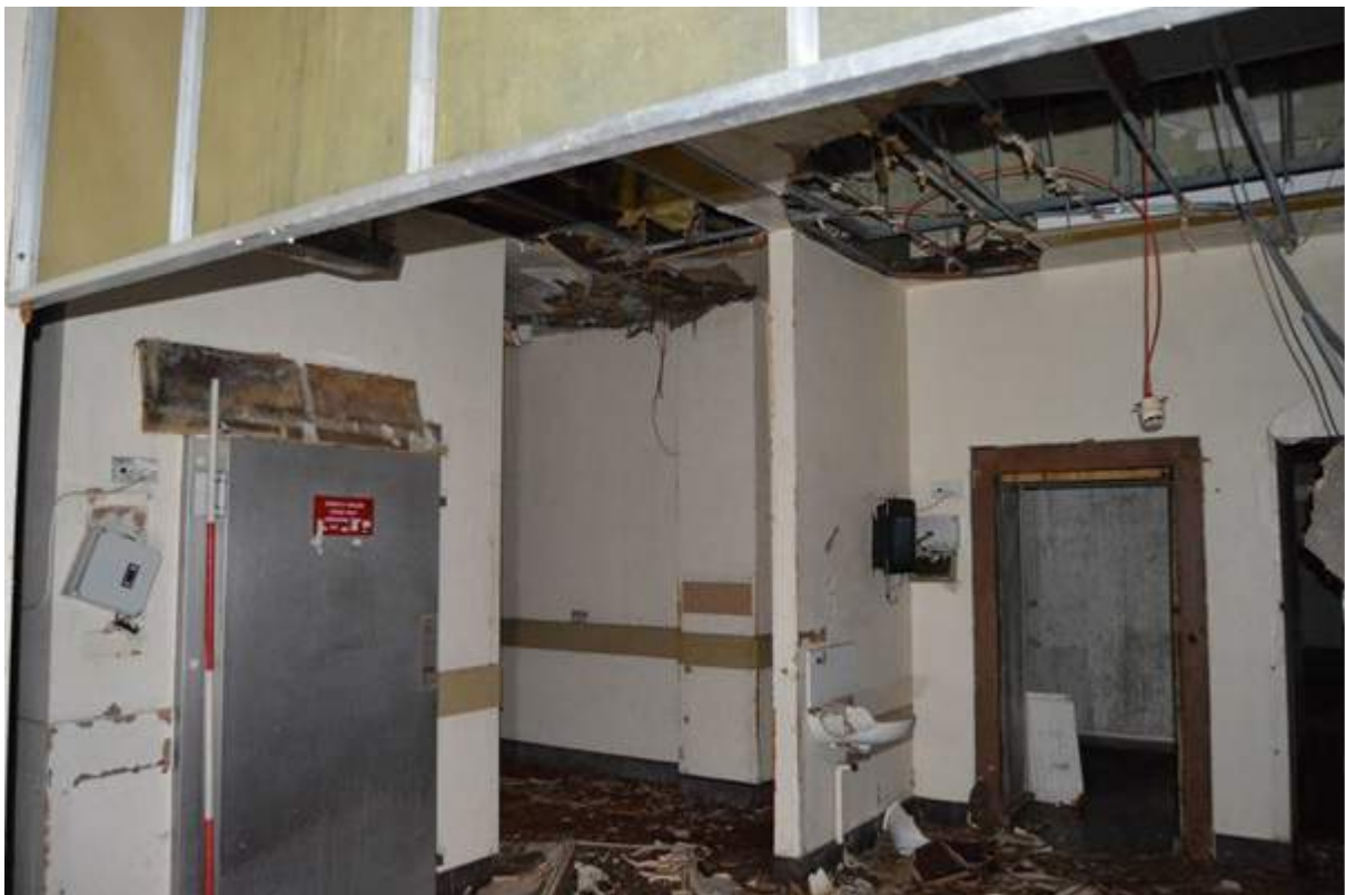
Plate 78: View towards the south back wall of the kitchen. Scale 2m.
