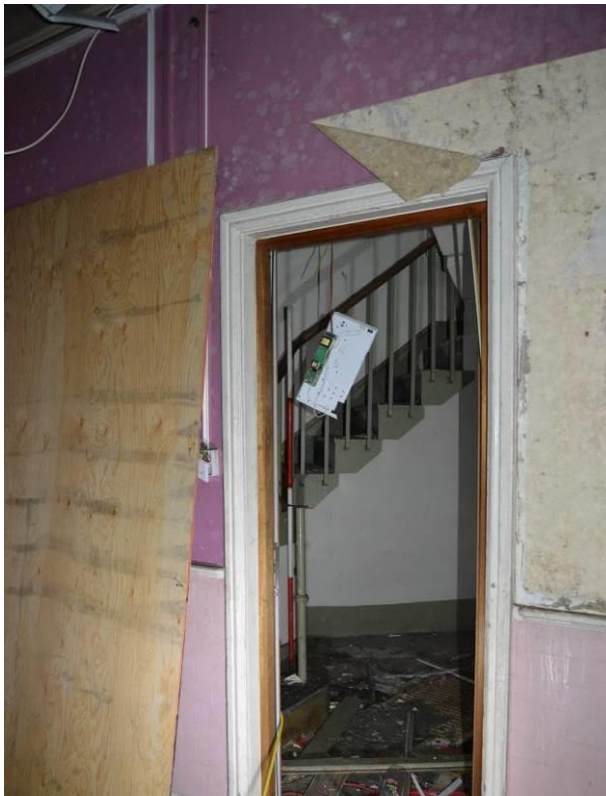
Plate 101.3: View from nurses' home hall to side stairs (facing north east).
