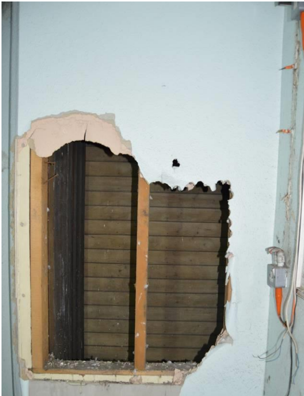
Plate 67.8: Tongue and groove partition behind modern plasterboard. Facing north west.
