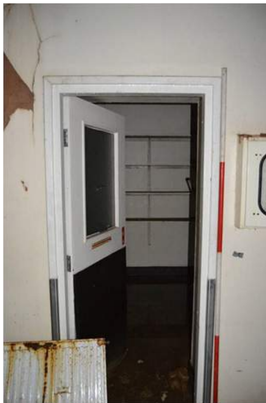
Plate 79.4: Detail into room G11.2. Scale 2m.
