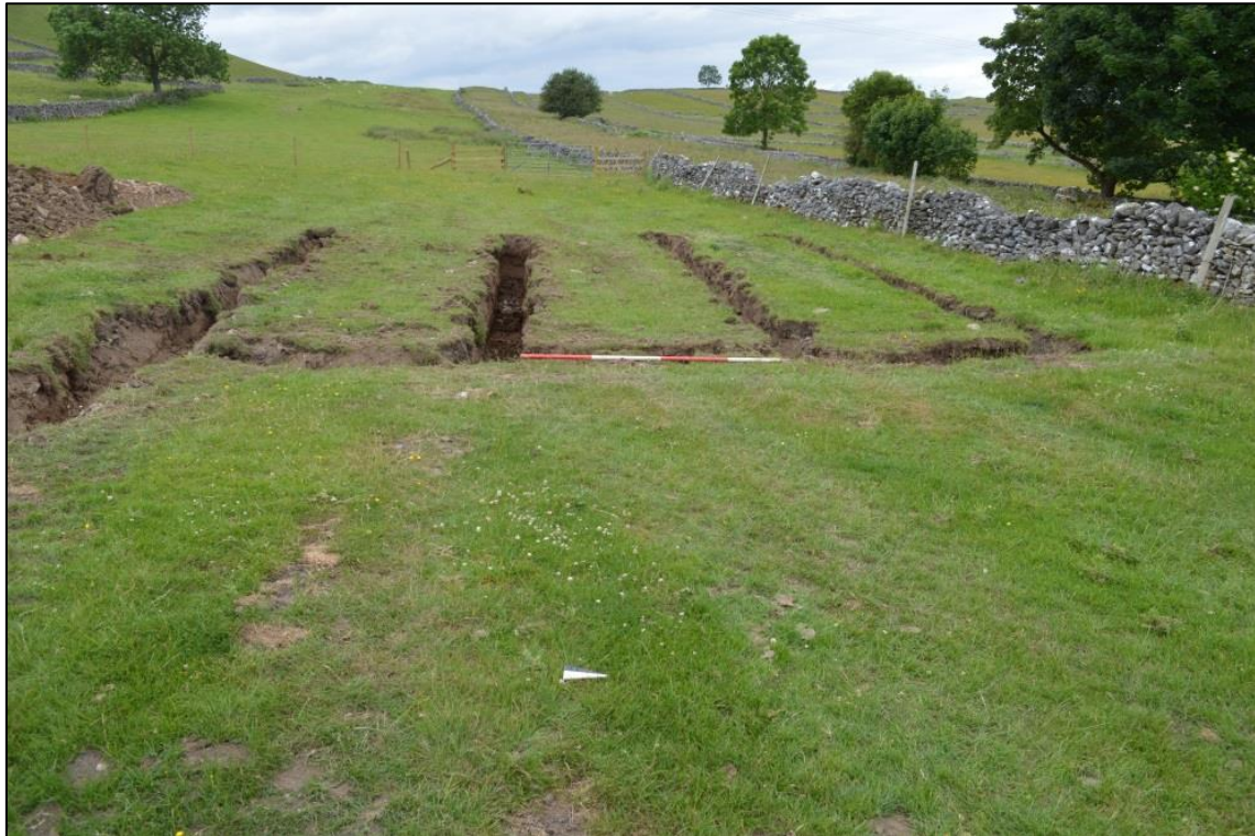
Figure 19: East view of drainage system (scale = 2m).
