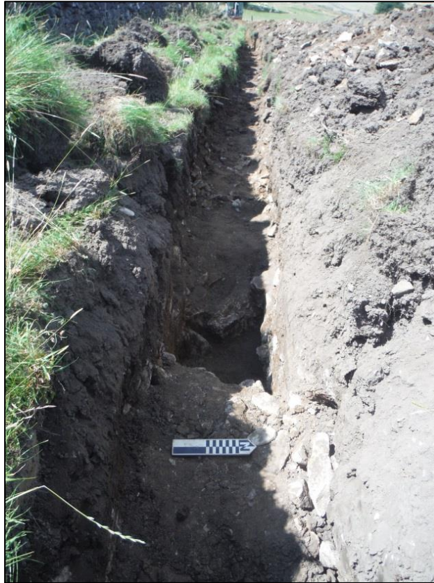
Figure 20: East view of electrical cable trench including rake [023] (scale = 0.25m).
