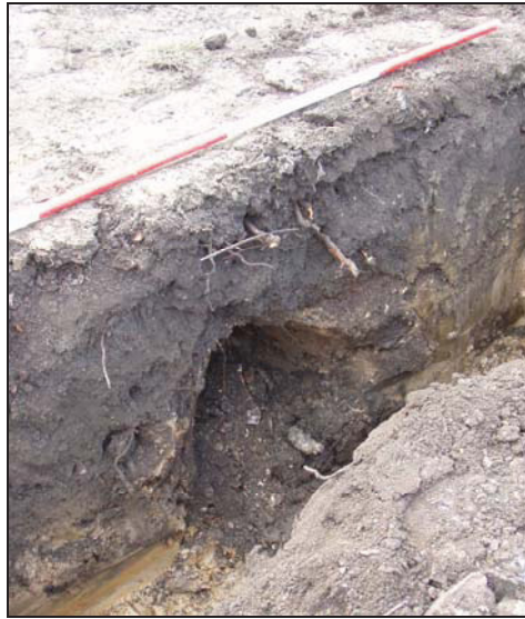
Fig. 15 Footing three showing the ceramic land drain, looking south (Scale: 0.5m graduations).
