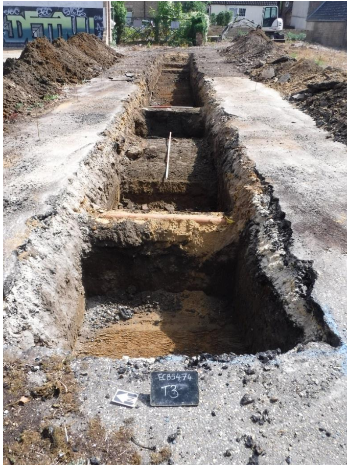
Figure 13. Western end of Trench 3, looking east. Three un-excavated baulks across the trench represent a modern pipe trench, an asbestos contaminated area and a concrete encased fuel pipe overlying contaminated ground. Scale: 0.5m graduations.
