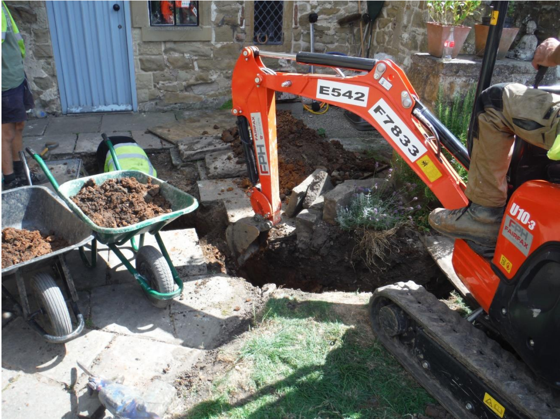
Figure 8. Excavations in the northern garden area
