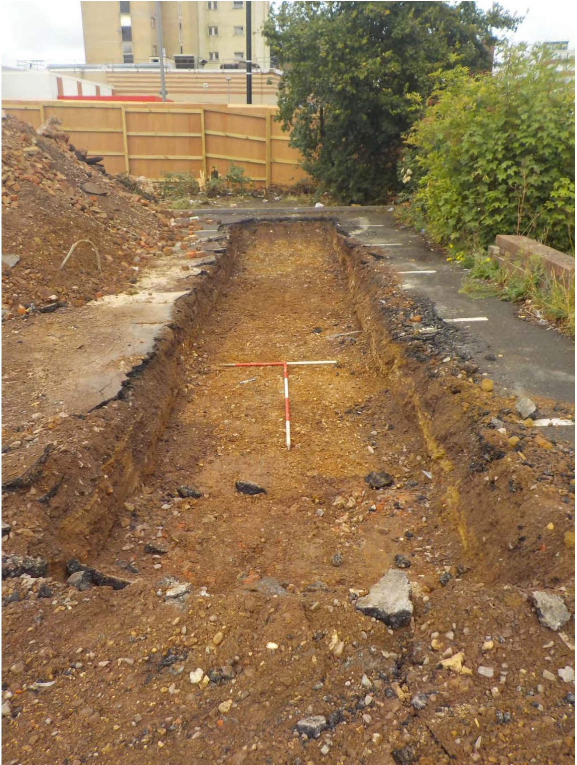
Figure 12: Trench 2 looking North west
