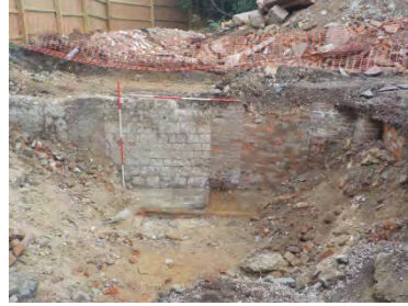
Chalk block wall in trench 1 looking north
