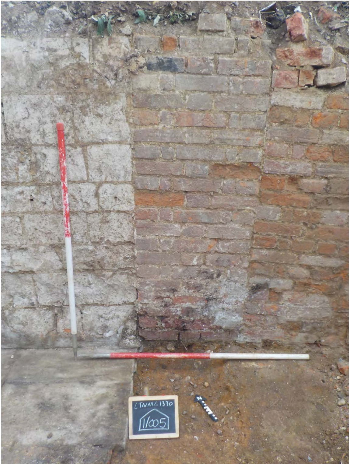
Figure 8: Wall (1/005) looking north east
