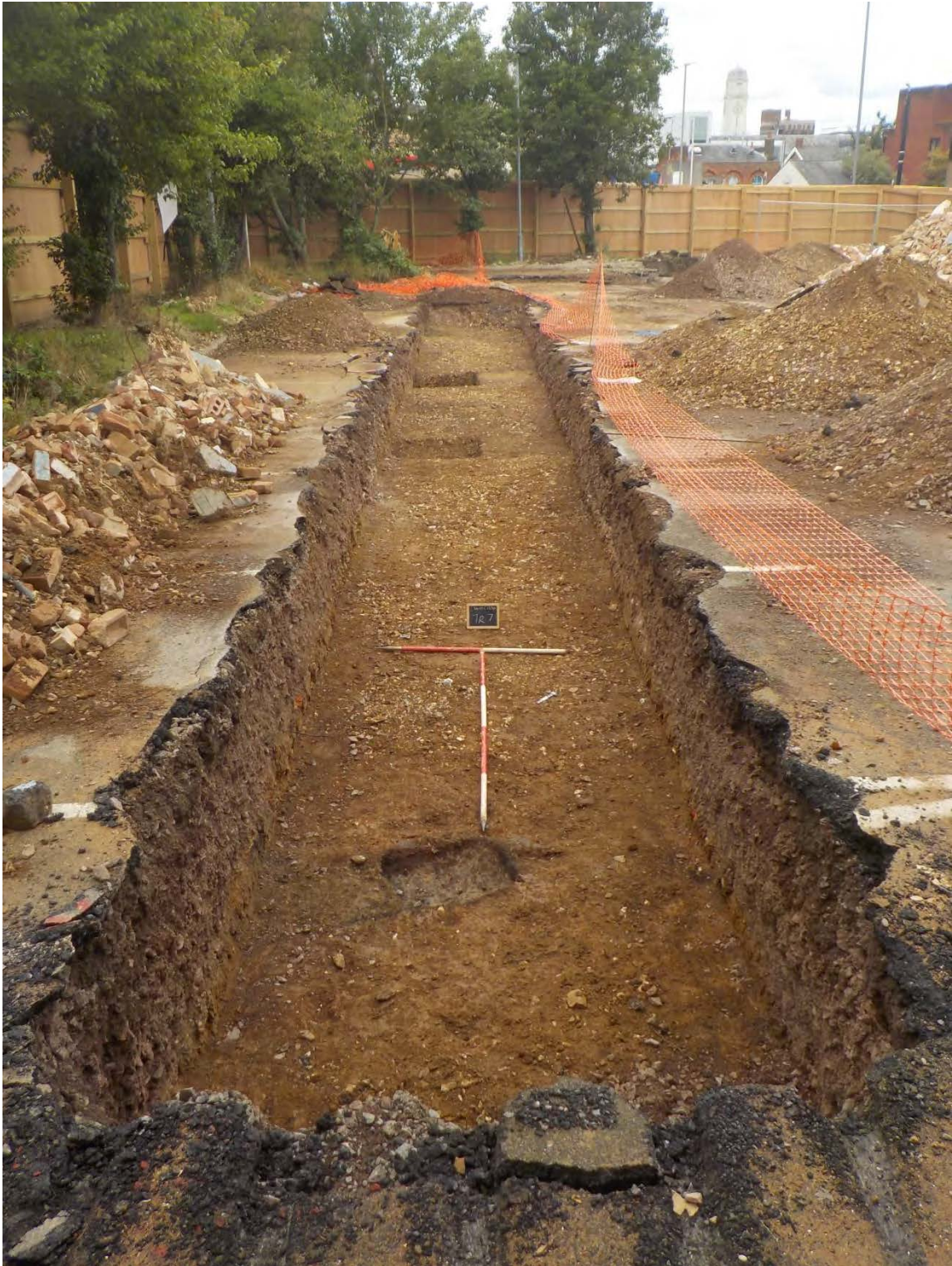
Figure 15: Trench 7 looking north west
