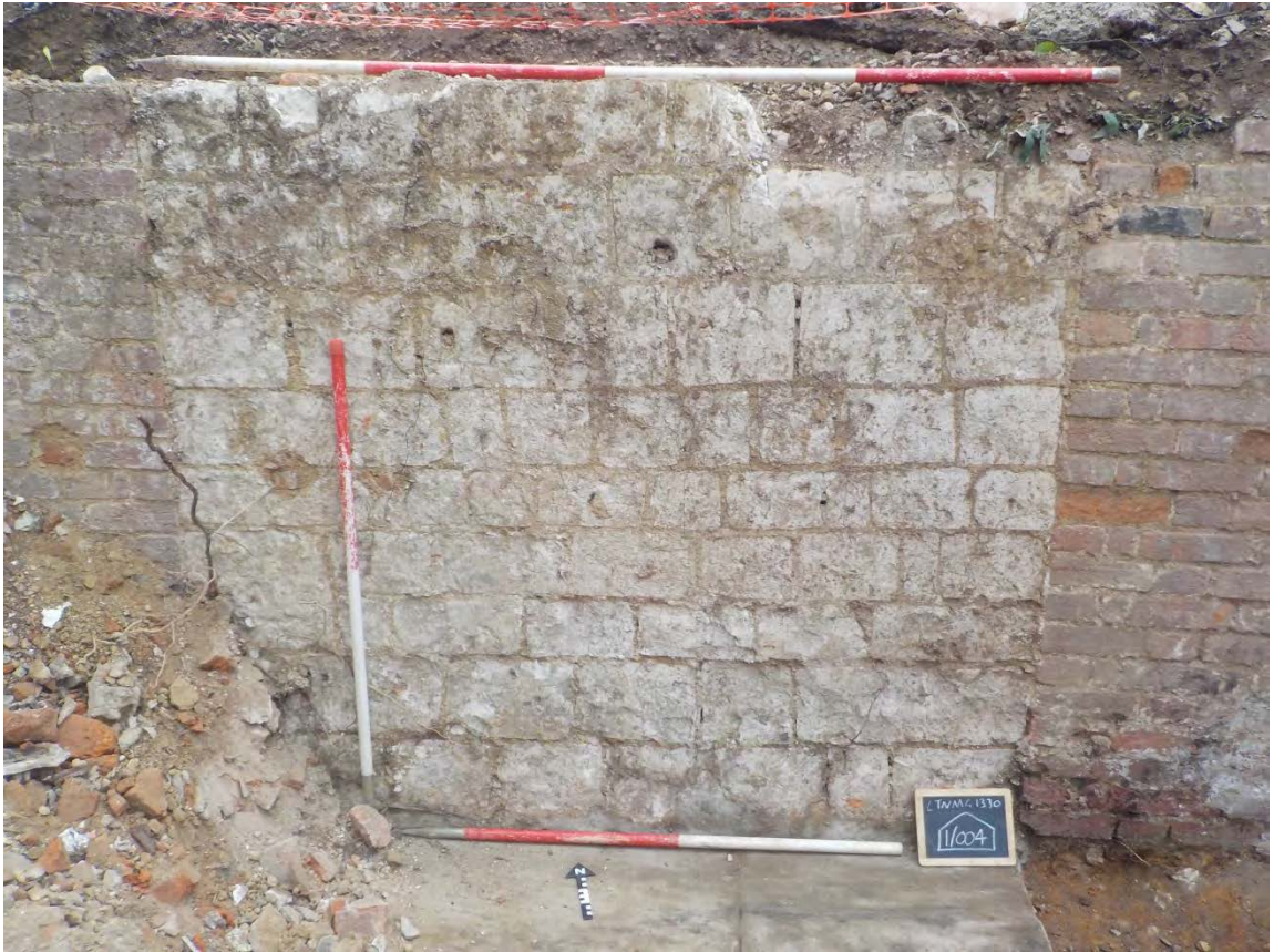
Figure 7: Wall (1/004) looking north east
