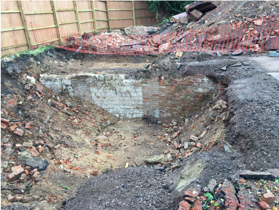
Figure 5: Trench 1 looking north
