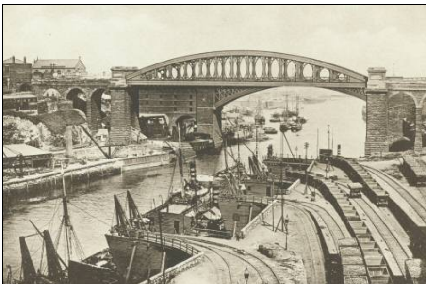
Fig. 7. (Anonymous) picture showing the bridges of Sunderland and dock workings of 1908.
