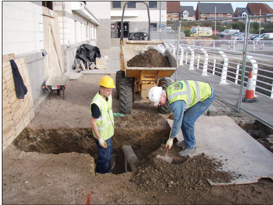
Fig. 9. Hand excavation of the foundation pit looking east
