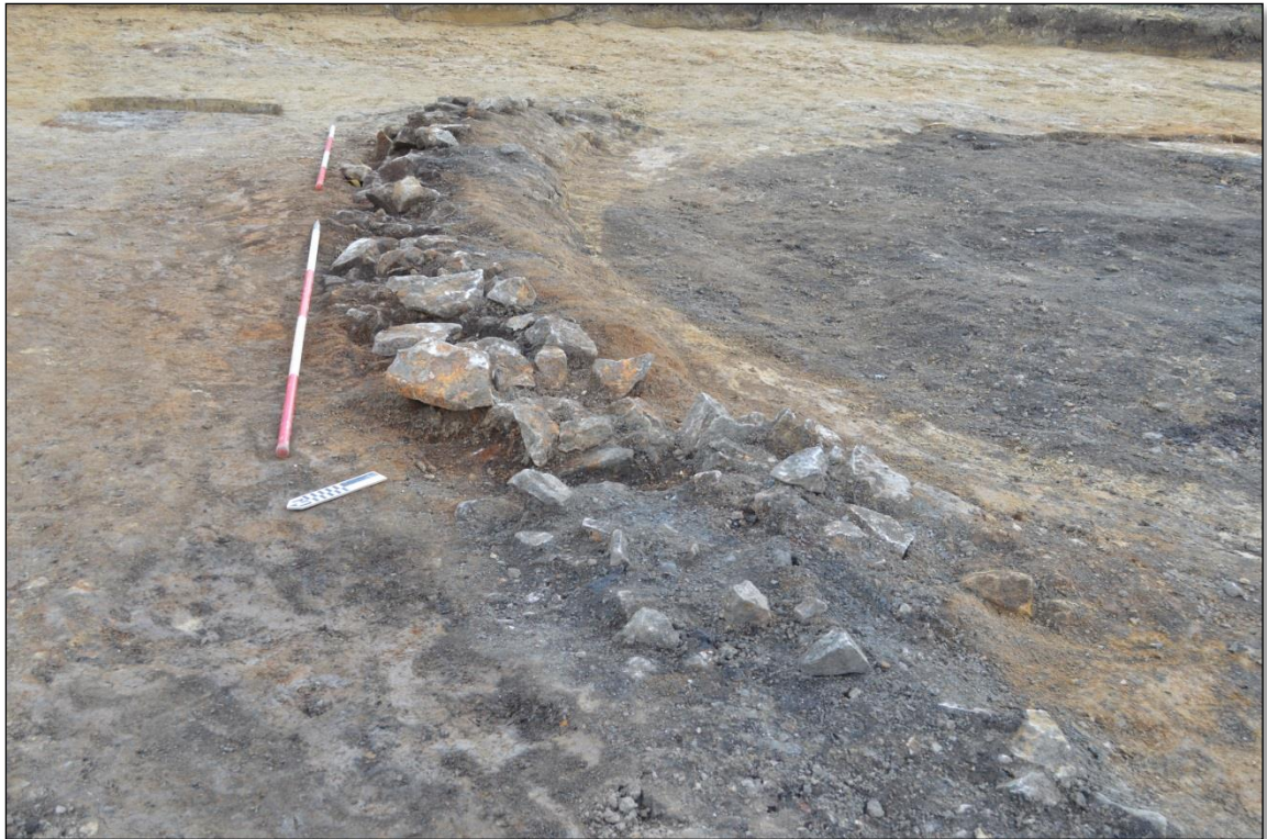
Figure 15. View south-east showing the southern wall [1048] of Enclosure 2 to the north surrounding mineshaft [1032] (scale = 2 x 2m in 0.5m graduations)
