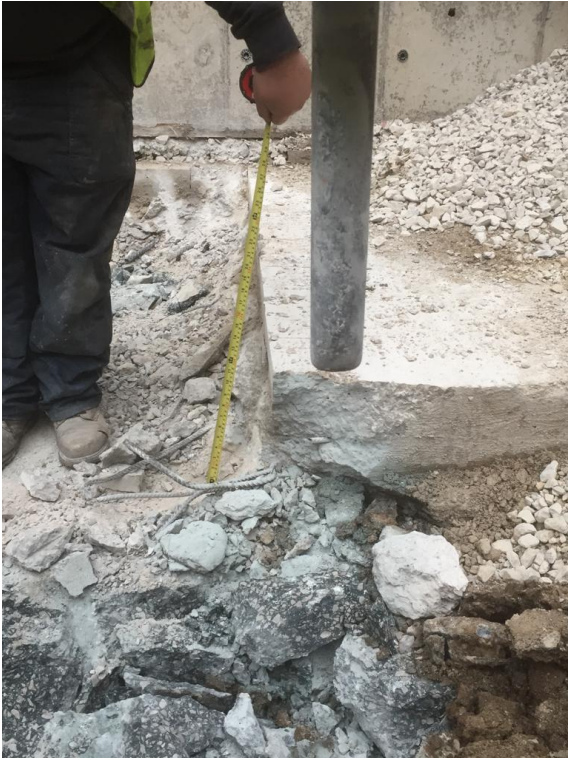
Removal of upper slab (103)
