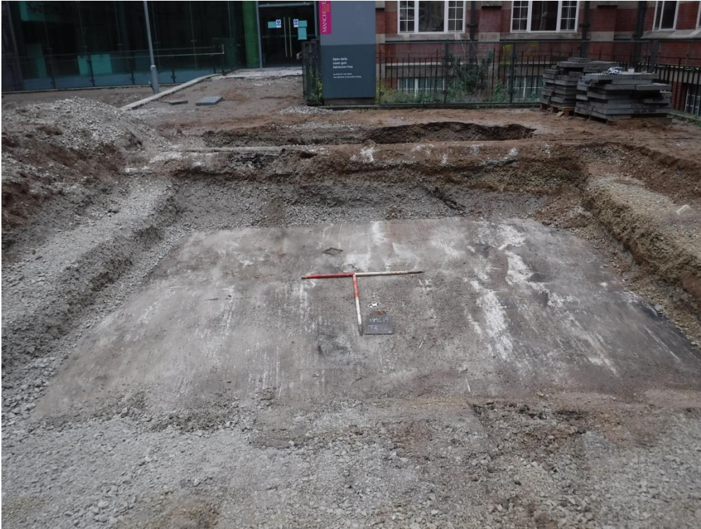
Figure 11. Trench 2, post-excavation. Slab (205) visible across the base of the entire trench. Scale: 2x1m.
