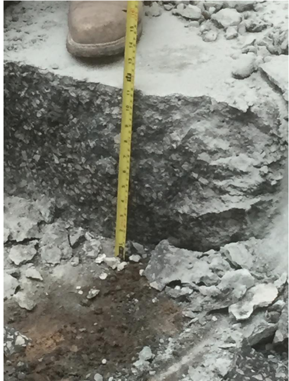
Removal of lower slab (105)
