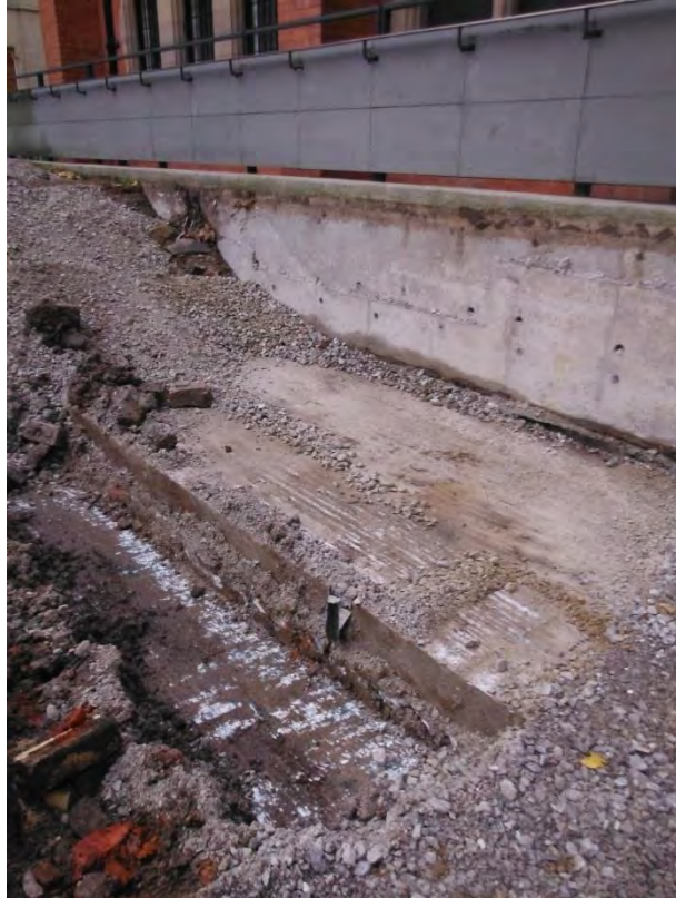
Figure 2. Concrete slabs (103) and (105) looking south.
