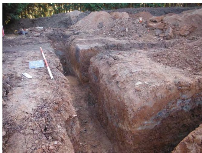
Figure 15. Footings, dwelling (Unit) 3, looking south-west. Scale 1 x 2m in 0.50m gradations
