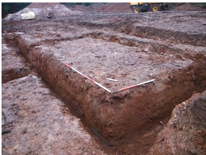
Figure 16. Footings, dwelling (Unit) 1, looking west. Scale 1 x 1m and 1 x 2m in 0.50m gradations
