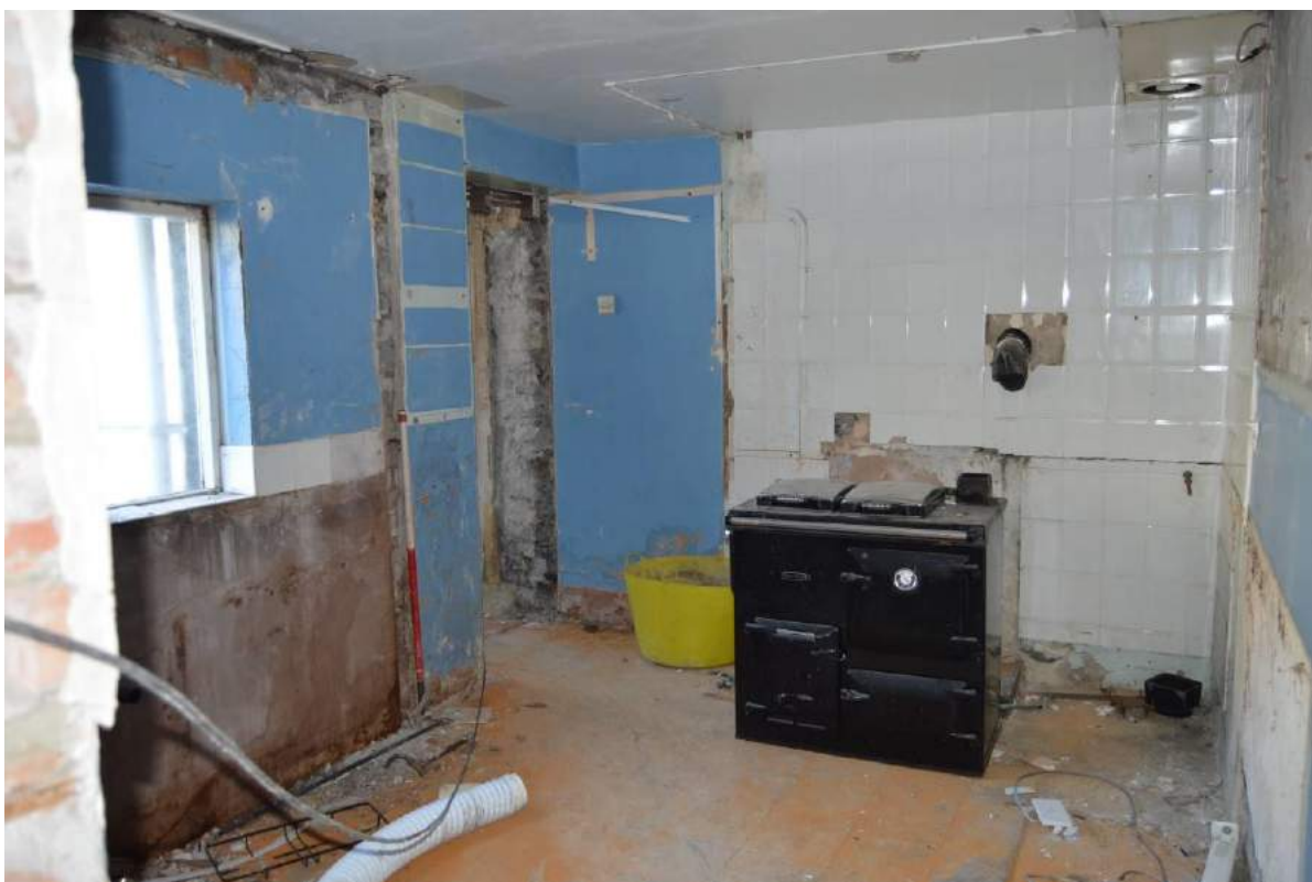
Plate 53: Kitchen in rear service range (Scale: 1 x 1m).
