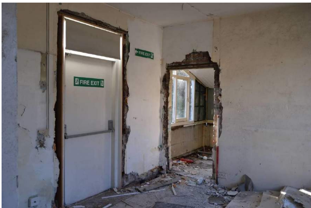
Plate 73: The room adjacent the photographic studio looking north (Scale: 1 x 2m).
