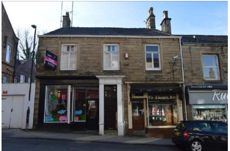
Front elevation of 3 King Street, Clitheroe.
