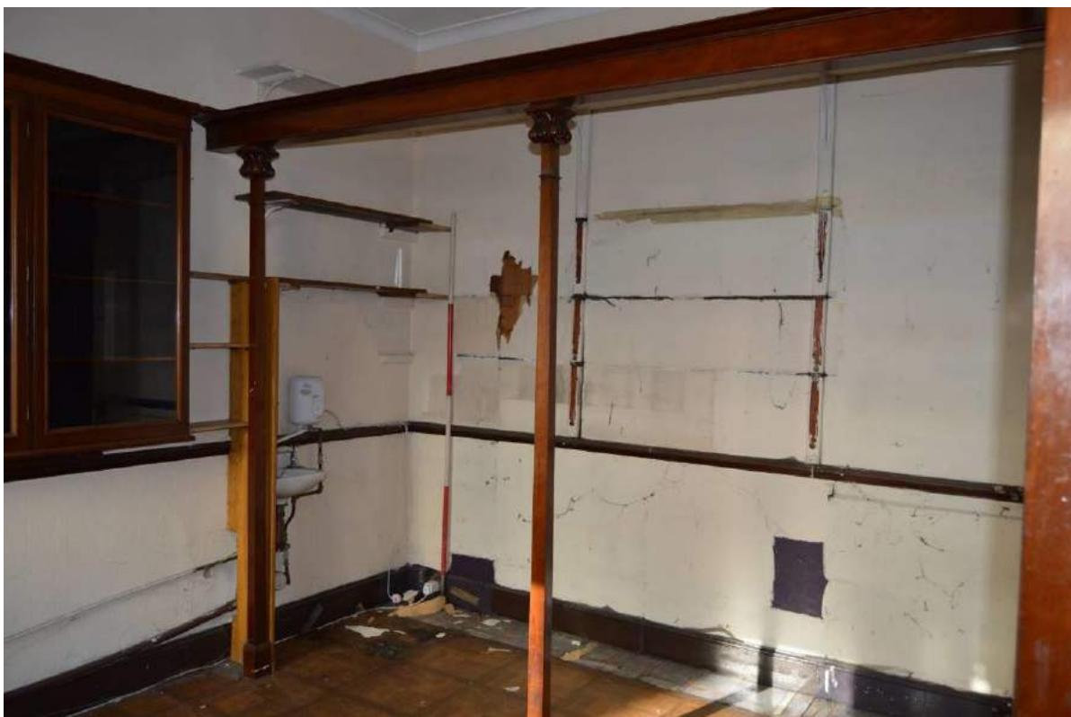
Plate 33: Rear of the shop (G2). Note a doorway is blocked adjacent the far corner (Scale: 1 x 2m).
