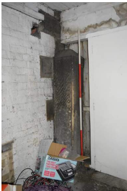
Plate 14: Stone gate pillar and also the building's quoin stones (Scale: 1 x 2m).
