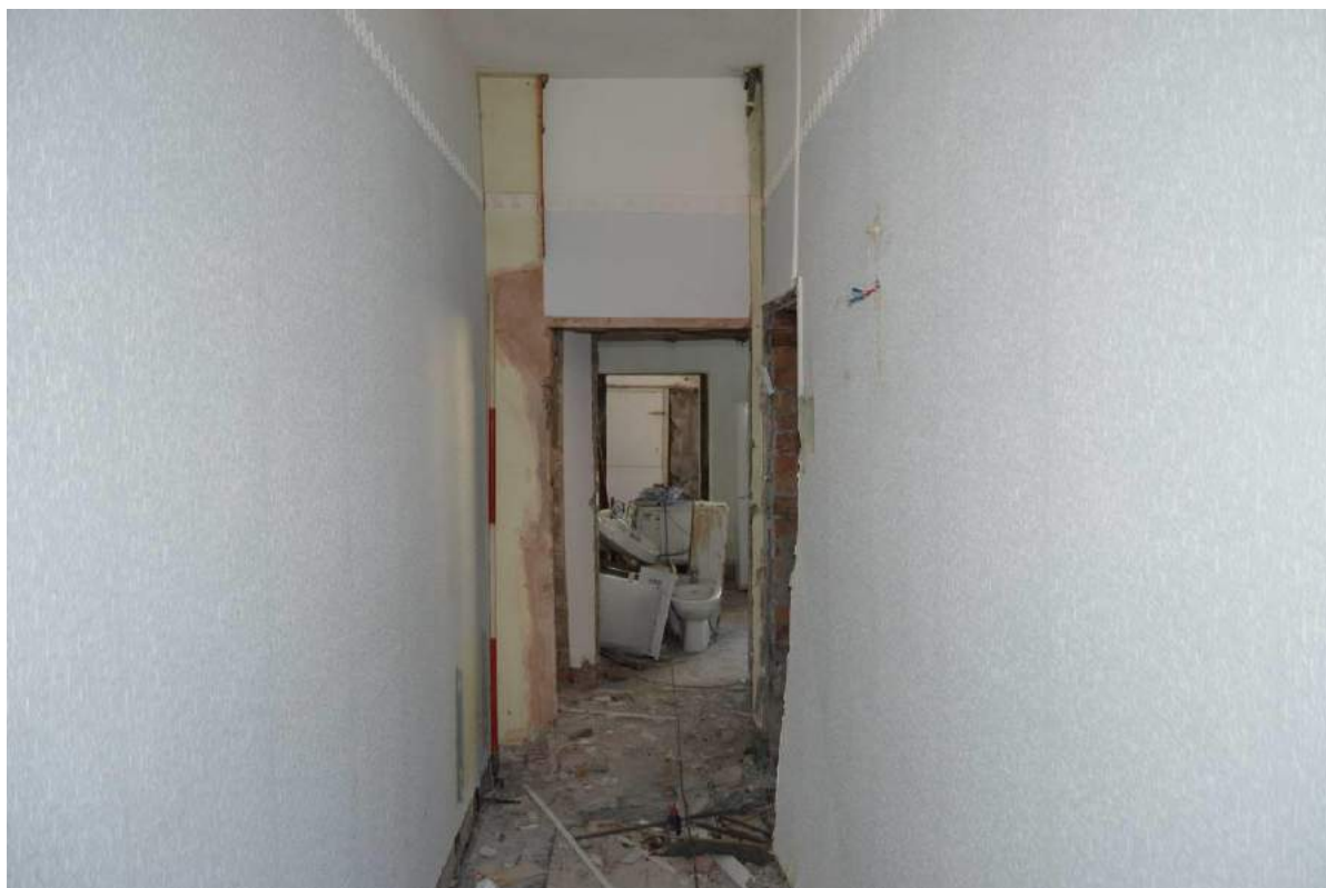
Plate 35: Interior of hallway (Scale: 1 x 2m).
