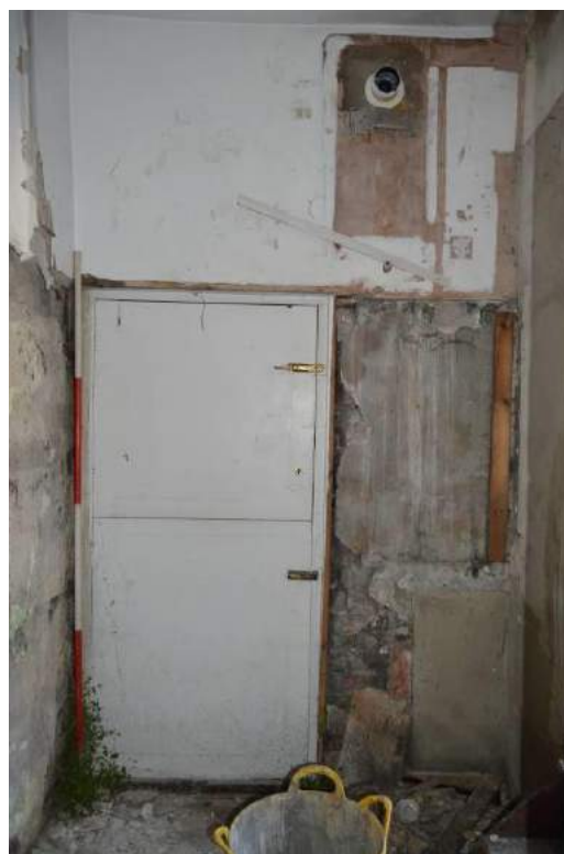
Plate 52: Lobby, with stable type door to rear yard/garden (Scale: 1 x 2m).
