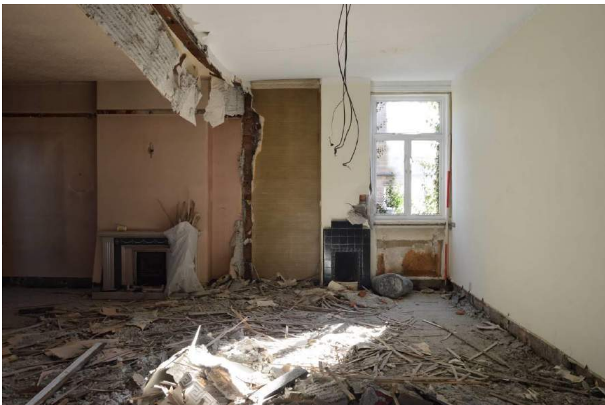
Plate 64: View towards the small first floor room (F3) (Scale: 1 x 2m).
