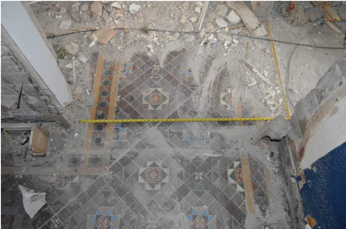
Plate 43: Hallway geometric tiles. Note the line of a later partition wall over the top.
