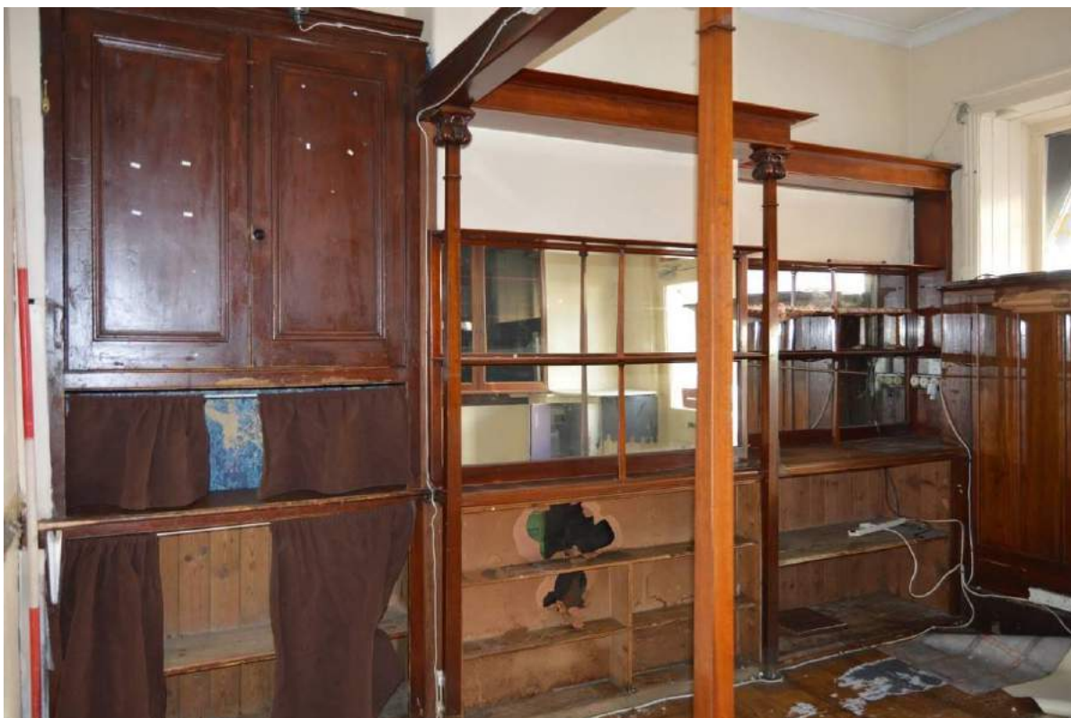
Plate 32: Interior of hallway (Scale: 1 x 2m).
