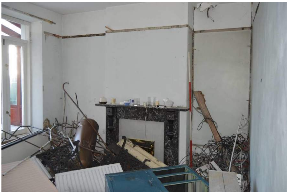
Plate 48: View of north west reception room (G5) (Scale: 1 x 2m).
