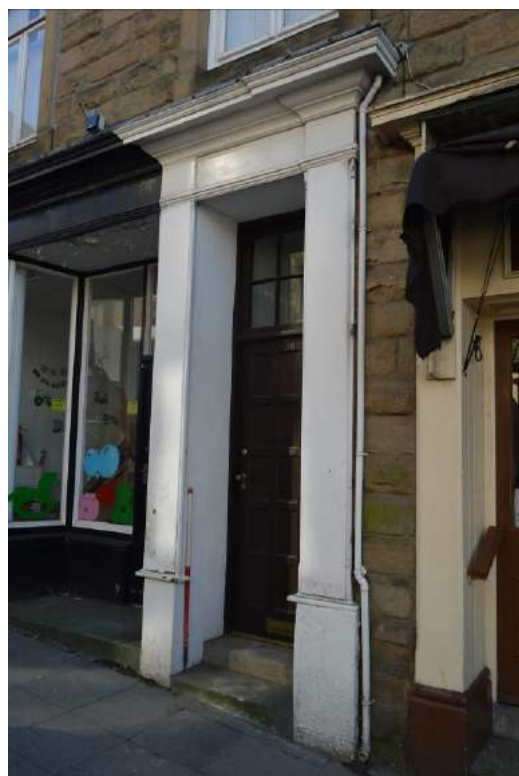
Plate 4: Central domestic entrance. Note the mismatched pilasters (Scale: 1 x 1m).
