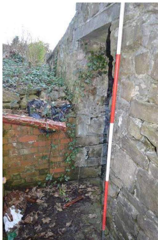
Plate 27: Entrance to stone outbuilding, originally a privy/washhouse (Scale: 1 x 2m).
