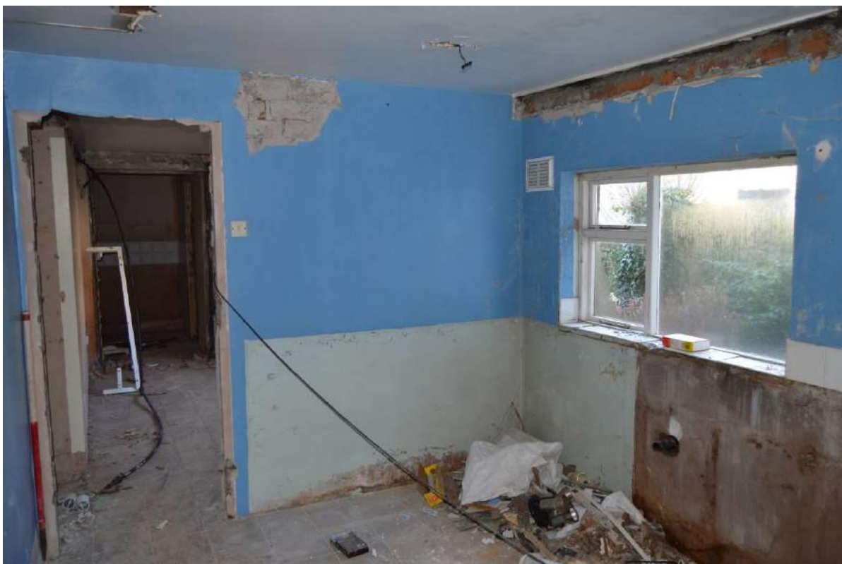
Plate 54: Kitchen in rear service range (Scale: 1 x 2m).
