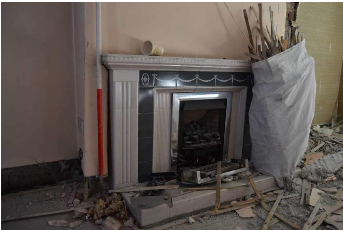
Plate 63: Fireplace in front first floor room F2 (Scale: 1 x 2m).
