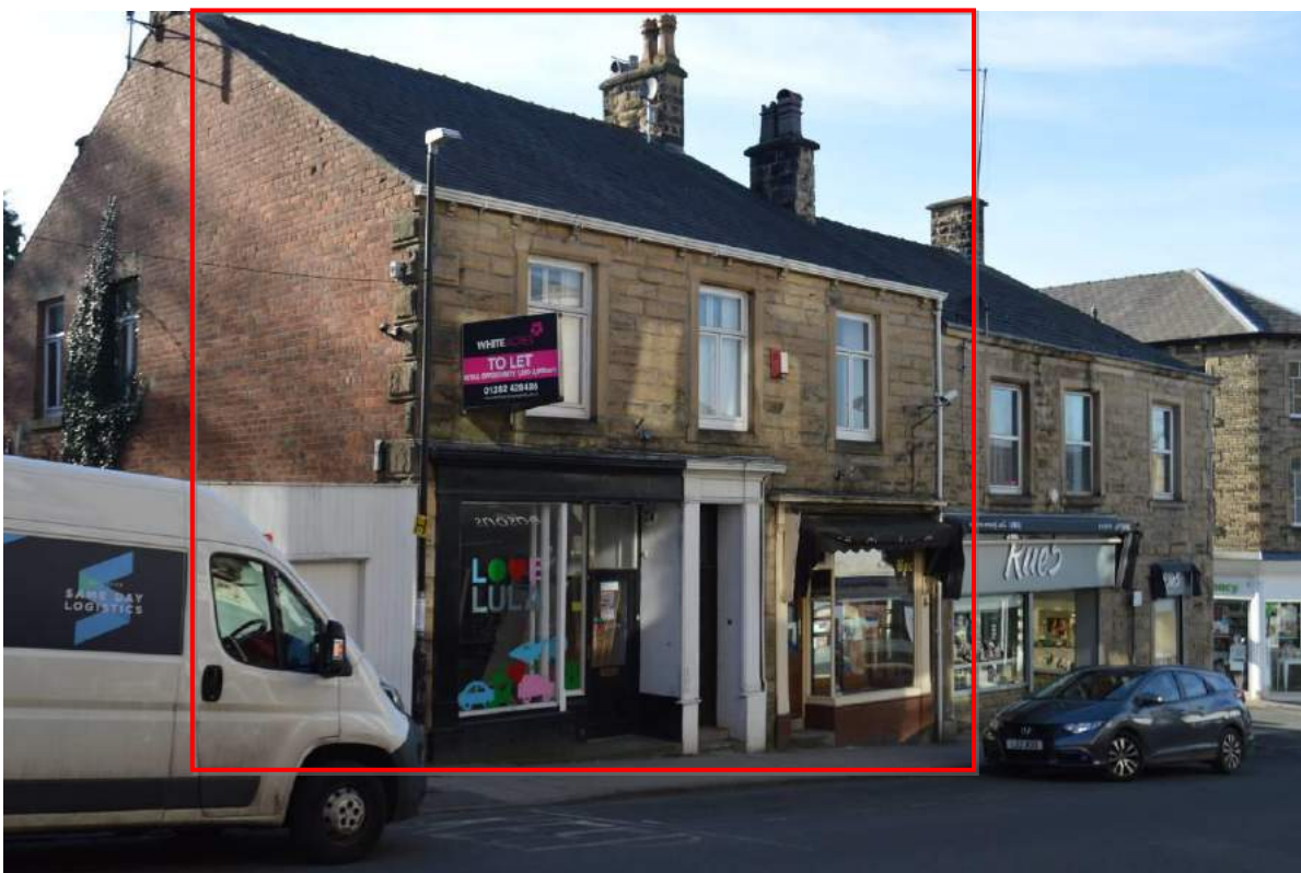
Plate 2: Oblique view of the front elevation of 3 King Street, facing west.
