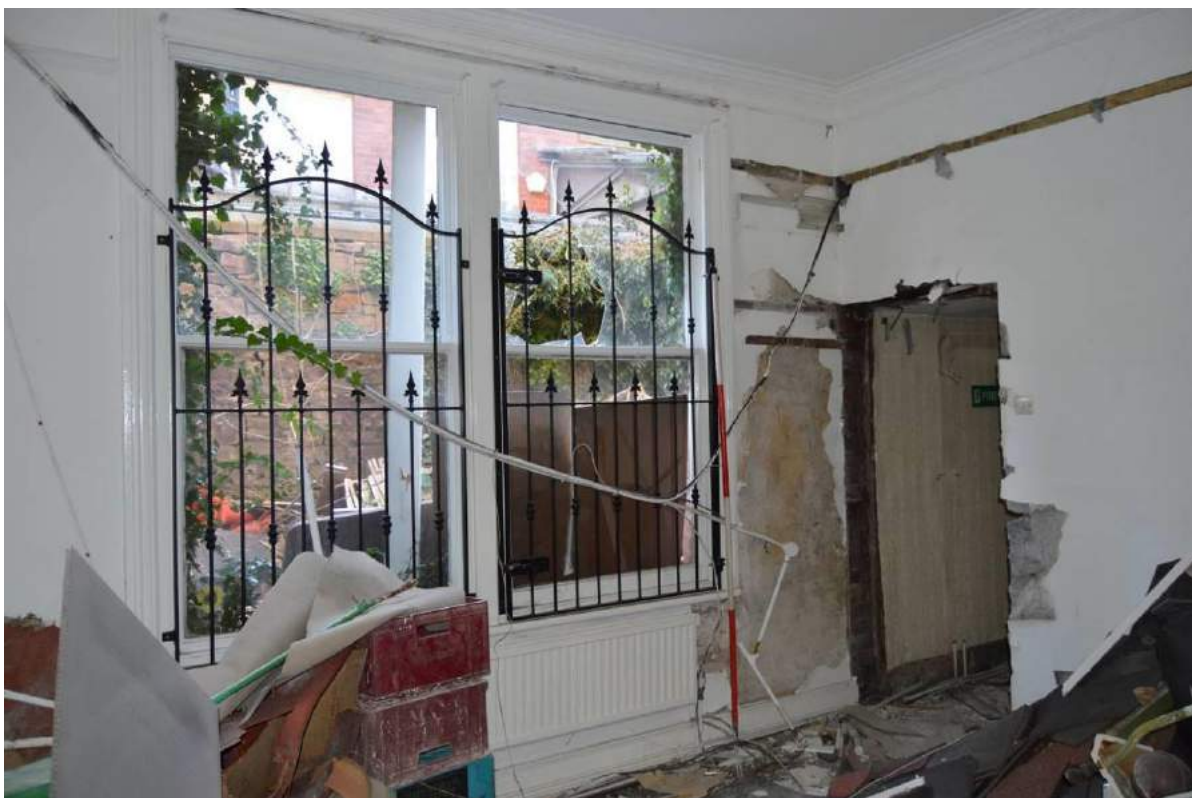
Plate 45: Double sash windows to G3 (Scale: 1 x 2m).
