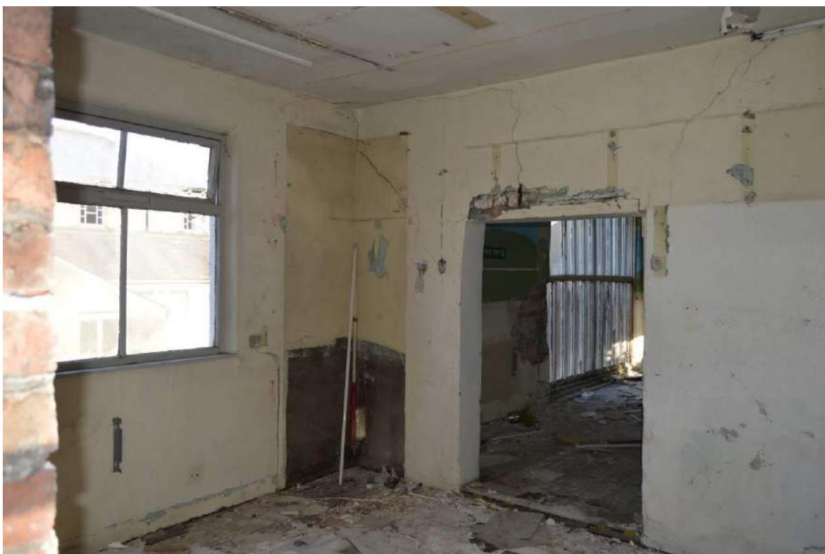
Plate 72: The room adjacent the photographic studio looking north (Scale: 1 x 2m).
