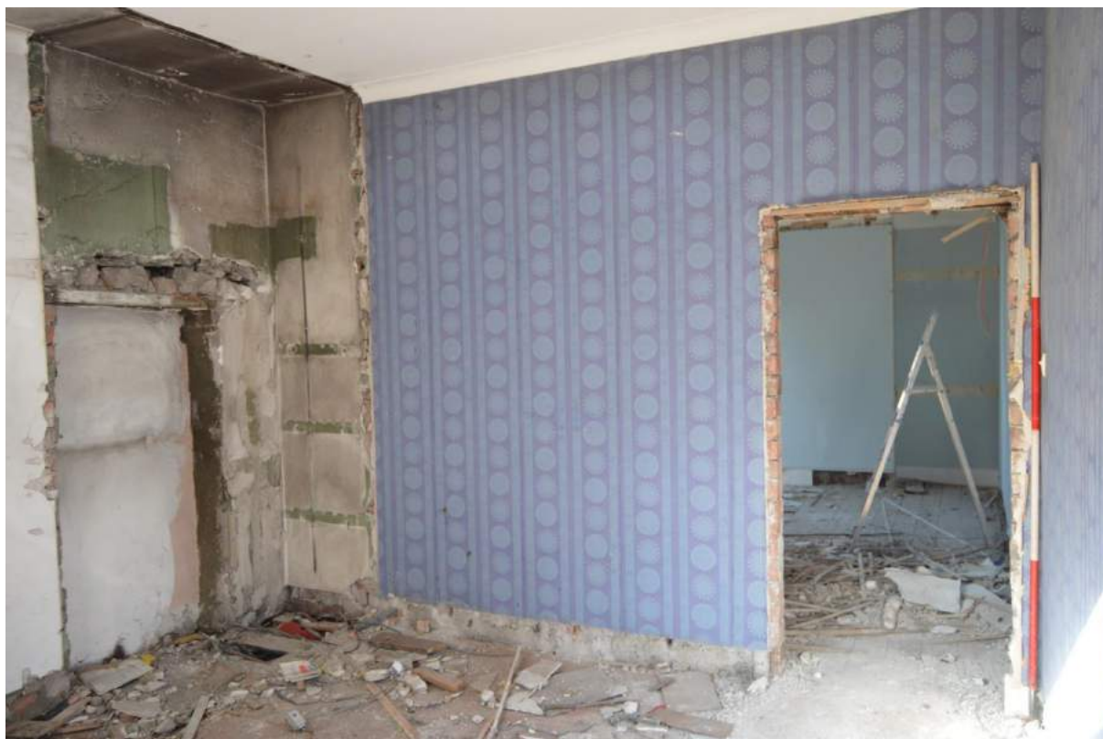
Plate 67: Interior of rear bedroom (F5) (Scale: 1 x 2m).
