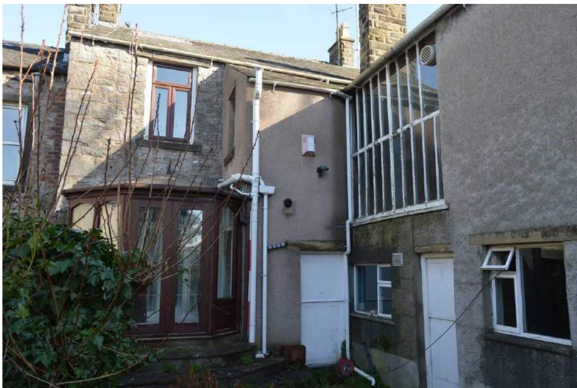
Plate 21: North west elevation of rear service range where it meets the principal building. Note the large daylight studio window (Scale: 1 x 2m).
