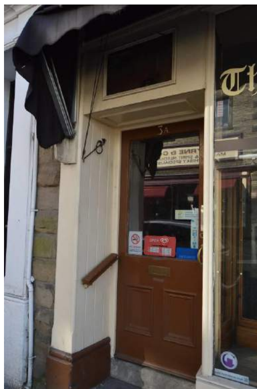
Plate 5: View of the north shop front entrance, the older of the two entrances (Scale: 1 x 1m).
