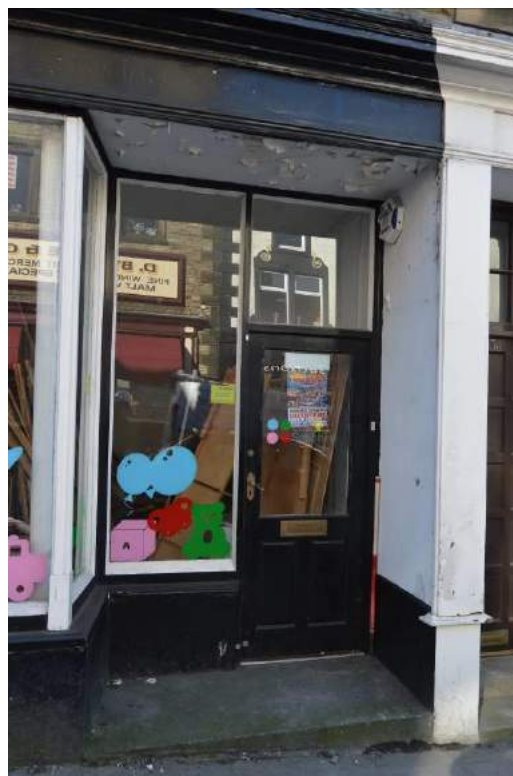
Plate 8: View of south shop front entrance (Scale: 1 x 1m).
