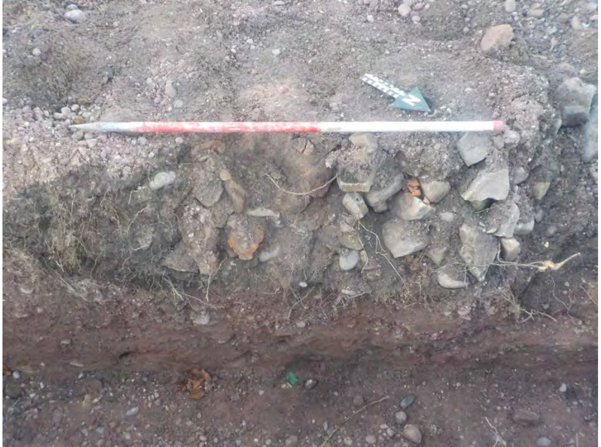
Figure 6: South-east facing baulk section of the north-west part of the site, showing the made ground in this area (scale 1m in 0.5m graduations).
