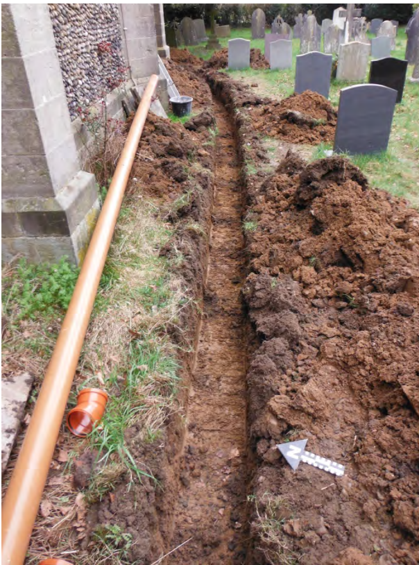
Figure 12 Trench for new storm drain, looking east
