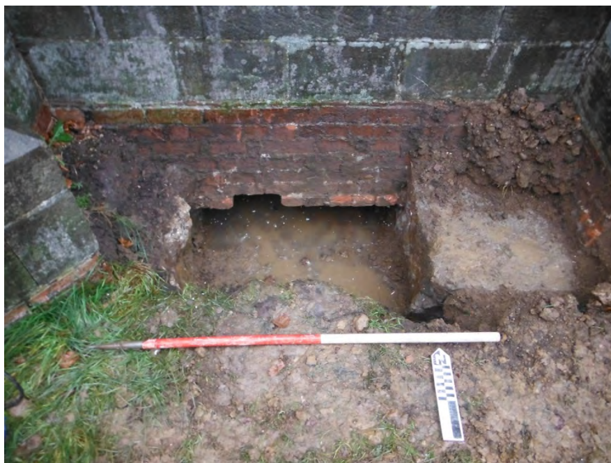
Figure 7 South wall brick foundation
