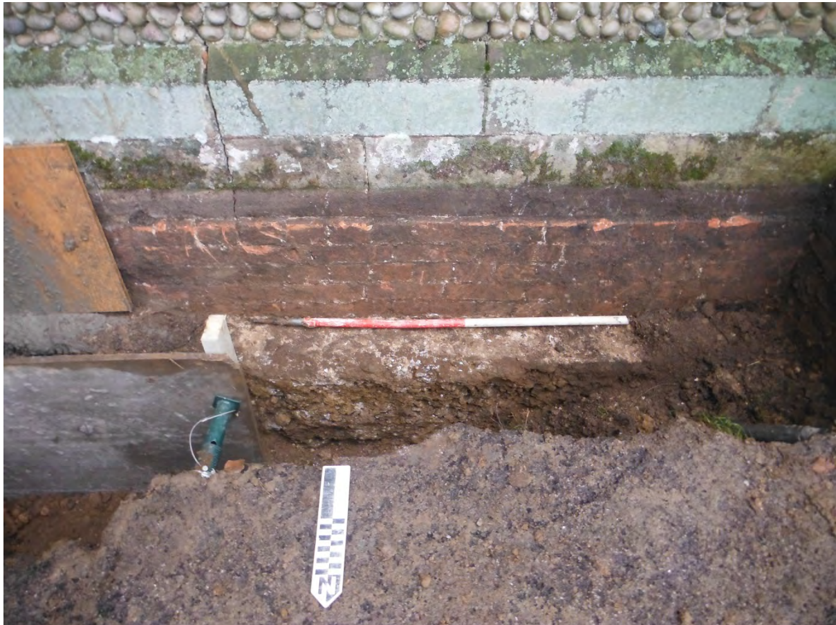
Figure 4 Brick foundation (006) and concrete underpinning (005) of north wall of nave
