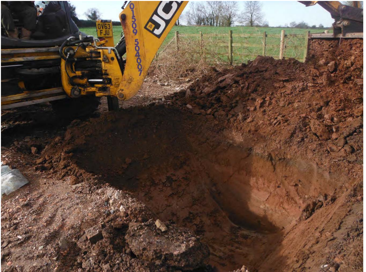
Figure 9: Test pit 1 looking south-west
