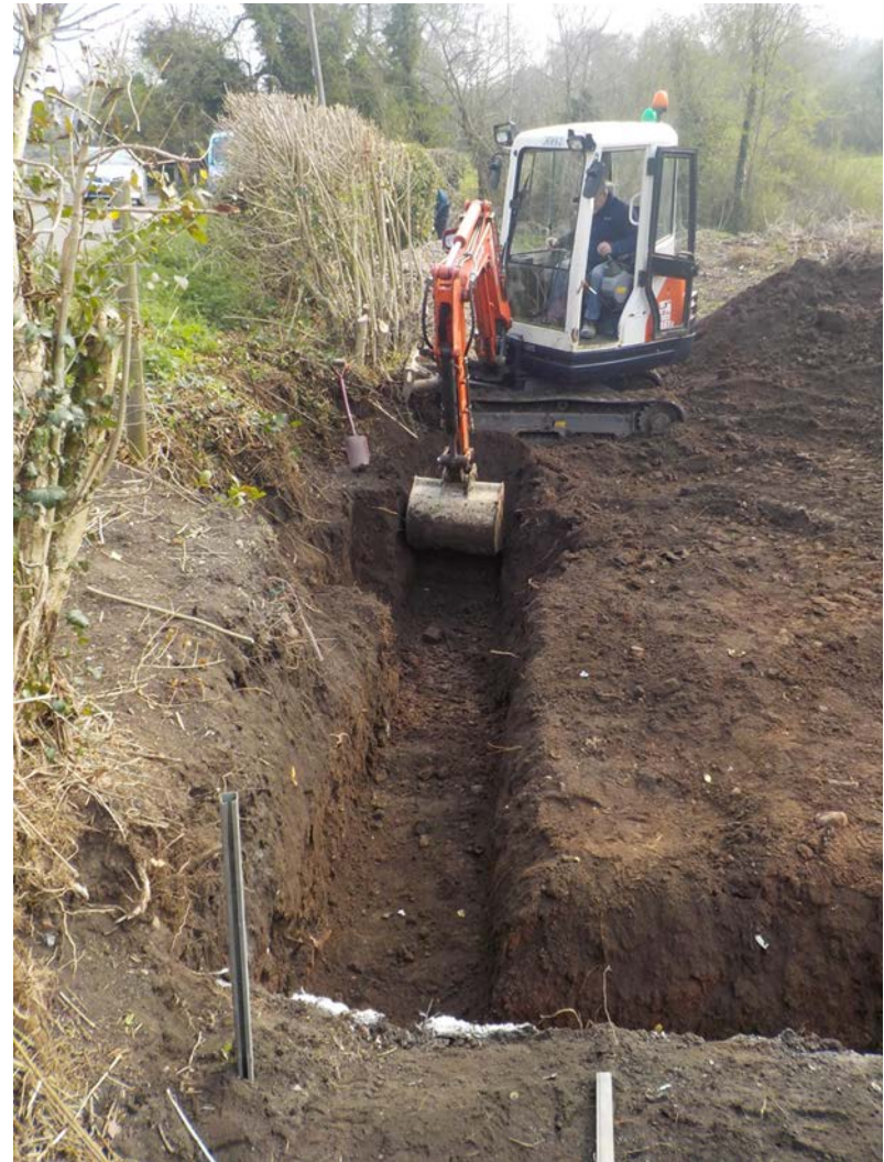
Figure 8: North wall foundation trench looking east
