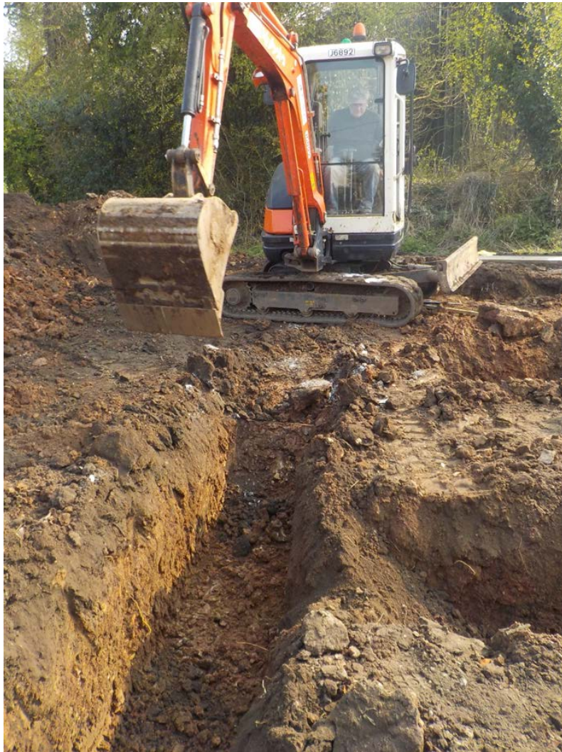
Figure 9: Excavation of the east wall foundation trench.
