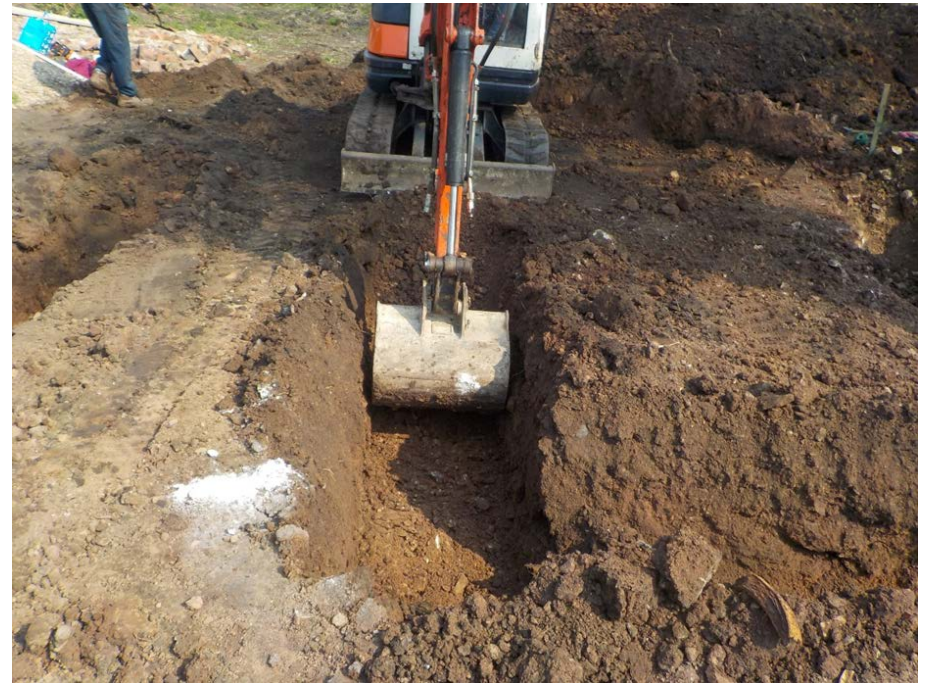
Figure 10: Excavation of internal dividing wall foundation.
