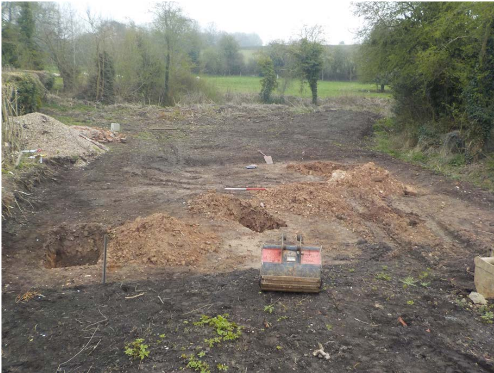
Figure 3: Post-ex test pits 1, 2 & 3 (left to right)
