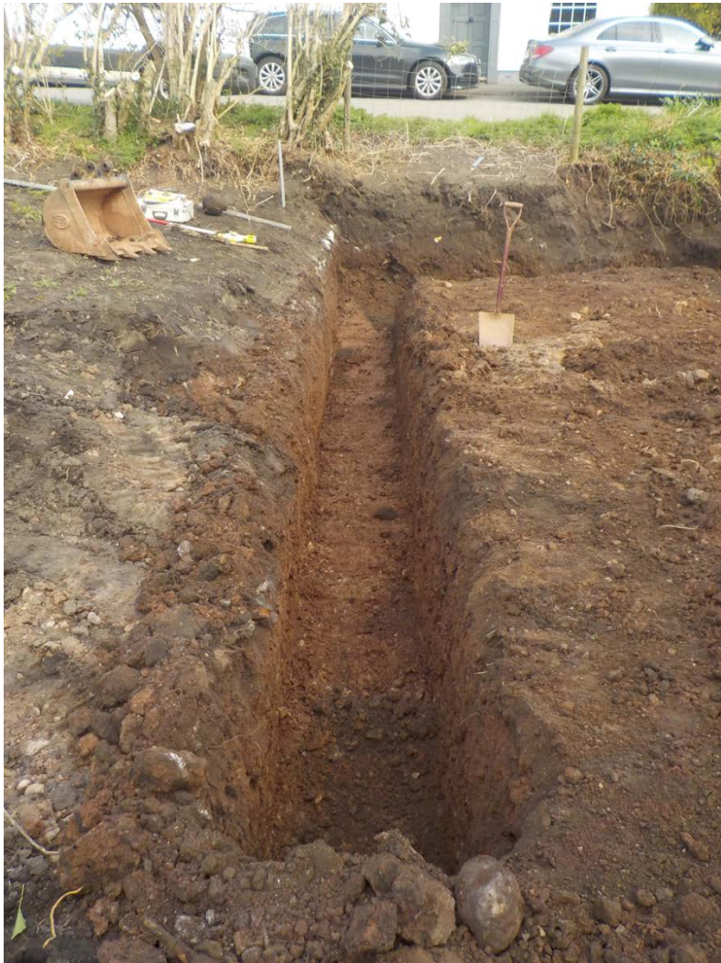
Figure 7: West wall foundation trench looking north
