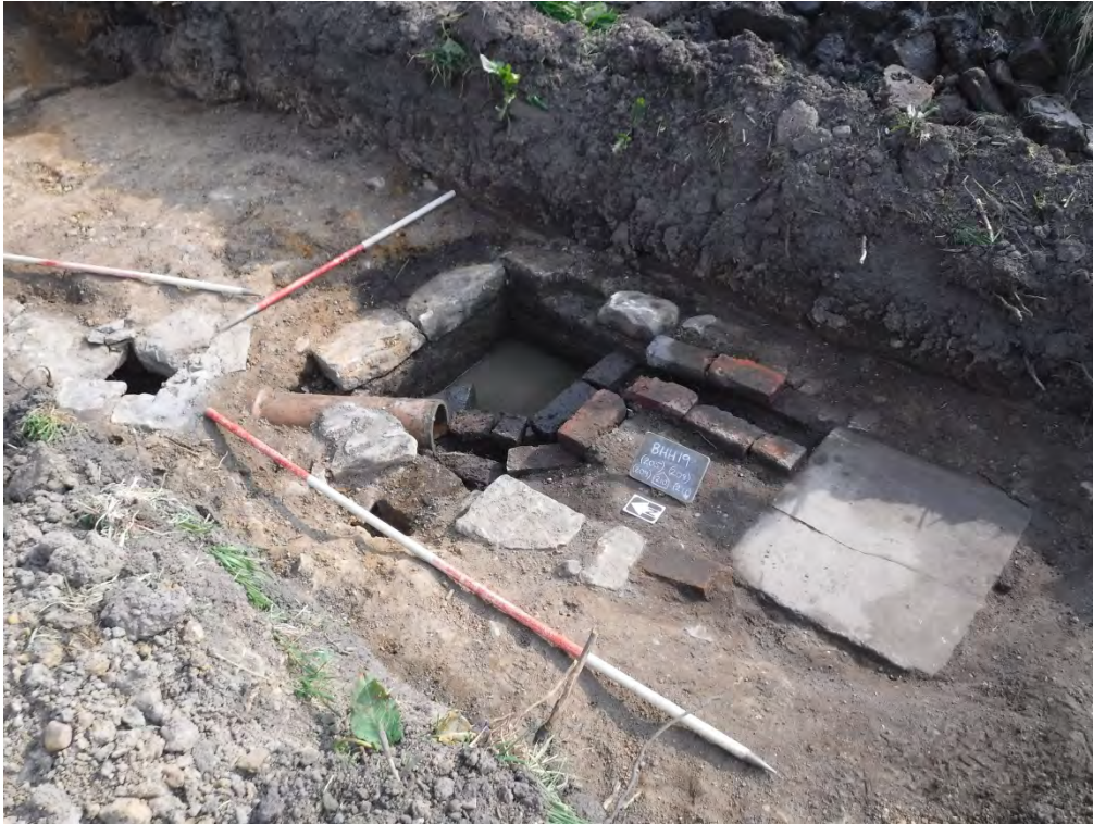
Figure 12. Culvert (205) on the left, repaired with pipe (208) that directs water into brick channel (209) through stone-lined sump/tank (210). Cap for lower chamber of tank visible on the right. Scale: 0.5m graduations.
