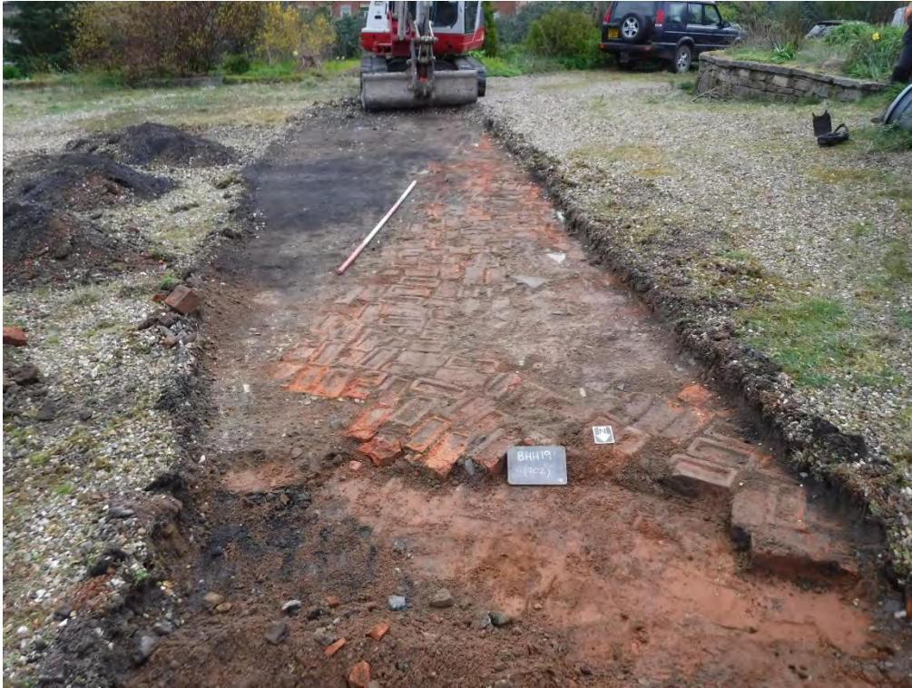
Figure 20. Trench 7, looking south-south-east. Rough brick surface (702) identified just under the modern surface, with sand deposit (703) in the foreground and compacted black, gritty surface (704) adjacent to bricks in the background. Scale: 2m.
