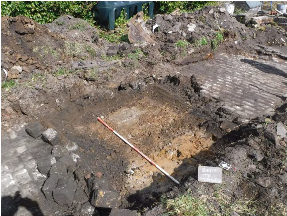
Figure 19. Removal of a portion of the granite setts was undertaken in order to reveal any hidden remains of earlier structures that might correspond with a building depicted on the 1842 Lower Tottington Tithe map. No such features were identified.
