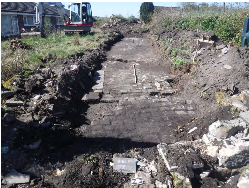
Figure 17. Trench 6, looking west. Road surface of granite setts (603) covering much of the trench, partially edged on the southern side by kerb stones (604). Cut through centre of surface is modern and housed a redundant oil pipe linking the bungalow to the tank at the right of the photo. Scale: 2x2m.
