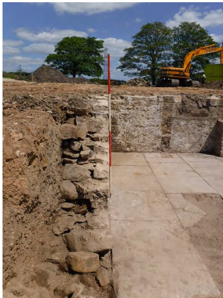
Figure 17. View through truncated wall (1175). Section shows the construction of the wall with a finished internal face and a rougher finish against the construction cut. Scale: 2m.
