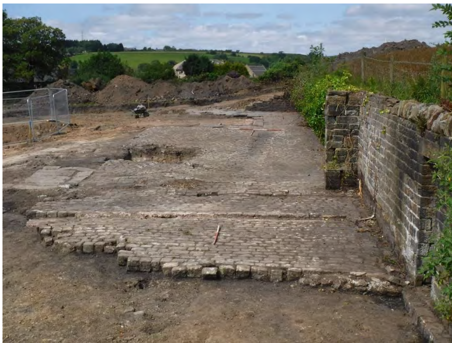
Figure 8. Overview of the cobbled road, looking west. Sunken alignment of setts visible running east/west through the surface. Scale: 0.5m graduations.
