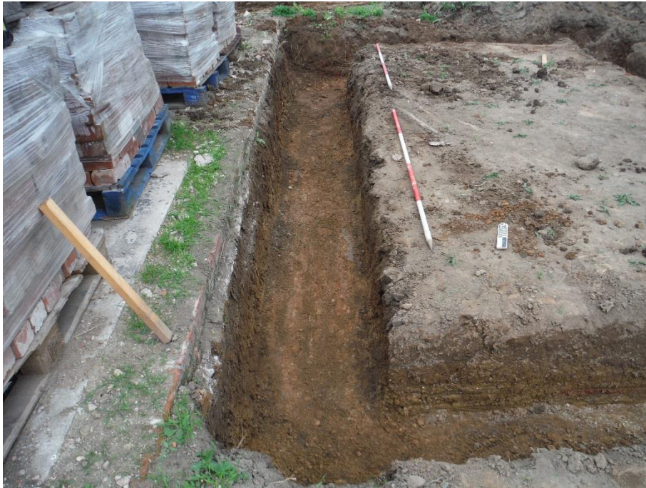
Figure 7: Excavated foundation trench, looking north-west (scale in 2x2m in 0.5m graduations)
