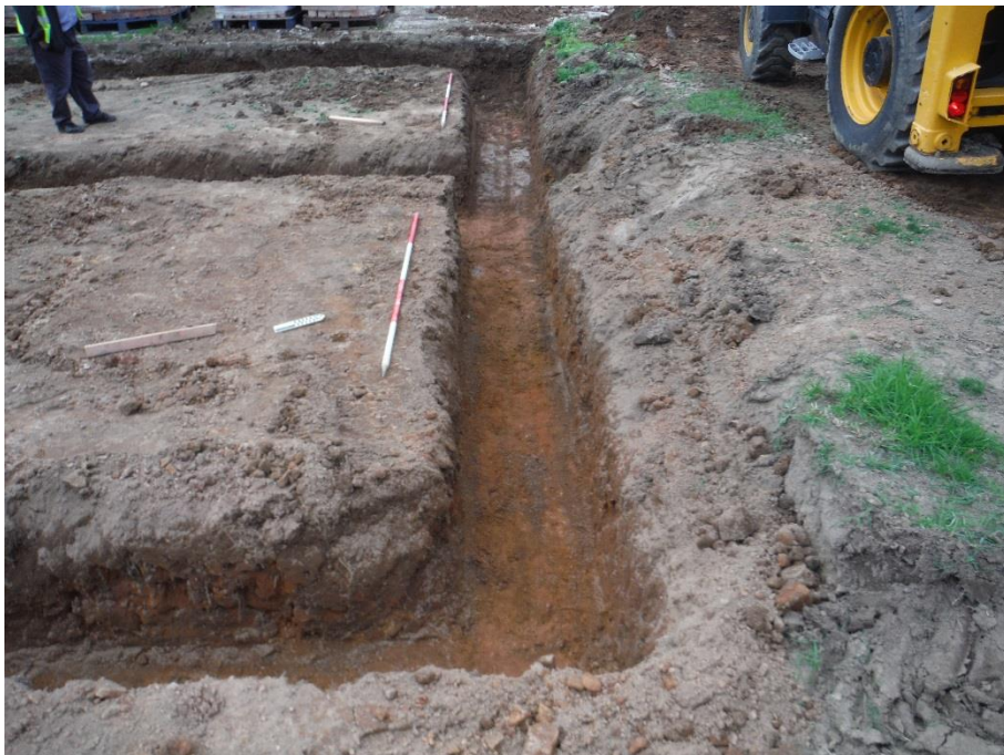
Figure 4: Excavated foundation trench, looking north-west (scale 2x2m in 0.5m graduations)
