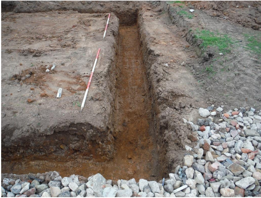
Figure 5: Excavated foundation trench, looking north (scale 2x2m in 0.5m graduations)
