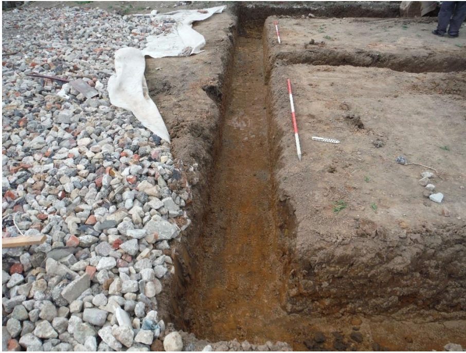
Figure 3: Excavated foundation trench, looking south-west (scale 2x2m in 0.5m graduations)
