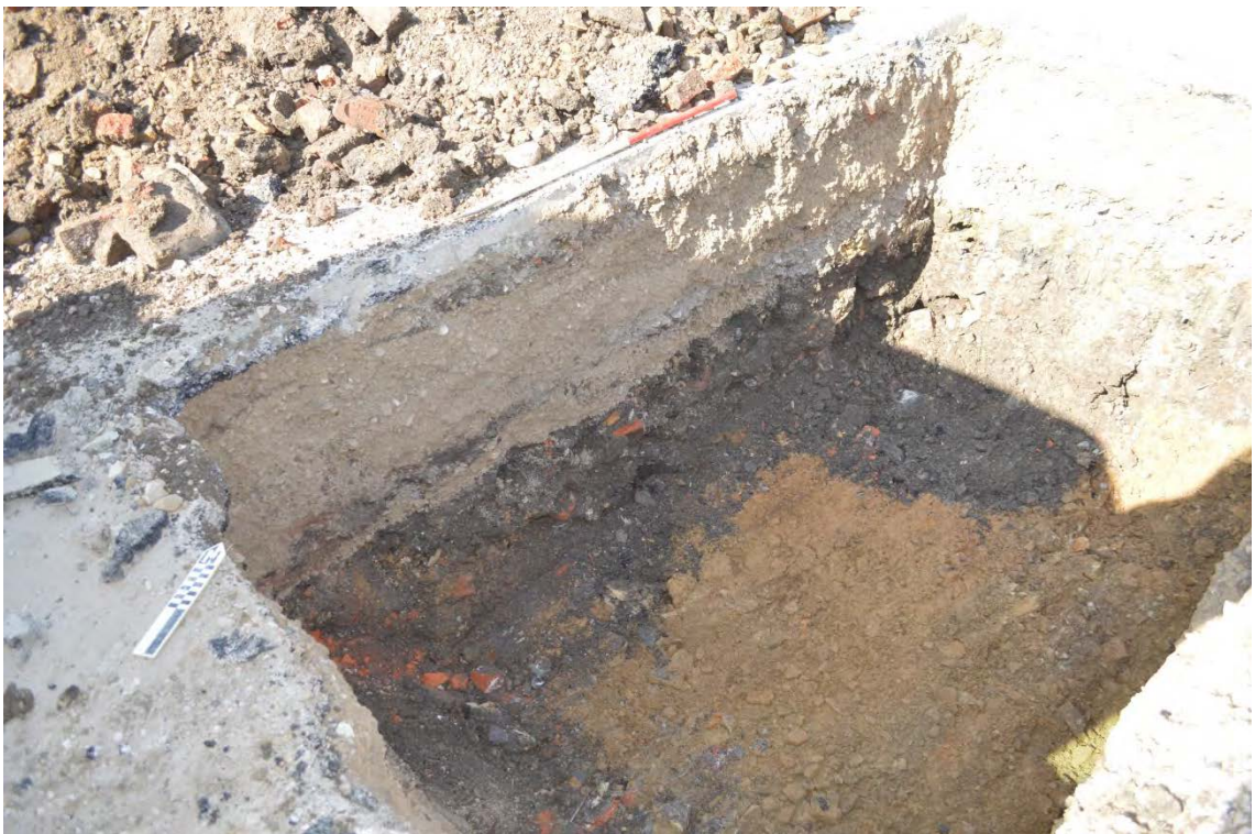
Figure 10. View north east of Trench 4, showing pit [405] in the north-west corner (scale =1x1m in 0.5m graduations).
