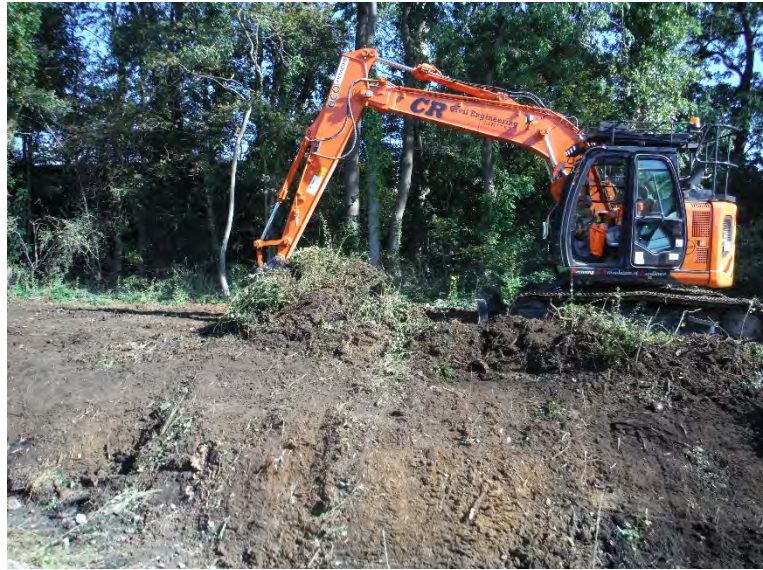
Working shot during the initial stripping of site
