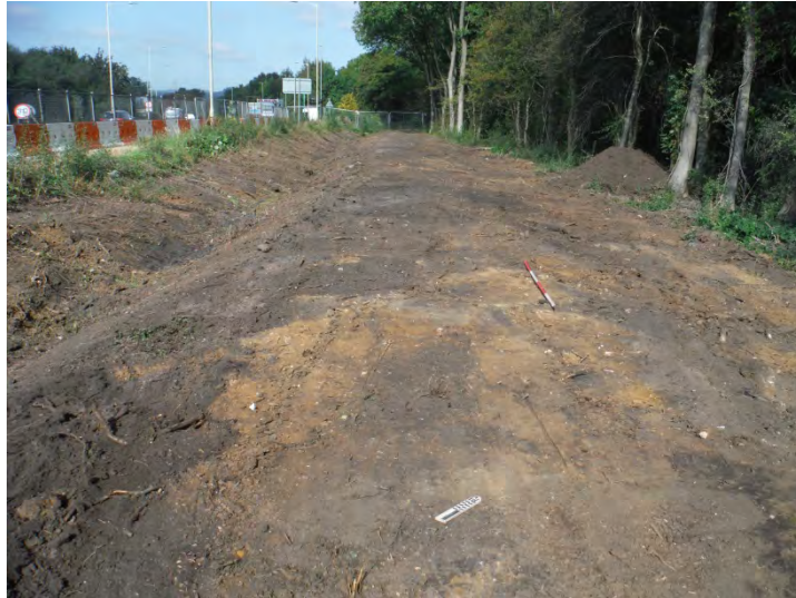
Figure 9. Area Shot of Stripped Area
