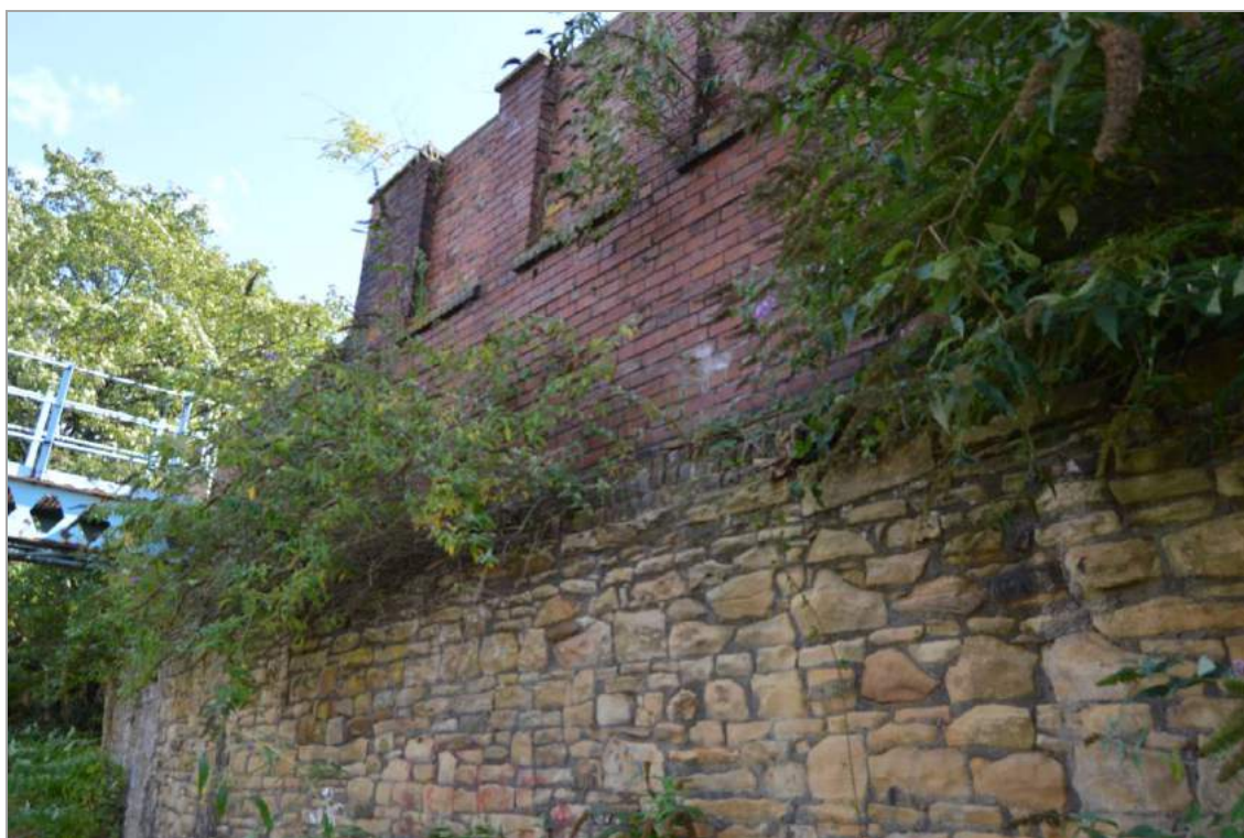
Plate 17: Structure 4 from the canal towpath (facing south east).
