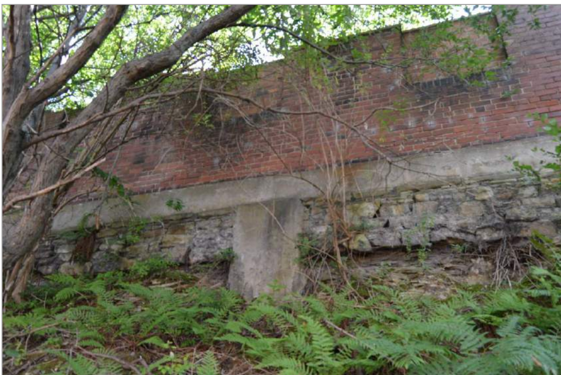
Plate 6: The north aspect of Structure 1 intermediate section (facing south east).
