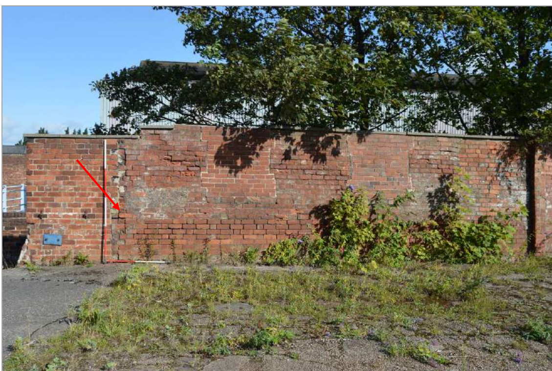
Plate 14: South face of Structure 2. Scale 2m.
