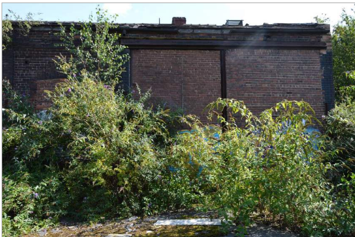
Plate 37: Two bays to the south of the east. Scale 2m.
