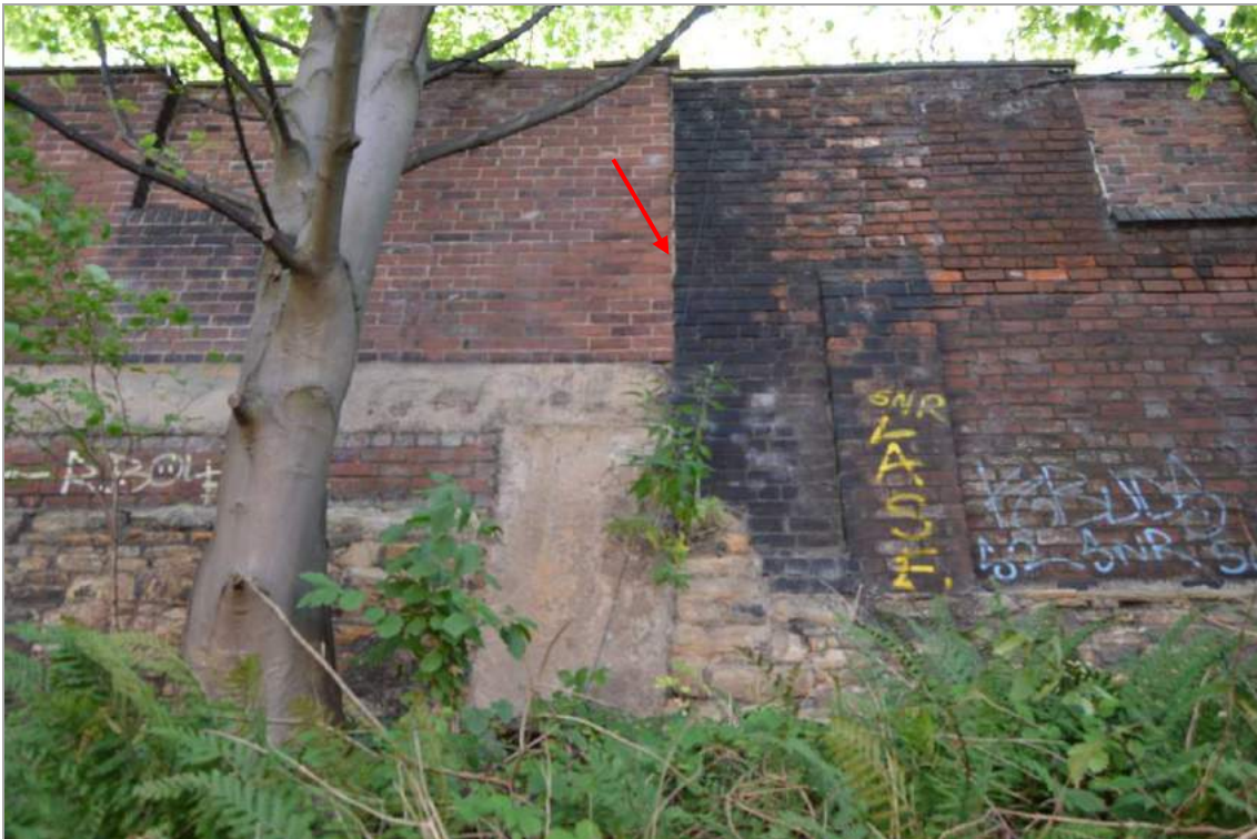
Plate 12: Structure 2, to right (facing south).
