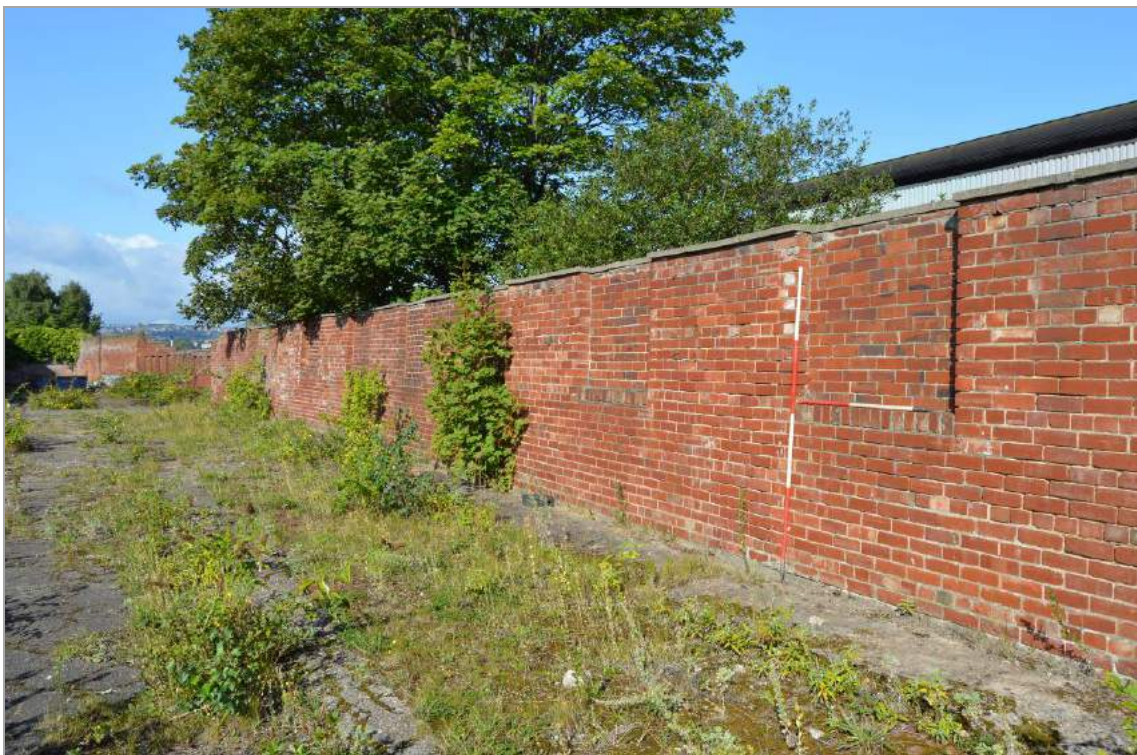
Plate 9: South aspect of Structure 1 (facing north west). Scale 2m.
