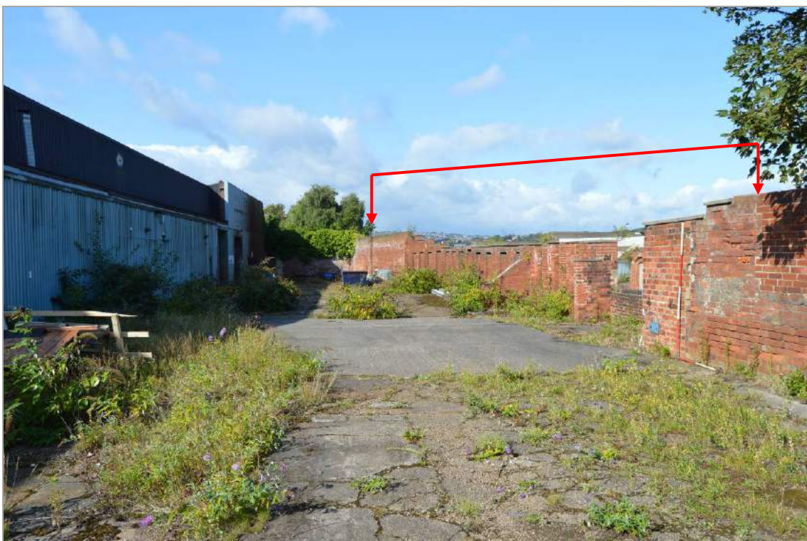
Plate 4: The extent of former structures along the north perimeter of the site (facing west). Scale 2m.
