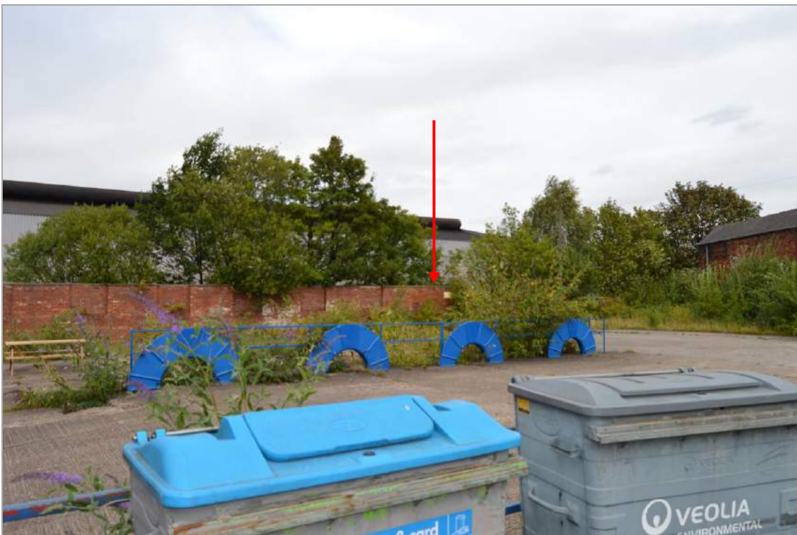
Plate 2: Inside the Pinfold Works site showing part of the structures forming the north perimeter subject to recording.
