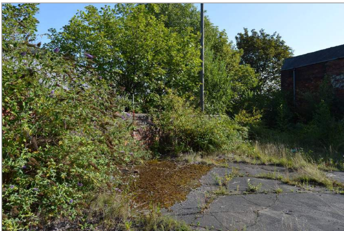
Plate 33: Structure 8 section of perimeter wall. Scale 2m.
