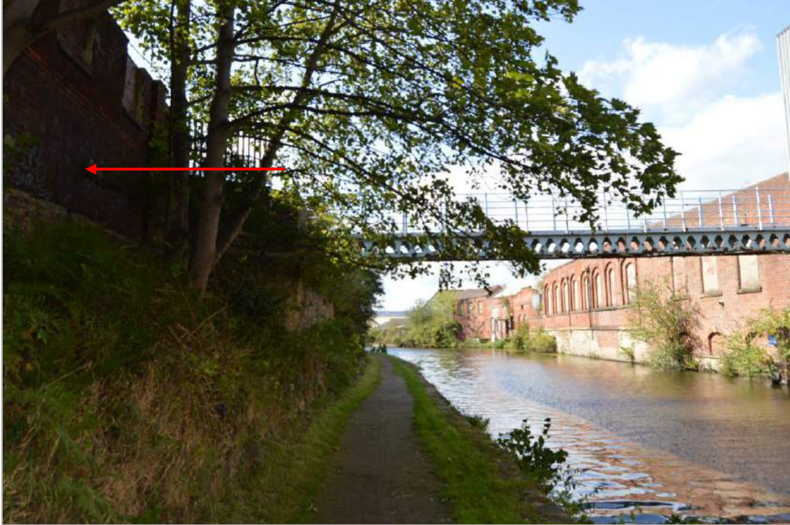
Plate 1: North aspect of the perimeter wall structures (indicated), the canal, towpath and footbridge.
