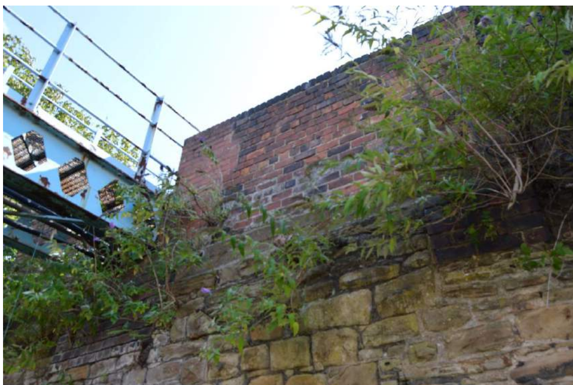
Plate 14: Structure 3, section of parapet walling to west of the footbridge.
