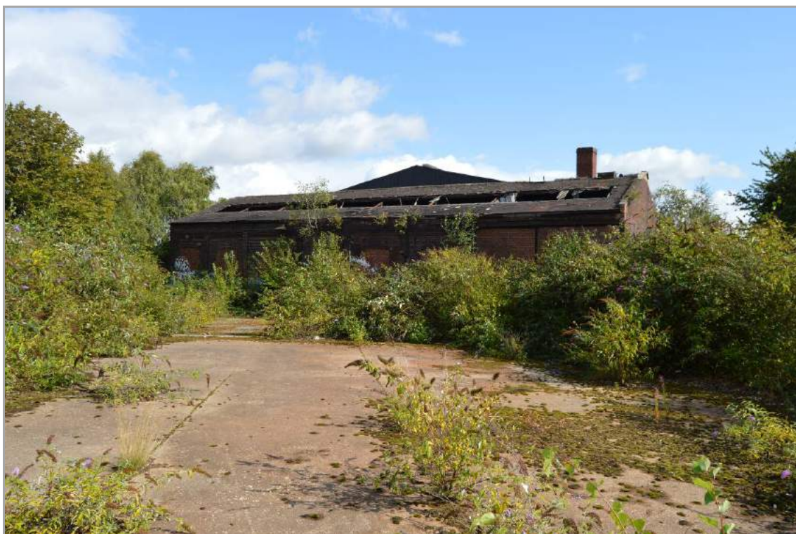
Plate 35: West elevation of Structure 9 (facing east).
