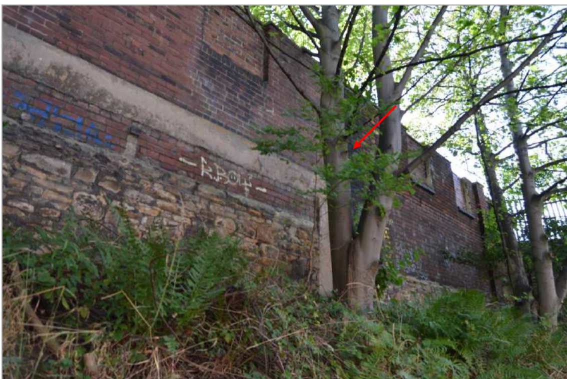
Plate 7: North aspect of Structure 1 (facing south west) with construction break indicated (with structure 2, right).
