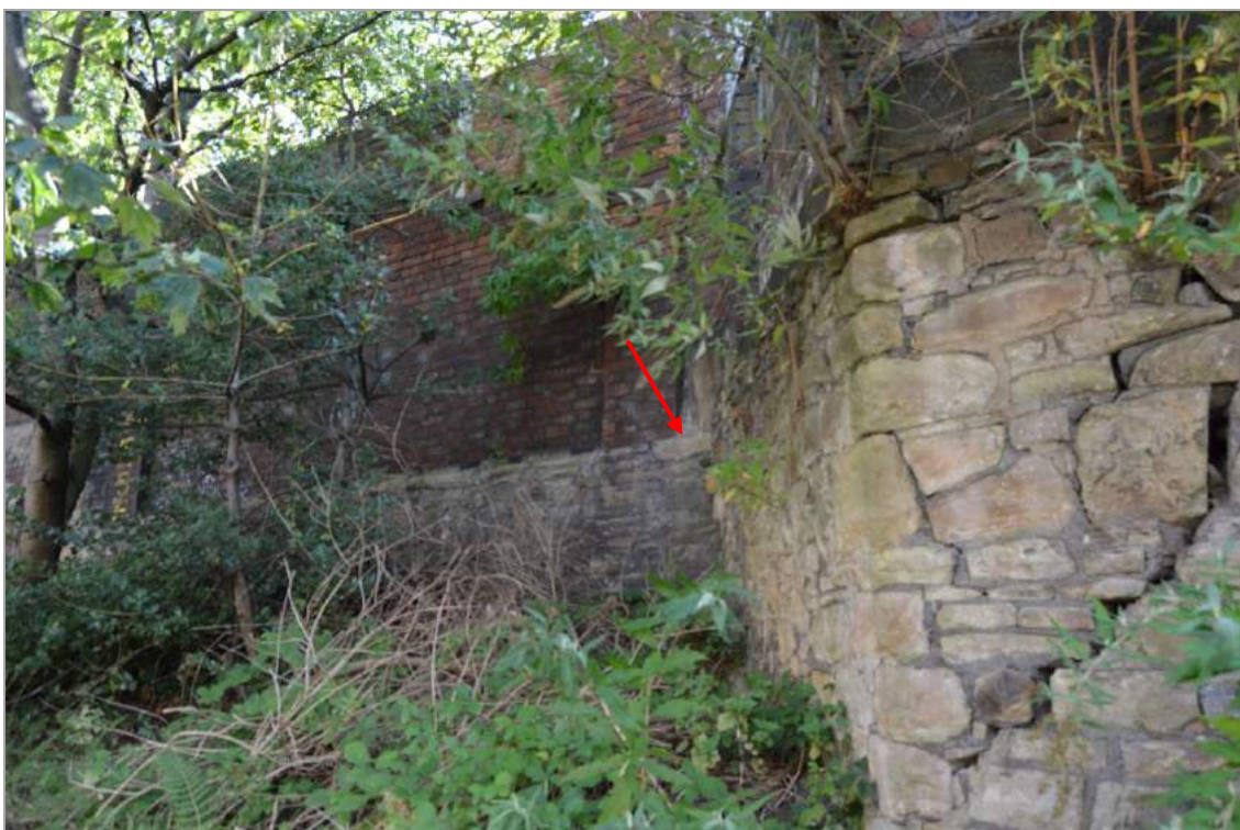
Plate 13: Structure 2 where it meets the projection for the footbridge (facing south).
