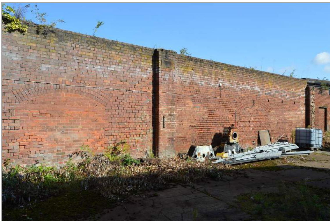
Plate 30: South side of Structure 6 (facing north east). Scale 2m.
