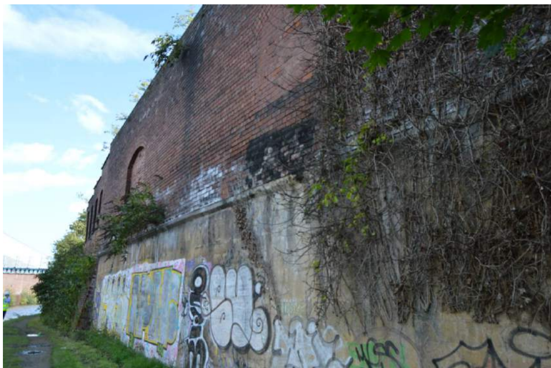
Plate 29: Structure 6, brick built structure over a section of concrete retaining wall.
