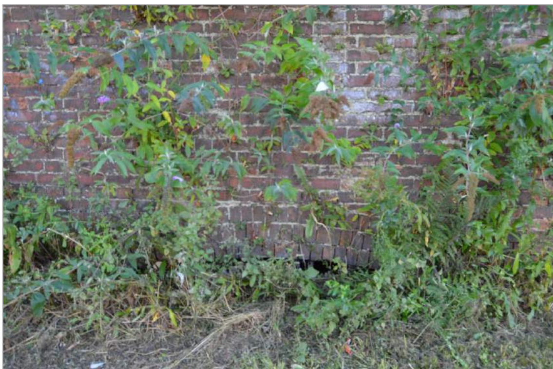
Plate 22: Vaulted arch at tow path level of Structure 5.
