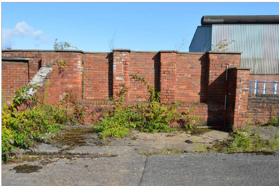
Plate 18: South aspect of Structure 4, facing north. Scale 2m.
