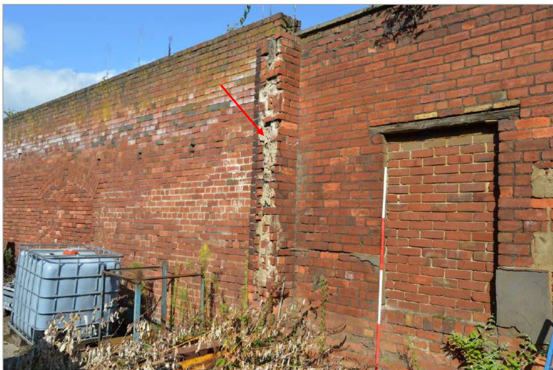
Plate 26: West return (indicated) to south side of Structure 5. Scale 2m.
