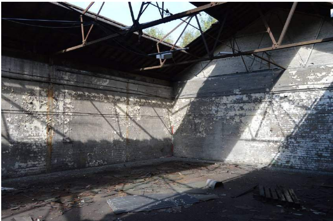
Plate 40: Inside the extension building (facing north west). Scale 2m.
