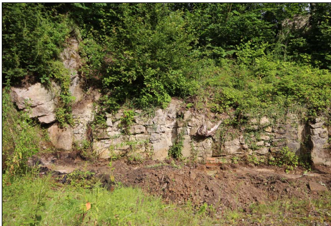
Figure 12: View of the recesses along the north-west retaining wall.
