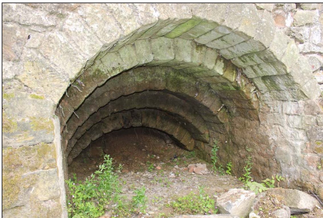
Figure 7: General view of the interior of the archway.
