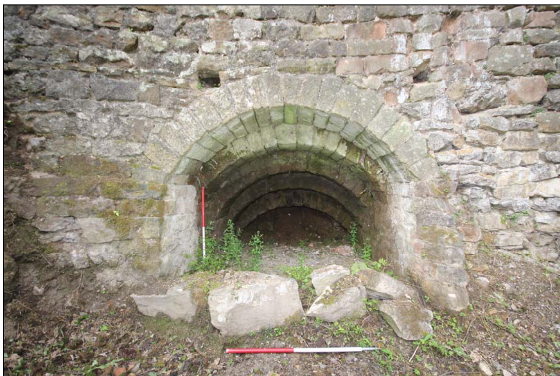
Figure 5: View of the interior of the lime kiln, 2 x 1m scale.
