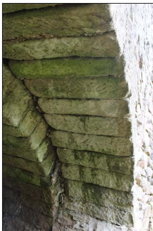
Figure 9: View of the voussoirs forming the archway.
