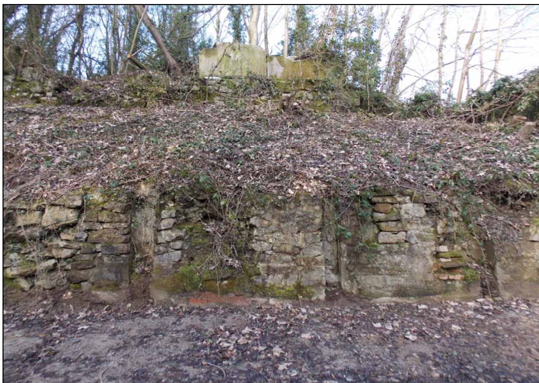
Figure 14: View of the grooves in the north-west retaining wall.
