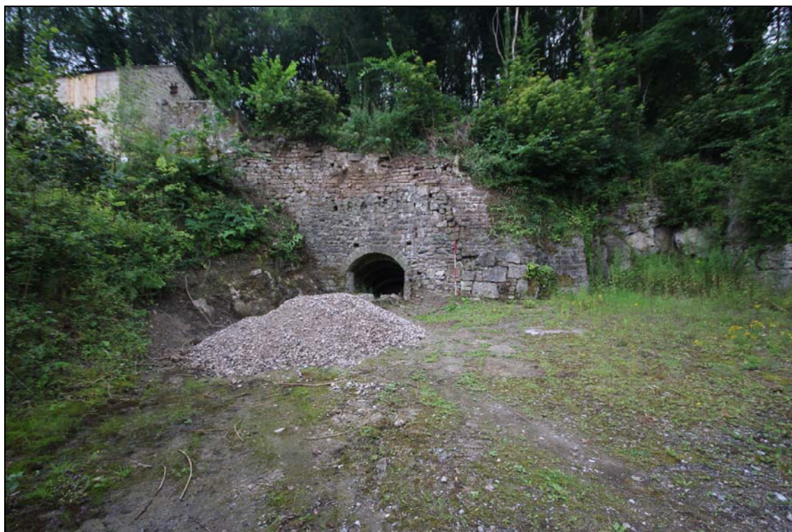
Figure 3: General view of the south west retaining wall, 2m scale.
