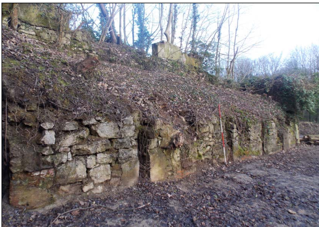
Figure 15: General view of the north-west wall, 2m scale.
