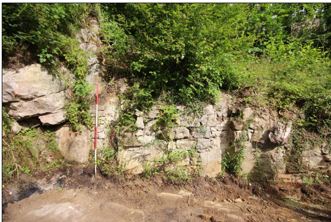
Figure 13: View of the recesses along north-west elevation, 2m scale.
