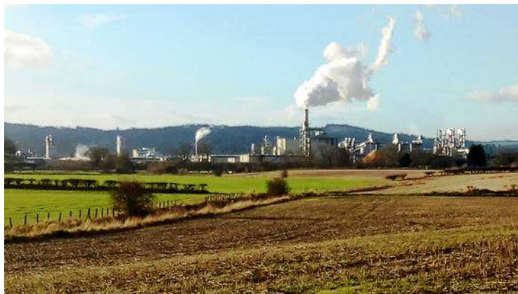
View across the PDA looking west.
