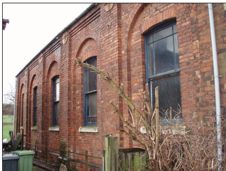
Fig. 57 North exterior elevation of the chapel.
