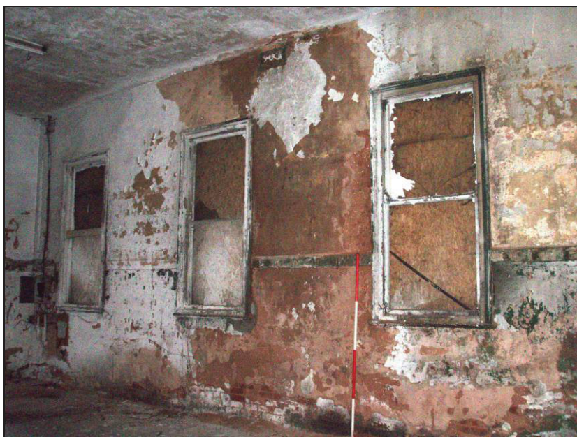
Fig. 19 The west wall of the schoolhouse showing three of the four sash windows. (Scale: 2m)
