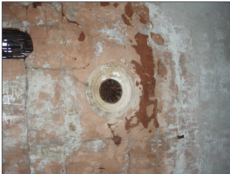
Fig. 23 Moulded air vent on the ceiling in the schoolhouse.
