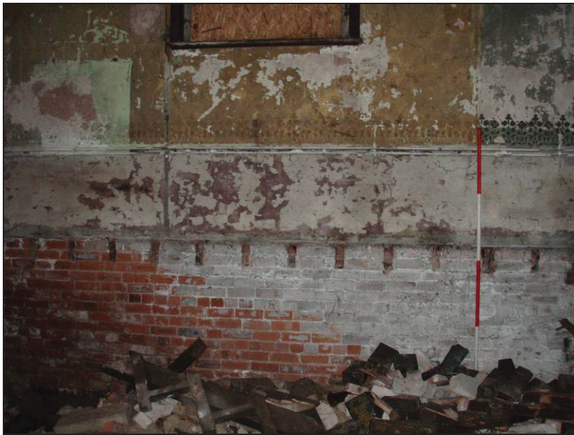
Fig. 17 East wall of the chapel showing the height of the altar and the position of the supporting struts. (Scale: 2m)
