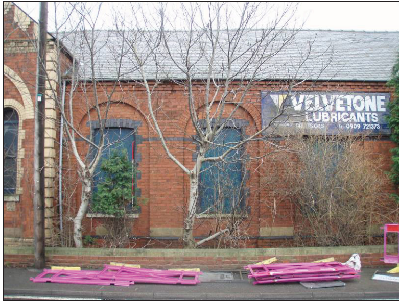
Fig. 59 West exterior elevation of schoolhouse, looking east. (Scale: 2m)
