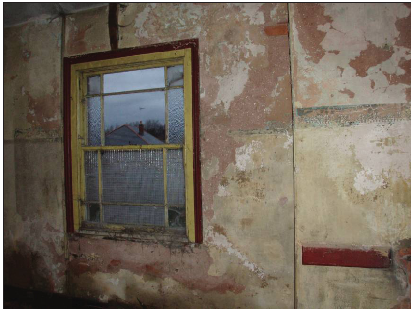
Fig. 34 Sash window on the east wall of the upper storey of the rectory.
