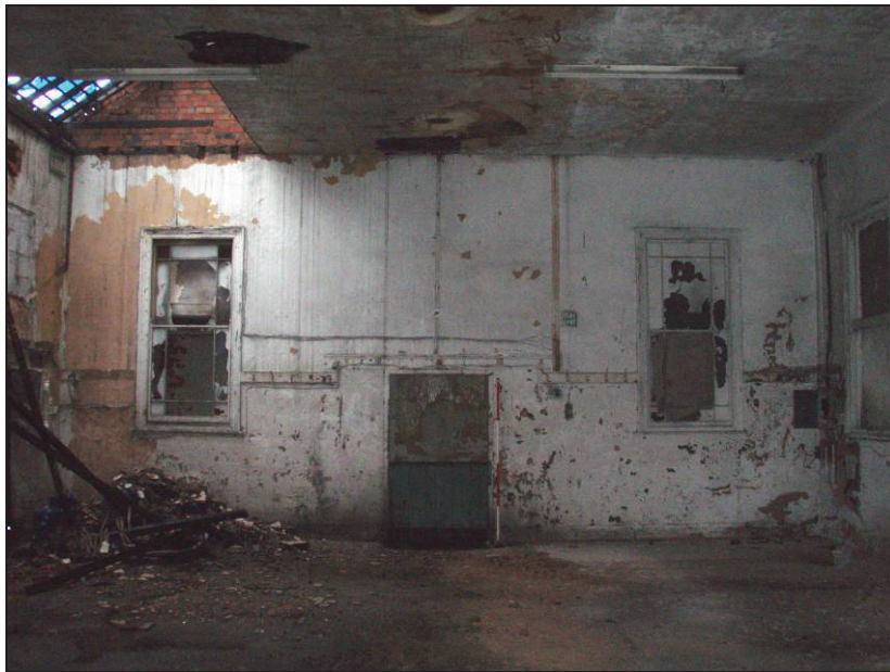
Fig. 22 South wall of the schoolhouse with the entrance at the centre. (Scale: 2m)
