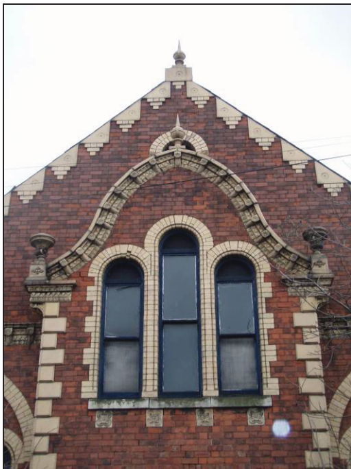
Fig. 53 Entrance porch with arched window.
