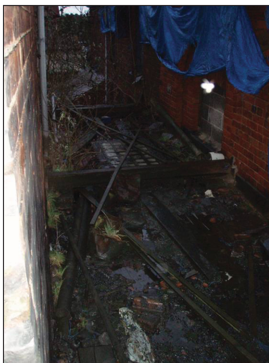
Fig. 37 View from the doorway overlooking the modern passage roof.
