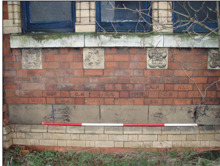
Fig. 55 Carved sandstone blocks below window frames on Chapel entrance. (Scale: 2m)
