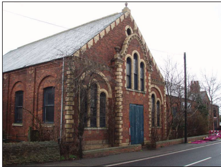
Fig. 49 View of the Chapel, looking south-east. (Scale: 2m)
