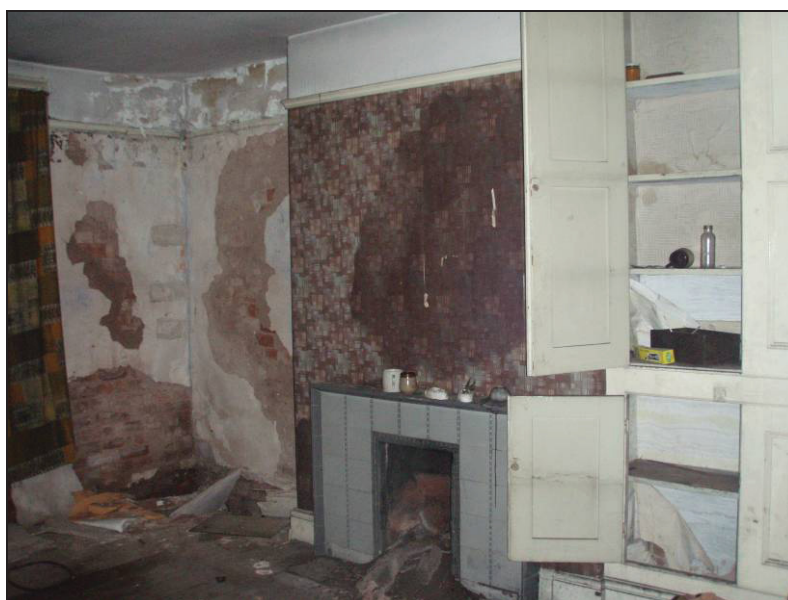
Fig. 45 Room Two of the 1908 extension, looking north-west.
