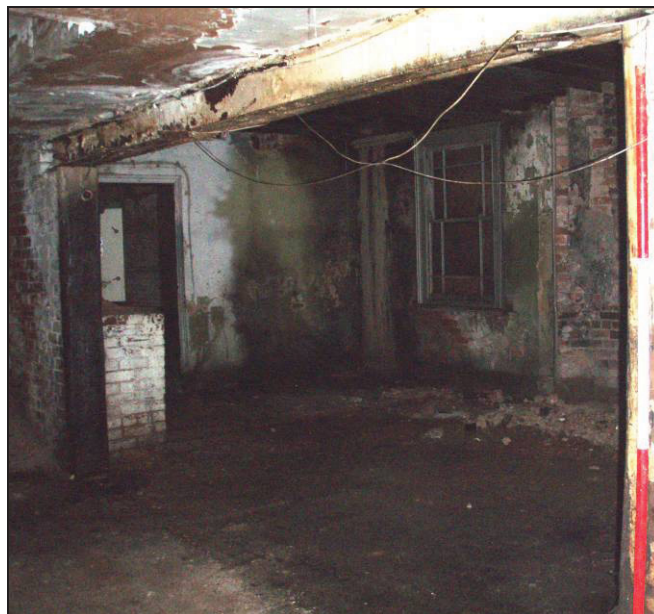
Fig. 30 Modern RSJ entrance to the rectory from the modern passage. (Scale: 0.5m graduations)
