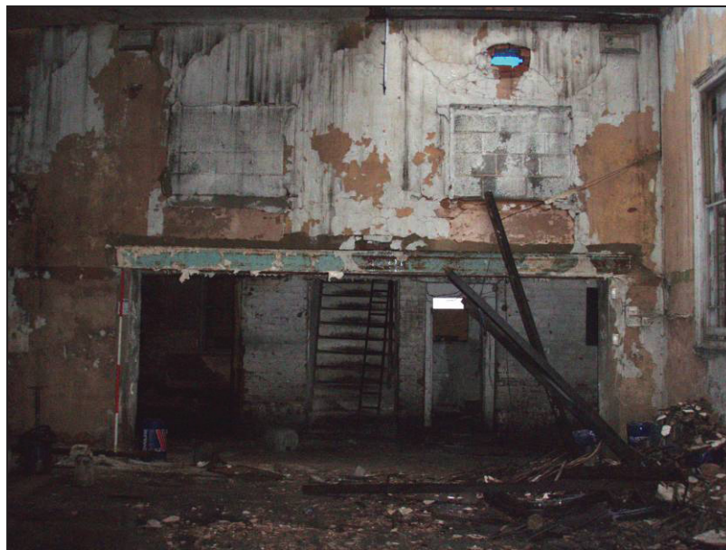
Fig. 21 The east wall of the schoolhouse showing the in-filled windows and the new entrance. (Scale: 2m)
