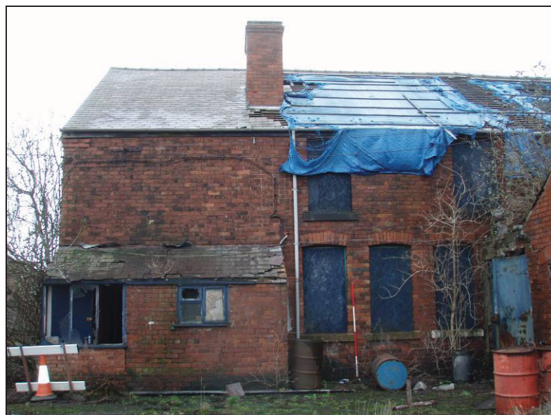
Fig. 68 East elevation of 1908 extension, looking east. (Scale: 2m)
