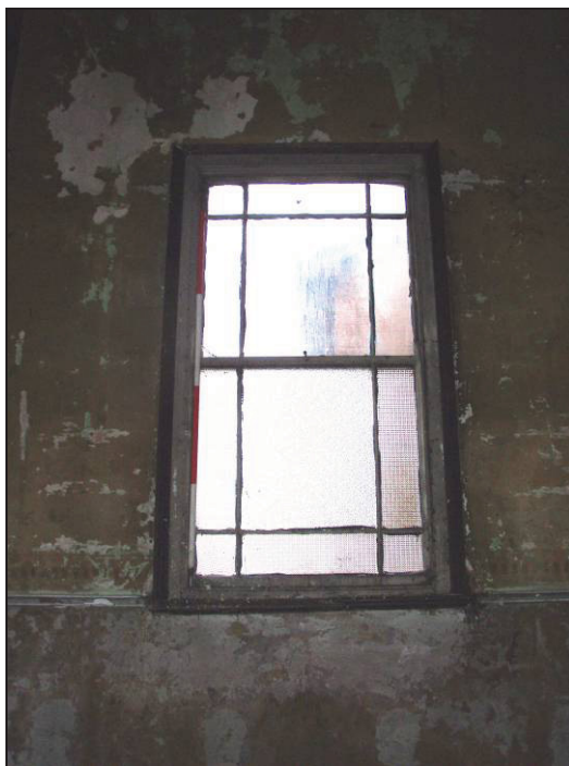
Fig. 9 One of the northern walls rectangular sash windows. (Scale: 2m)
