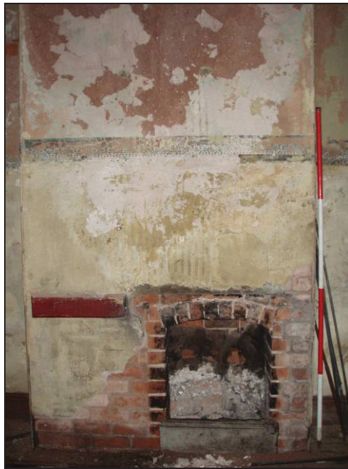
Fig. 33 Fireplace located on the east wall of the upper storey of the rectory. (Scale: 2m)
