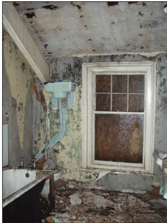
Fig. 48 The bathroom in the 1908 extension.
