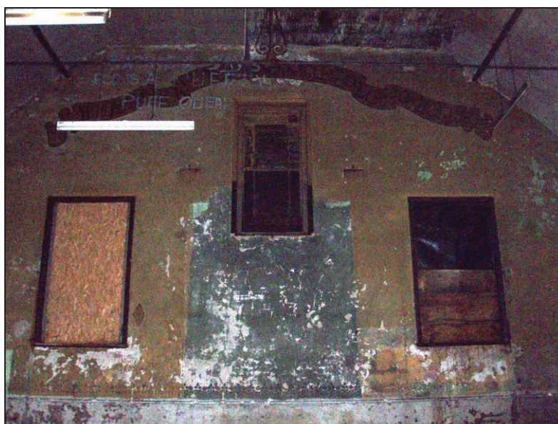
Fig. 10 East wall of the chapel showing the three boarded up windows.
