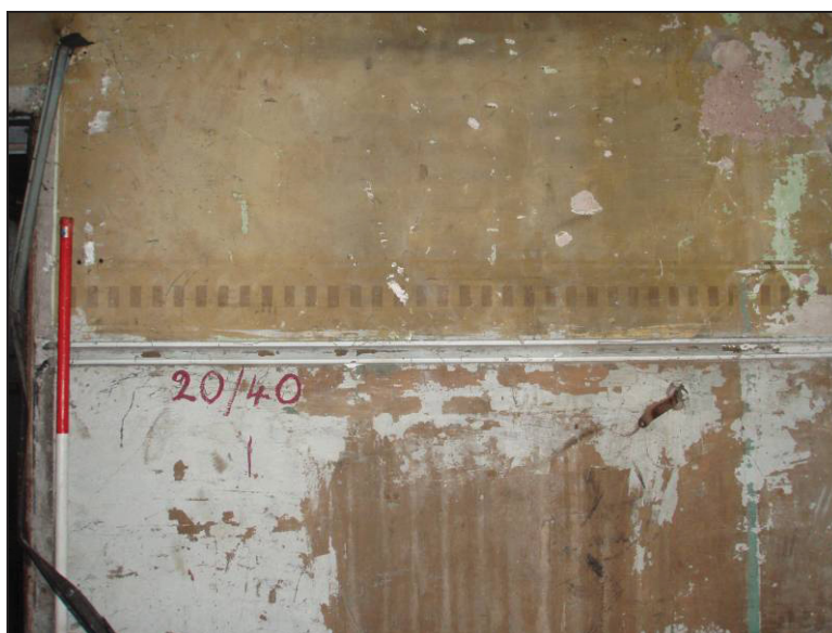
Fig. 15 Remains of the decorated plaster on the south wall. (Scale: 0.5m graduations)
