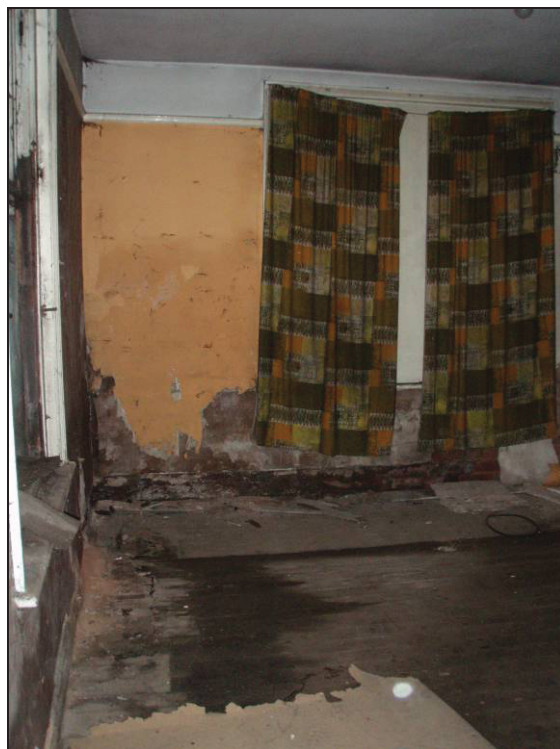
Fig. 44 Room Two of the 1908 extension looking west.
