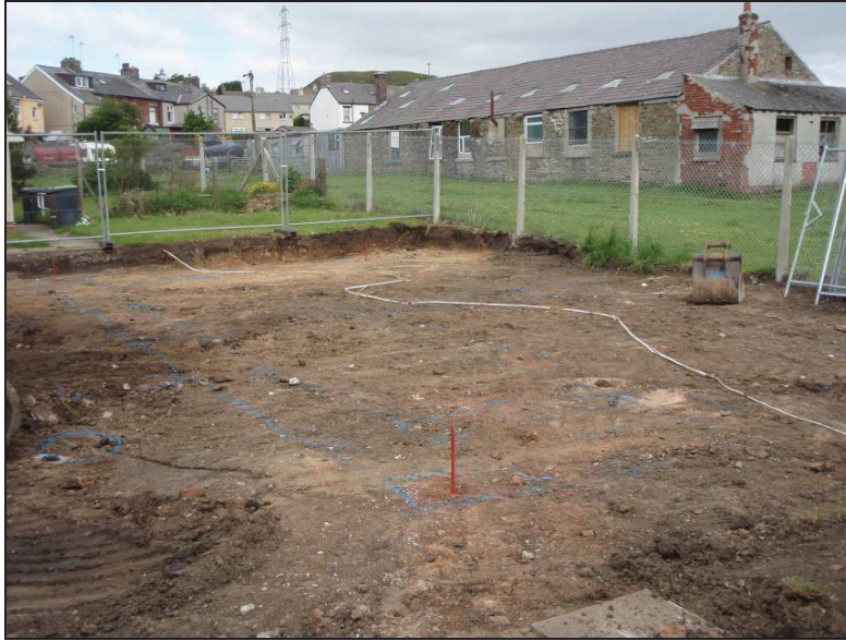
Fig. 8: Foundation trenches marked out. Facing north.
