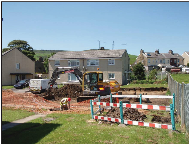
Fig. 7: Ground reduction completed. Facing west.
