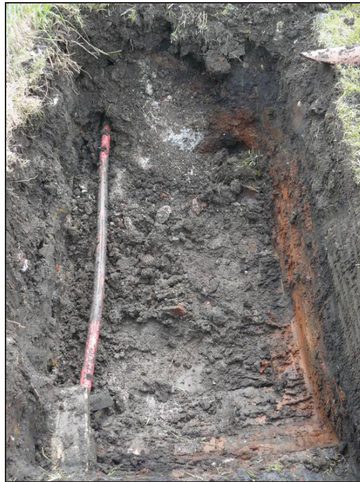
Fig. 3: Pit excavated to expose electric cable. Facing east
