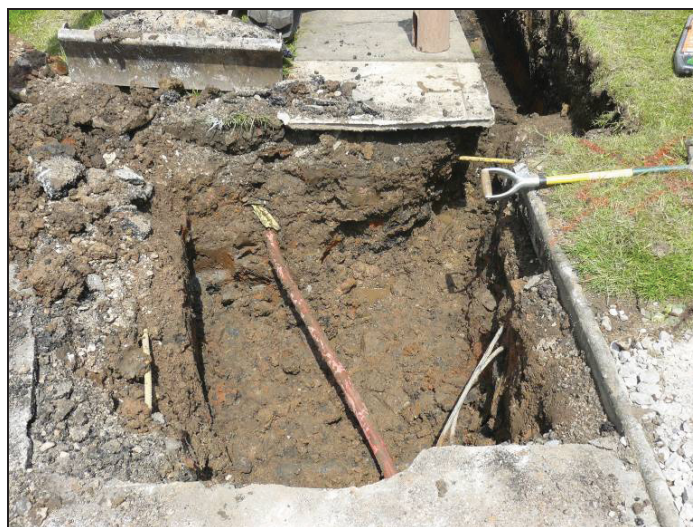
Fig. 5: Southern pit showing utility cables and pipes. Facing north
