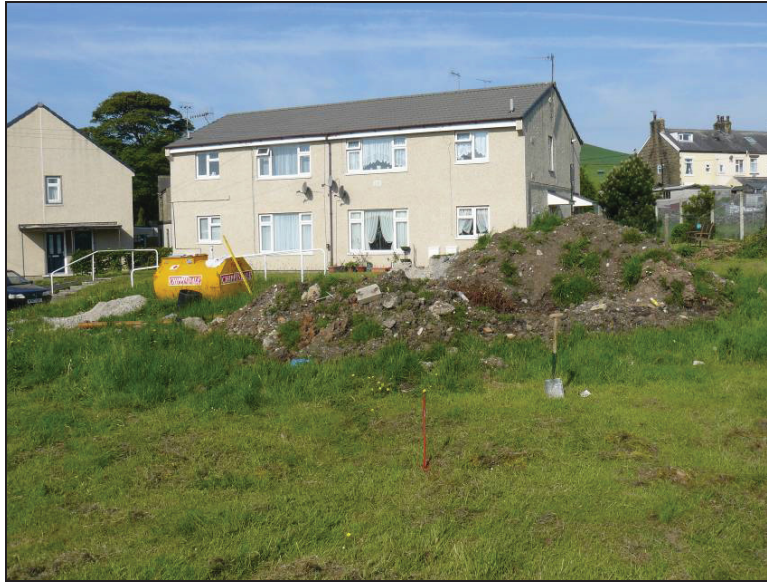
Fig. 6: Pre excavation conditions on site. Facing west.
