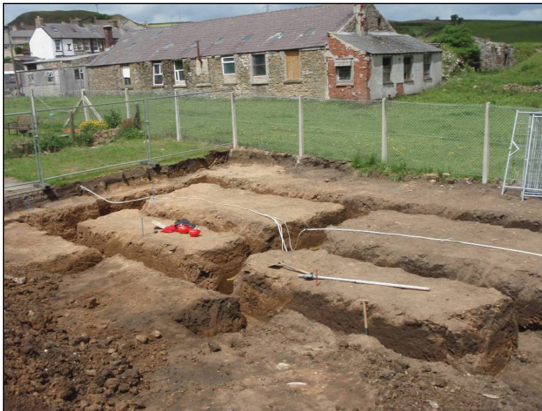
Fig. 9: Completed trenches. Facing north.
