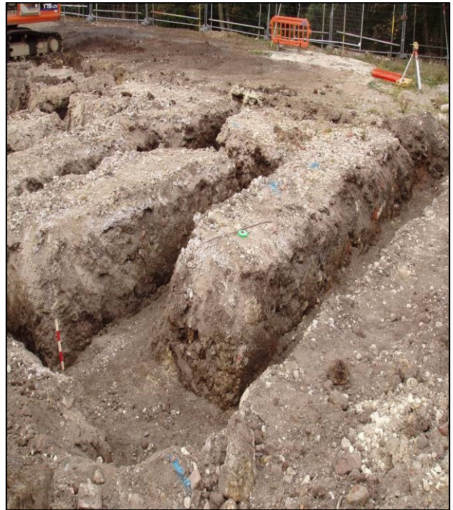
Foundation trenching for Plots 9-12 at Crane Road, Kimberworth, Rotherham.
