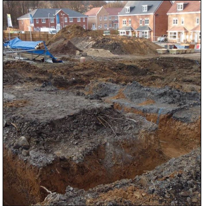
Foundation trenching of Plots 45-48 at Crane Road, Kimberworth, Rotherham.
